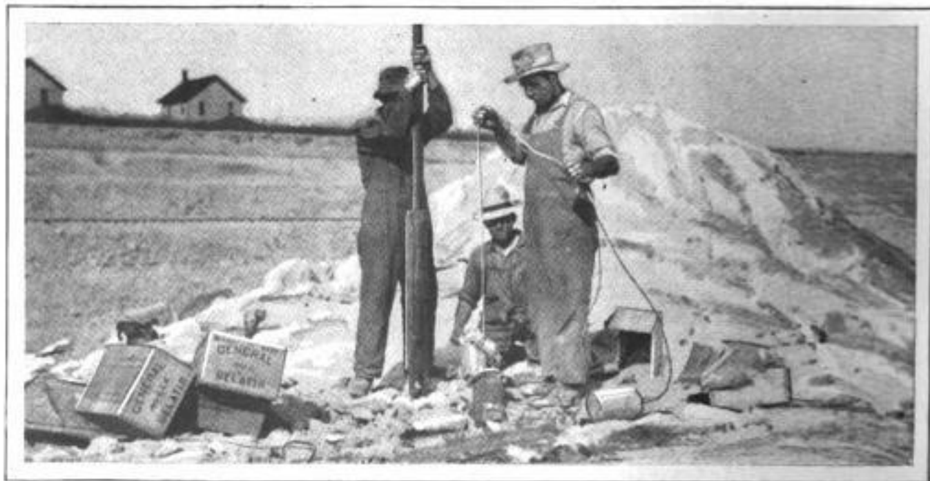
Preparing Heavy Charge of Explosive, Which Is Fired by Electric Current
