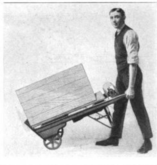
Combination Hand Truck and Scales to Eliminate Disputes over Exact Weights
