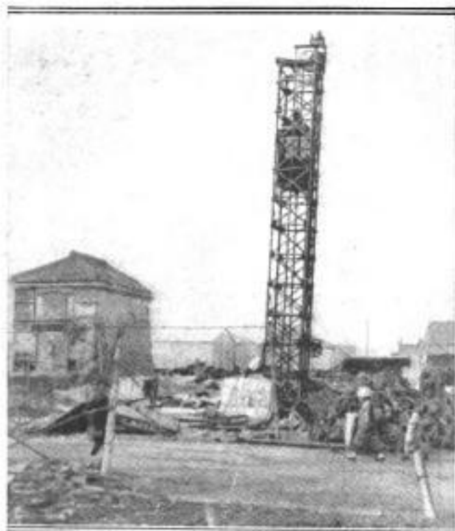
Elevator Shaft that Defied the Earthquake in Japan While Building Housing It Was Destroyed
