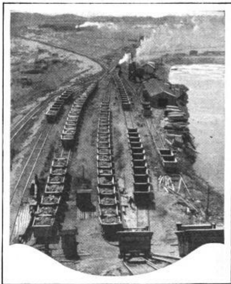
Long Lines of Dunn Cars that Clear Away Debris from Quarry So that Larger S'abs May Easily Be Moved
