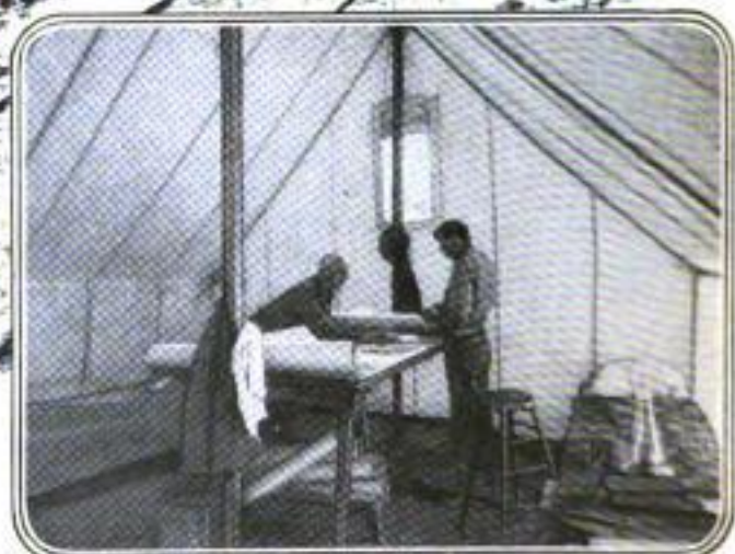
Bridge Builders, Track Layers and Engineers Busily Engaged on Great Railway Extension Program
