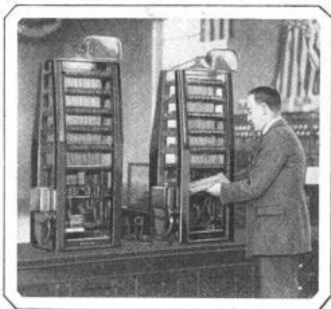
Putting a Fire-Alarm "Record" into Telegraph Instrument that Summons Fighters to Blaze
