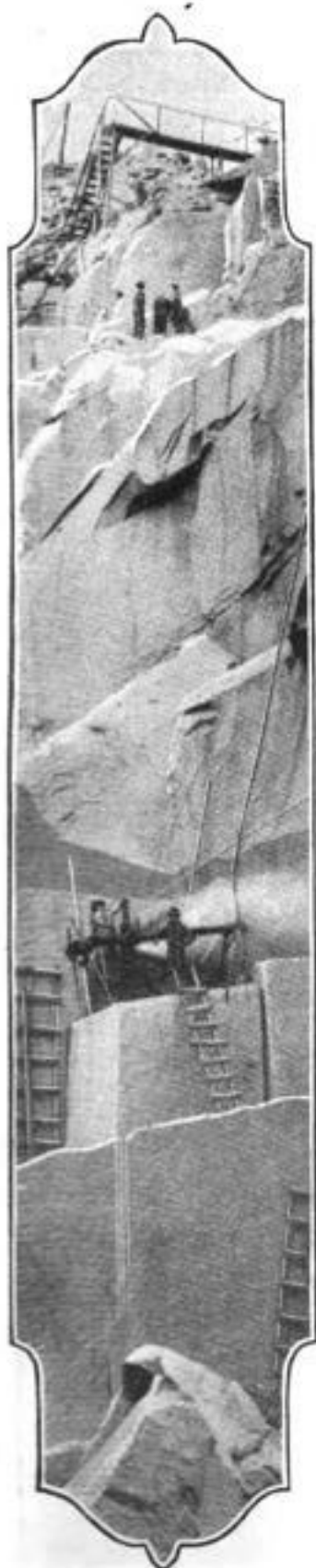
Drill at Work on Narrow Ledge in Granite Quarry
