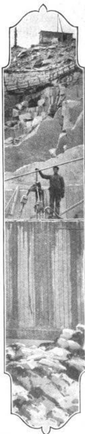
Channels Cut with Air Drills in Side of Cliff
