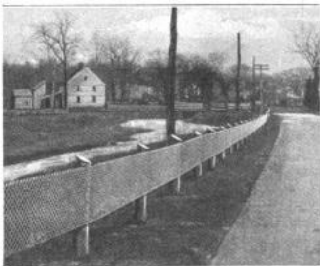
White Wire-Fence Guard at Dangerous Curve to Protect Motorists and Their Cars
