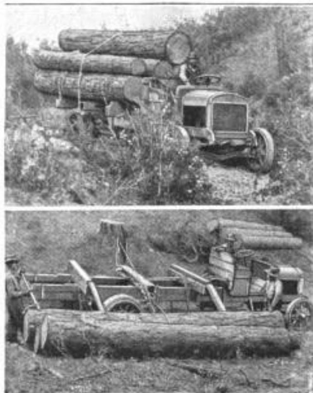
How Logs Are Loaded Directly on Motor Truck with Power Winch for Transportation to Mills
