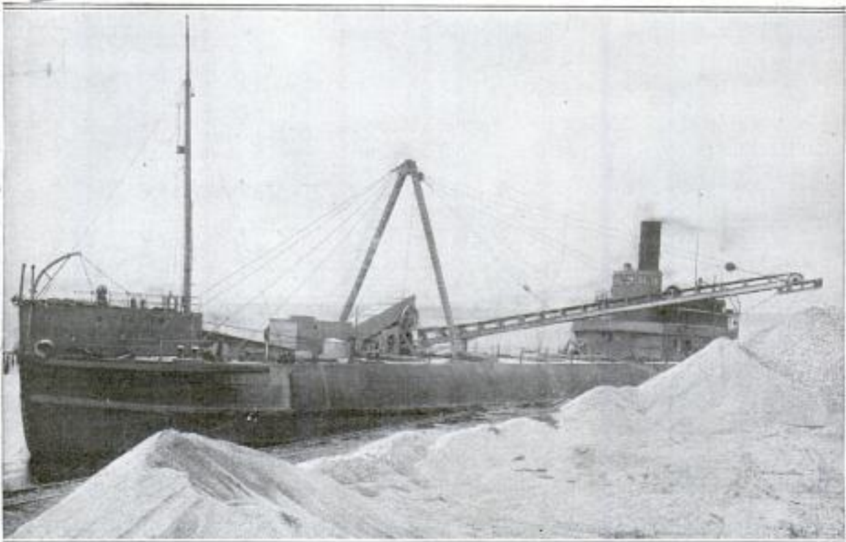
Unloading Cargo of Crushed Stone with Automatic Rigging Installed in an Old Lake Freighter: The Belt Conveyor Placed the Material where It Could Be Reached Easily
