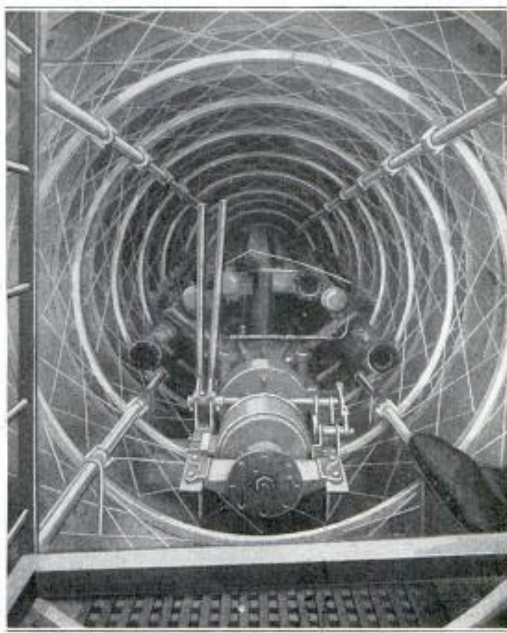
View through the Hull of Speed Boat that is Built over Circular Steel Ribs and is Two Inches Thick
