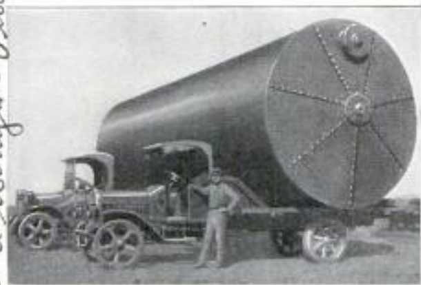
Hauling Huge Tank on Team of Motor Trucks that Were Guided by Arm Signals
