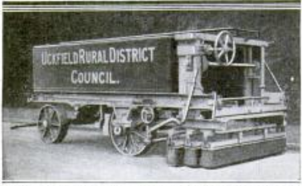
Road Sprayer with Moving Brushes for Spreading Tar or Other Liquids on Highways
