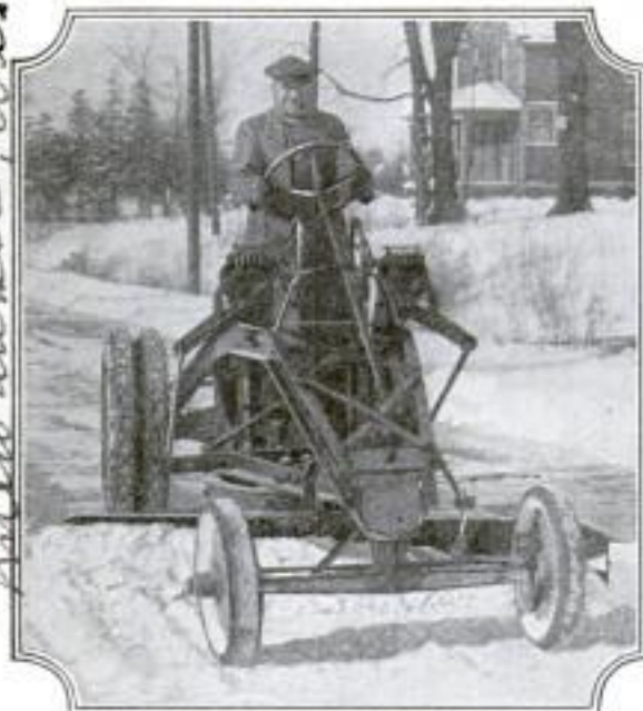
Road Grader Operated by Kerosene Engine that Requires Services of Only One Man
