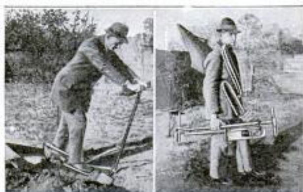
Road Grader Operated by a Long Lever that Requires Services of Only One Man
