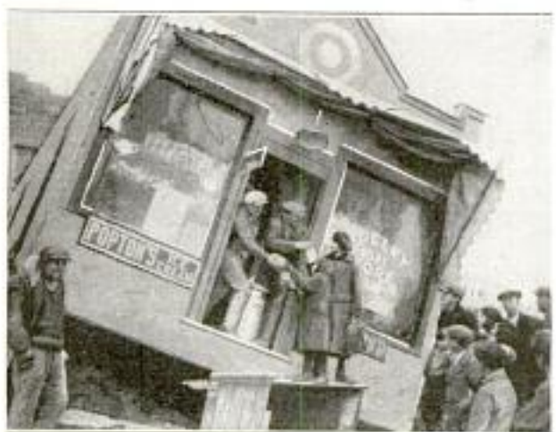
Even Windows Didn't Break When This Concrete Store Building Tilted on Its Side
