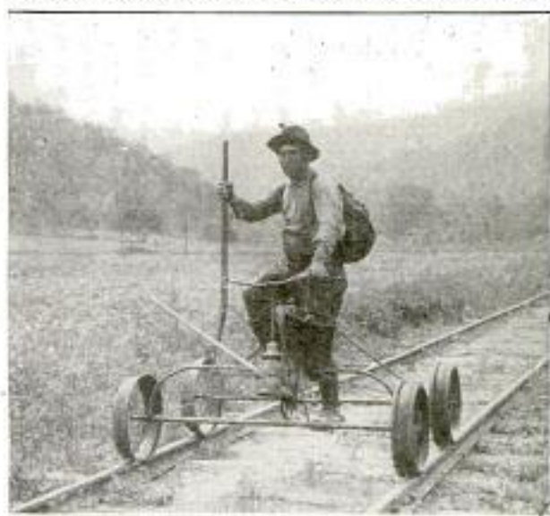
Railroad Bicycle to Enable Members of Forest Patrols to Travel Speedily through Their Areas
