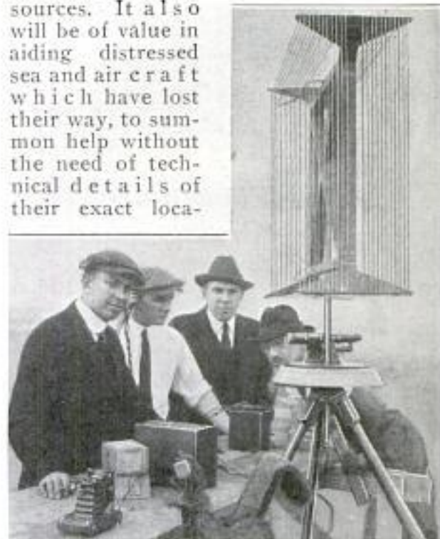
Testing Radio Direction-Finder on Roof of Hangar Occupied by Giant Dirigible, Shenandoah
