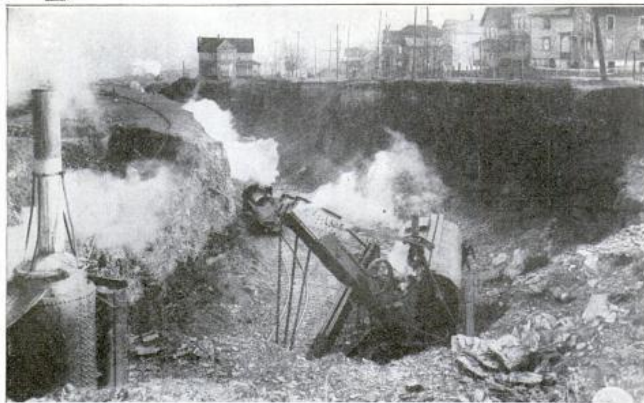
Steam Shovels Tearing Deep, Winding Excavation Along Streets of Residential City where a Rich Vein of Coal Was Discovered to Run Close to Surface of Ground
