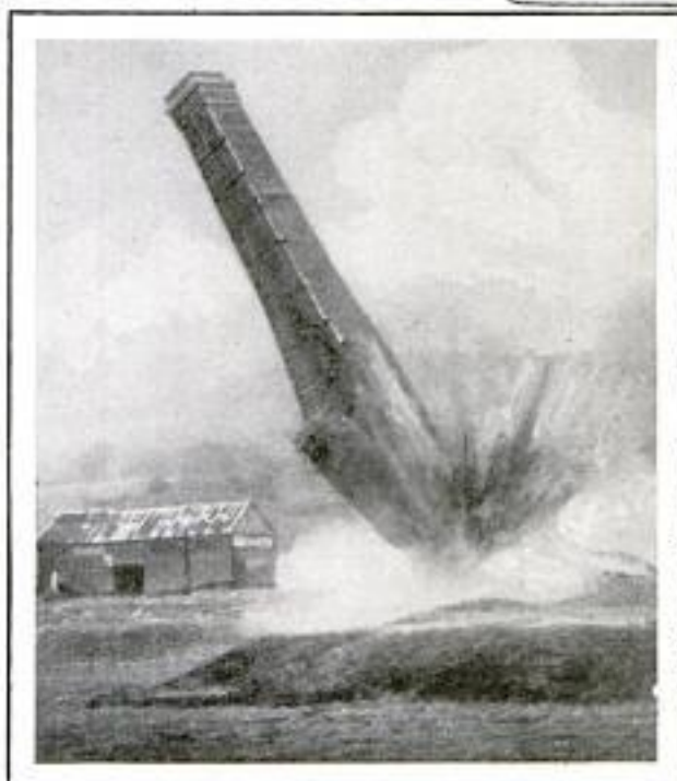
Falling Smokestack with Cracks Showing Clearly the Tremendous Forces Pulling It to the Earth
