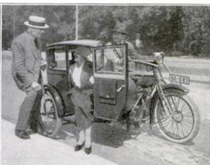
Left, Limousine Side Car that Carries One Passenger, Attached to Motorcycle; and Right, Showing the Wide, Full-Length Door that Makes Entrance and Exit Easy for Occupant
