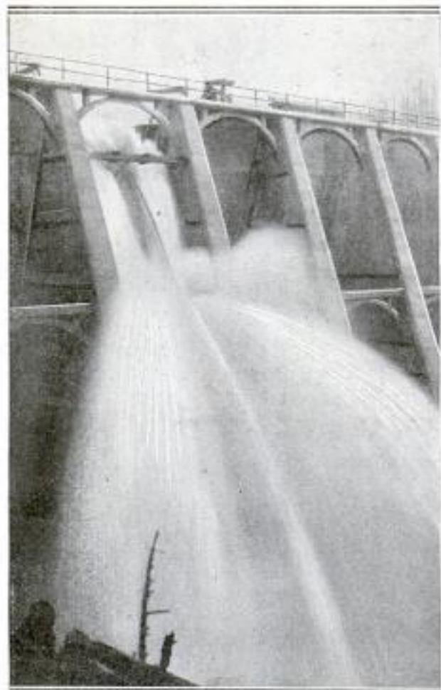
Spillway of High Dam Braced by Concrete Arches that Held Back Heavy Floods
