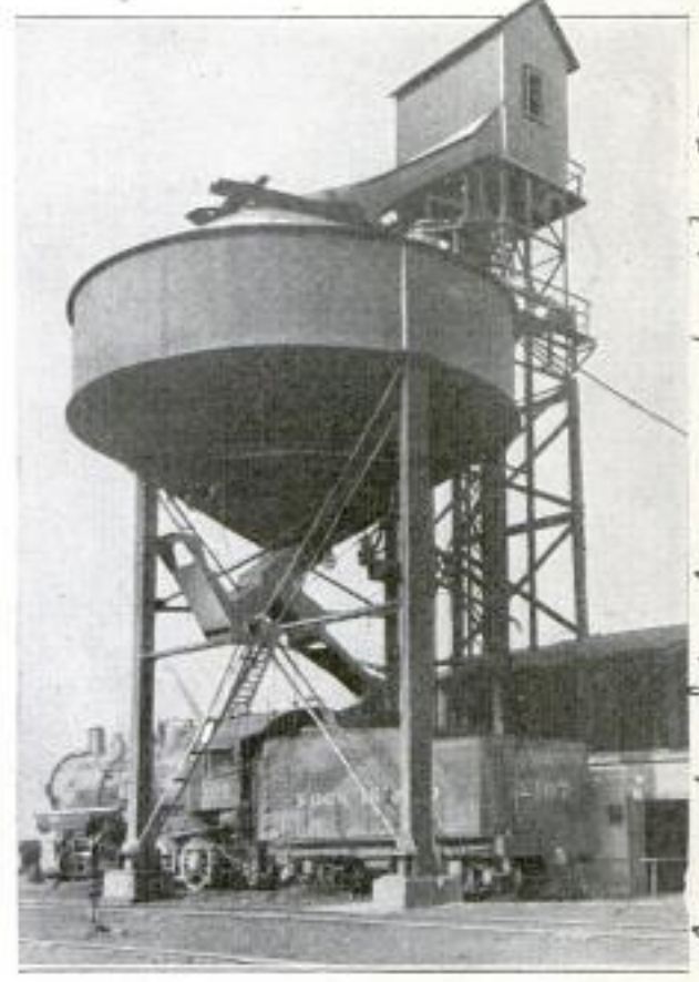
Coal Hopper with Two Chutes that Make Possible Loading Two Tenders at Once
