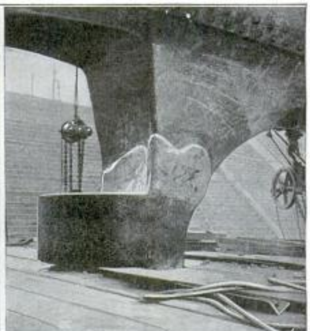
Greatest Marine Weld on Record: Sternpost Stronger than Before the Break Occurred
