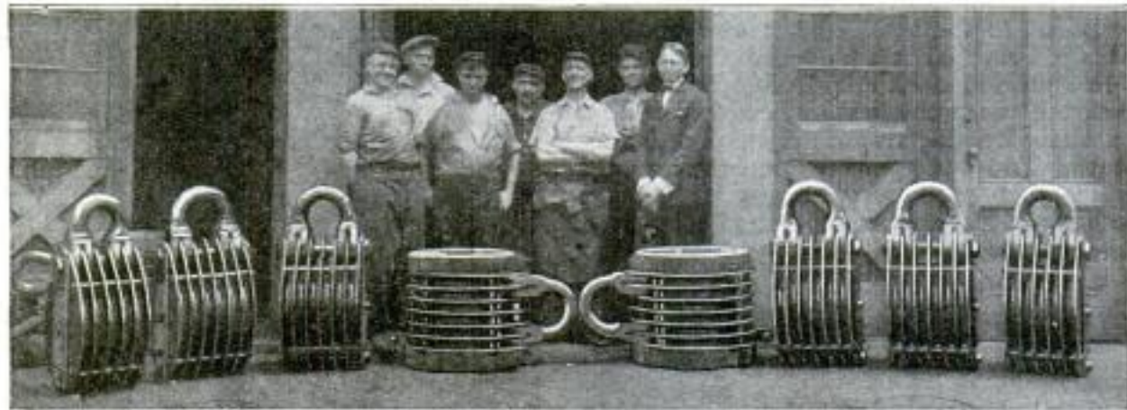
Giant Tackle Blocks Made by Hand to Move Huge Steel Girders Used in the Construction of a Thirty-Two Story Office Building
