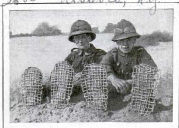
Wire-Mesh "Sand Shoes" that Make Desert Marching Easier by Lessening Strain
