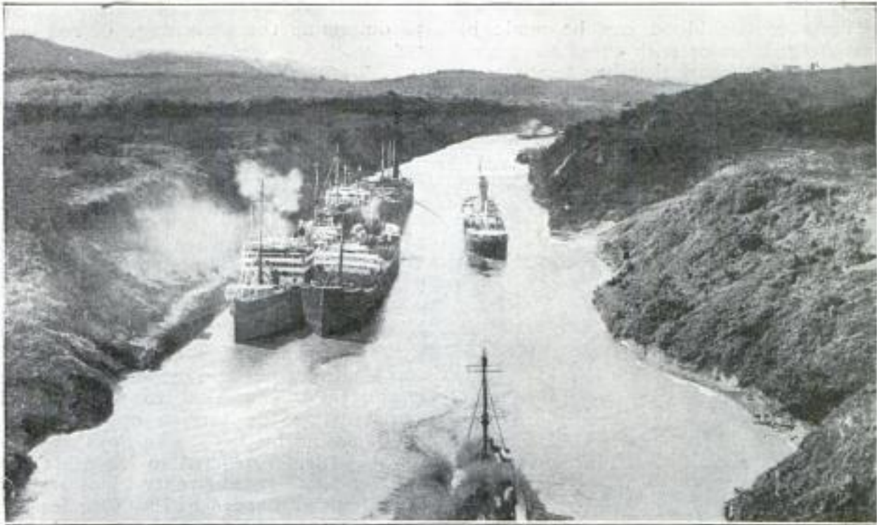
South-Bound Ships Waiting for Dredges While North-Bound Steamers Proceed, After a Minor "Slide" in the Panama Canal Blocked Part of the Passage
