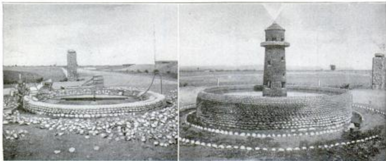
Miniature Lighthouse and Fountain Built of Cobblestones by the Convicts in a Western Prison Who Used a Revolving Wooden Frame to Make a Perfect Circle
