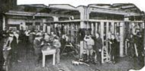
Students Practicing House-wiring In Skeleton Houses
