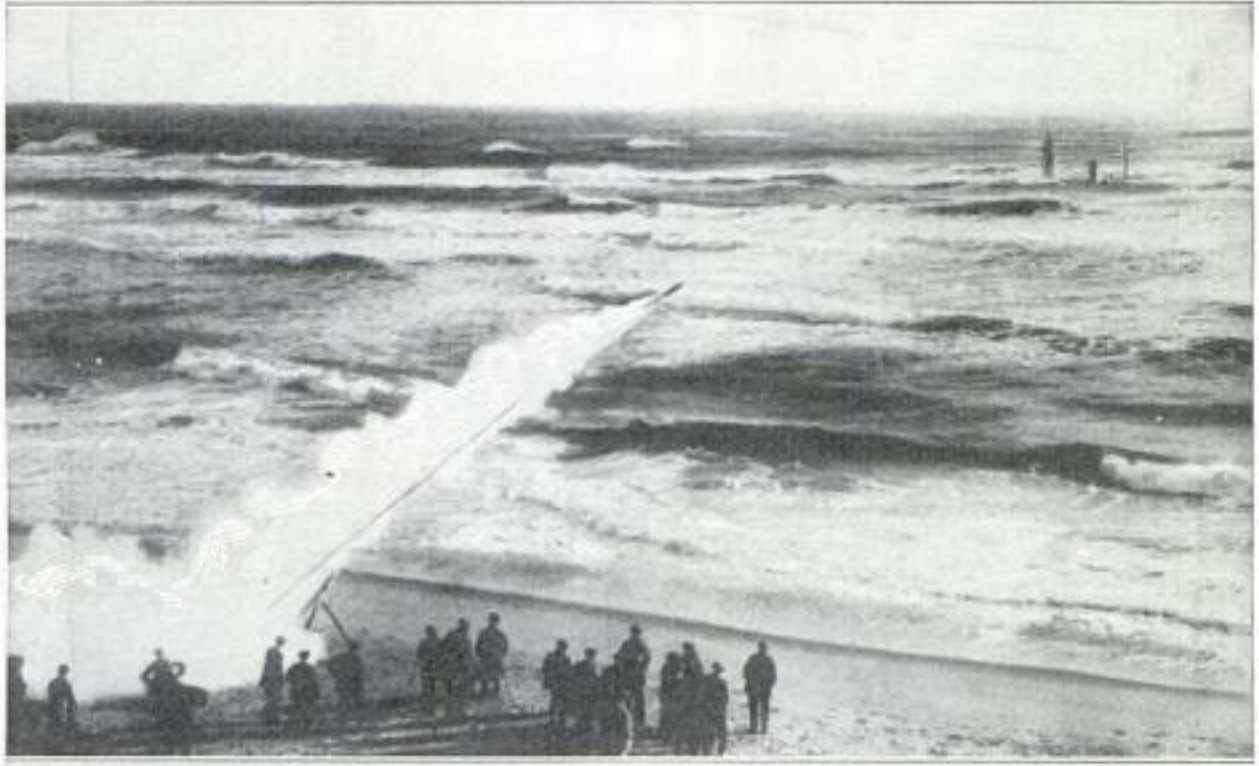
Rocket Being Used to Carry Life Saver's Line to Wrecked Ship: This Method Has Been Adopted to Do Away with the Cannon Formerly Employed for the Same Purpose
