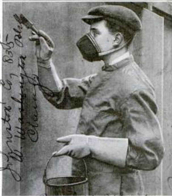
Protecting Gloves and Mask for Use of Painters to Guard Them from Lead Poison
