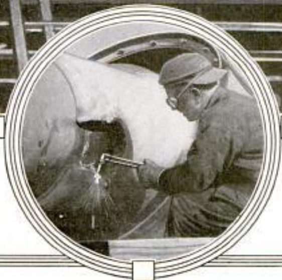
—:— The United States Steamship "South Dakota" under construction, but which will be junked
