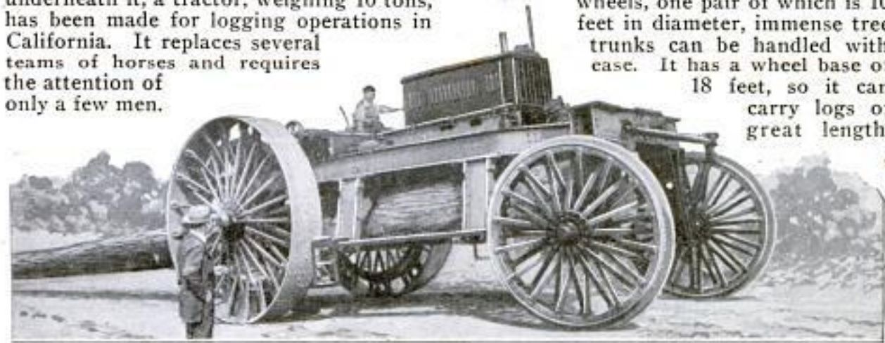
Mammoth Tractor Built for Logging Operations, so Huge that Automobile Can Pass between Its Wheels, One Pair of which is 10 Feet in Diameter
