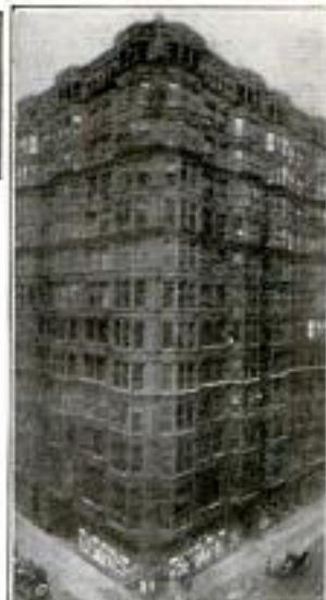
Our Chicago Office 1114 Tacoma Building
