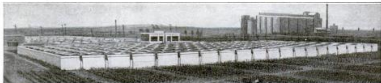
Experimental Farm, Surrounding Sewage Plant where Fertilizer Undergoes Tests in Actual Use with Various Crops: Its Effect on Each Is Carefully Studied and Compared with Other Materials
