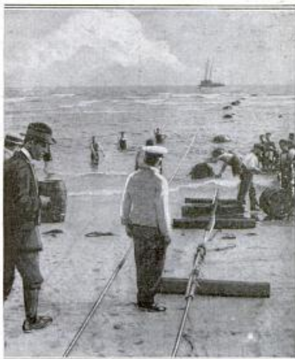
Hauling Shore End of Cable through the Surf and onto the Beach from a Distant Ship
