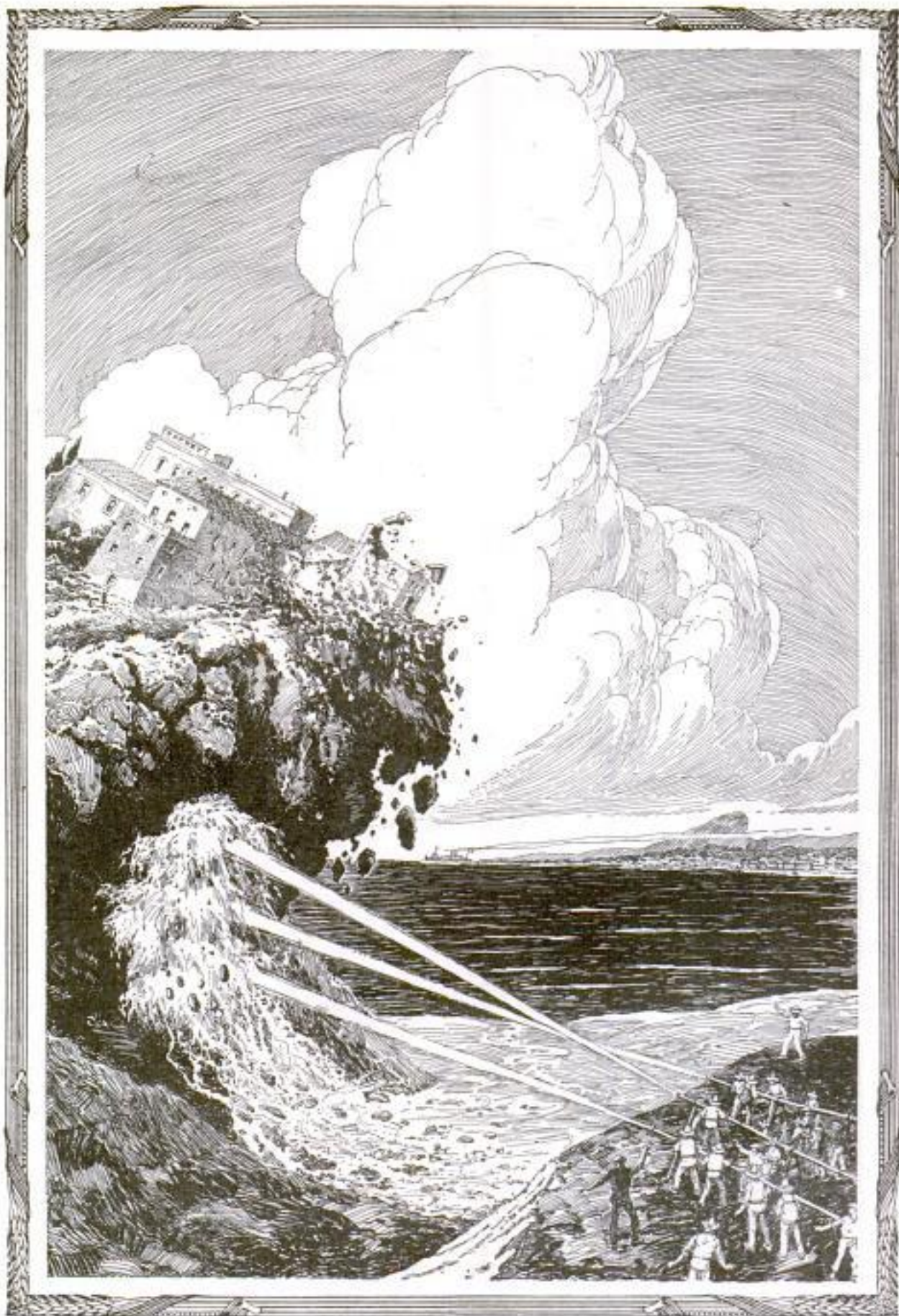
Washing a Mountain into the Sea to Make an Extension of New Land for a South American City's Business District: Seven Million Cubic Yards of Ground Were Transferred
