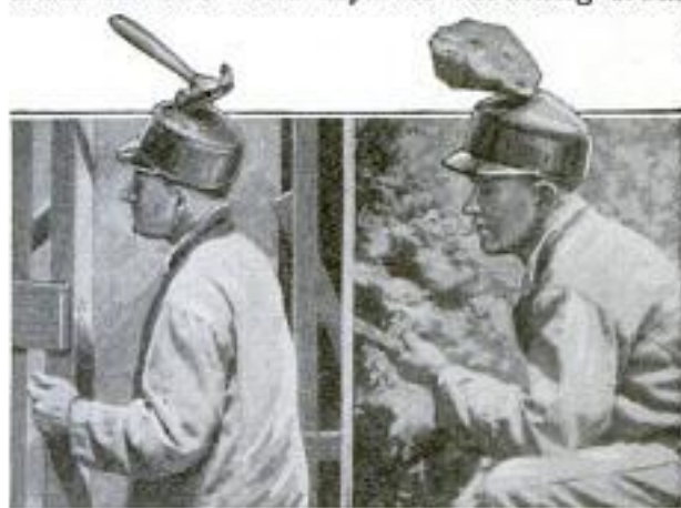
Wearing Hard Hats, These Two Workmen Escaped Possible Serious Injury from Falling Objects
