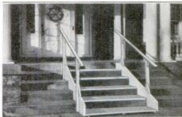
A Portable Step and Rail for the Porch Prevents Accidents Due to Slippery Steps
