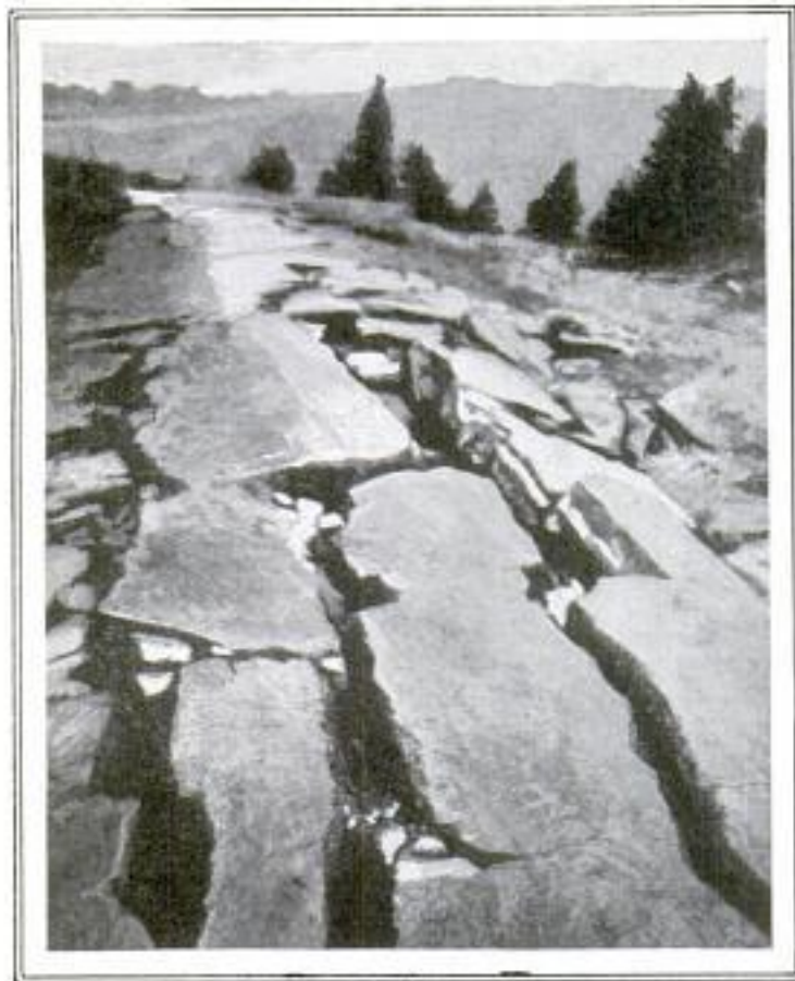
Modern Roadways Were Reduced to Bits by Yawning Gorges that Opened When the Ground Rose Up
