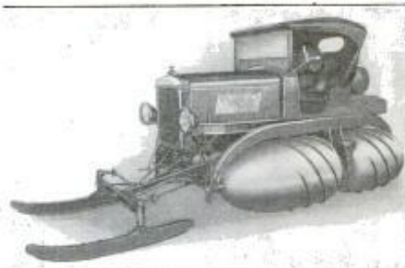
Courtesy Engineering & Mining Journal Egg-Shaped "Wheels" on Tractor for Use over Snow or Ice
