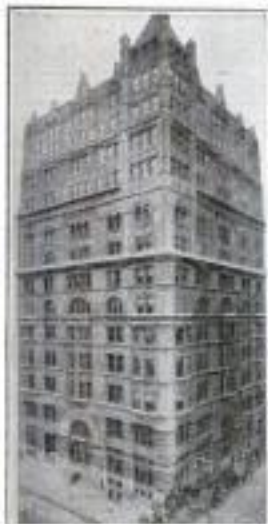
Our Philadelphia Office 714-15 Liberty Bldg.
