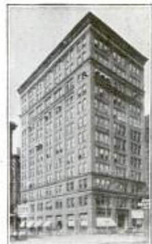
Our Pittsburgh Office 514 Empire Building
