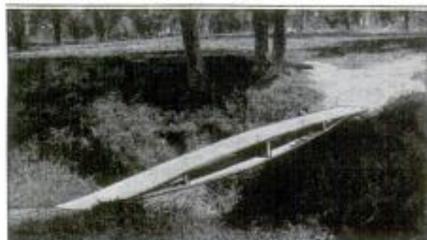
A Strong and Simple Bridge Made from Two Planks, Used across a Gully on a Western Golf Course
