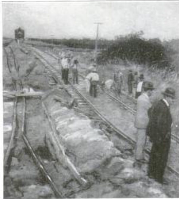
Instead of Repairing Damaged Roadbeds, New Ones Were Built of Inferior Material Alongside Them
