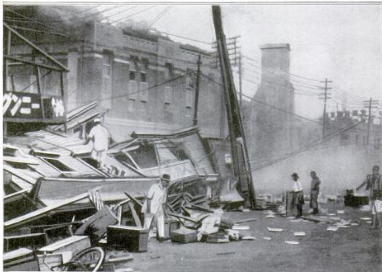
Abandonment of the Old Method of Bamboo Construction Was Blamed for the Collapse of Many Buildings that Buried the Occupants Beneath Tons of Bricks and Timbers
