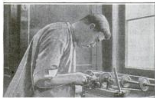
Sawing Faulty Stones into Pieces
