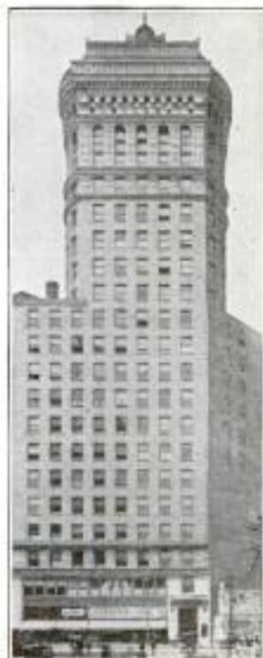
Our San Francisco Office 1010 Hobart Building
