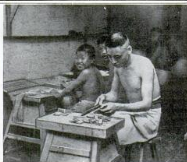
Fitting the Blocks with Bamboo Backs
