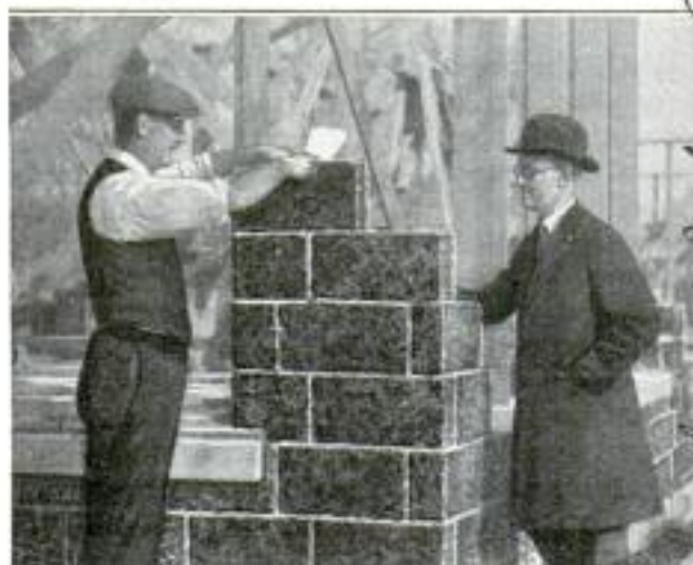
Latest Form of Cinder Building Blocks Being Laid in a Model Cottage
