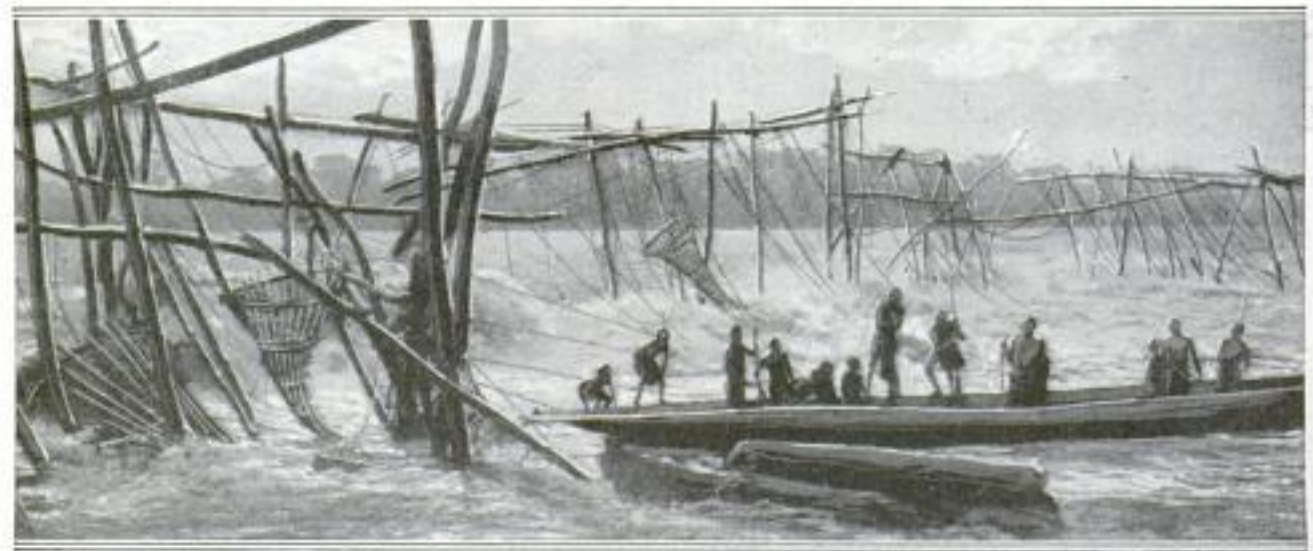
As a Result of Ages of Experience, African Fishermen Fastened Cone-Shaped Nets on a Frame of Tree Trunks and Branches Built Across a Swift River
