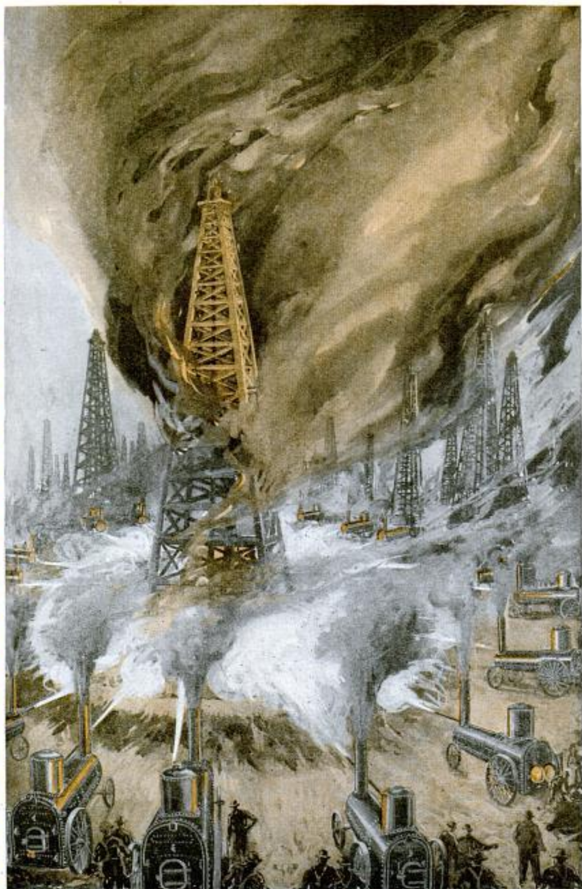
How High Pressure Steam from Boilers is Used to Smother a Burning Oil Gusher, about Which a Wall of Sand Has Been Built to Dam the Flaming Flood
