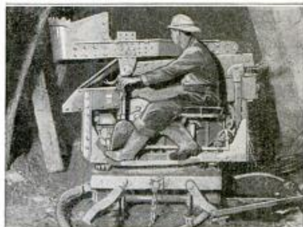
View of Underground Shovel Swinging in Drift, Showing Small Clearance Required
