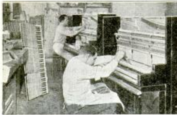
Above, Experts Placing Strings and Putting Finishing Touches on Piano; Left, Workmen Installing the Keyboard and Action; Right, Fashioning and Gluing Together Parts of the Case
