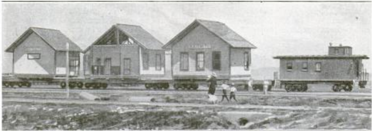
Railroad Station from Abandoned Town Being Transported to New Location, Where It Will Remain until Another Shift of Population may Cause It to be Moved Again
