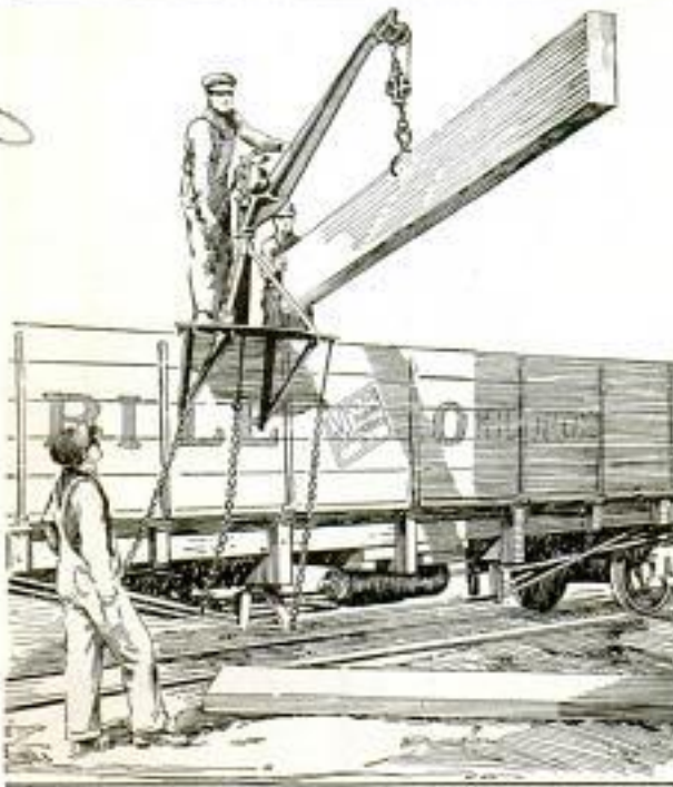
One-Man Portable Derrick Unloading Heavy Beams from Gondola
