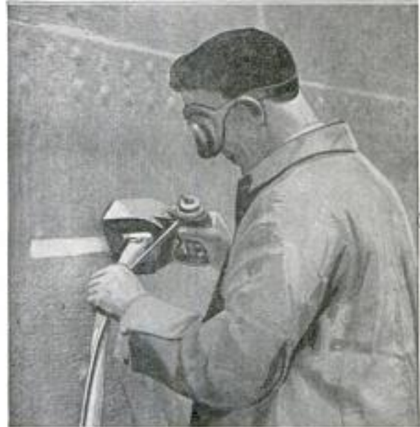
Scraping Rust-Coated Steel Plates of Ship's Hull with Machine Operated by Electricity
