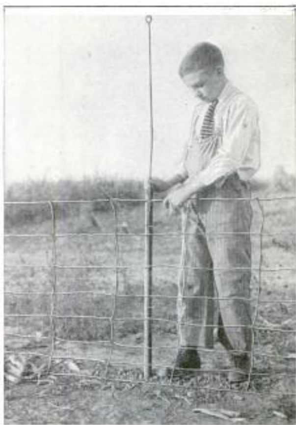
Temporary Wire Fence That can be Set Up or Taken Down in a Very Short Time
