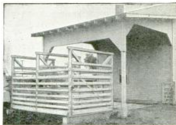
Convenient Live-Stock Frame for Farm Scales: It is Mounted on Rollers Running on Tracks
