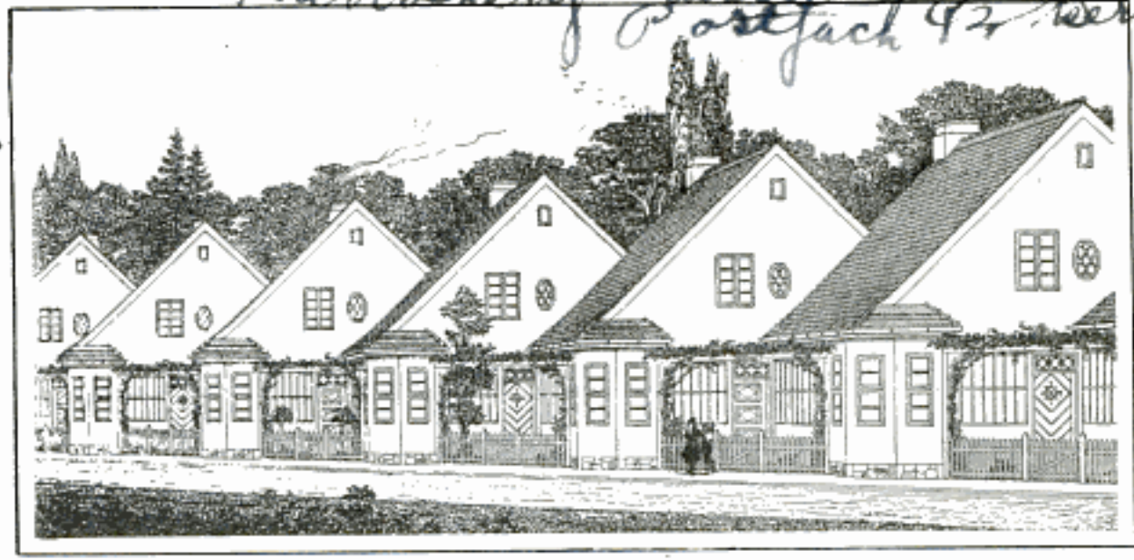
Small Dwellings Set at Angle to the Street to Give More Light and Air and Greater Security against Intrusion: Heat and Electricity are Supplied from a Central Plant
