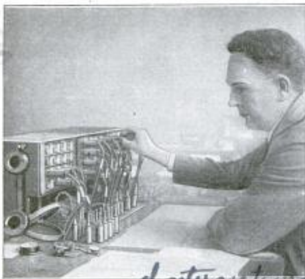
Switchboard Used by Naval Radio Operators to "Plug In" on Different Aerials
