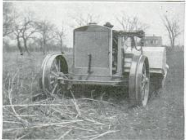
Rotary Plow Going over Field Covered with Sunflower Stalks 10 Feet Long
