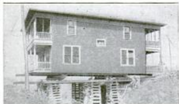
Left: View of Two-Story House being Moved across 20-Foot Cañonlike Street, Showing Arrangement of Cribs. Right: Safely Across; Movers Bridged the Gap in Two Days without Hindering Traffic
