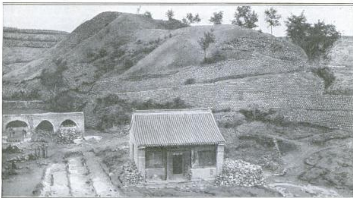
An Impressive Example of the Extent to Which the Small Jars Used in Making Iron have Accumulated through Years of Turning Out the Metal in China
