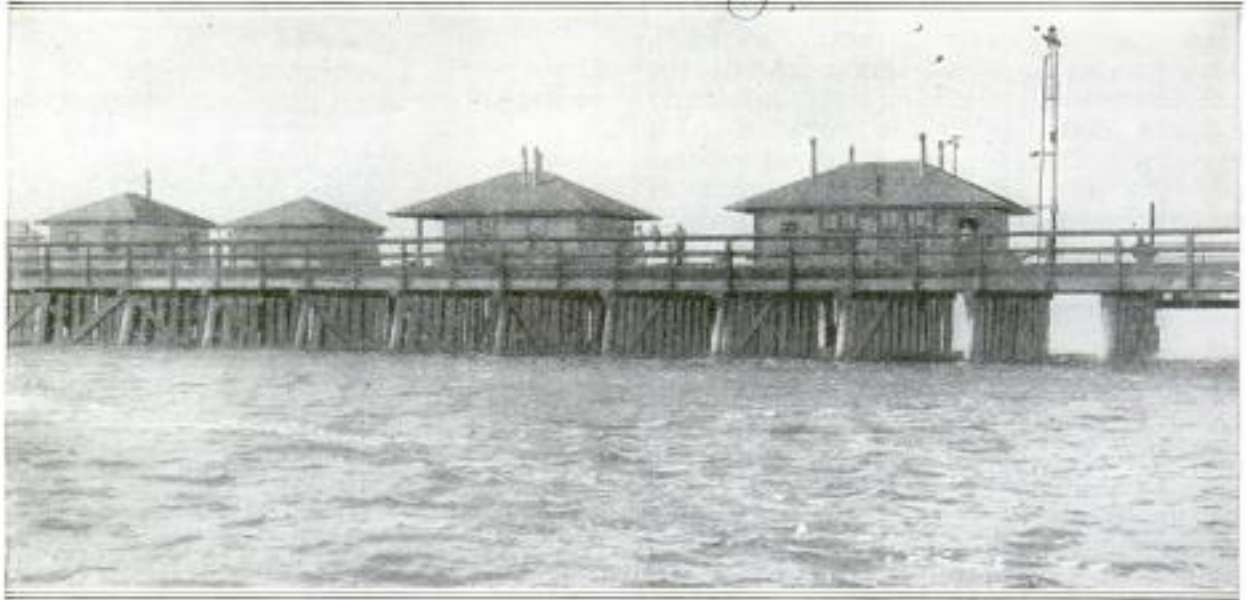
Where Operators Keep Ceaseless Vigil over the Lives of Untold Thousands of Passengers Who Ride on Trains Crossing Trestle over Great Salt Lake
