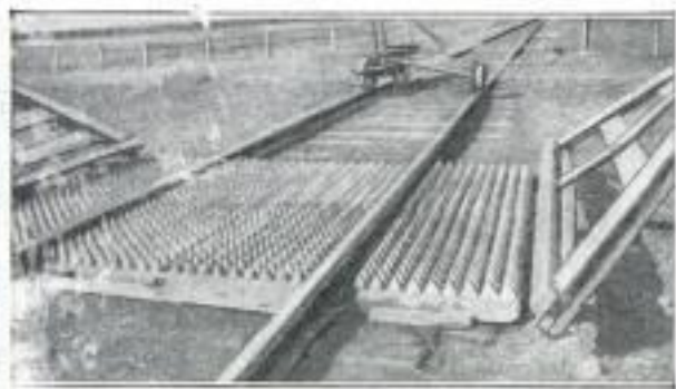
Cones on Heavy Concrete Slab Keep Cattle off Railway Tracks
