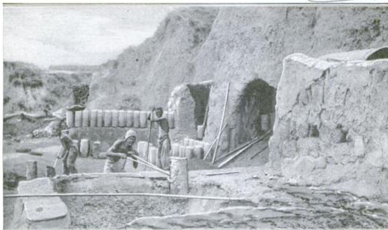
How Natives in China, Using Only the Most Primitive Methods of Iron Making, Remove the Jars Containing the Metal from Crude Furnaces
