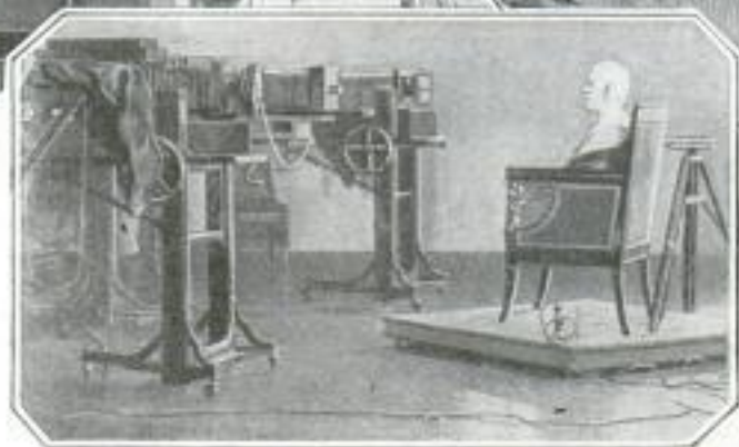
Two Cameras with Projector, in Center, That Throws Lines on Model in Chair
