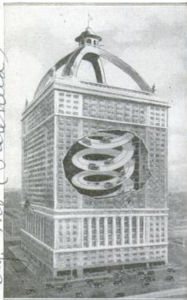
Proposed Skyscraper Cut Away to Show Double-Spiral Driveway in Center
