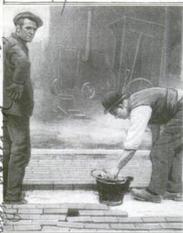
Copyright, Underwood & Underwood An Experimental Rubber-Block Pavement in London
