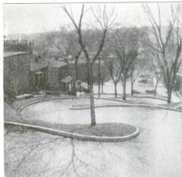
One of the "Hairpin" Curves on Sixth Street, Burlington, Iowa: There Are Five in a Single Block
