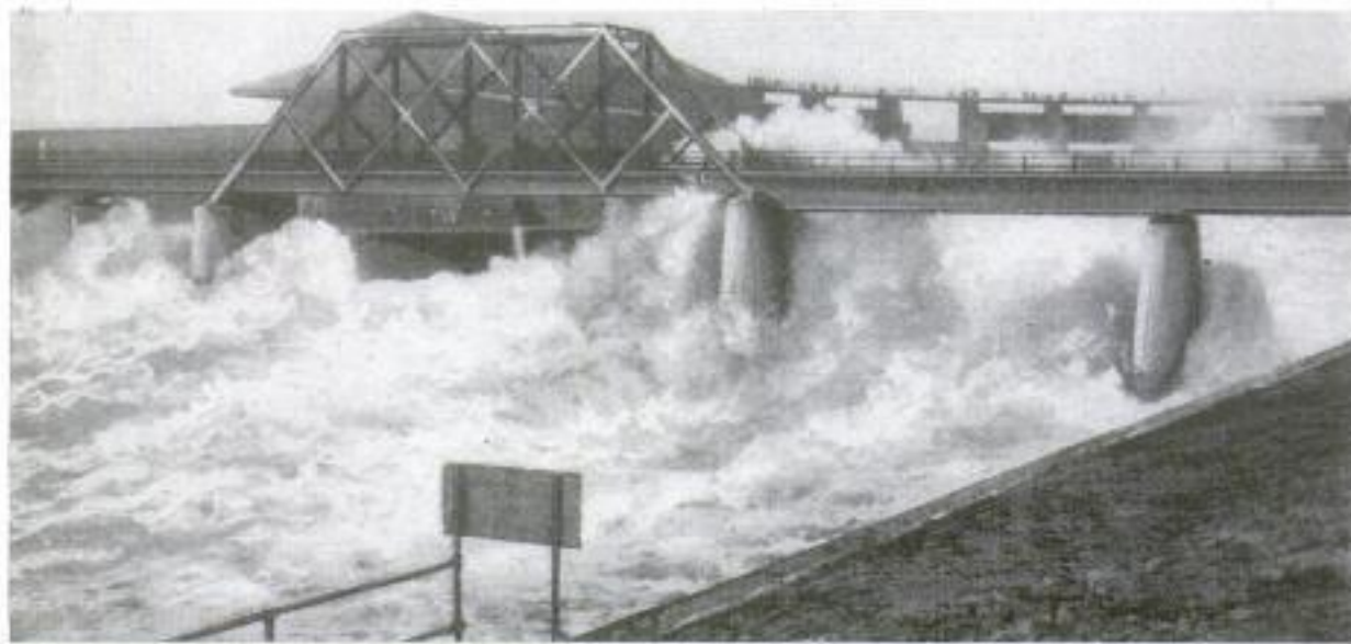
Some of the 'Great Spillways' at the Panama Canal, Showing Torrents of Water Rushing toward the Ocean
