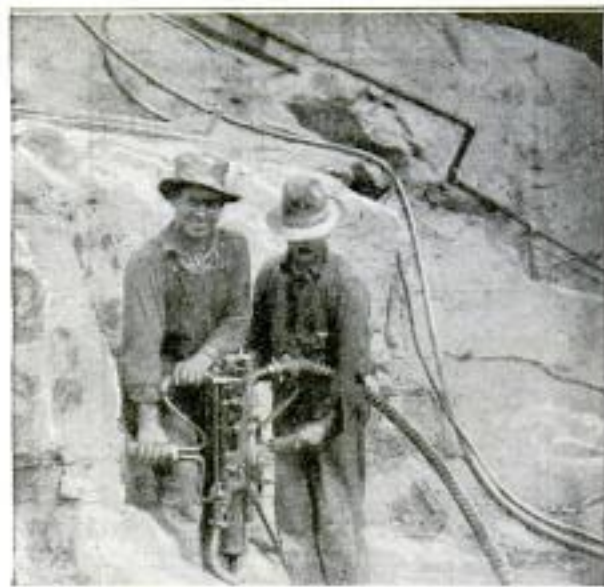
Adaptation of a Tripod Drill for Use as a Portable Hand Drill for Vertical Holes of 6 Feet and Over
