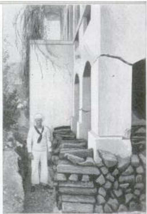
Upper Left: Government Building at Balboa, Vacated Because of Sinking Foundations. Lower Left: Cracks in Walls and Pig Iron Piled on the Ground. Above: Trench Dug around Building
