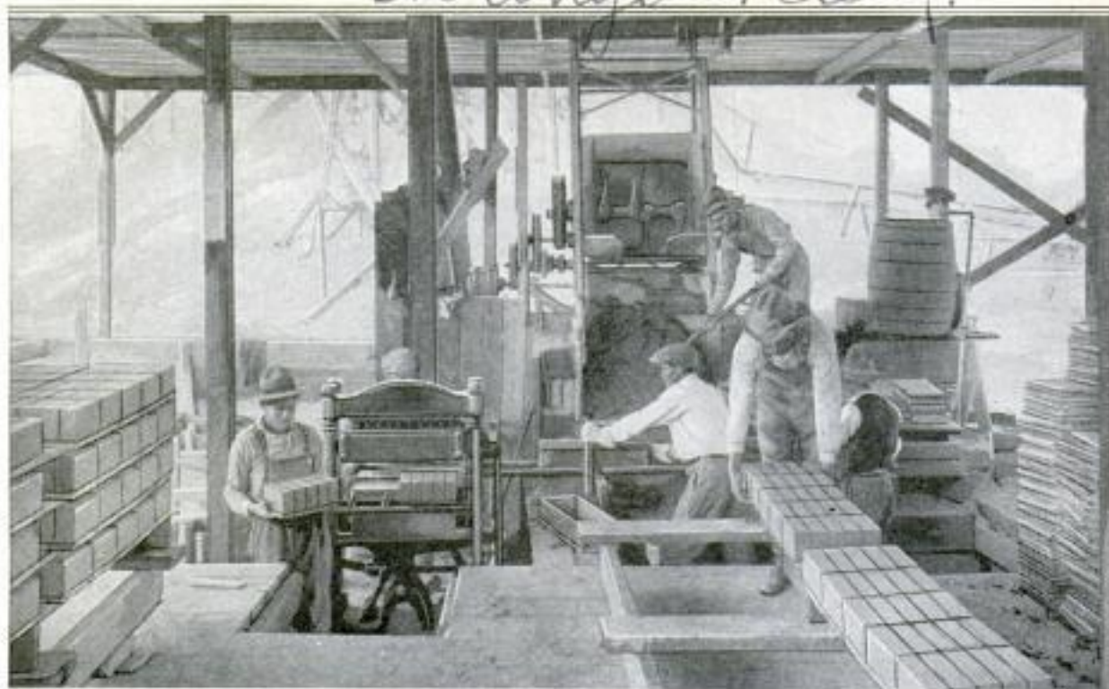
Looking into the Concrete-Brick Plant, Where a Force of Only 10 Laborers will Eventually Turn Out 35,000 Brick a Day
