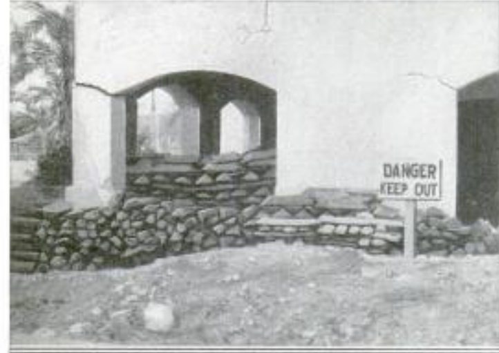
Upper Left: Government Building at Balboa, Vacated Because of Sinking Foundations. Lower Left: Cracks in Walls and Pig Iron Piled on the Ground. Above: Trench Dug around Building
