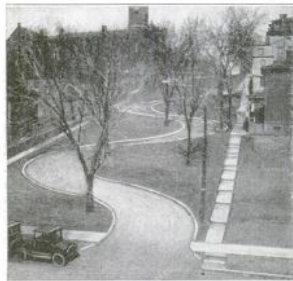
At the Foot of the Brick-Paved "Hairpin" Road: Note the Winding Turns to the Top
