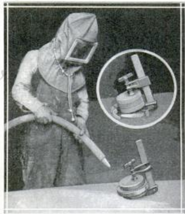
Sandblasting Porthole Lenses to the Proper Size: The Insert Shows a Close-Up of the Finished Operation
