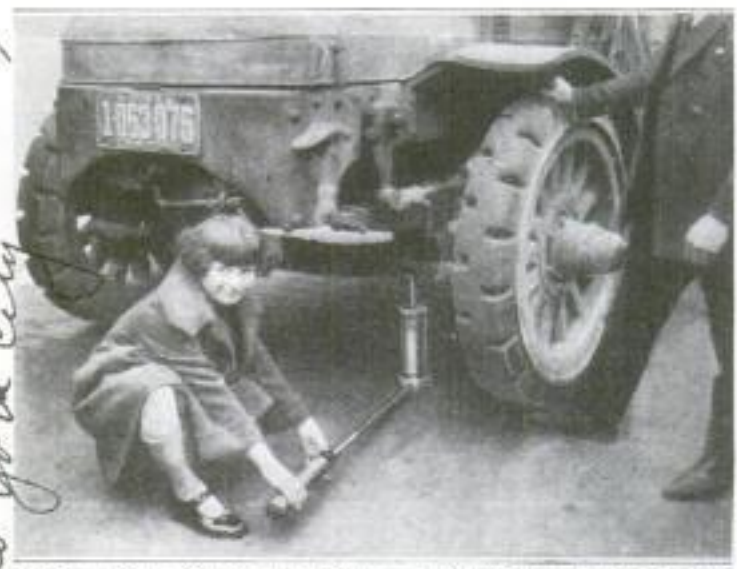
Child Lifting Truck with Force of Expanding Fluid in Steel Container Which is Easily Recharged
