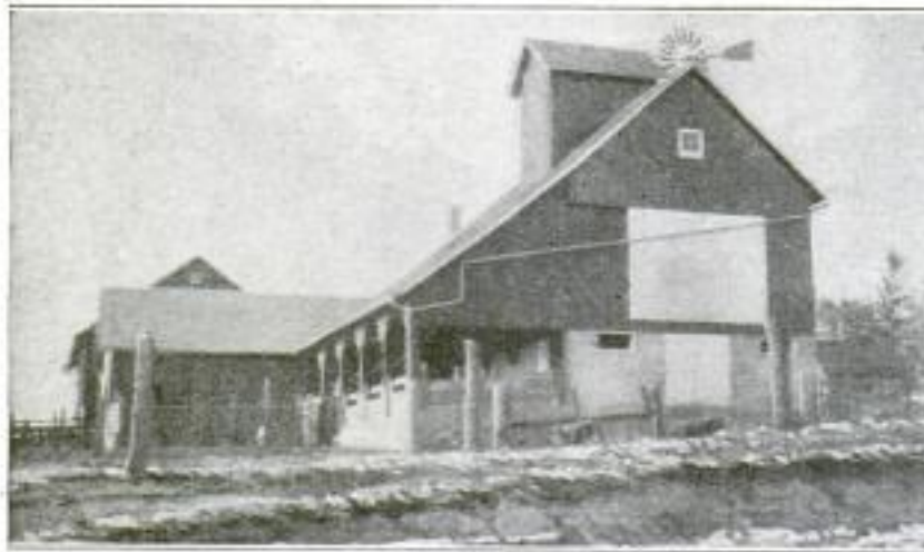
Barn with a Grain Elevator: From the Cupola on Top, the Grain is Distributed into Bins in the Second Story, and Thence by Chutes to the Mangers
