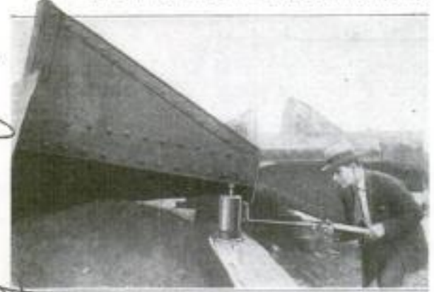
Energy Stored in Small Bottle Used to Lift Heavy Steel Beam
