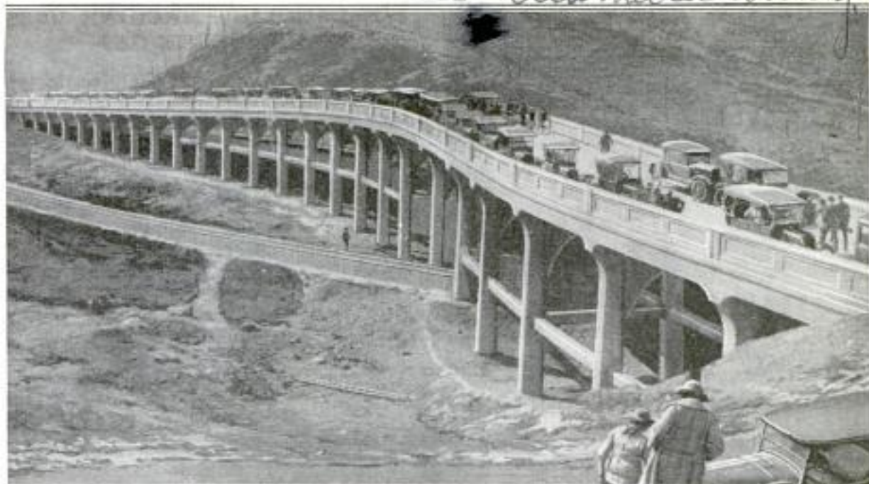
A Glance at This View of the Altamont Pass Viaduct, on the Stockton Highway, California, Brings Home at Once the Dangerous Nature of the Crossing before the Completion of the Structure
