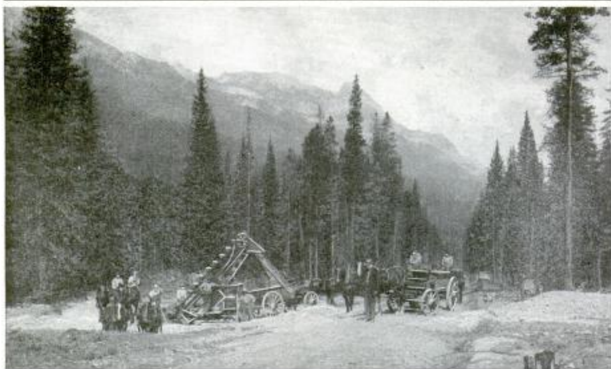
A Construction View on the Banff-Windermere Highway, Indicating the Mountainous Nature of the Country: In the Left Foreground a Portable Bucket Loader can be Seen Elevating Material from the Roadway and Depositing It into a Wagon for Removal
