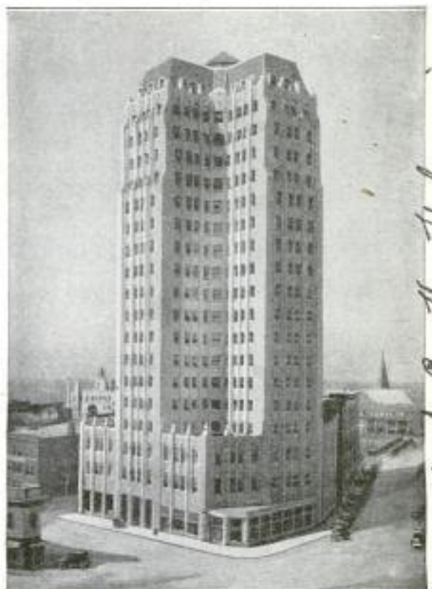
How the 21-Story Concrete Office Building in Dallas, Texas, Appears from a Neighboring Structure
