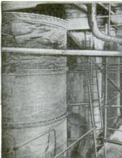
Twenty Tanks Similar to Those Shown at the Left are Required in the Boneblack Process of Refining Sugar, for Doing the Work That can be Done by Three Filters Like the One Shown at the Right, When Using Carbonized Rice Waste
