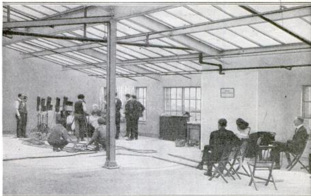
View of a Room in the Department of Agriculture's New Moving-Picture Laboratory, Showing the Arrangement of the Lights and Camera: Note the Open Construction of the Room, Providing an Abundance of Light from Both the Skylights and the Windows
