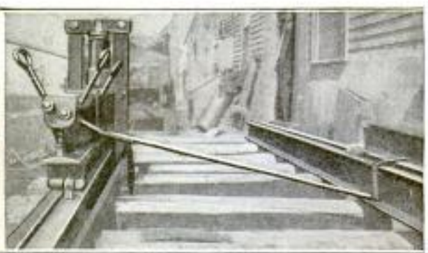
Left: Side View of Rail Bender in the Process of Straightening the Bent Ends at a Rail Joint. Right: End View of Bender, Showing the Yoke That Holds the 35-Ton Jack to the Rails, and the Brace Which Keeps It from Tipping
