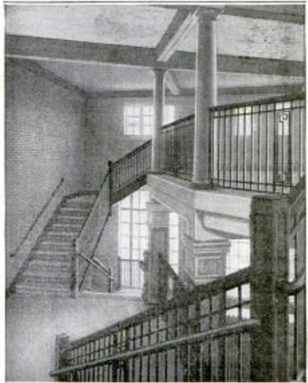
General View of the Interior of One of the Stations on the New Philadelphia Elevated Railway: Entrance to Platform Is from Upper Level
