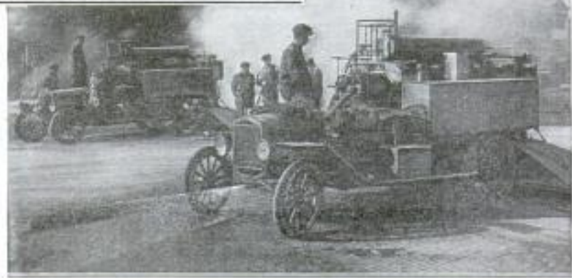
Pavement-Repair Machine Which Carries an Oil-Fired Brick-Lined Furnace, Extending along the Top to the Overhanging Hood at the Rear
