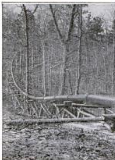
Above: The Force of a Stream of Water under High Pressure is being Used to Break Down the Bank of This Coal Deposit, Making It Easy to Handle. Below: A Section of Cast-Iron Pipe, Conveying the Water
