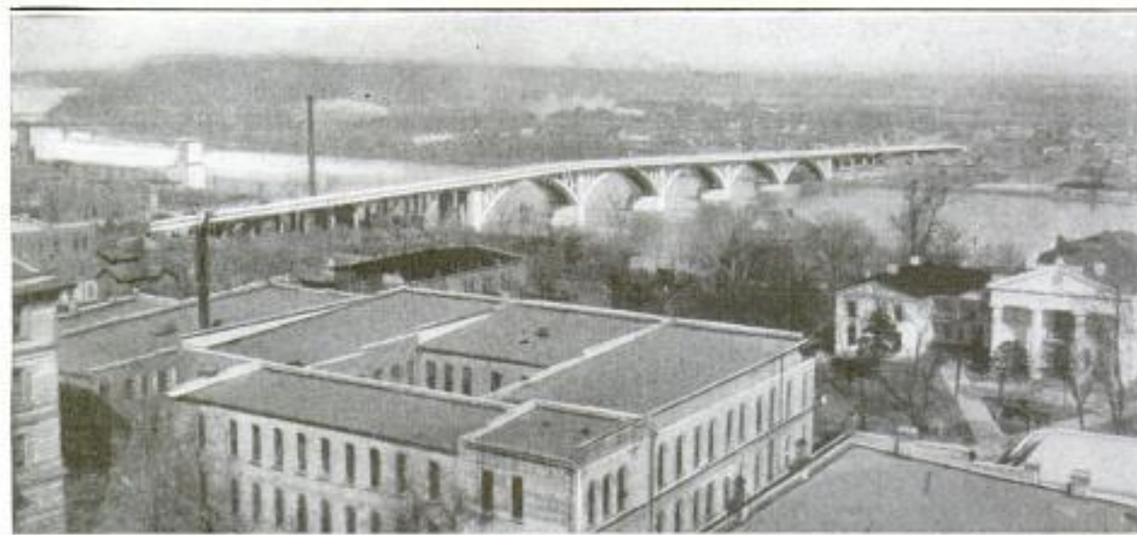
A Bird's-Eye View of the New Concrete-Arch Bridge Thrown across the Arkansas River at Little Rock: This Structure was Built to Commemorate the Soldiers, Sailors, and Marines Who Died during the War. Five Arches Span the River, with Long Approaches on Each Bank
