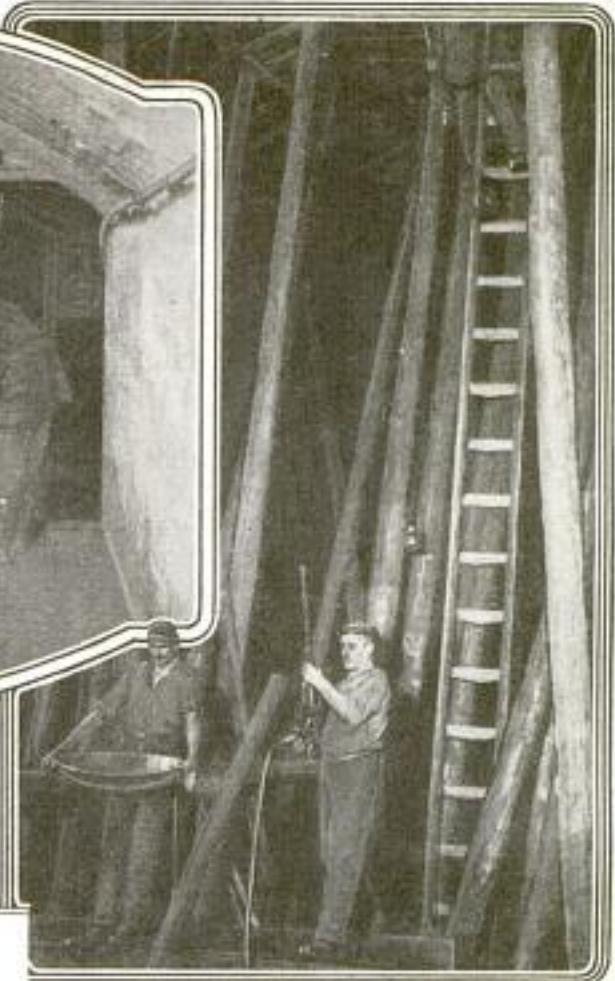
Above: A Workshop 400 Feet Underground Where Mechanics Repair Electric Locomotives Used for Hauling Trains of Small Cars in the German Coal Mines. Right: Miners at Work with Compressed-Air Machines Drilling Holes in the Coal
