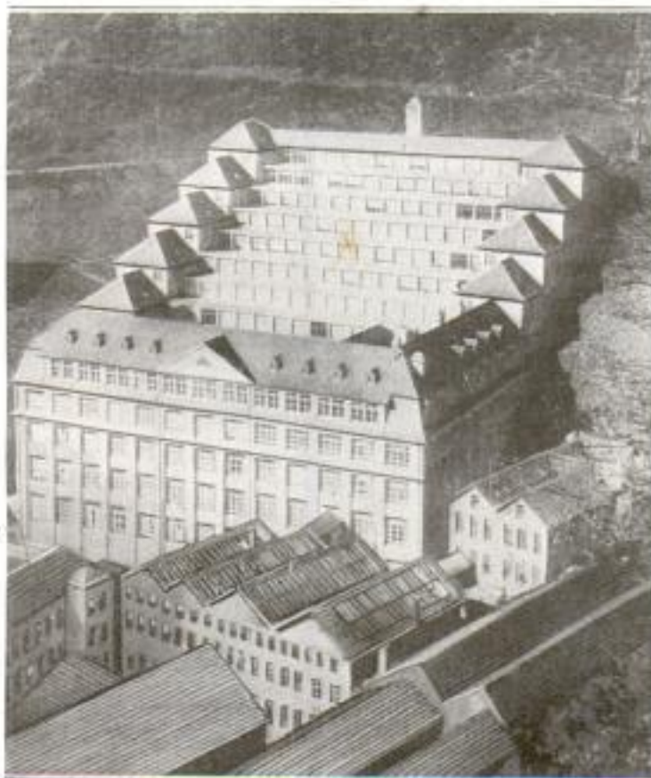
PHOTO BY GILLIANG SERVICE German Watch Factory Which Expands by Climbing a Mountainside in the Only Possible Direction: Its Growth is Marked by Additions Which Rise like Steps
