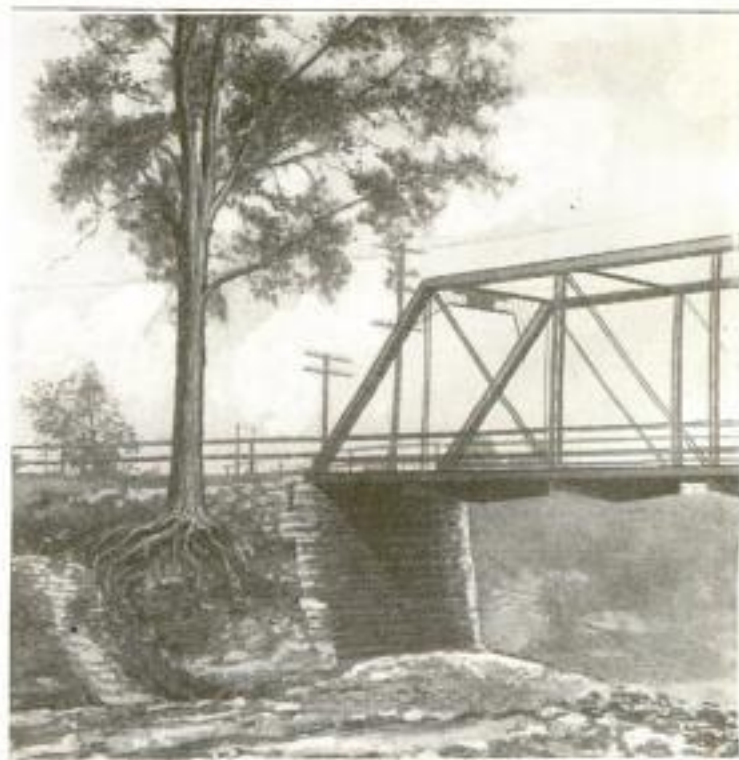
The Roots of This Tree beside a Trunk-Highway Bridge Destroyed the Wall of the Abutment, as Shown; Hence It was Removed When a New Bridge was to be Built
