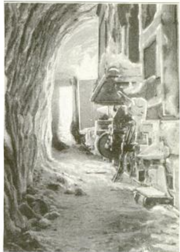
Tunneling in the Snow to Dig Out a Buried Locomotive on the White Pass and Yukon Route: Note How Firm and Hard the Frozen Side Walls Look
