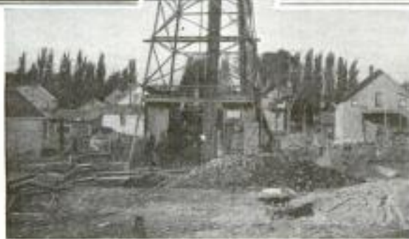
This Is a View of a Diamond-Drilling Outfit, with Its Supporting Derrick, Taken in the Lake Superior Iron Region of Minnesota
