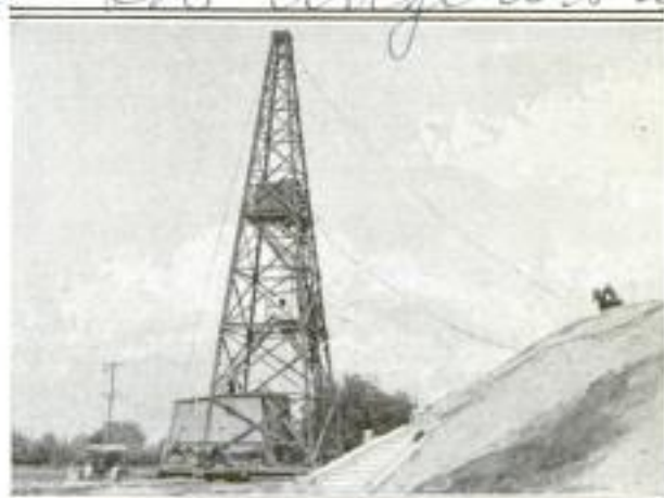
Towering Derrick Used to Operate Bucket for Excavating, and Endless Cable on Which the Bucket Moves
