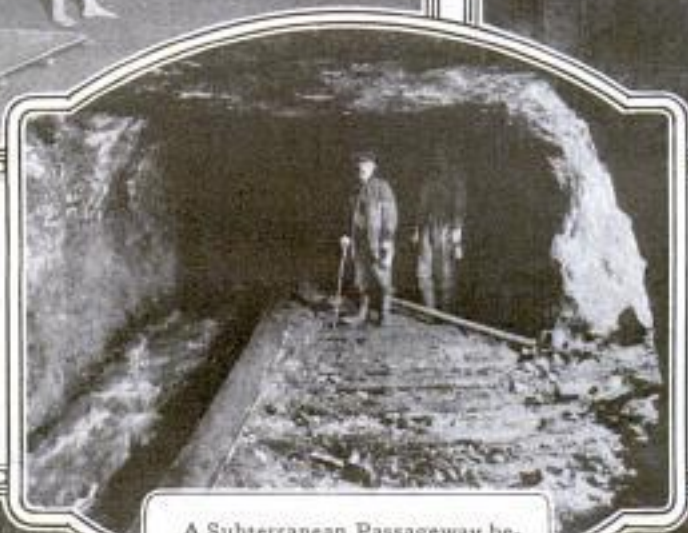
A Subterranean Passageway between Two Ruhr Coal Mines: The Trench at the Left is for Drainage Purposes
