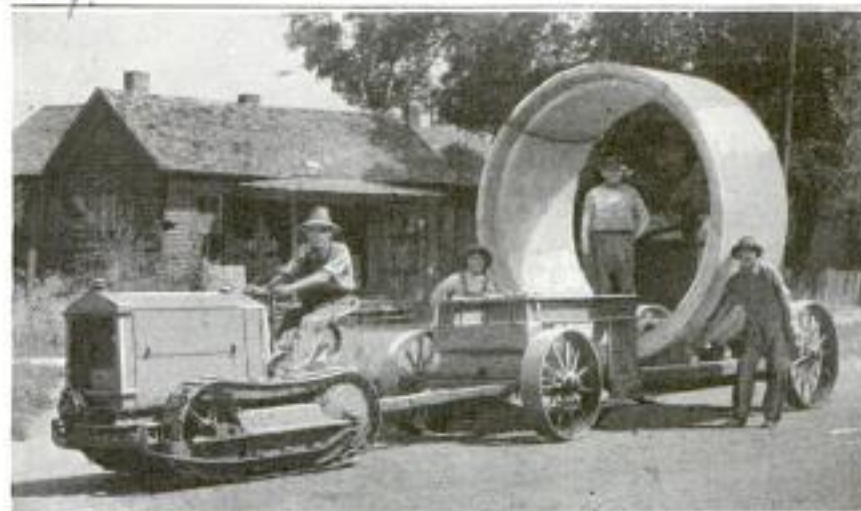
Transporting a Section of Concrete Sewer Pipe, 108 Inches in Diameter: One of These Pieces of Pipe Weighs About Six Tons
