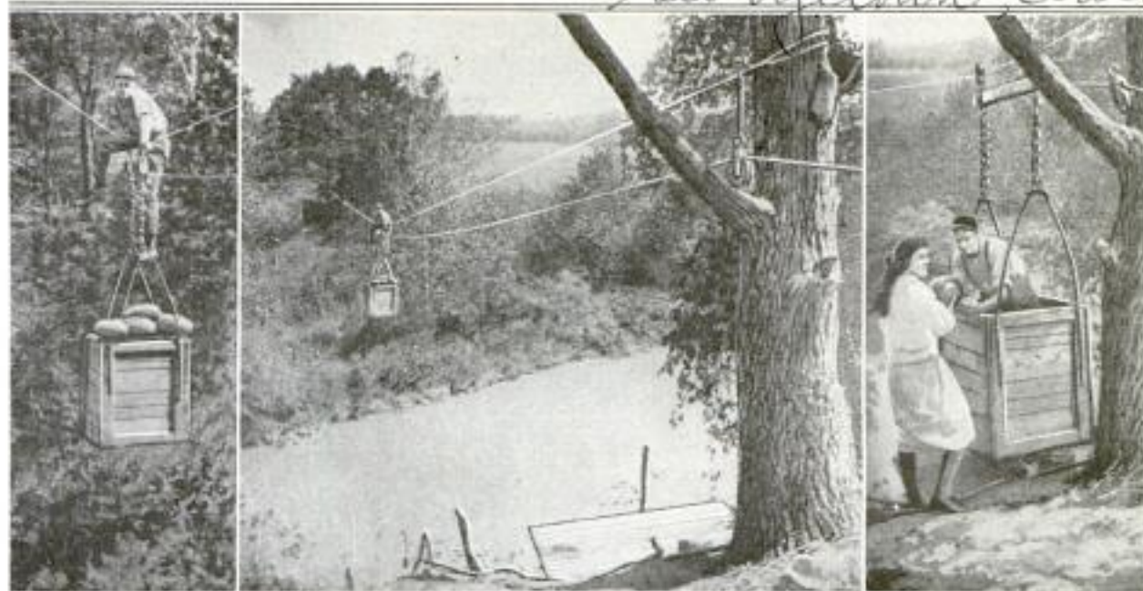
Saving Time and Distance Carrying Melons over a Creek on a Cable: Left, Starting with the Load; Middle, Crossing the Creek 100 Feet above the Water; Right, Unloading Melons on Farther Side of the Creek on Receiving Platform
