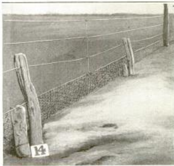
Original Boundary Fence in Australia Covered by Sand Drift, Which is Creeping Up on the Second Fence
