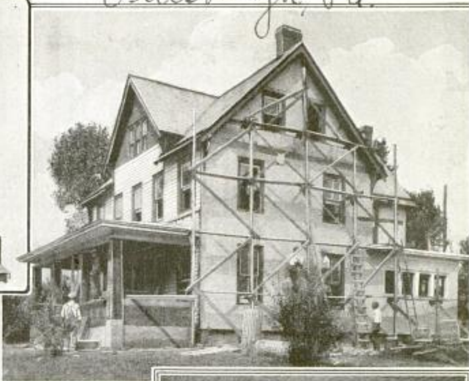
An Exterior View, Showing the Application of the Steel Fabric to Both Exterior and Interior Walls, as Well as to Porch Floors
