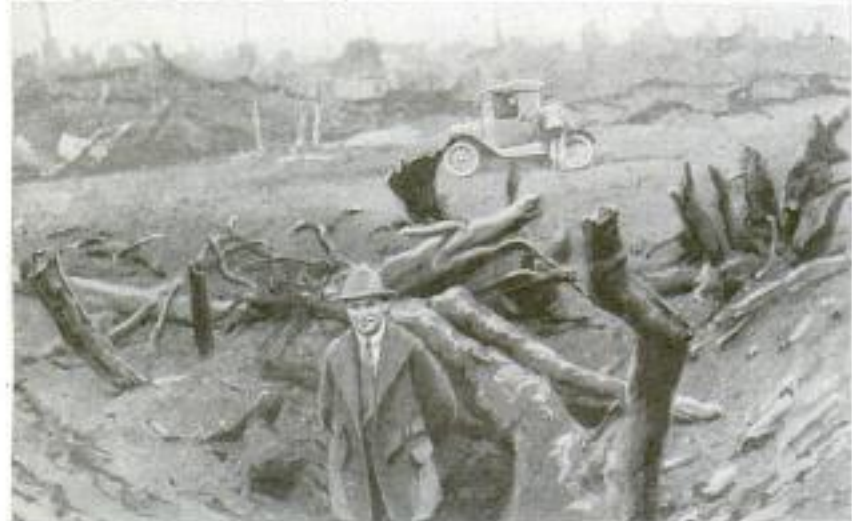
Above: Fir Stump, 14 Feet in Circumference, Used in Demonstrating the Effectiveness of the New Explosive Compound. Below: Result of the Explosion of 25 Pounds of the New Compound under the Stump
