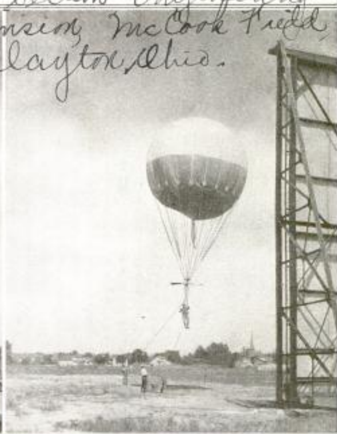
Left: New "Jumping Balloon" Developed by Employees of the Engineering Division at McCook Field, Dayton, Ohio, Ready to Begin an Ascent. Right: Balloon About to be Cut Loose for an Ascent. The Feature of This Balloon Is a Small Control Propeller
