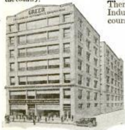
Here's the big, 7-floor GREER building, with its thoroughly up-to-date equipment. You learn by actually doing the jobs, after you master the theory.
