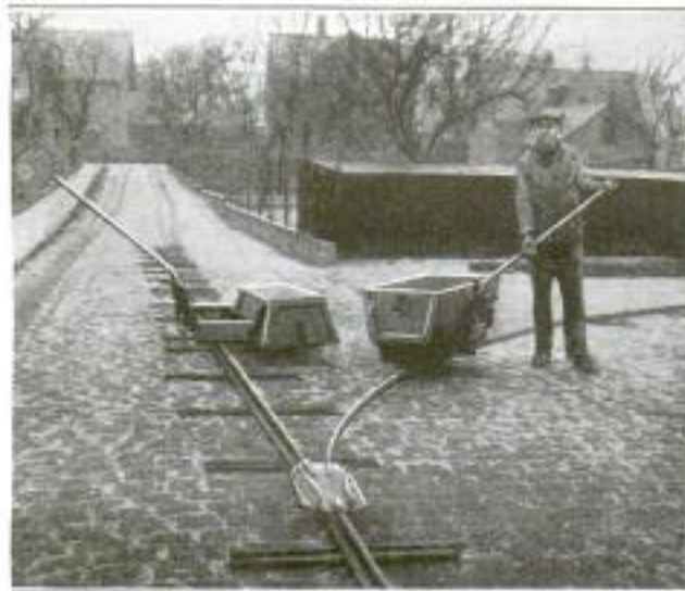
A Monorail Hand Car Which is Supplanting the Wheelbarrow in Germany: At the Left, It is Used on a Temporary Portable Single-Rail Track, and at the Right, on the Right of Way of a Railroad
