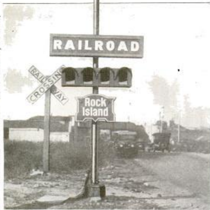
COPYRIGHT UNDERWOOD & UNDERWOOD Railroad Safety Signal for Level Crossings: Whenever a Train is Approaching, the Four Lights under the Sign "Railroad" Display the Word "Stop" in Bright-Red 10-Inch Letters
