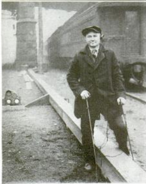
This Signal Inspector Saves Himself Much Extra Labor with His Iron Walking Sticks. With the Receiver at His Ear He "Listens In" for Trouble.
