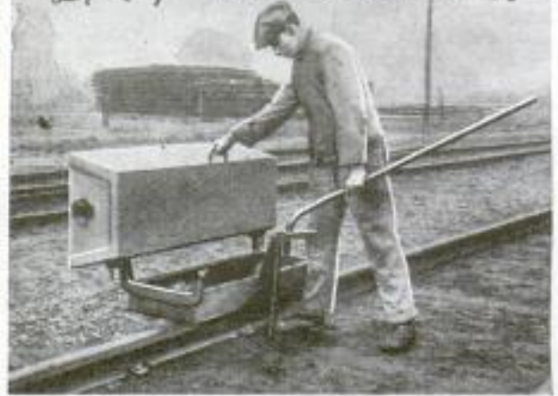
A Monorail Hand Car Which is Supplanting the Wheelbarrow in Germany: At the Left, It is Used on a Temporary Portable Single-Rail Track, and at the Right, on the Right of Way of a Railroad
