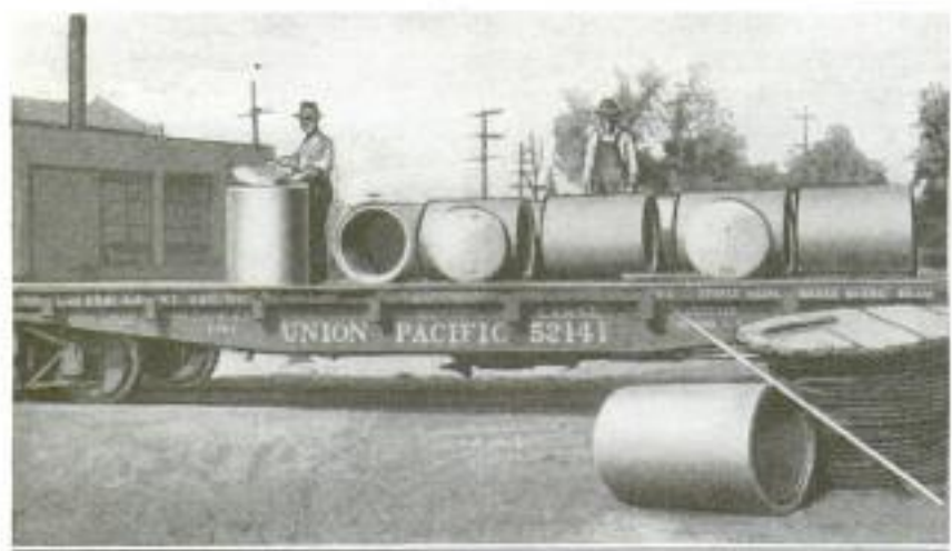
Concrete Water Barrels Which are being Introduced on the Union Pacific System, and on the San Diego and Arizona Branch of the Southern Pacific: Less Evaporation Is One of the Benefits Expected
