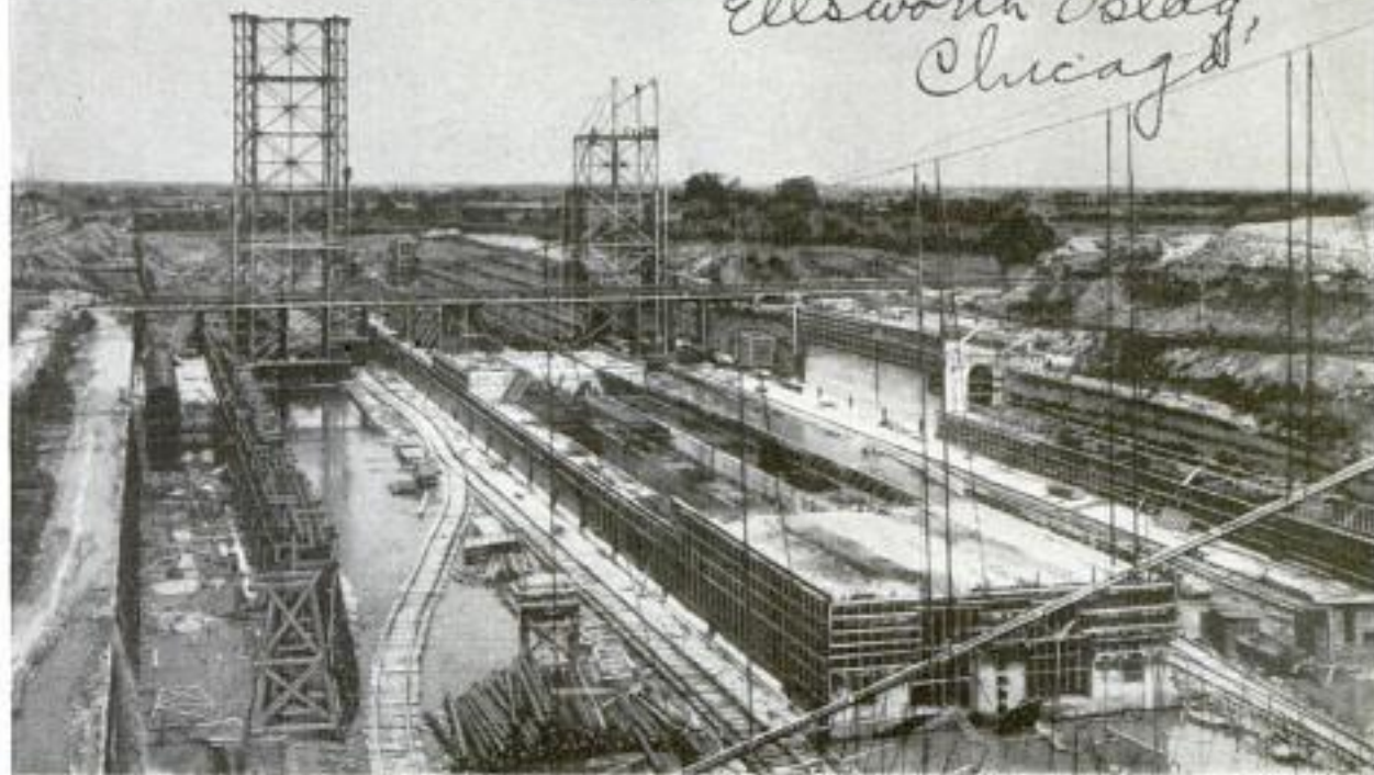
A View during Construction of Lock Number Six of the New Welland Ship Canal, as Seen from the Upper West Entrance Wall: Each of the Locks, of Which There Are Seven, Has a Usable Length of 800 Feet, a Usable Width of 80 Feet, and a Depth of 25 Feet
