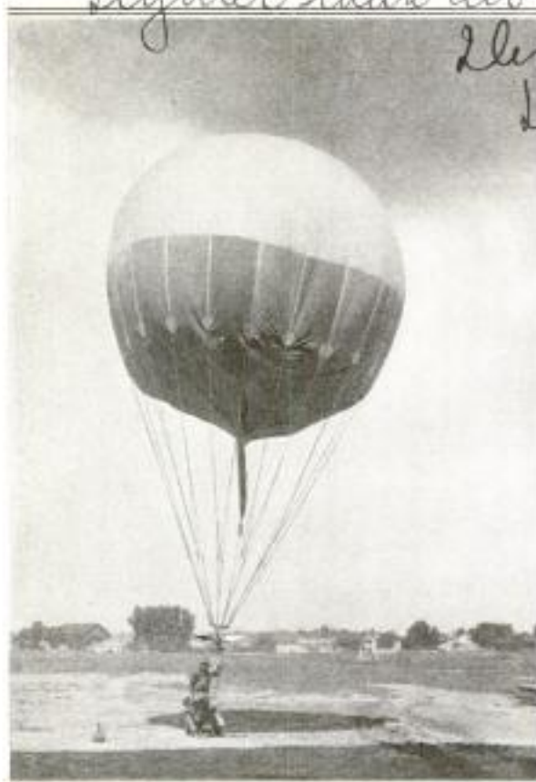
Left: New "Jumping Balloon" Developed by Employees of the Engineering Division at McCook Field, Dayton, Ohio, Ready to Begin an Ascent. Right: Balloon About to be Cut Loose for an Ascent. The Feature of This Balloon Is a Small Control Propeller
