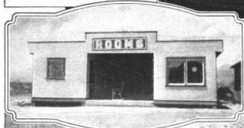
Rooming House in Small Town in the Mohave Desert, Built like a Garage So That the Ends may be Left Open to Permit Circulation of Air
