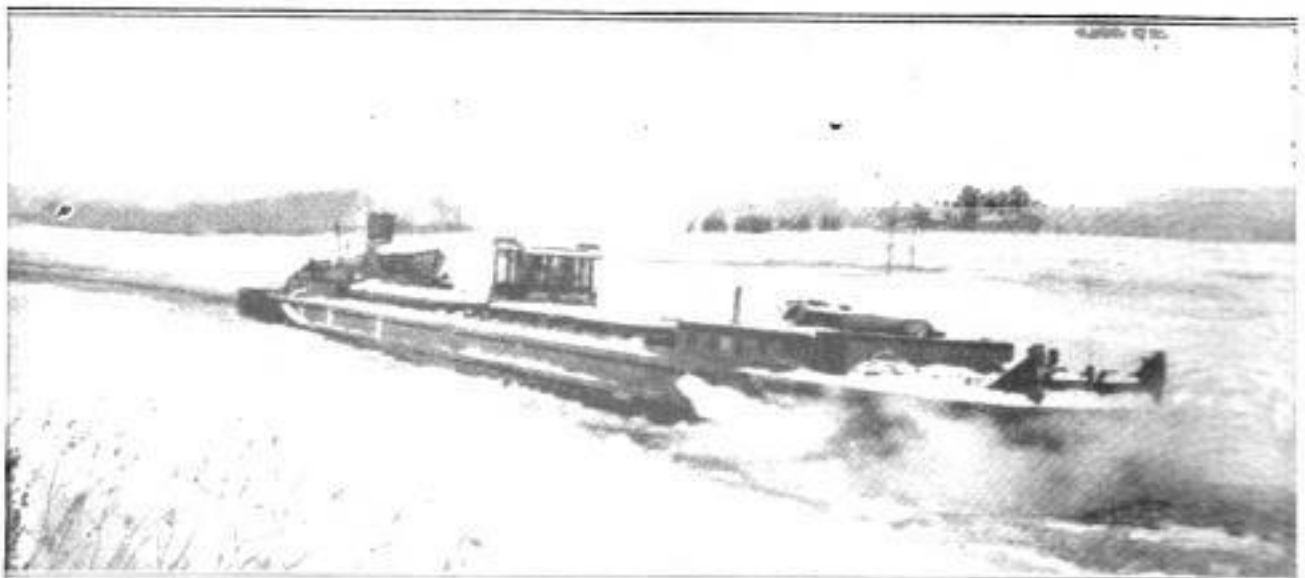
One of the Ice-Bound Canal Boats being Towed through the Channel of Floating Ice That was Opened Largely through the Use of Dynamite: The Progress Was But a Mile a Day Until the Boats Finally Found Safety at a Canal Lock
