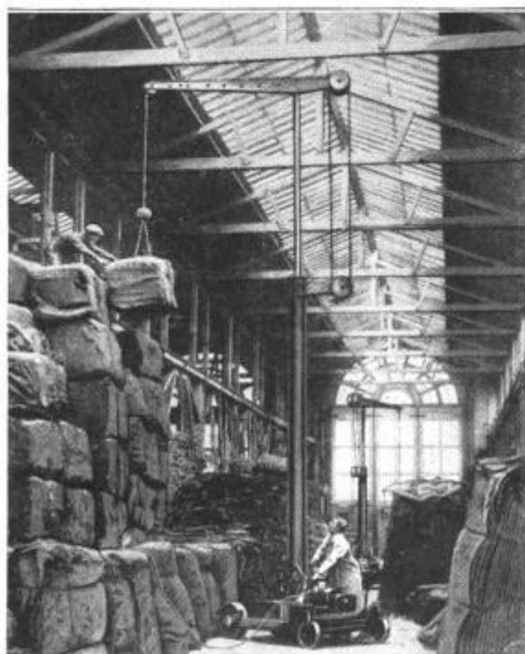
Portable Hydraulic Crane, Operated Electrically and Used for Piling Goods in Warehouses: In This View the Main Plunger is Telescoped Almost to Its Full Height
