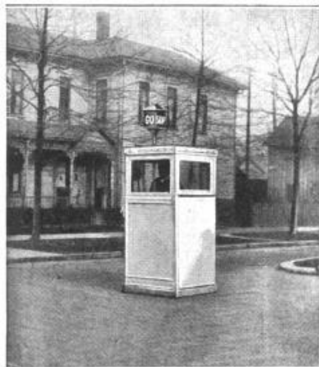
This House for a Traffic Officer Weighs Only 35 Pounds. The Stop and Go Signals on the Roof are Operated from Within
