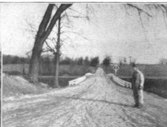
Left: Michigan Country Road before Improvement as Trunk Highway. Right: Same Road after Improvement, Showing Smoother Surface, More Uniform Grade, Fences on Elevated Stretch, and Less Danger at Railroad Crossing. Note Cattle Guard and Change of Danger-Signal Position
