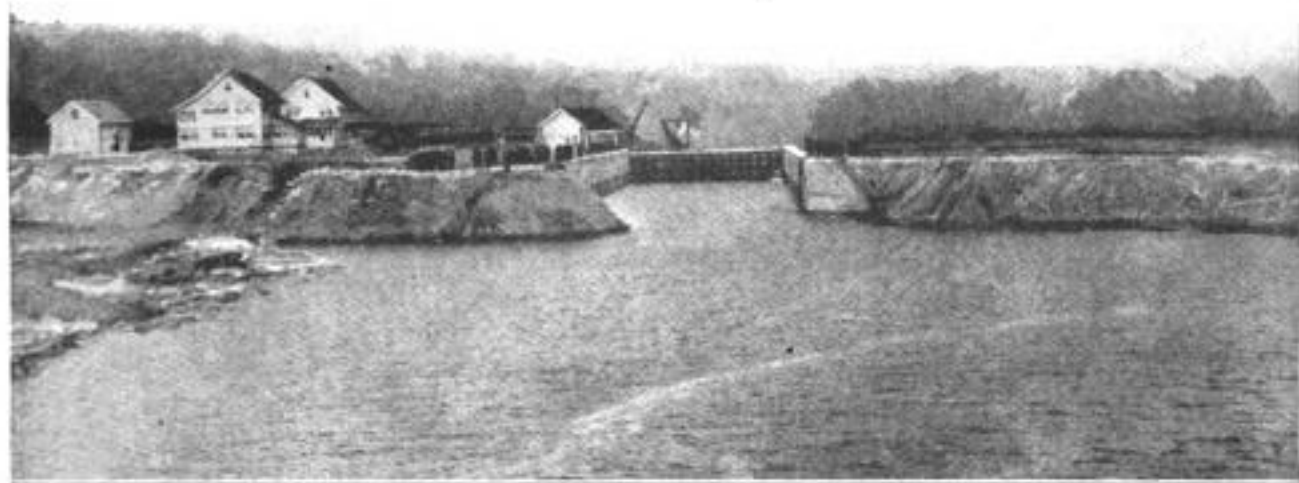
Another View, Looking Upstream and Showing the Approach to the Lock, the Lower Gates of Which Are Open: To the Left Are the Homes of the Lock Tender and Workmen
