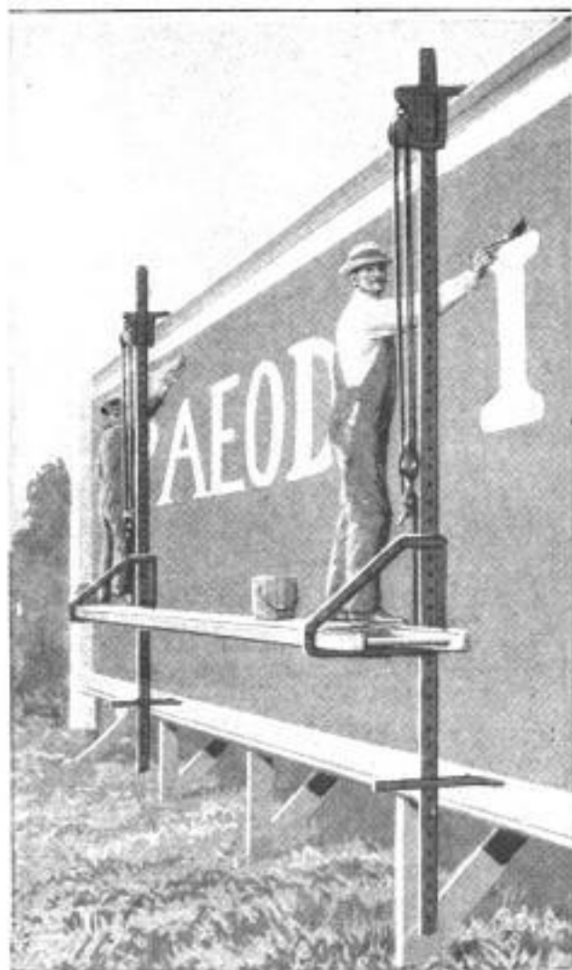
Easily Erected Scaffold, the Two Wooden Uprights of Which Have Adjustable Hooks So That They can be Swung in Place over the Billboard
