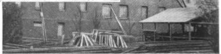
Erection of a Clubhouse in Washington with New Method of Concrete Construction in Which Units are Cast on the Ground and Then Raised to Position: Above, Three-Story Wall Raised with Shaft and Jackscrews; Right, Finished Wall in Place
