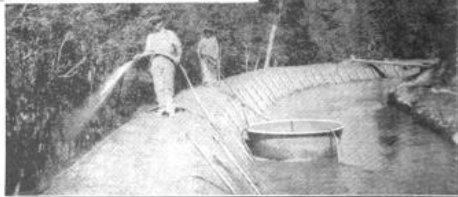
Above: A Section of Canal Lined with Wood Panels to Prevent Erosion of Its Banks; Note How the Panels are Held in Place by Long Pieces of Pipe Straps Passing through Two Loop Straps, and Then into Bottom of the Canal
