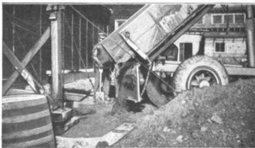
Delivering Factory-Mixed Concrete in Trucks of This Type has been Tried with Success in Larger Cities
