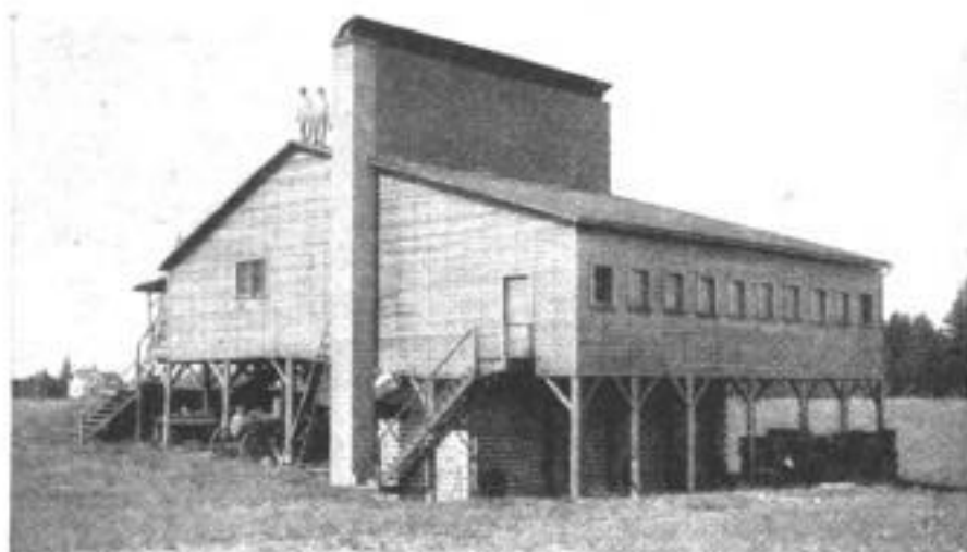
A Prune-Drying Plant in Oregon, Constructed with a Recirculation System for the Air, Which was Developed at the Oregon Agricultural College and is Rapidly Replacing the Tunnel Type of Drier
