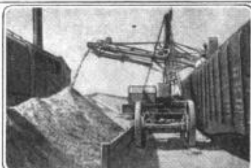
Left: Conveyor and Elevators Raised to Clear Top of Car, and Ready to be Swung into It; Note That Lower Portion of Elevators is Folded Up. Above: Rig Unloading Sand
