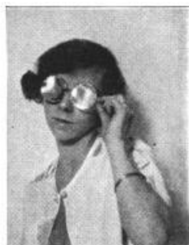
The Spectator must Wear Glasses with One Red and One Green Lens in Order to See the Screen Picture in Relief
