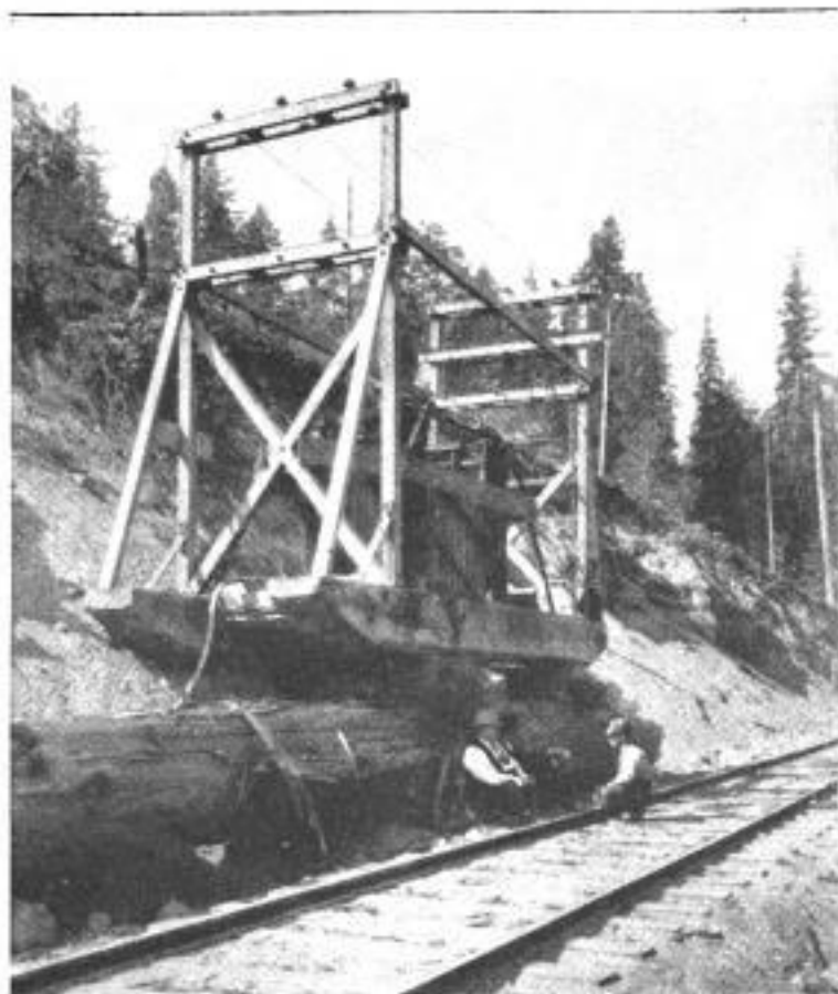
These Transformers, Which Supply a Large Lumber Camp with Electric Power, are Mounted on Sleds and Easily Moved
