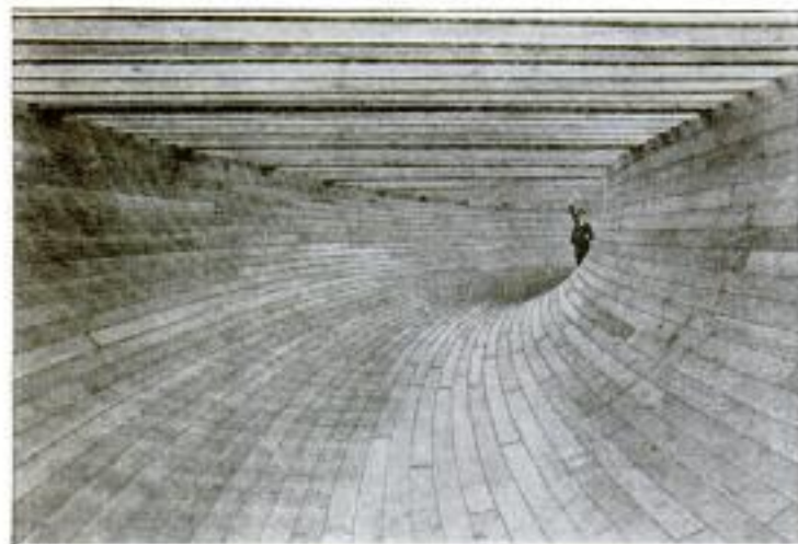
View Showing the Curve of 100-Foot Radius to Which This Wooden Flume was Constructed in Spite of the Fact That It was Pronounced by Many to Be Impossible
