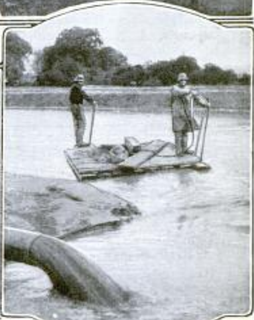
Below: Hydraulic Monitor Washing Clay from Bank Used as Fill for the Dam. Right: Measuring Level of Clay Settlement Pumped into the Dam as Indicated by Discharge in Lower Left-Hand Corner
