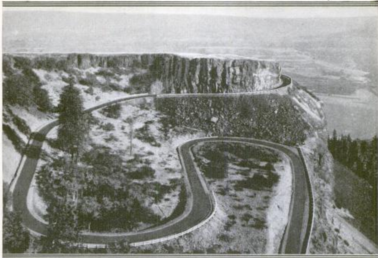
Near the Top of the Rowena Loops, Showing How the Road has been Cut through Solid Rock and Made to Wind about the Edge of the Cliff: Note, Too, the White Fence Guards Which are Built at Curves in the Highway and Other Possible Points of Danger
