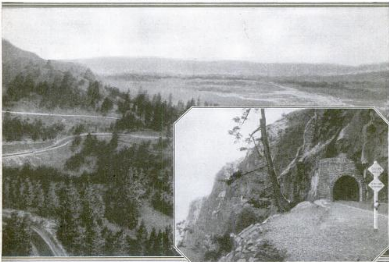
been Taken in Keeping the Average Grade of the Road below Five per Cent. The Complete Cost of the Grading Inserted at the Left and Right Are Picturesque Views of Two Tunnels on the While the Other Is Entirely without Artificial Support
