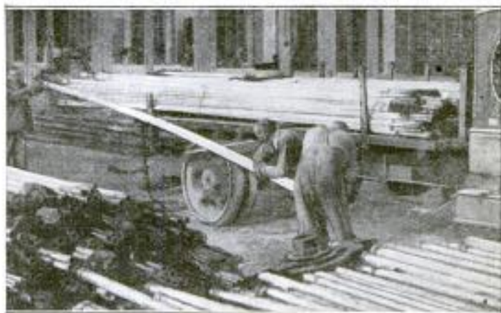
A Method of Loading Pipe onto a Truck That Enables the Work to be Accomplished in One-Half the Time Otherwise Required
