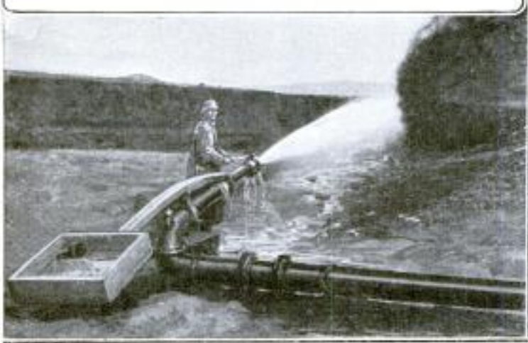
Below: Hydraulic Monitor Washing Clay from Bank Used as Fill for the Dam. Right: Measuring Level of Clay Settlement Pumped into the Dam as Indicated by Discharge in Lower Left-Hand Corner
