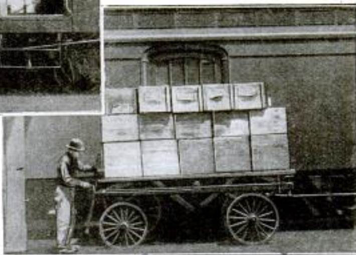
Above: New Station Truck Raised to Height of Floor in Baggage Car. Right: Man in the Act of Elevating the Truck Floor, Which can be Raised and Lowered through a Range of 18 Inches
