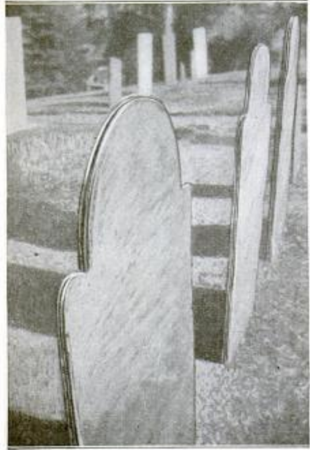
Side View, Showing the Condition of the Headstones before being Treated: This Type of Marker is Seldom Used at Present
