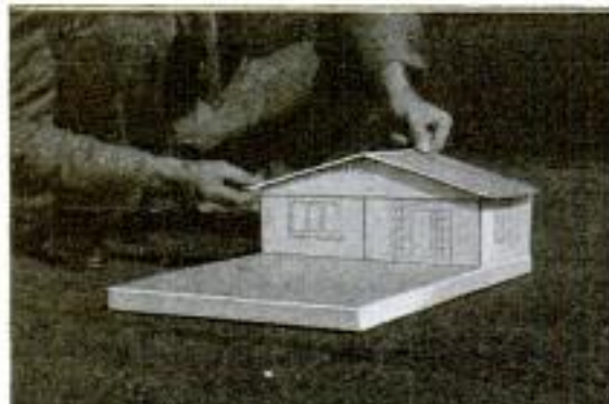
Two Completed Miniature Models of Houses: The Full-Size Buildings are Erected in Accordance with the Models with Standard Sections That Correspond on an Enlarged Scale with the Cardboard Sections of Which These Models are Constructed. The Latter Sections Are Interchangeable, Permitting Great Variation in Design
