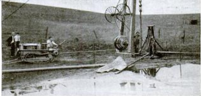
The Same Winch at Work Pulling an Oil-Well Casing, Which was Anchored at the Bottom by Several Feet of Closely Packed Sand, Long Undisturbed
