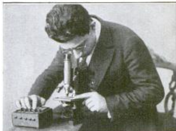
Automatic Machine Invented by Chicago Physician to Count Cells in Blood Analysis: With One Hand He Operates Keys for Five Cell Species
