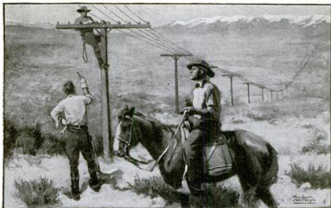
The Bell System's transcontinental telephone line crossing Nevada.
