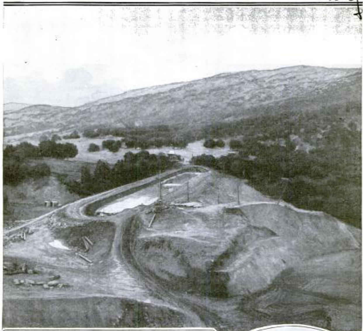
Below: Hydraulic Monitor Washing Clay from Bank Used as Fill for the Dam. Right: Measuring Level of Clay Settlement Pumped into the Dam as Indicated by Discharge in Lower Left-Hand Corner
