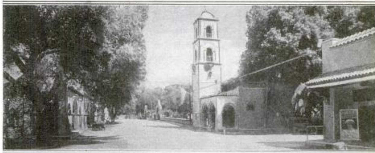
View of Main Street in the Renamed Town Ojai: The Improved Appearance of the Street Is Striking, Despite the Fact That the Buildings Themselves were Not Materially Altered but Only Concealed from View by an Arcade of Cement Construction, as Seen to the Left. The Tower on the Church, However, Is an Addition to the Old Structure
