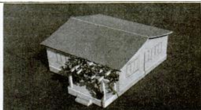
Two Completed Miniature Models of Houses: The Full-Size Buildings are Erected in Accordance with the Models with Standard Sections That Correspond on an Enlarged Scale with the Cardboard Sections of Which These Models are Constructed. The Latter Sections Are Interchangeable, Permitting Great Variation in Design
