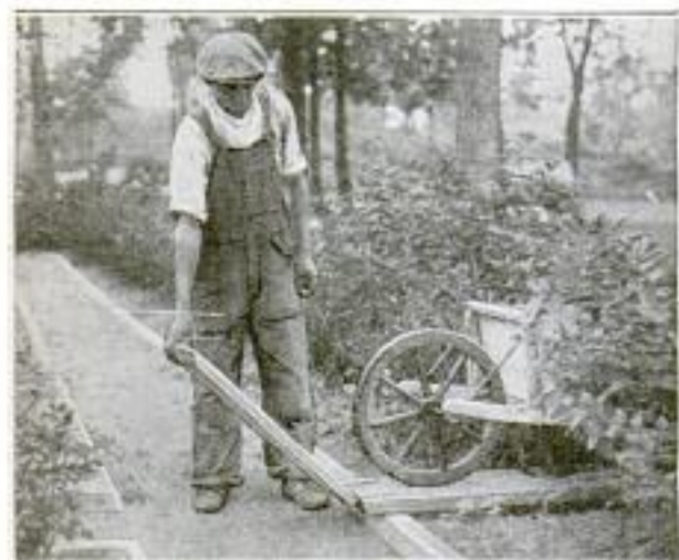
A Runway Used by a Gardener to Protect Concrete Curbing from being Damaged When Pushing a Heavily Loaded Wheelbarrow over It
