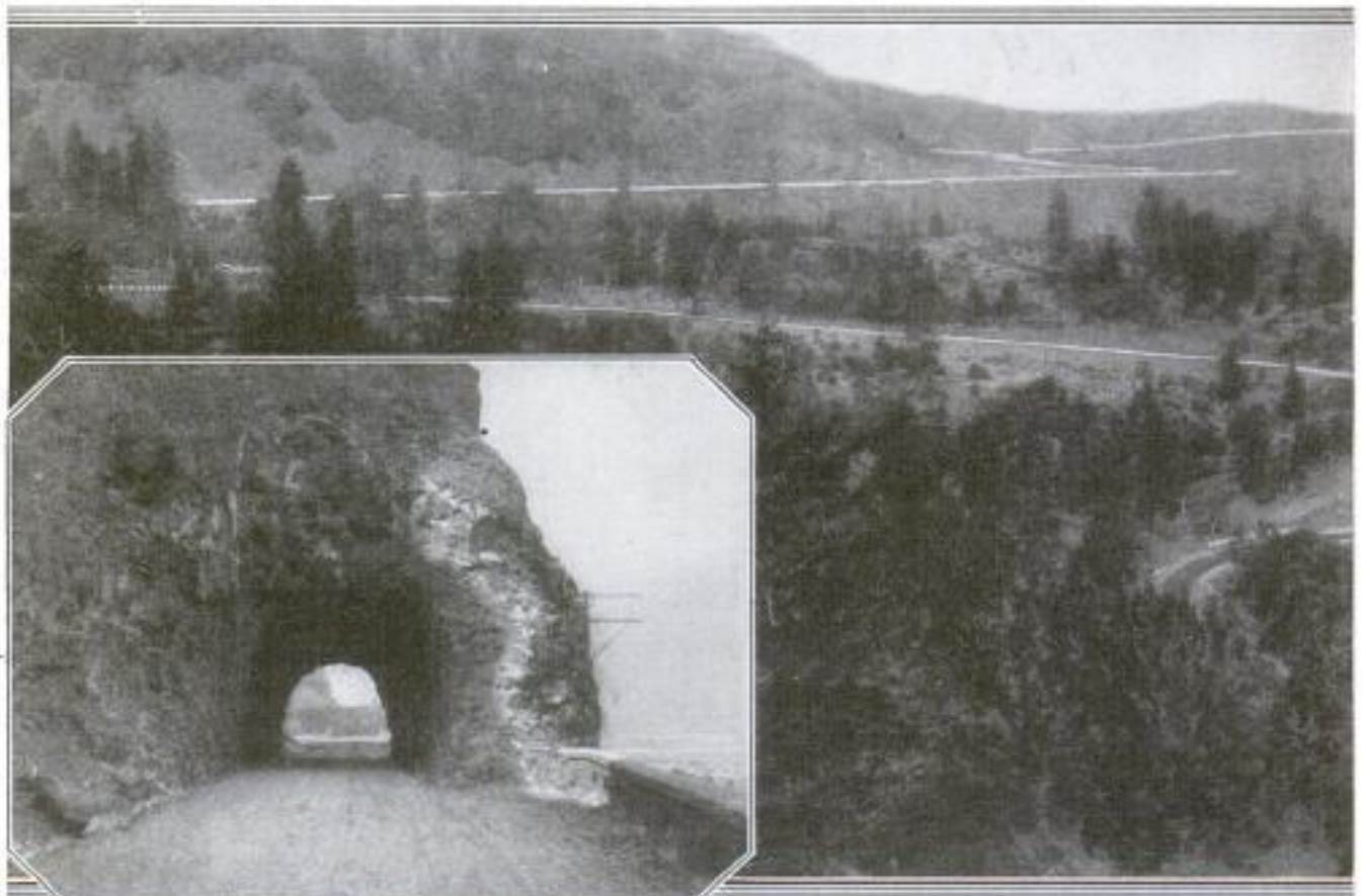
This Panorama of the Loops Gives a Good Idea of the Beauty of the Surrounding Country, and the Care Which has Been Taken in Its Construction. The Total Cost of the Highway, the Entrance to One being Built of Stone, Was Approximately $185,000, and the Cost of Paving the Section About $90,000.
