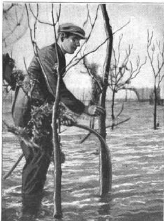
Close-Up, Showing Operator Holding Nozzle in the Same Hole, with a Fish-Trap Pole That has Just been "Pumped In"
