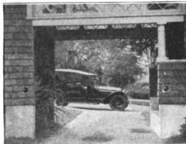
Porte-Cochère of a Residence, Showing the Special Electric Lights Which were Installed at Each Side of the Narrow Driveway
