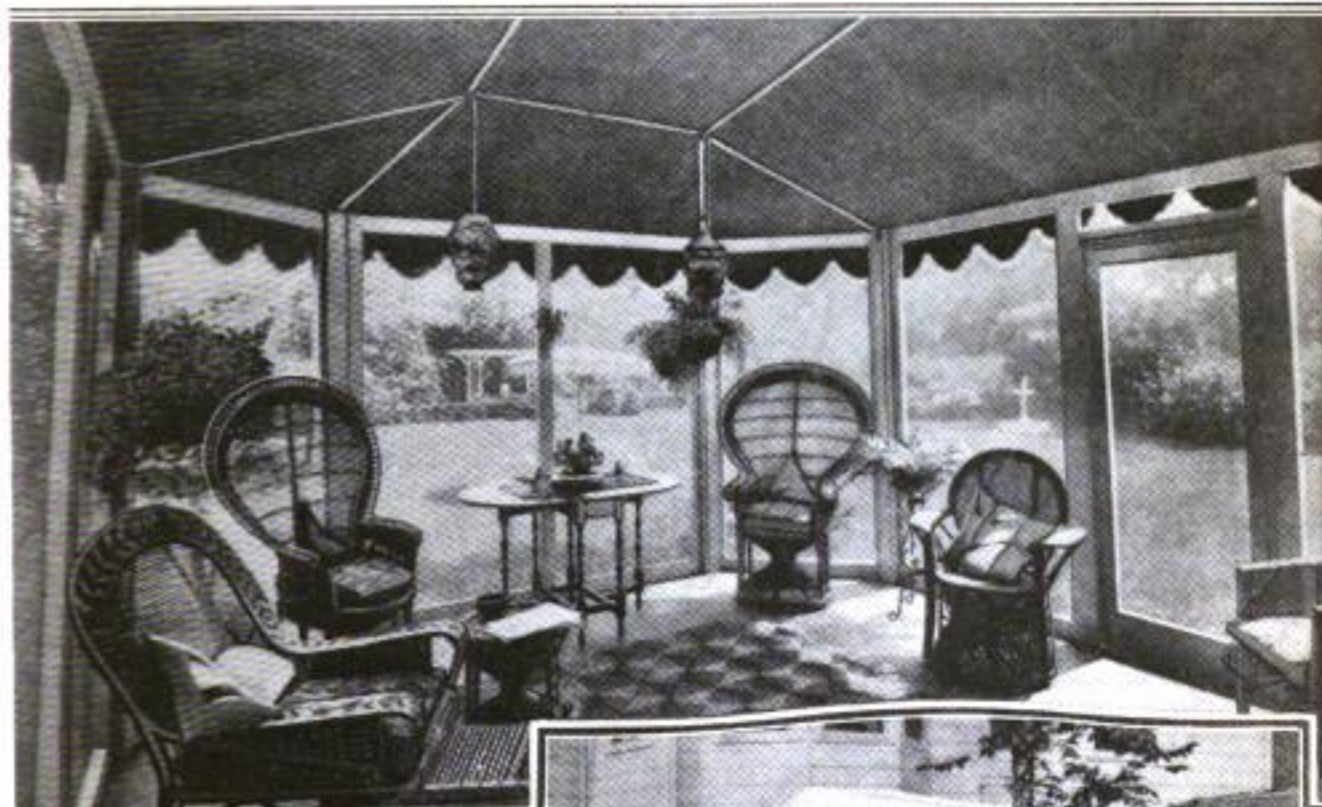
Above: Interior of the Collapsible Porch Which was Built for the Residence of a Lover of Sunshine, Showing the Roomy Inclosure with the Wooden Frames for Supporting the Screening, and the Canvas Roof Stretched over the Framework of Iron Piping. Right: Exterior of Porch, Illustrating Its Neat Appearance
