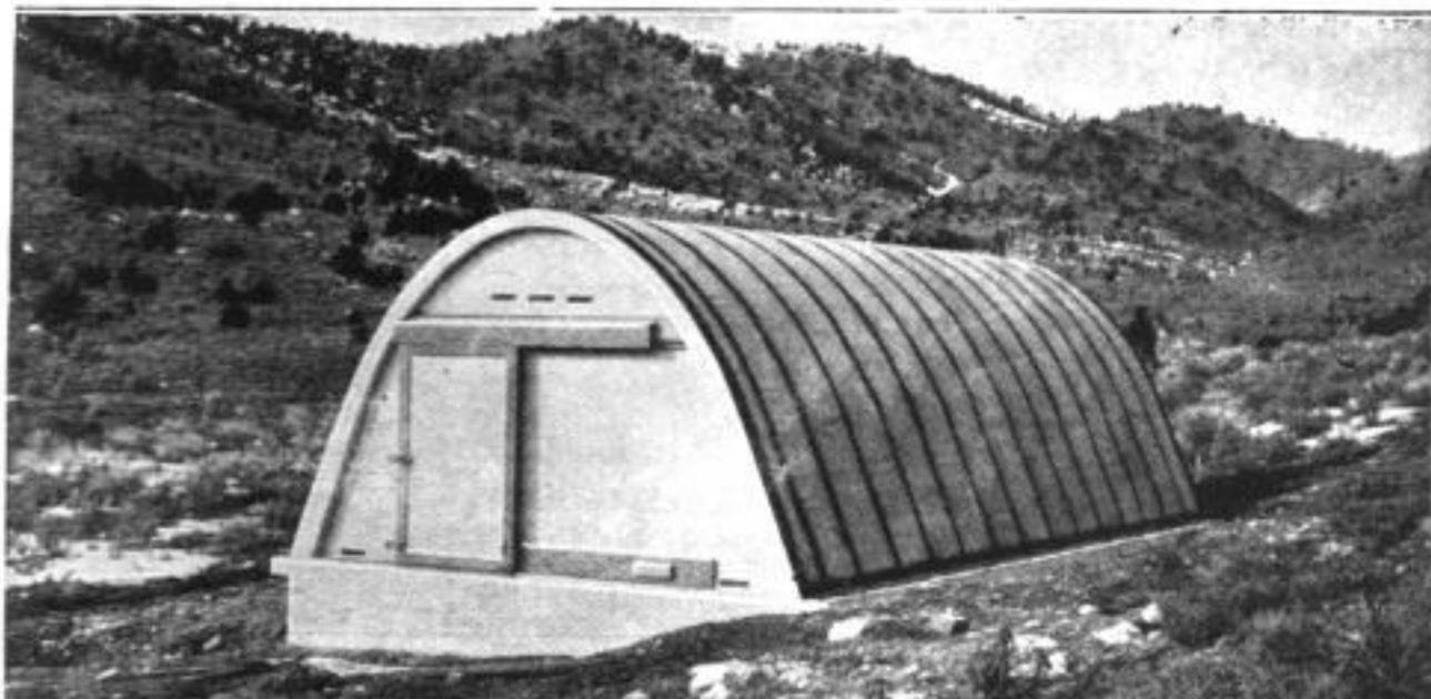
This Magazine for High Explosives, Designed to Offer as Little Resistance as Possible in Case of Accidental Explosion of Its Contents, Allows the Explosive Action to be Dissipated into the Air, Thereby Minimizing the Danger to Adjacent Property
