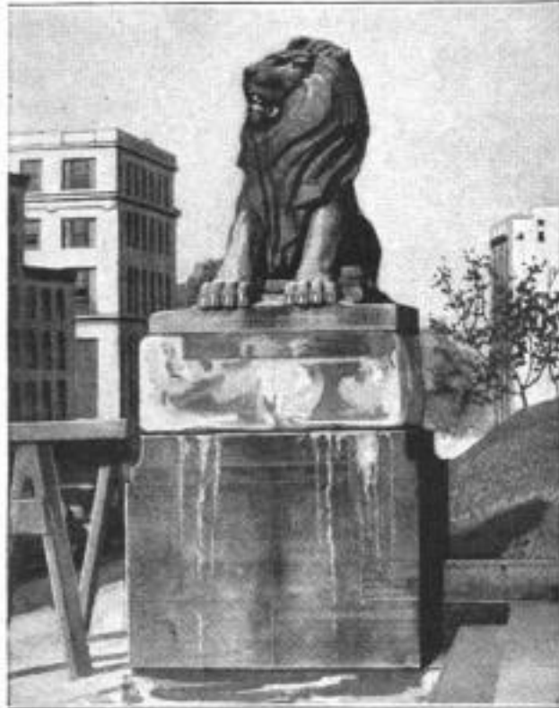
Sculptured Stone Lion Shown Resting upon Cakes of Ice, the Melting of Which Slowly Lowered the Statue to Its Foundation
