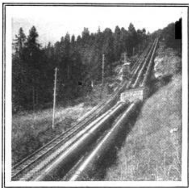
Conduits from Ritom Lake, the Huge Reservoir of the St. Gothard Railway, to the Power Station at Piotta, Where There Are Turbines of 48,000 Horsepower
