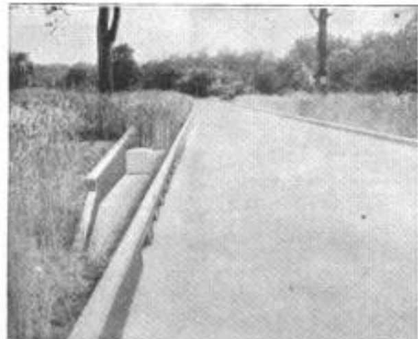
Left: Section of New Pavement Grade, Showing the Drainage Scheme Whereby Holes are Left in the Curb So That the Rain Water may Run Off Before It Reaches the Bottom of the Incline. Right: Side View of Pavement, Showing, More Clearly, the Construction of the Curb and Concrete Drain
