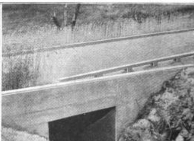
Left: Section of New Pavement Grade, Showing the Drainage Scheme Whereby Holes are Left in the Curb So That the Rain Water may Run Off Before It Reaches the Bottom of the Incline. Right: Side View of Pavement, Showing, More Clearly, the Construction of the Curb and Concrete Drain
