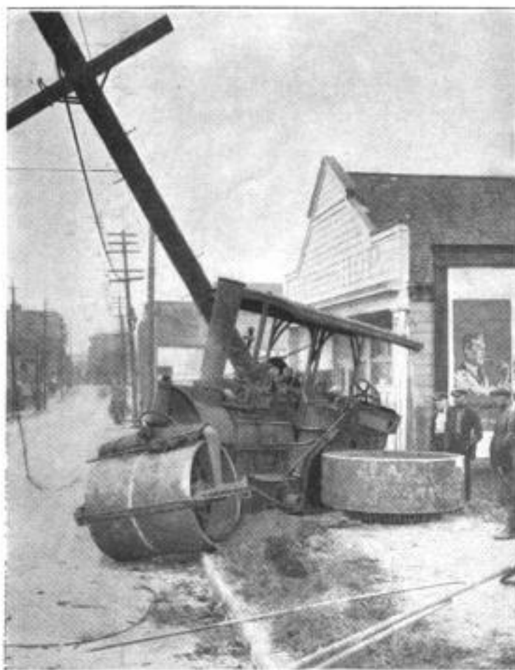
Steam Roller Which Ran Amuck down a Steep Grade, Finally Coming to Rest of Its Own Accord After It had Jumped the Curb and Lost One of the Rear Wheels
