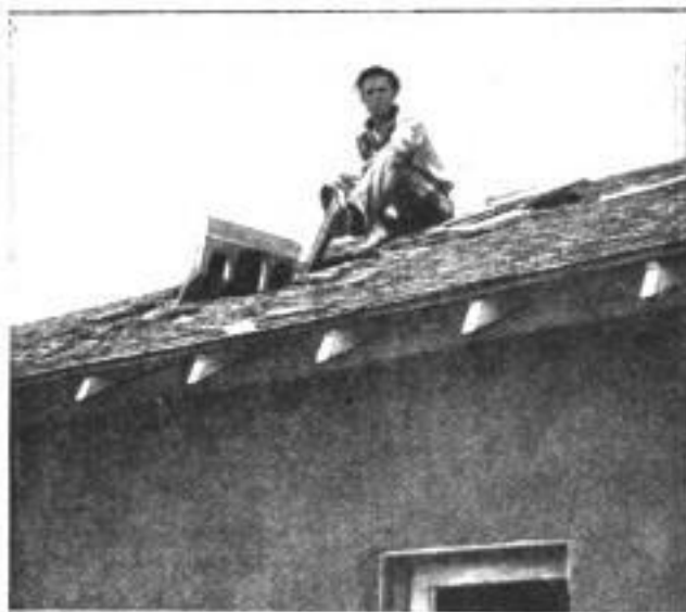
Filling-Station Roof, Showing Part of Vulcanizing Steam Generator Which was Thrown Up by the Terrific Force of the Explosion
