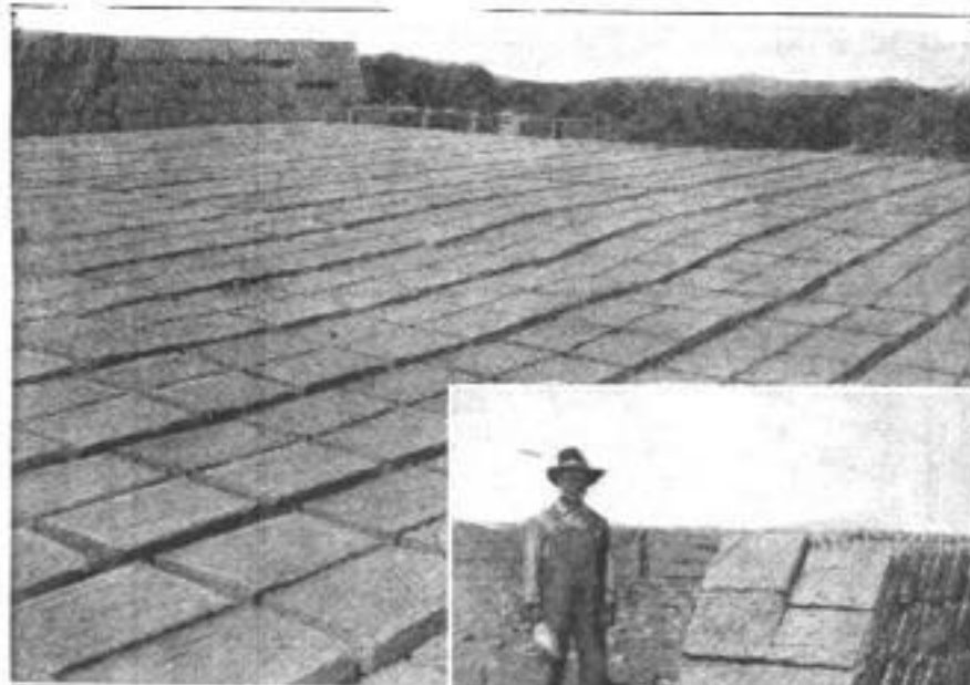
Adobe Bricks Made for Building the Keeper's Lodge at Torrey Pines Park, San Diego, California, Shown Above, Lying Flat on the Ground After the Frames in Which They were Made had been Removed: When Sun-Dried They are Piled in Ricks, as Shown to the Right. In Constructing the Building, the Bricks will be Laid in Cement
