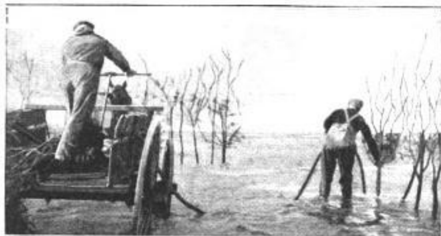
Modern Method of Setting Poles for Fish Traps, Used by Cape Cod Fishermen: The Man on the Wagon Operates a Pump That Forces Water through the Hose Nozzle Held by the Man Standing
