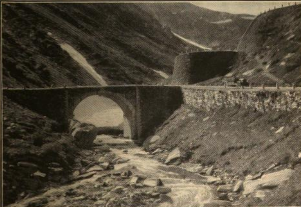
An Even More Rugged Section of the Railway in the Val Tremola, of the Swiss Alps, Where It Descends More than 3,000 Feet from the Southern Entrance of the St. Gothard Tunnel to Airolo, Requiring No Less than 40 Curves: The View Shows the Supporting Walls of Two of Them
