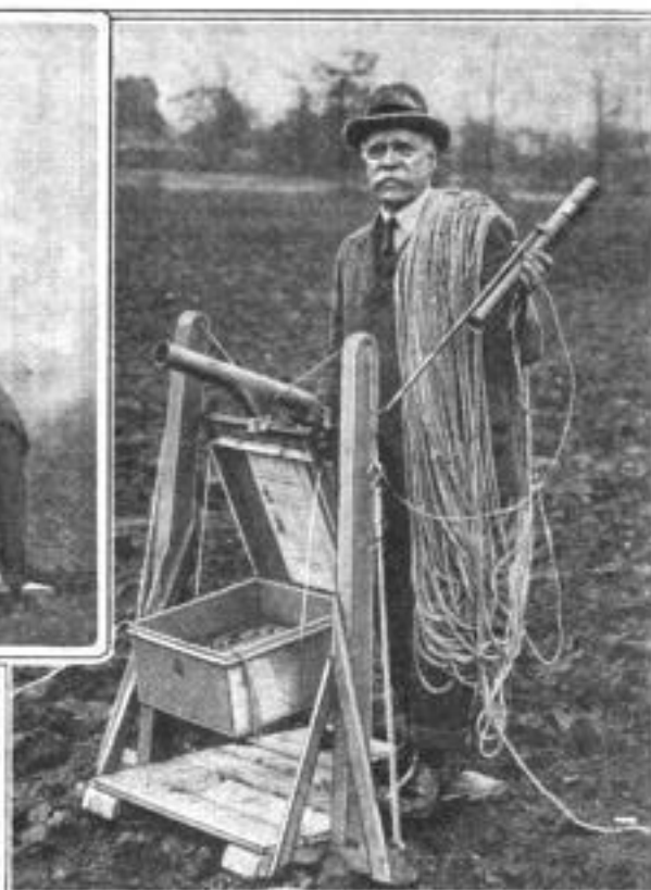
Above: Aiming the Pistol and Firing from It the Rocket Which can be Seen Drawing the Lifeline That is Attached to It. Right: Inventor of the Apparatus Seen Holding in His Left Hand the Steel Rocket to Which the Long Lifeline is Attached. With His Right Hand He is Holding the Pistol, below Which is the Lifeline Box
