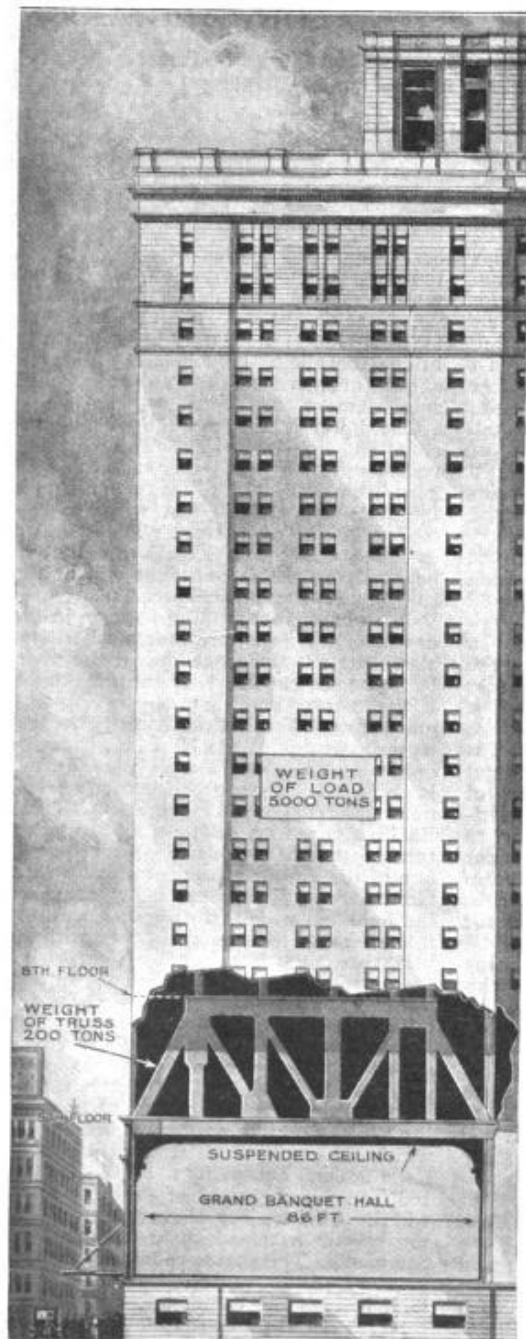
Part of the East Façade of the Hotel, Showing One of the Steel Trusses That Are the Largest of Their Kind in the World
