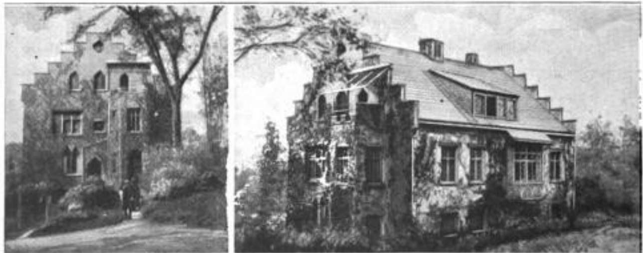
Left: Residence of Horace Greeley's Daughter, Which was Recently Remodeled from a Concrete Barn, Built by the Famous Editor on His Estate Over 70 Years Ago. Right: Another View of the Residence, the Hall of Which Was Formerly the Cow Stalls of Greeley's Barn
