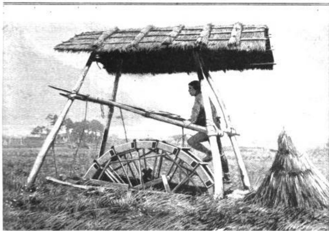
FOOT-POWER MILLS USED TO IRRIGATE JAPANESE RICE FIELDS
