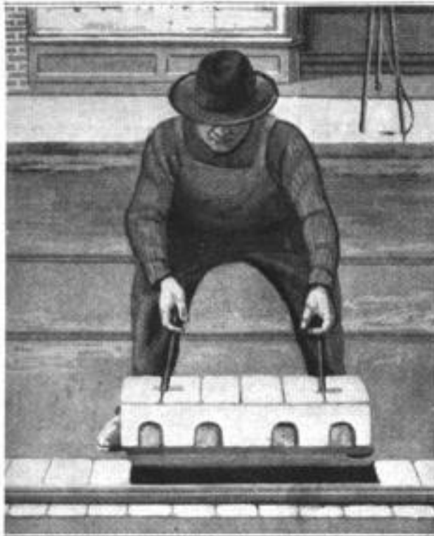
Special Paving Blocks Easily Removable and Replaceable around a Track Joint by Means of a Tripod, or by Hand without the Tripod
