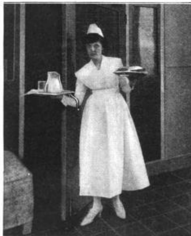
A Hook having been Substituted for the Regular Door Knob, the Nurse can Open the Door with Her Arm
