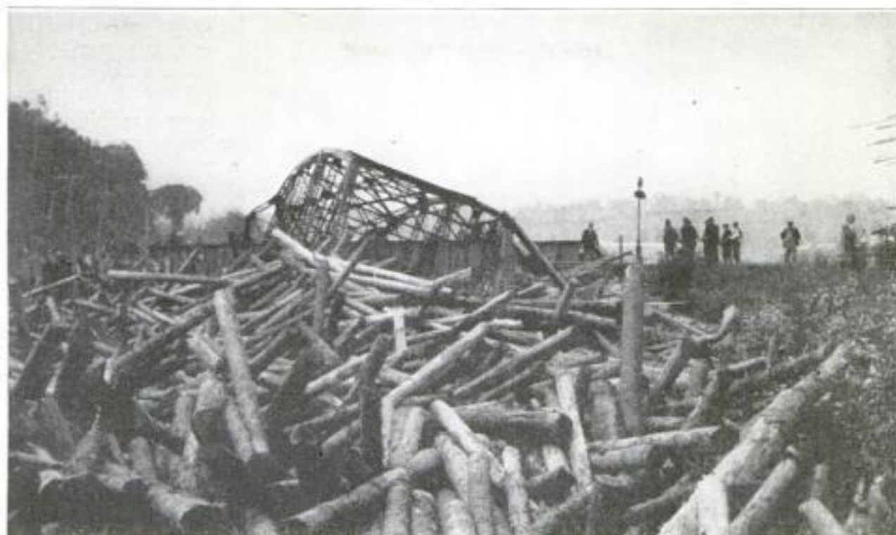
At the Railroad Trestle near the St. John River in New Brunswick, Canada, Where the Runaway Logs and the Bridge were Finally Stopped: The Force of the Jam Was So Great at This Point That the Steel Bridge was Bent over the Trestle, While the Trestle Itself was Pushed Four Feet Out of Alinement
