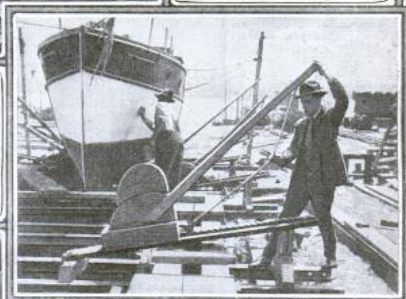
Above: The Bilge Blocks of the Cradles of the Marine Railway are Easily Slid into Position and Automatically Lock in Place under Water. Clamps Hold Them to the Cross Rails of the Cradle and They are Quickly Unlatched by a Jerk on a Cord. Left: Large Iron Sheave Made from Elevator Scraps and Used on the Head of One of the Smaller Cradles. It is Only One of the Many Evidences of Resourcefulness
