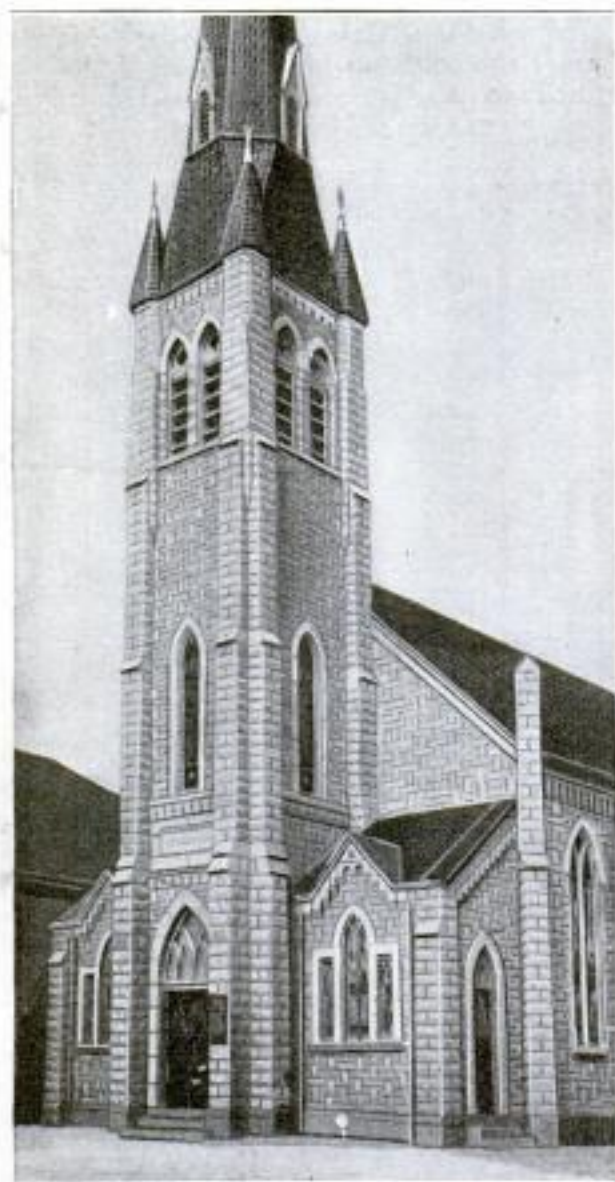
Red-Brick Church in Detroit, Michigan, 50 Years Old, That has been Veneered with Cement and Made to Look like a Church Built of Concrete Blocks
