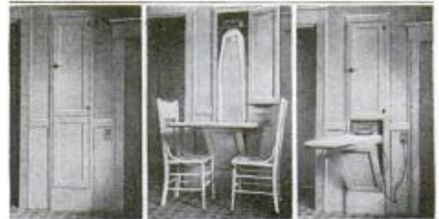
Left to Right: Support and Ironing Board Concealed in Wall; Support Let Down as Table, and Ironing Board Ready for Use
