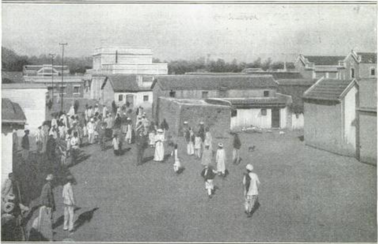
A Congested Part of the City of Bangalore Which has been Greatly Improved by the Removal of Some of the Small Overcrowded Houses, Thus Allowing the Admittance of Fresh Air and Sunlight to the Remaining Houses: This Was a First Means of Plague Prevention
