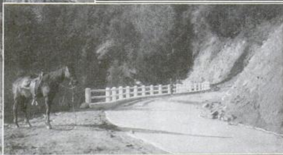
Left: One of the Concrete Viaducts, Built along Cañon Wall 100 Feet above Railroad Tracks, on Highway to "Big-Tree" Country. In Places, the Outer Edge of the Viaducts were Supported by Bents 20 Feet High. Right: One of the Curves of the Big-Tree Highway
