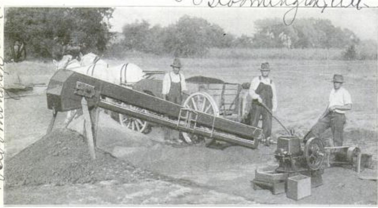
Sand, Soil, and Humus Mixer: In the Foreground Is the Gasoline Engine, Belted to the Shaft That Drives the Inclined Conveyor over the Screen. The Fine Particles of the Mixed Ingredients are Seen underneath the Screen, While the Lumps and Foreign Matter are Shown below the Raised End
