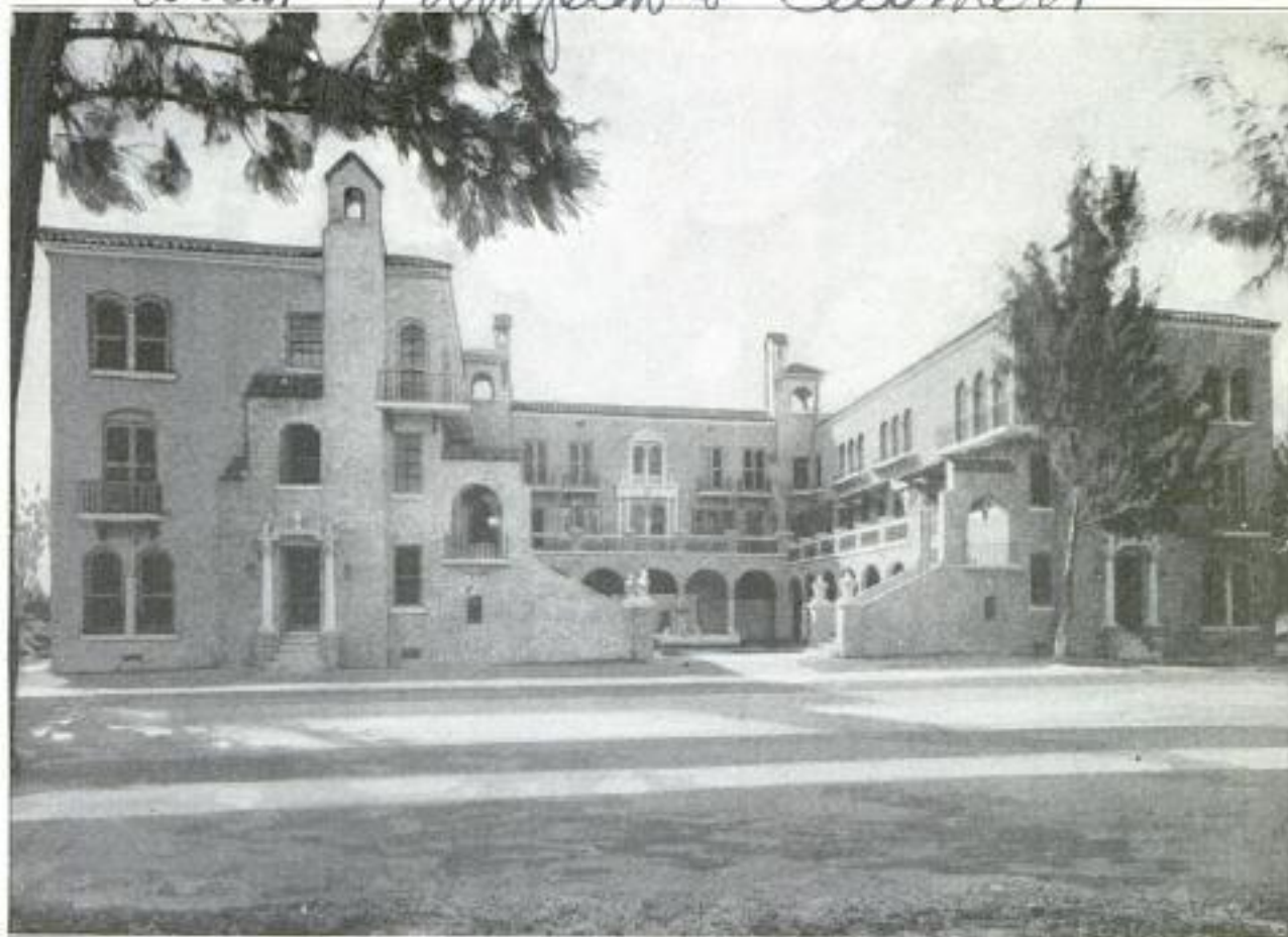
A Departure from Conventional Lines of Architecture is Seen in This Beautiful Apartment Building Which has been Erected at Miami Beach, Florida. The Walls are Treated with Waterproofed Stucco of a Two-Tone Mottled Design. Red Tile Cover the Court and Floors of the Gallery
