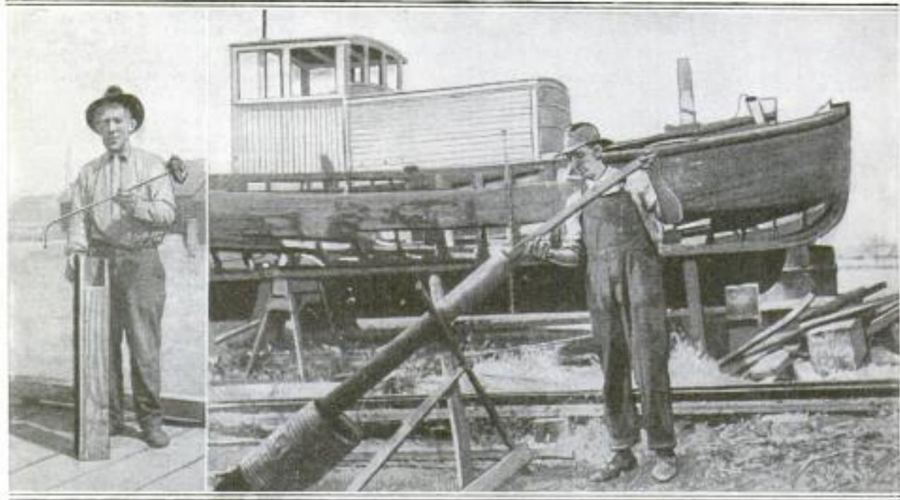
Left: Simple Emergency Pump Made of Four Strips of Wood, Four Inches Wide, Nailed Together to Form a Long Box. A Square Piece of Flexible Leather Bolted to the Handle Acts as a Check Valve. Right: A Four-Inch Iron Pipe Serving as an Improved Steam Box, Used in Bending Ribs for a Quick Repair Job on the Launch in the Background
