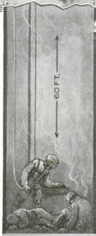
This Illustrates How a Threshing-Machine Blower, Driven by an Automobile Engine, was Used to Purge a Gas-Filled Well from Which It was Desired to Remove the Bodies of Two Men Asphyxiated There
