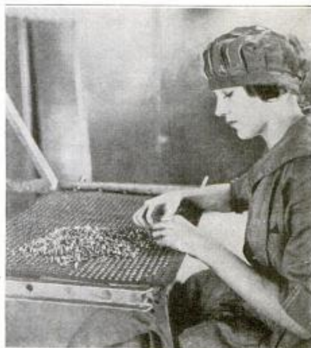
Perforated Plate in Which Small Bolts are Inserted for Painting Their Heads: This Plate Holds 1,800 Bolts, and It Takes 45 Minutes to Insert Them
