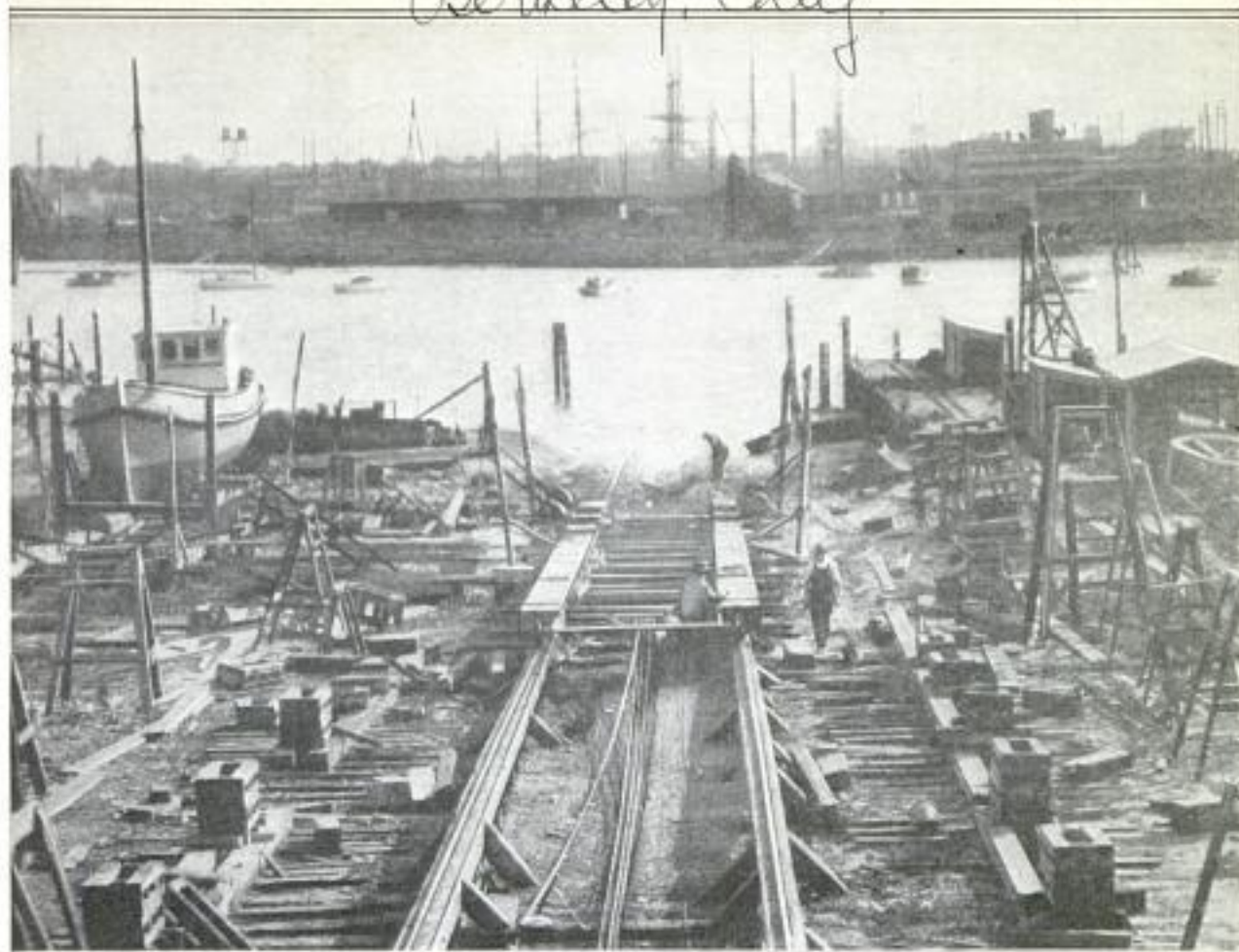
A View of the Lower End of the Bagley One-Man Shipyard, Looking toward the Water: The Marine Railway, on Which Vessels are Hauled High and Dry on the Land, and Its Largest Cradle Appear in the Center of the Picture, Which was Taken from the Roof of the Main Building
