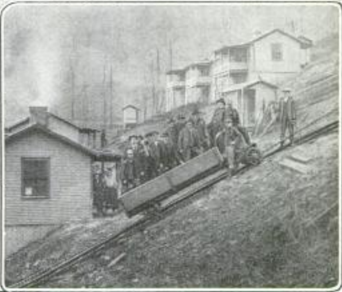
Above: Safety Car near the Top of Incline, Stopped Automatically after Running 25 Feet with the Hoisting Rope Cut. Upper Left: Side View of Car with Hood Open, Showing Details of Safety Device. Right: Car on Grade with Hoisting Rope Disconnected
