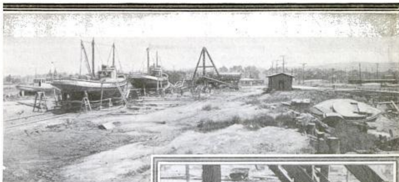
Above: A Continuation of the Bagley One-Man Shipyard from the Same Viewpoint, Showing Two Vessels Hauled High and Dry on the Marine Railway. Right: A Wood-Turning Lathe, Which Holds Anything from Dowels Up to Flagpoles and Rudder Posts, is Assembled on a Wooden Form, from Odd Parts of Machinery Picked Up Here and There
