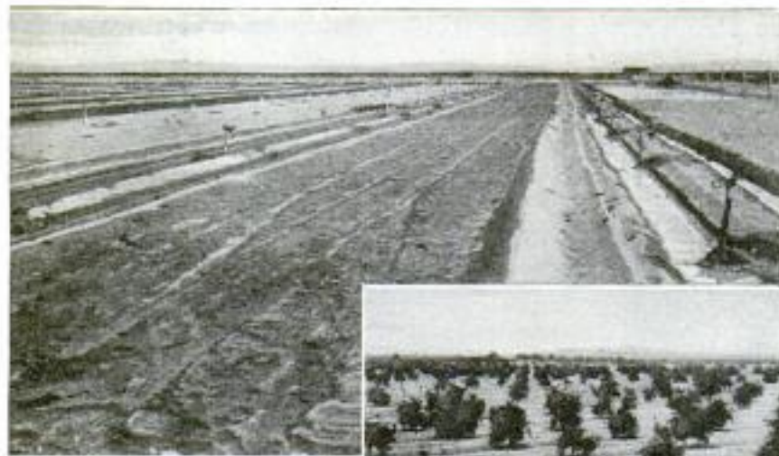
A Citrus Orchard in the Planting on the Mesa of the Yuma Irrigation Project, in Southern California
