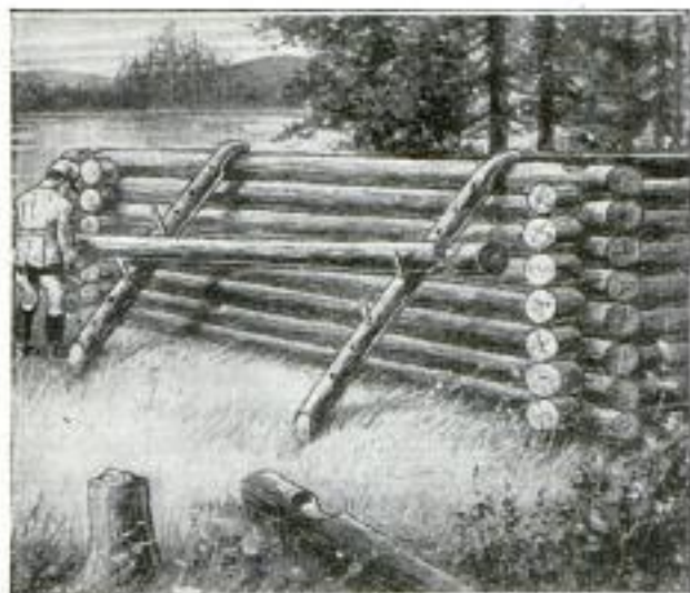
Placing the Logs, Used in Constructing a Stable, by Means of Skid Poles, Enabled One Man to Do the Job Alone
