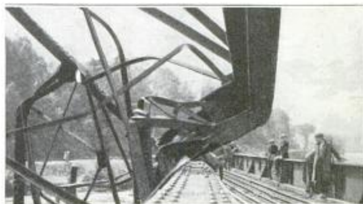
The Great Power behind the Thousands of Logs Piled Up in the Stream is Clearly Demonstrated by This Picture, Which Shows How the Heavy Steel Bridge was Bent over the Trestle
