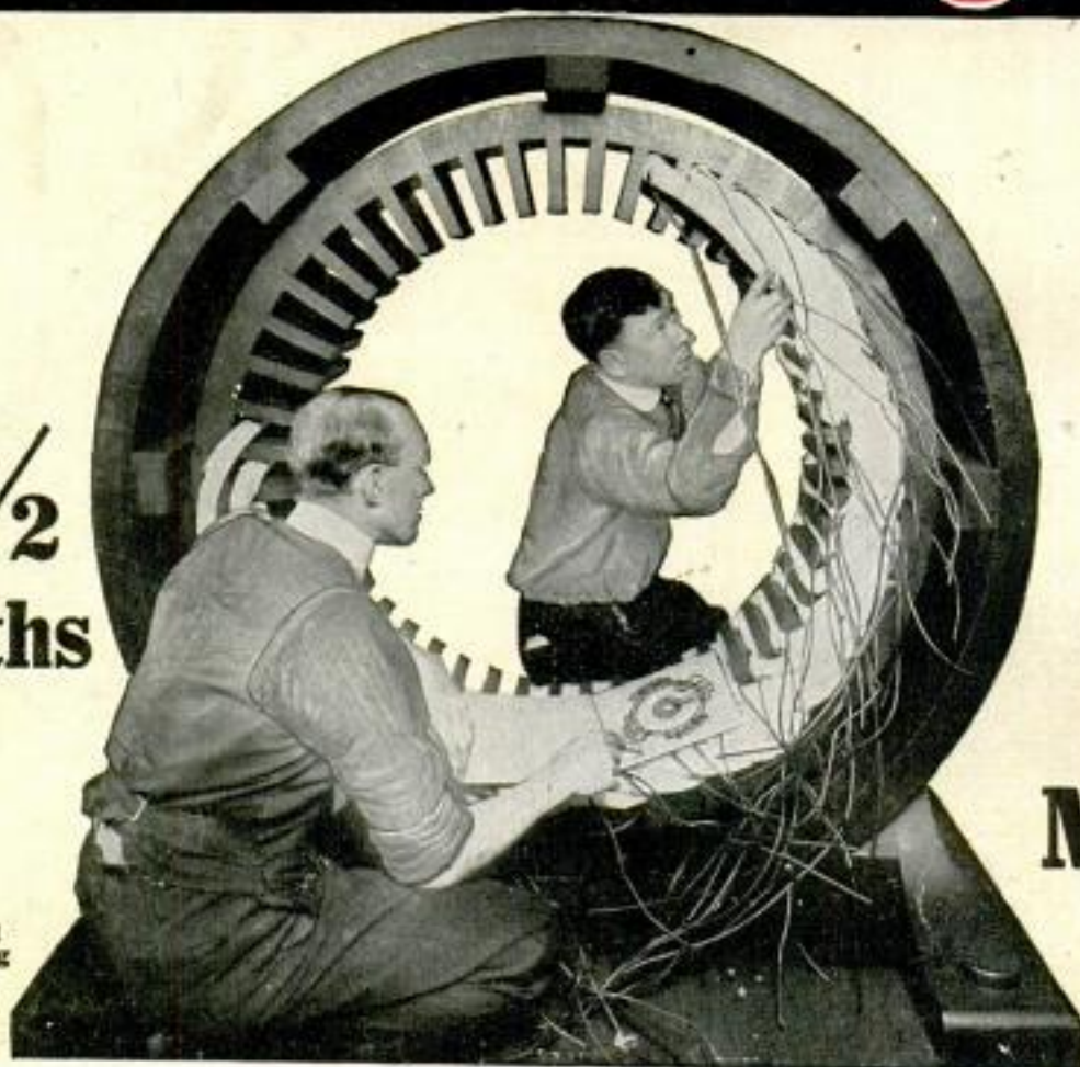
Student Winding Stator
