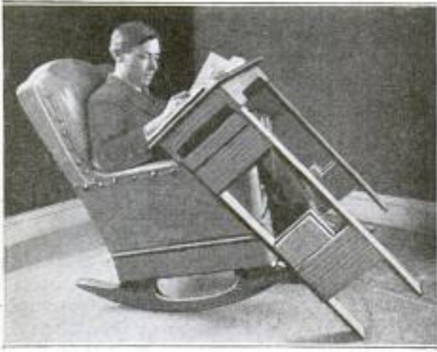
This Convenient Reading or Writing Table can be Tilted at the Proper Angle for Fatigue Elimination and for Comfort
