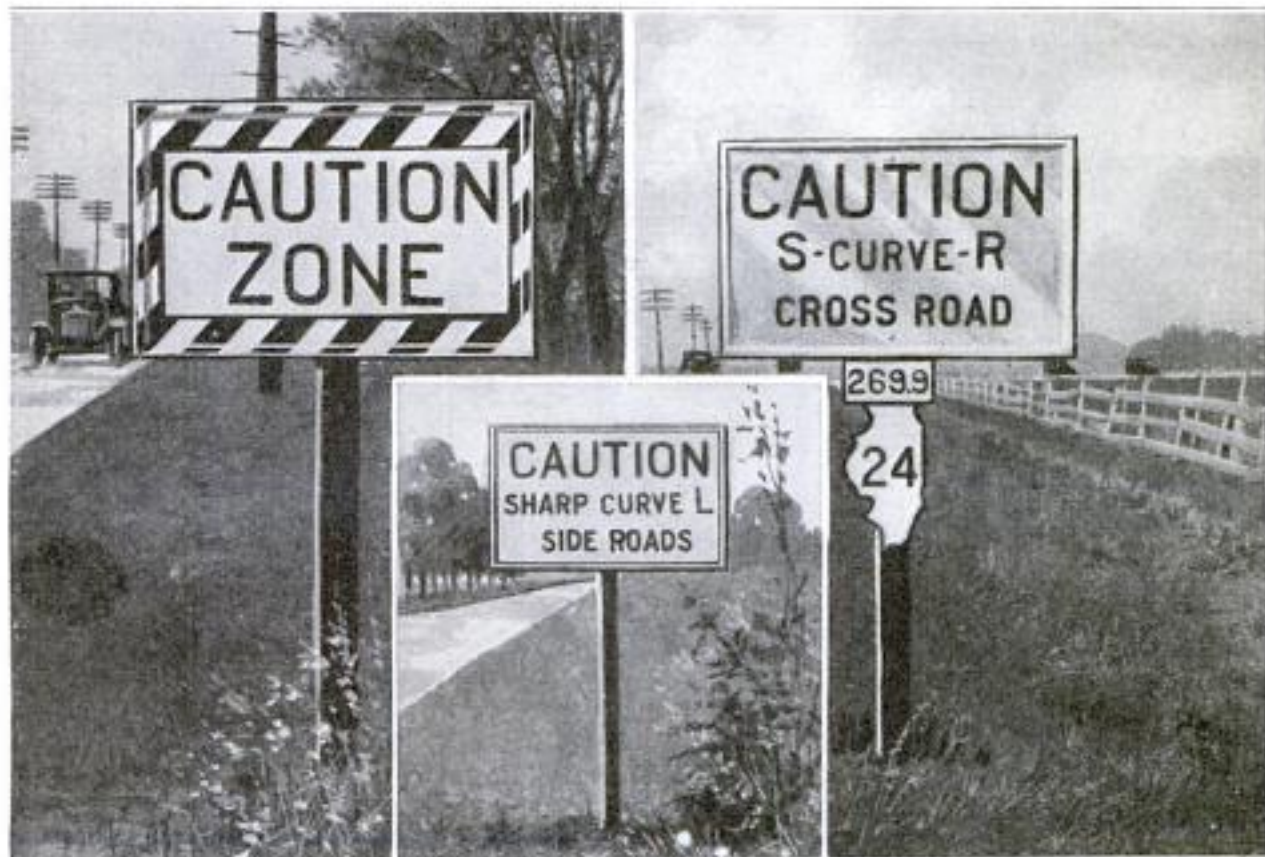
Left: Signs Indicating Caution over a Certain Distance Have Black Letters on a White Field with Diagonal Black and White Border. Center: Sign Denoting the Reason for Caution. Right: This Black-and-White Sign Indicates Slowing Down, and Degree of Care Necessary
