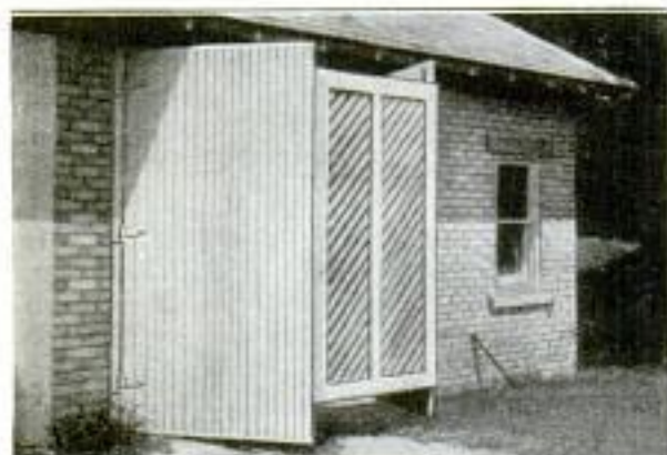
A Lattice Gate, Hinged to One Garage Door and Hooked to the Other, Keeps Undesirables Away When the Owner is Working on the Car
