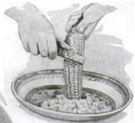
Sweet-Corn Slicer That Quickly Cuts the Corn from the Cob: It Has an Adjustable Blade, Guarded to Prevent Accidents
