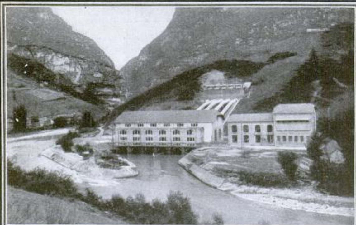
Hydroelectric Plant on the Fier River in France: On the Side of the Mountain can be Seen the Bulkheaded End of the Tunnel, and the Penstocks Which Conduct the Water to the Turbines in the Power House Below
