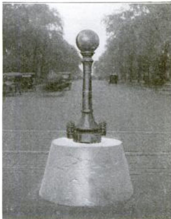
This Street Signal Has the Usual Large Red Globe and Two Additional Smaller Red Lights near the Base, to Indicate a Railway Crossing
