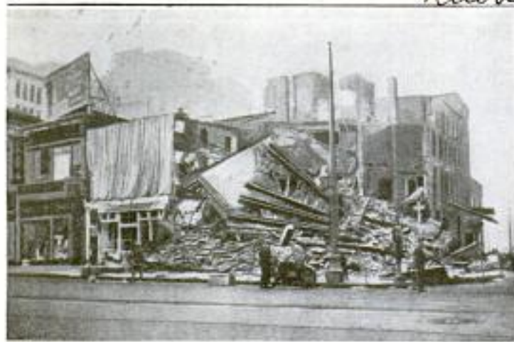
Ruins of the Two Buildings Which Collapsed Because of Excavations being Made underneath One of Them, Showing the Havoc Caused and the Narrow Escape of the Inmates
