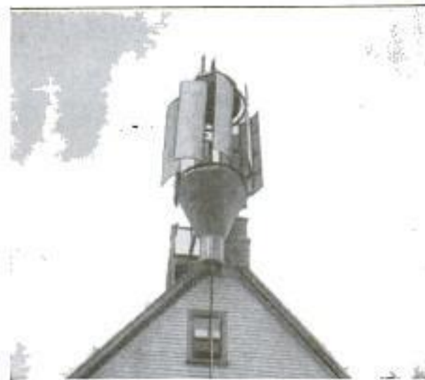
Eight-Vane Windmill Which Supplies Electric Current to the Dwelling on Which It is Erected
