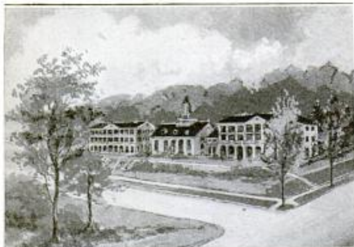
The Hospital Group of Buildings Which are Situated near the Convalescents' Home
