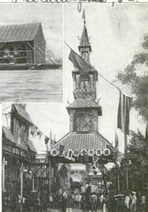
Bamboo Archway and Tower over a Street in Canton: There Is Not a Nail Nor a Peg in the Entire Structure. The Covering Is of Oiled Paper
