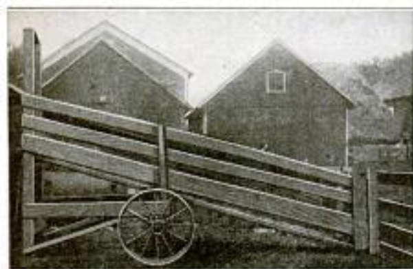
A Substantial Homemade Stock Loader That can be Moved to Any Point on the Farm
