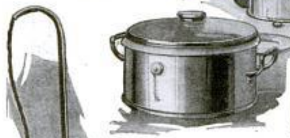
Heat-Retaining Dish in Which the Housewife may Prepare Food before Mealtime and, Due to the Vacuum Insulation of the Dish, Keep the Edibles Steaming-Hot until the Proper Serving Time
