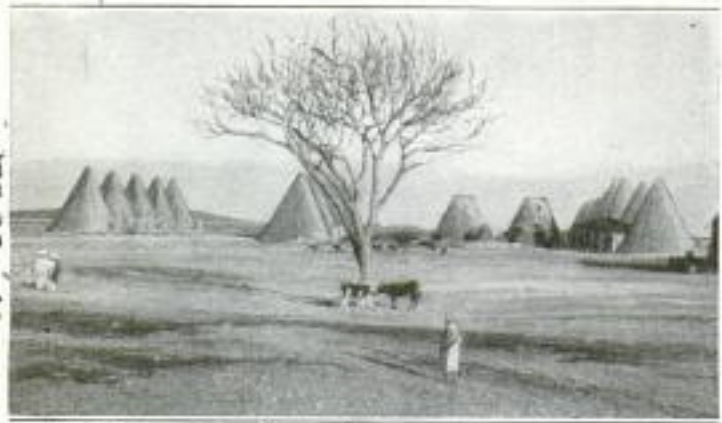
Conical Concrete Silos for the Storage of Corn in Mexico: They are Well Built, of Concrete Made with the Best Portland Cement, and Preserve the Corn for Use in Lean Seasons
