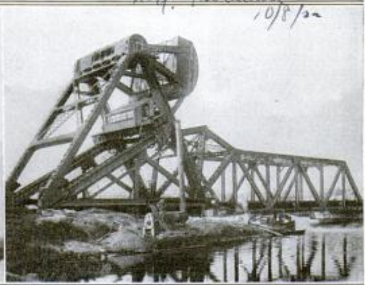
Left: New Type of Bascule Bridge Operated by a Moving Counterweight, Shown Open with the Counterweight Moved Down into the Supporting Tower. Right: The Bridge is Shown Closed with the Counterweight Moved Radially Upward, So That It Hangs Directly above the Bridge Trunnions
