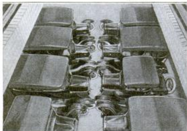
This Picture, Showing Eight Automobiles Parked in the Furnace of One Boiler, Gives an Idea of the Unusual Proportions of the Boiler
