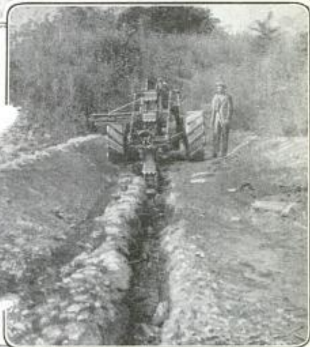
Above: A Tractor, Equipped with New Trench-Digging Machinery, is Here Shown Ready to be Transported. Right: Tractor Trench Digger at Work on Deep Vertical Ditch. Below: Another View of the Tractor with the Attachment by Which It is Converted into a Trench Digger in an Hour
