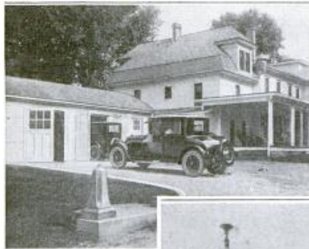
Automobile Approaching a Garage Entrance, and Opening the Door by the Action of a Plate Pressed Down by the Weight of the Car
