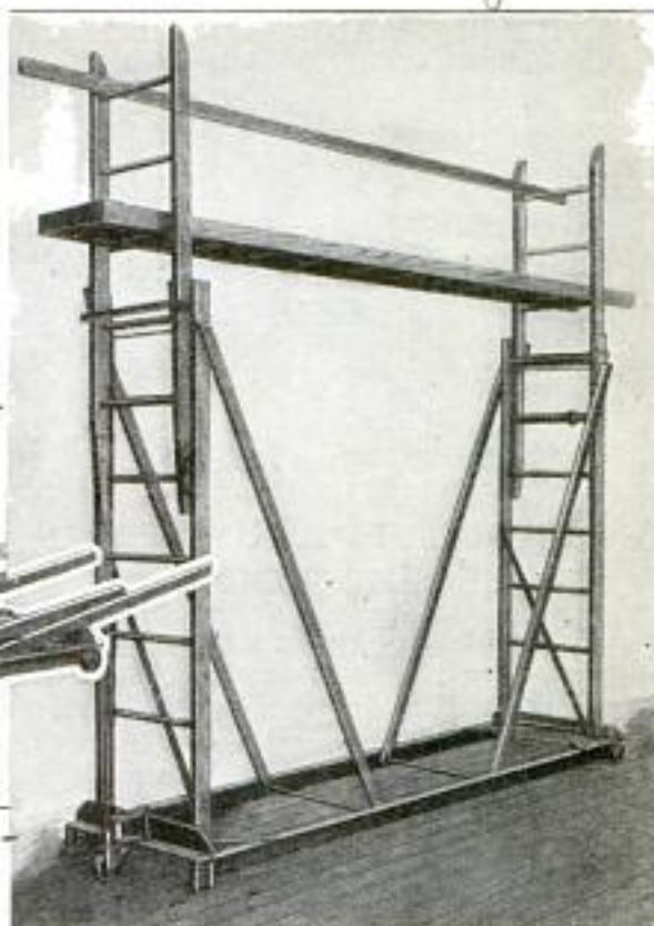
Above: Portable Scaffold Collapsed, Showing Steering Handle and Wheel. Right: Scaffold Shown Solidly Erected, Ready for Use
