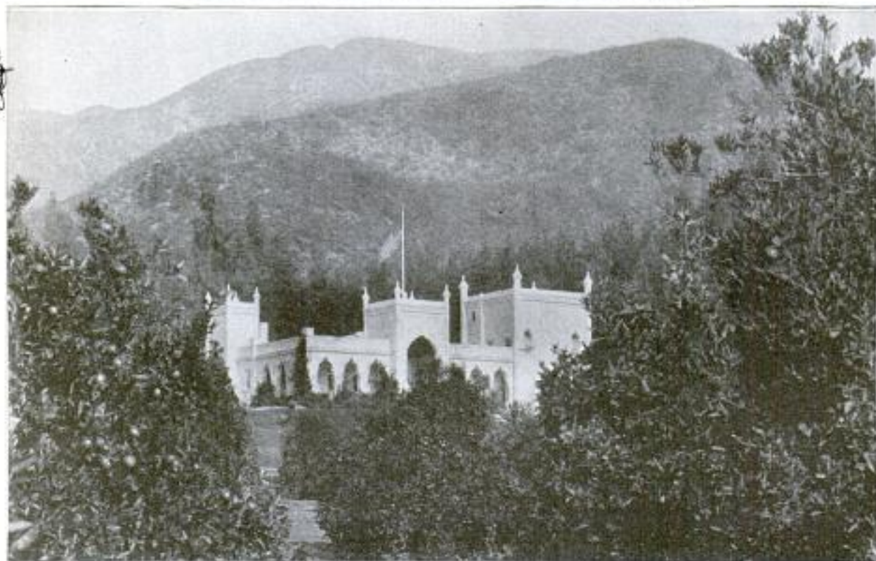
Above: Entrance to a California Estate, Which is Made of Concrete and Ornamental Ironwork. The Large Pillars Are 26 Feet High and the Smaller Ones 16 Feet High. Below: The White Walls and Slender Turrets of This Castlelike Home are Built of Concrete
