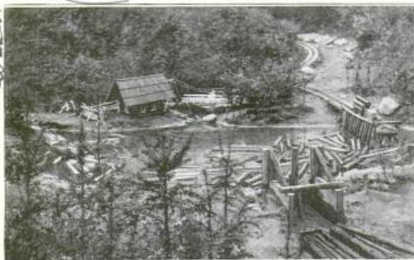
Above: Miniature Splash Dam Built by Students of the Forestry College and Engineering Branch of the University of Washington. At the Right Is the Working Model of a Water-Power Plant, Together with a Roadway, Tunnel, Bridge, and Transmission Poles, All Made of Concrete
