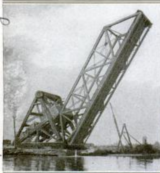
Left: New Type of Bascule Bridge Operated by a Moving Counterweight, Shown Open with the Counterweight Moved Down into the Supporting Tower. Right: The Bridge is Shown Closed with the Counterweight Moved Radially Upward, So That It Hangs Directly above the Bridge Trunnions
