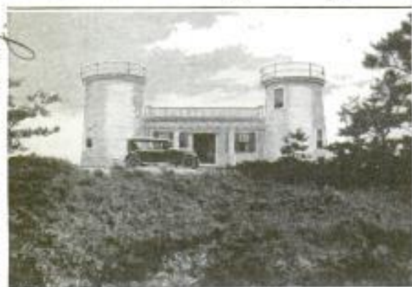
The Tower Wings of This House Were the Base Sections of Two Condemned Lighthouses Which the Owner Was Able to Buy for a Small Sum
