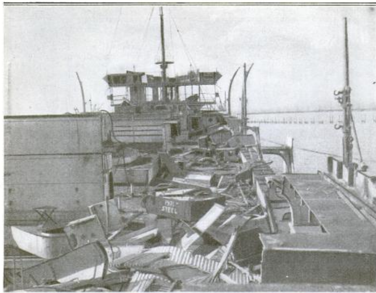
Another View of the "Minneapolis," Showing the Deck After the First Course of Steel Plating had been Removed for Part of the Distance around the Ship; This Illustrates the Effectiveness of the Gas Torches in Reducing the Heavy Armor Plate of Battleships to Salable Junk
