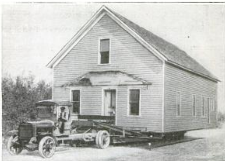
Above: First of the 80 Houses being Moved from Jennings to Cadillac. Right: Backing the Trailer under the Jacked-Up House
