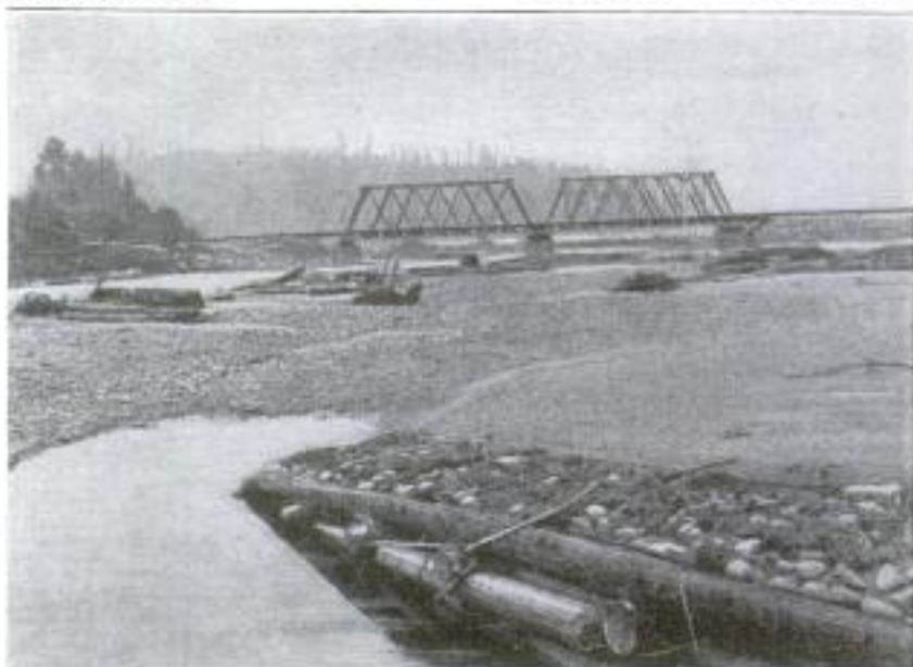
View of River during the Dry Season, Showing the Railway Bridge in the Background and One of the Jetties with the Sand Bar Which It Caused to Form in the River Bed
