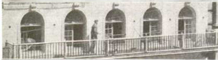
Ornamental Balcony Which has been Designed to Conceal a Gravity-Type Fire Escape, Showing a Man About to Descend
