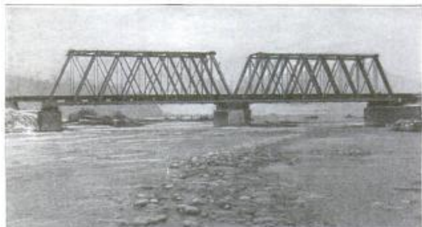
Railway Bridge with Two 100-Foot Openings Bottling Up the River Which Was Formerly Nearly a Mile Wide at Its Mouth
