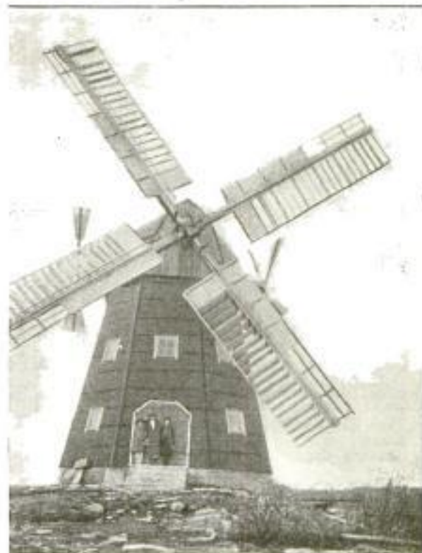
Old Windmill on an Island in Lake Vänern, Sweden: The Mill is Built Entirely of Wood, Including Its Driving Shafts and Gears
