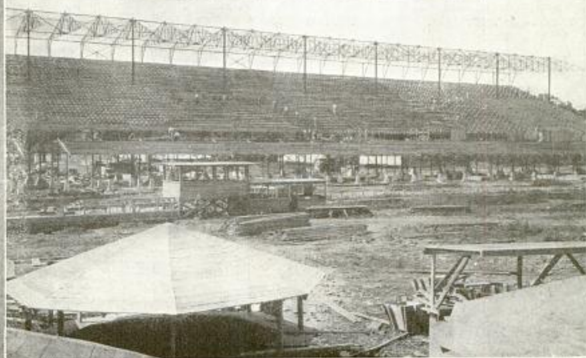
Large Automobile Speedway. Below: Large Steel Grand Stand Erected in Seven Days
