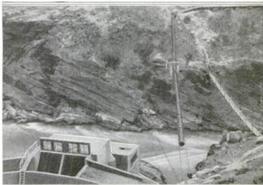
View of the Part of the Raceway Where It Enters the Power House, the Top of Which is Seen in the Immediate Foreground
