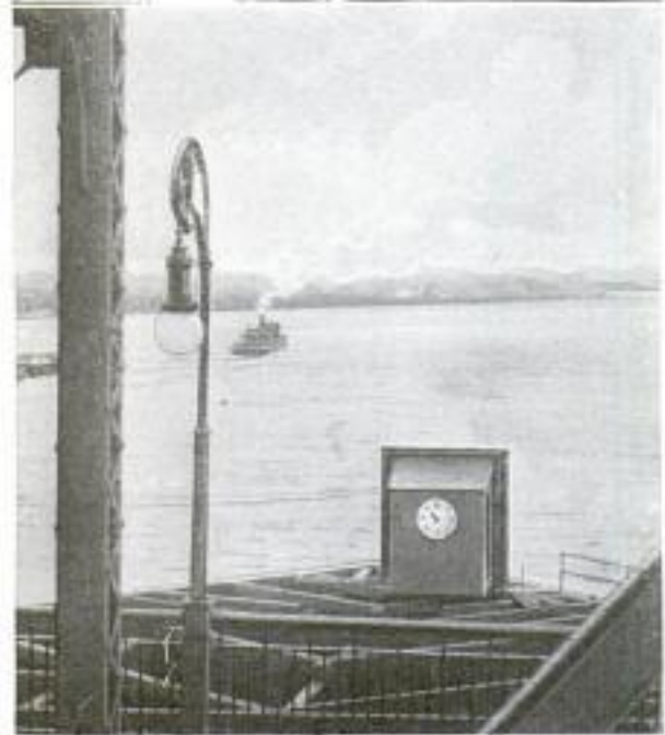
International Tide Gauge on a Bridge across the Potomac River Shows at Any Time the Number of Feet of Clearance between the River and the Bridge
