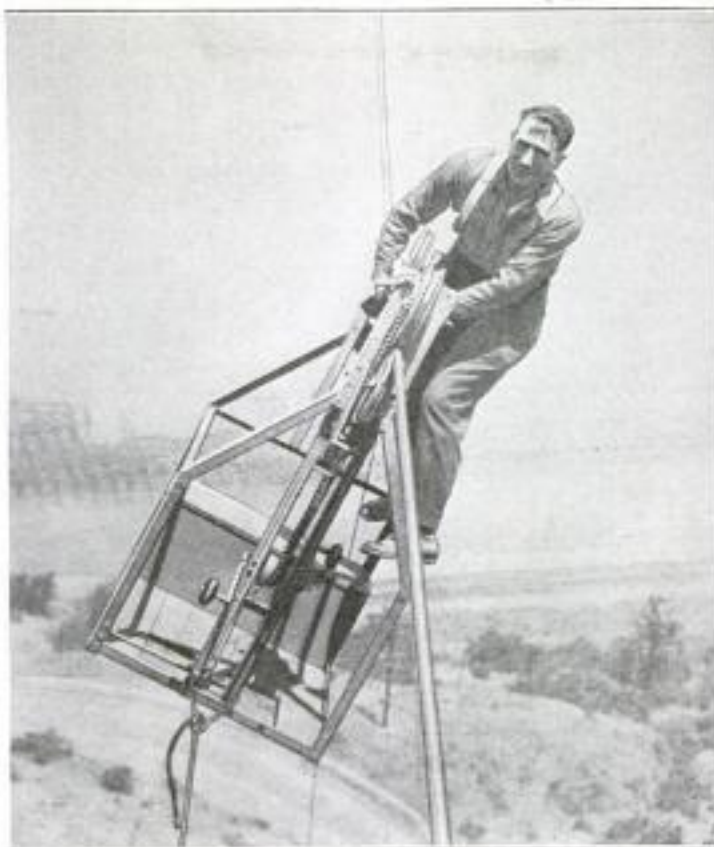
Little Car in Which "Pete" Lindsay, the Fearless Line Foreman, Coolly Trolleyed Out upon the Damaged High-Tension Transmission Cable to Make the Necessary Repairs
