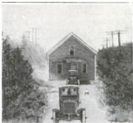
Above: First of the 80 Houses being Moved from Jennings to Cadillac. Right: Backing the Trailer under the Jacked-Up House
