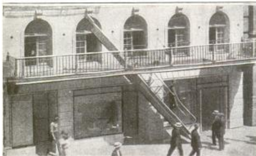
Here the Fire Escape is Shown Lowered by the Weight in the Front End, and a Man is Seen Descending It
