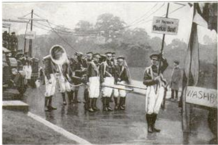
Parading Band without Instruments, Showing the Batteries and Receiving Set on the Litter, the Amplifying Horns, and the Portable Antenna
