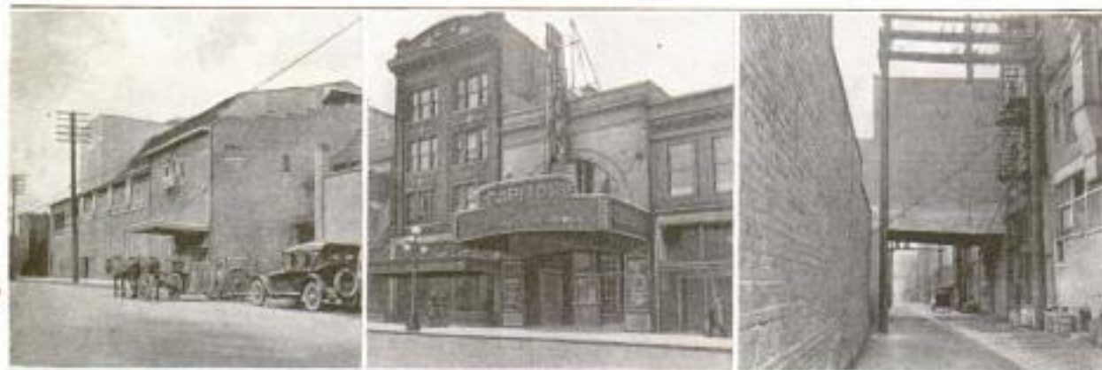
From Left to Right are Shown: The Frontage of the Theater on the Back Street Where Property Is Cheap; the Front Entrance to the Theater on the Busy Main Street Where Property Is Expensive, and Part of the Approach That Spans an Intersecting Alley without Interference with the Traffic.
