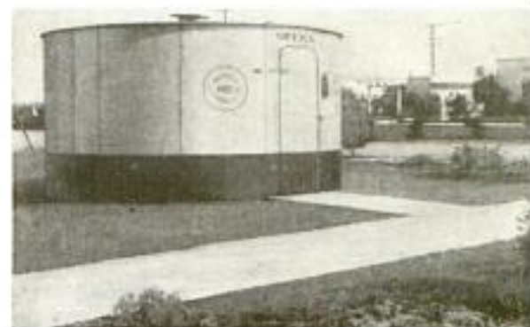
Appropriate Office of an Oil-Tank Salesman in a California Town
