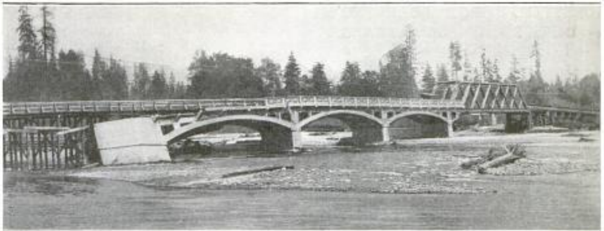
General View of Highway Bridge, Showing How the River Turned from One Side to the Other in Sweeping Out Both Approaches with Its Swift Current: Note Temporary Truss over the Most Easterly Span, and the Temporary Structure at Each Approach
