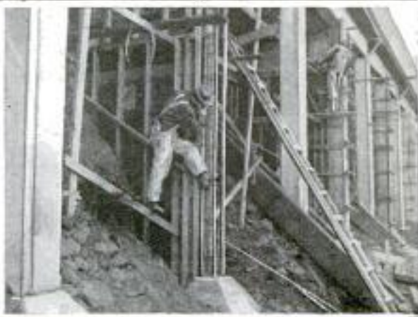
Top: Concrete Mixer, on the Viaduct, from Which Workmen are Taking the Mixture in Wheelbarrows to the Forms. Lower Left: Underside View, Showing the New Piers. Lower Right: Workmen Building Wooden Forms in Which the Concrete for the Additional Piers was Poured
