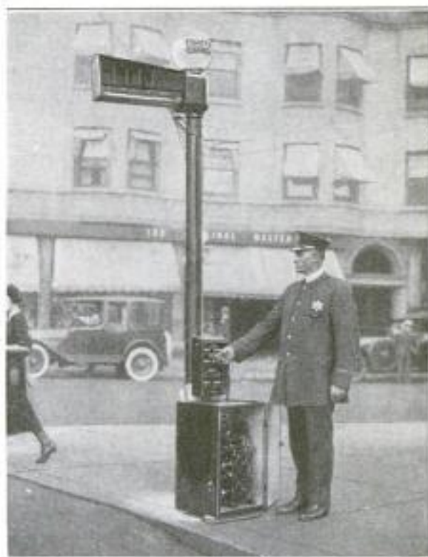
COPYRIGHT, INTERNATIONAL NEWSREEL CORP. Electrically Operated Traffic Signal Which is Controlled from the Curb by Means of Switches
