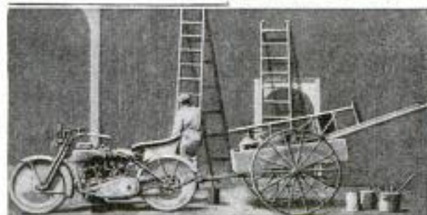
An Easily Made Trailer for Attachment to a Motorcycle and Sidecar: The Pictures at the Center and Left Show the Use of Such an Outfit for Hauling Painting Equipment. Right: The Same Equipment Used for Hauling Supplies to the Farm
