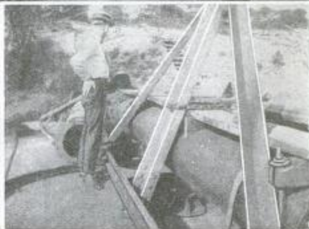
Dredge That Clears a River Channel and Builds Dikes or Levees on Shore: At Left and Above Are Two Views of the Derrick That Projects from the Stern of the Boat, and Has a Rotary Cutter at the End of It. At Right are Shown the Pipes That Connect the Vessel with the Shore
