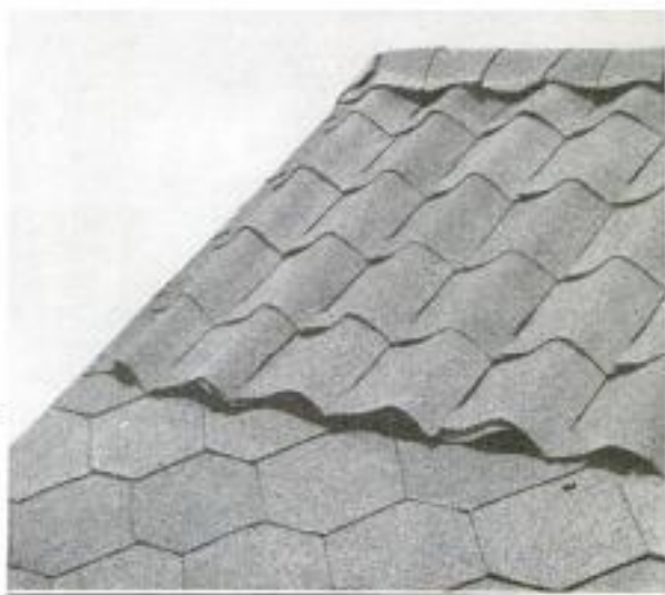
Roof Covered with New Composition Shingles, Which can be Laid Flat in a Geometric Pattern, or So as to Resemble Tile
