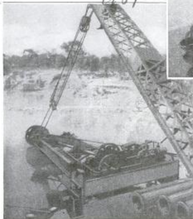
Dredge That Clears a River Channel and Builds Dikes or Levees on Shore: At Left and Above Are Two Views of the Derrick That Projects from the Stern of the Boat, and Has a Rotary Cutter at the End of It. At Right are Shown the Pipes That Connect the Vessel with the Shore
