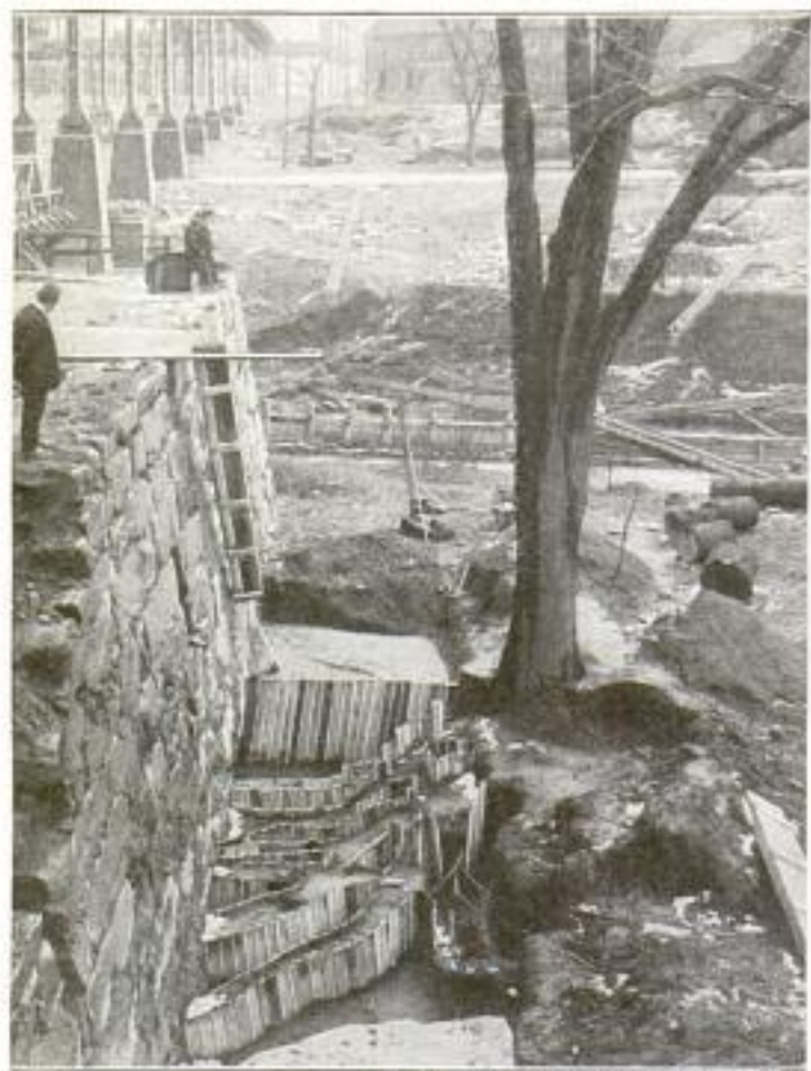
BY COURTESY OF THE AMERICAN FORESTRY ASSOCIATION Earth-Filled Channels were Formed to Protect the Roots of This Tree Where They Crossed the Excavation for the Foundation
