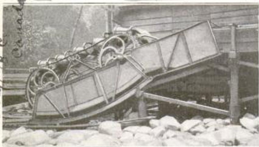
Side View of Motor for Use with Low Water Heads and Swift Currents: The End of the Water Flume Is at Extreme Right
