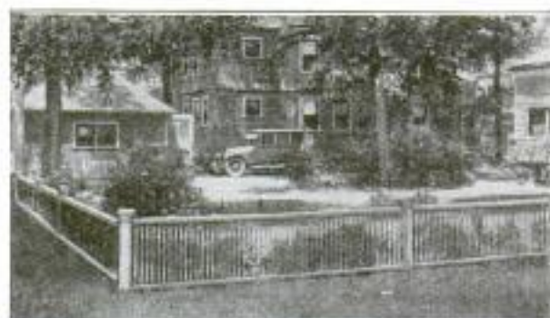
The Owner of a Suburban Home Removed the "Ornamental" Railing Which Style Demanded When the House was Built, and Used It to Make a Neat Fence
