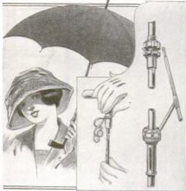
Left: Neat Appearance of the Wireless Umbrella. Insert: Manner of Attaching Handle, Also Ball-and-Socket Joint of the Ribs
