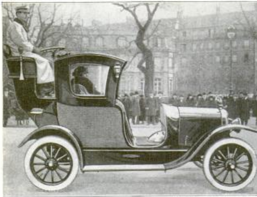
Here is Pictured the Hansom Cab of Today, Built on a Light American Automobile Chassis. The Only Missing Parts Are the Shafts and Horse. The Driver's Seat Being in the Rear, the Passenger Enjoys an Unobstructed View and a Feeling of Greater Privacy
