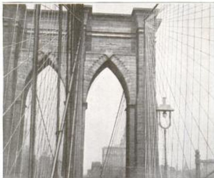
View of Brooklyn Bridge, Showing One of the Main Piers with Two of the Suspension Cables and Network of Smaller Cables Supporting the Decks
