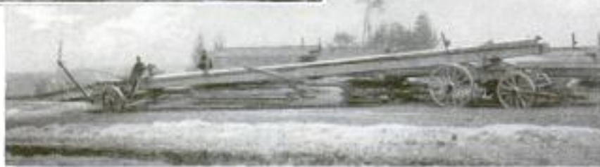
Full-Length View of the Rig, Showing That It would Be Impossible to Haul Such Long Timbers without the Special Steering Gear at the Rear
