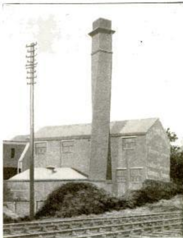
Spiral Smokestack, Built in England, with a Quarter Turn from Bottom to Top, Causing Less Resistance to the Wind than if Built with Vertical Sides
