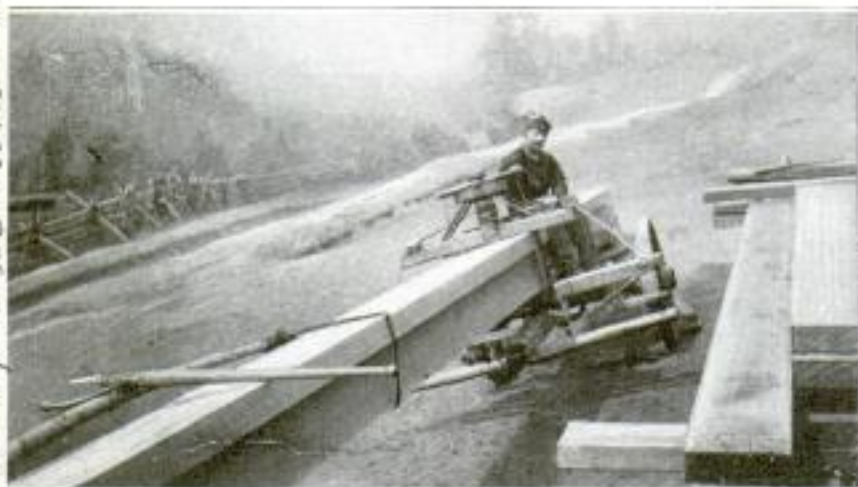
Rig for Hauling Long Bridge Timbers around Sharp Curves: The Man is Operating the Steering Apparatus of the Rear Truck
