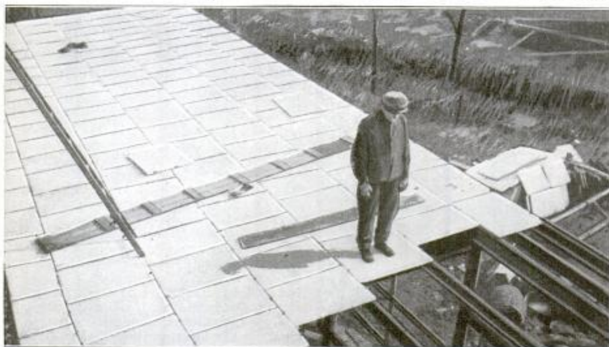
Construction of a Roof Deck with Slabs of the New Kind of Reinforced Concrete: These Slabs Are Only an Inch Thick, and Are of a Porous Structure. When Used for Such Purposes as Roofing or Flooring, the Slabs are Covered with a Thin Cement Finish
