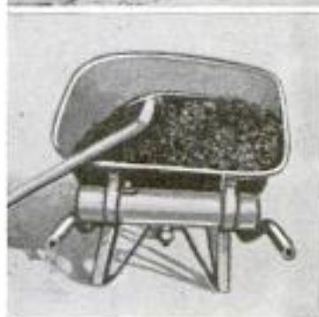
Above: Wheelbarrow Which Has a Gasoline Heater Incorporated in It for Facilitating Road Repairs. Below: Interior, Showing Road Material being Heated. The Fuel Tank is Seen between the Handles
