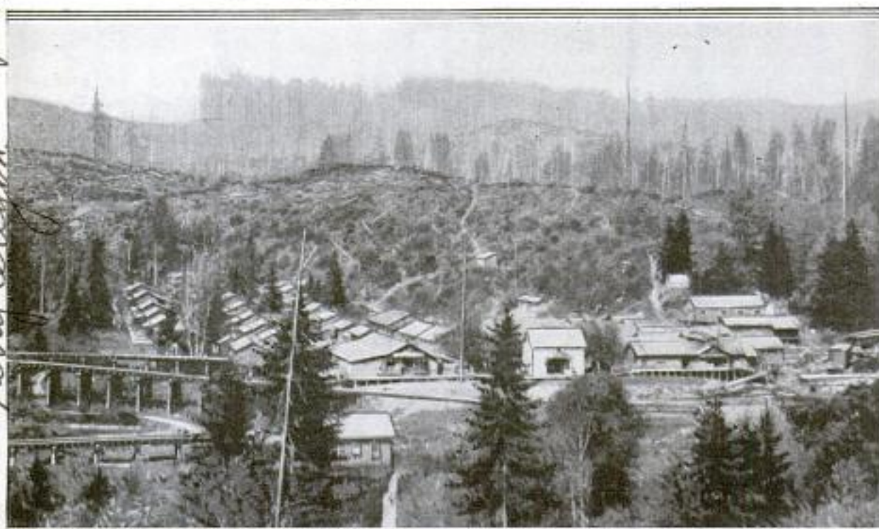
View of Western Lumber Camp Where a Single-Wire Antenna, 1,015 Feet Long, was Erected in Connection with a Radio Outfit Installed for the Entertainment of the Somewhat Isolated Inhabitants
