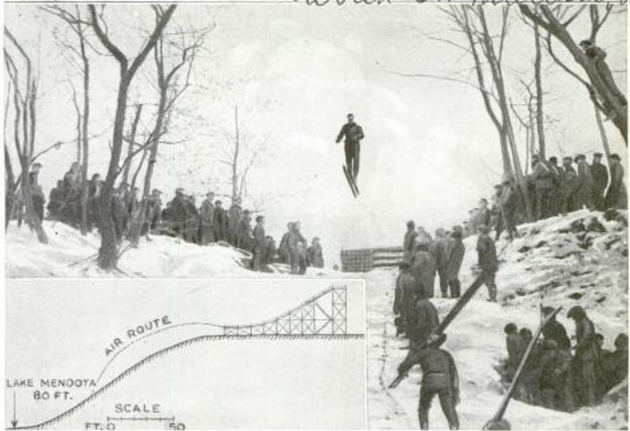
Ski Slide at the University of Wisconsin That was Designed Mathematically to Make Possible a Leap of 115 Feet; Inset Shows the Profile of the Ski Slide Drawn to the Scale Given Below. The Dotted Line Shows the Path of the Skis of a Jumper with a Fall of 58 Feet
