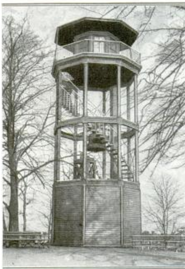
Old Tower and Bell, Relic of Early Fire-Alarm System, Still Standing in Mount Morris Park, New York City, Which at One Time Had a Number of These Bell Towers
