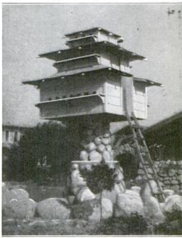
This Bungalow-Type Pigeon House Rests on a Pillar Made of Cobblestones That are Set in Cement
