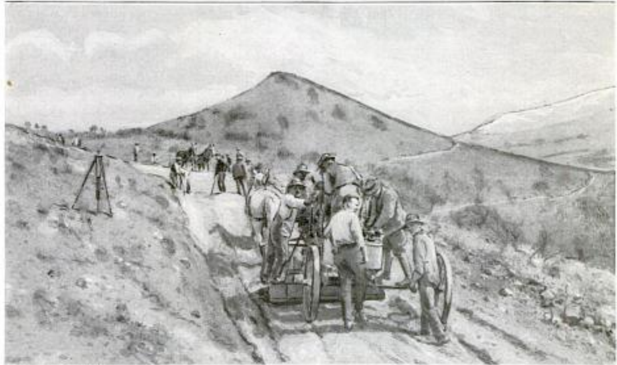
Grading a Portion of the Great Circle Drive: In the Center Is Tenderfoot Mountain with the Spiral Drive Showing at Two Places on the Side, as It Winds up the Mountain
