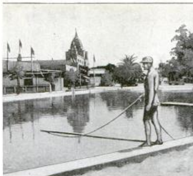
A Simple Method Used by a Swimming Instructor to Keep the Surface of an Open-Air Swimming Pool Free from Dust, Sticks, Paper, and Other Débris Blown into the Tank: Left, the Device in Use; Right, the Débris is Collected at a Corner of the Tank
