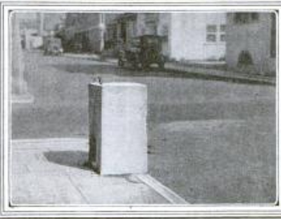
Below: At Venice, California, These Concrete Blocks Containing Electric-Light Connections have been Erected So That Temporary Light Posts may be Placed on Them and Connected
