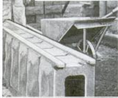
Above are Shown Two Forms of the Mortar-Stringing Apparatus Which was Designed for the Purpose of Speeding Up the Work of the Stone Mason. At the Left can be Seen a Row of Concrete Blocks That are Standing on End and upon Which have been Laid Two Symmetrical Strings of Mortar Preparatory to Placing Them in the Wall
