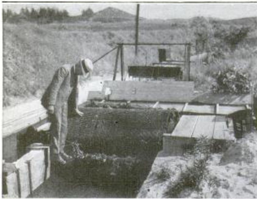
Débris Remover of Irrigation Canal. Showing Fingers of Cylinder Supporting a Man's Weight: In the Background is Shown the Paddle Wheel
