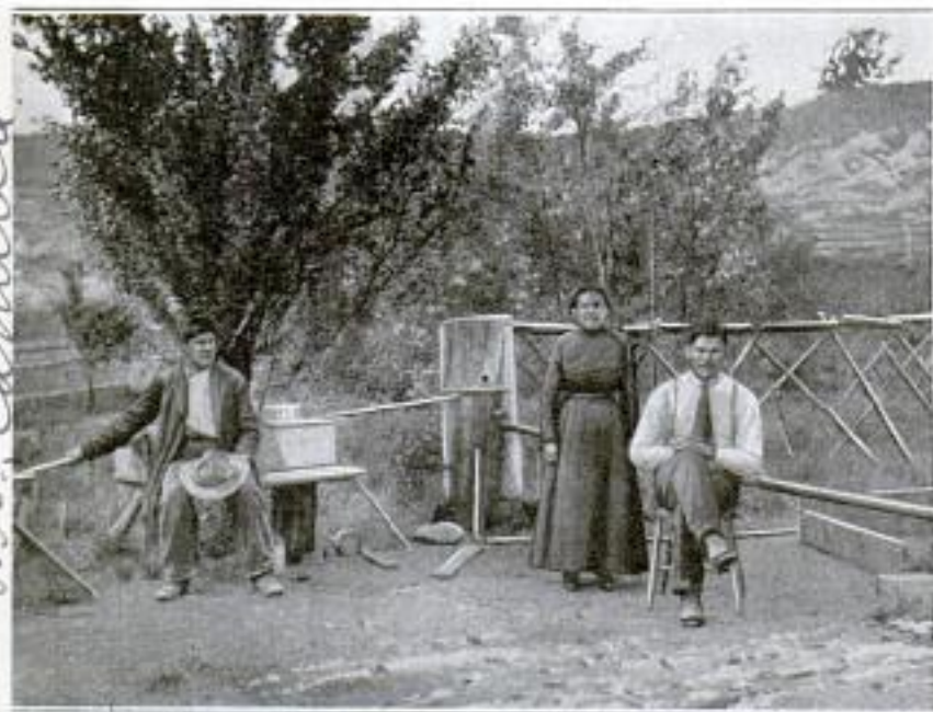
Water is Brought by Gravity from a Near-By Stream to This Cedar-Stump Reservoir and Distributed through Pipes for Refrigeration and Household Use
