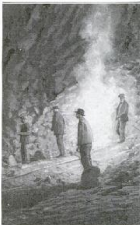
The Rock Salt as It Appears after having been Broken Down by the Charges of Dynamite
