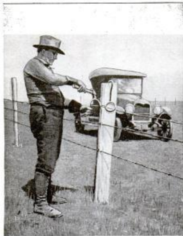
Using a Hay Hook to Pull the Staples from Wire Fence Greatly Reduced the Labor Involved
