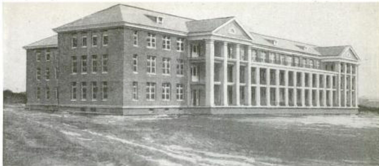
One of the Fireproof Dormitory Buildings of New York State's Great New Hospital: The Building Is of Brick, Steel, and Concrete Construction. Even the Floors Being of Concrete Covered with Linoleum. Large Airy Rooms, Wards, and Broad Screened Porches are Provided for the Patients
