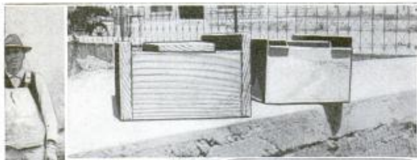
Above are Shown Two Forms of the Mortar-Stringing Apparatus Which was Designed for the Purpose of Speeding Up the Work of the Stone Mason. At the Left can be Seen a Row of Concrete Blocks That are Standing on End and upon Which have been Laid Two Symmetrical Strings of Mortar Preparatory to Placing Them in the Wall
