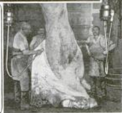
Above: Close-Up of the Electrical Skinning Tool. Showing the Blades of Clover-Leaf Design Which are Revolved at a High Rate of Speed. Below: Skinning a Steer with the Electrically Driven Tool
