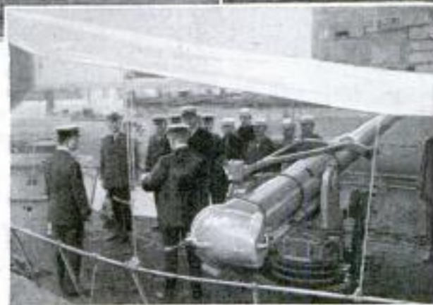
Formal Acceptance of the "S-50" at Bridgeport, Connecticut, by Officers of the United States Navy: Note How the Breechlock of the Rifle is Made Water-Tight
