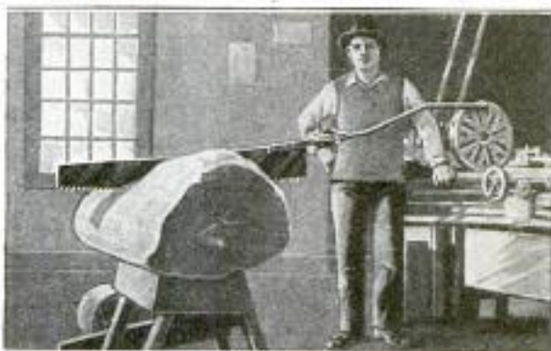
A Log-Sawing Attachment for the Engine Lathe That Relieves the Owner of a Lot of Back-Breaking Labor
