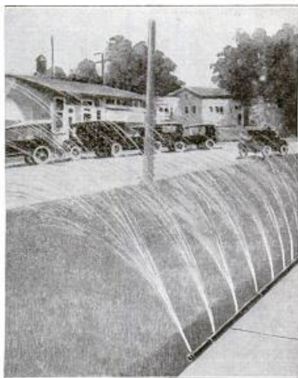
The Grass Plot along the Walk in Front of a City Hall is Kept Sprinkled during the Summer by a Perforated Pipe, the Water having First been Used to Test Water Meters
