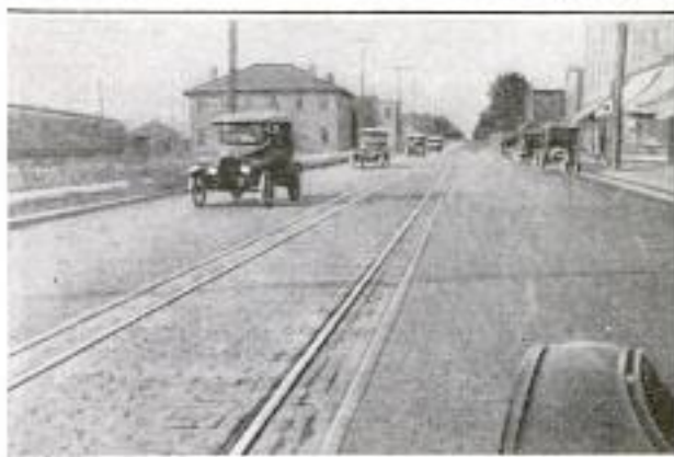
An Example of the Excellent Condition of the Pavement Where the Header Curb is Used to Localize the Movement Caused by the Street Cars
