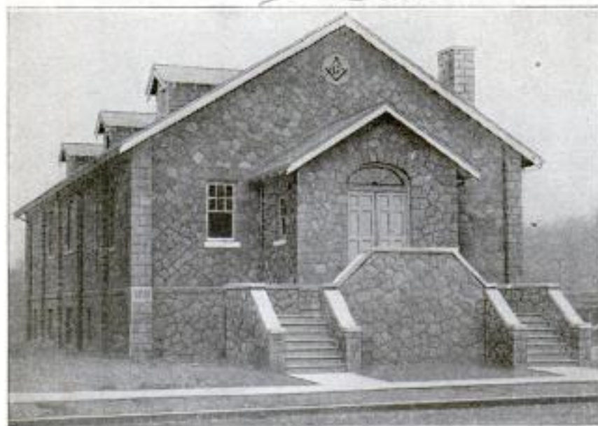
Masonic Temple of Townley Lodge, Palisades Park, New Jersey, Built with Their Own Hands by Members of the Lodge: The Structure is Very Solidly Built, with the Intention of Making It Almost Imperishable
