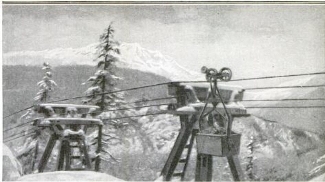
One of the Buckets, Containing 800 Pounds of Ore, Passing a Supporting Tower of the Tramway: The Cable for Loaded Buckets Is One Inch in Diameter and the Return Cable a Little Smaller
