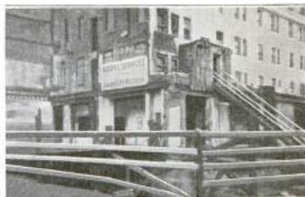
Fire-Damaged Hotel, Showing the Bridging of the Basement and the Stairway to the Second Floor
