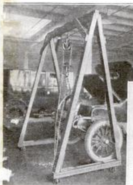
Left: A Portable Hoist, Built from Timbers and Mounted on Ball-Bearing Casters. Center: An Engine Puller Made from Two Spark-Plug Shells and a Piece of Steel Rod. Right: Both Devices Shown in Use for Lifting an Engine from Its Position on the Chassis
