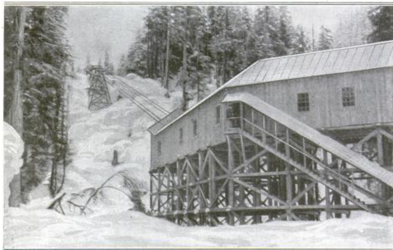
This Shows One of the Angle Stations Constructed Where the Tramway Makes a Turn. There Are Three Turns, All in the Same Direction, in the 11¼ Miles between the Mine and the Dock
