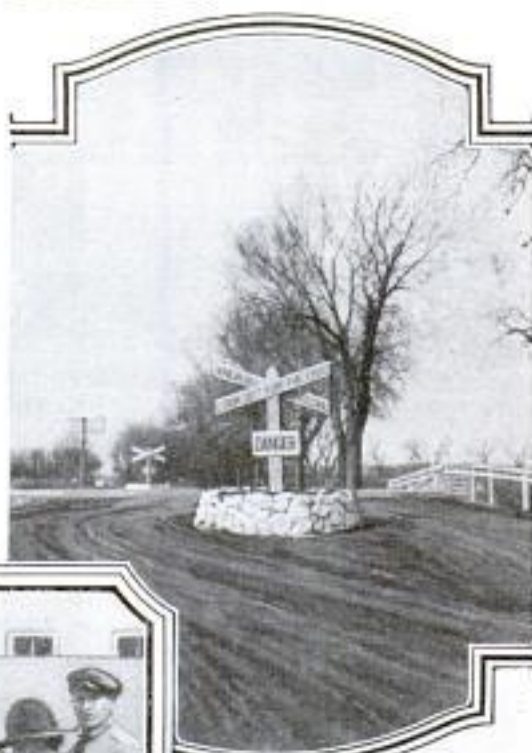
Safety-First Signals Built on Both Sides of a Dangerous Railroad Approach West of Norfolk, Nebraska: The Bases are Formed of Stones Painted White. In Their Centers are Installed the Crossing Signals
