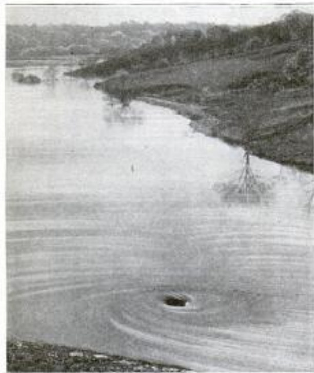
"Vortex Whirl," 25 Feet in Diameter, at the Germantown Dam near Dayton, Ohio, during a Recent Spring Freshet
