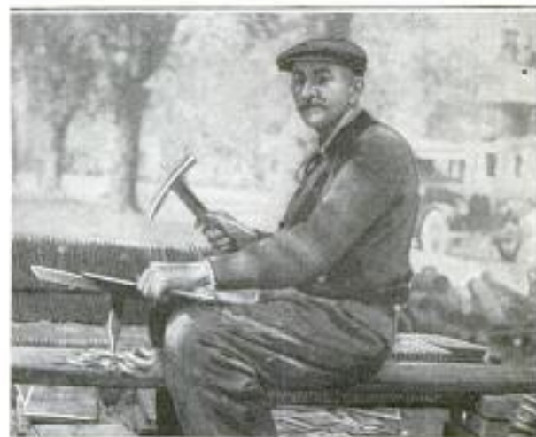
Workman Illustrating Method of Punching Nail Holes in Slate Shingles by Using Sharp-Pointed Hammer
