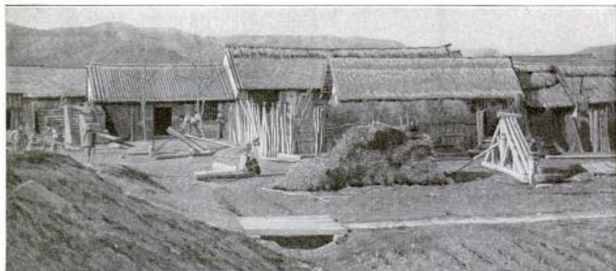
Typical Little Settlement of Oriental Farmers: The Roofs are All Thatched with Rice Straw. Preparations are being Made for the Erection of a New Hut, and the Roof Trusses can be Seen in the Right Foreground
