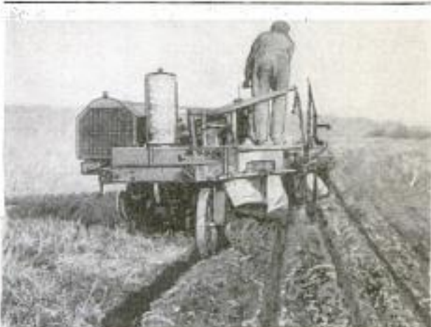
Rear View of Self-Propelling Gang Plow, Showing Furrows It Turns Up with Its Four Rotary Shares
