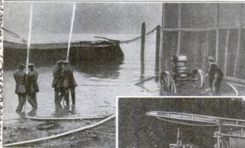
The Detachable Electric-Driven Pump Shown at Work, Power being Supplied from the Truck
