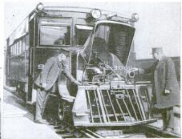
Another View of the New York and New Haven Car, Showing the Hood Raised, Exposing the Ordinary Gasoline Motor Similar to Those Installed in Trucks
