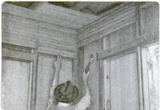
These Concrete "Boards" are Reinforced with Special Wire Forms and Develop Great Strength, as Shown in the Upper Views. Because of the Shape of the Boards, Regulation Wooden Studding and Laths can be Used on the Interiors, the Nails being Driven into the Joints, as Shown in the Lower Views
