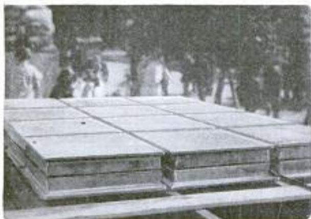
Illustrating a Type of Floor Construction in Which the Boxlike Concrete Blocks Rest on the Joists, Leaving Spaces between That are Filled with Wet Concrete, Forming a Solid Floor: A Floor 14 Feet Square Sustained a Weight of 100,000 Pounds without being Damaged, as Shown in the Lower View
