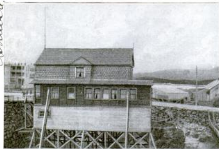
This House was Built before the Land was Graded, and While the First Floor Is at Street Level, the Basement is Supported on Stilts at a Considerable Height above the Ground
