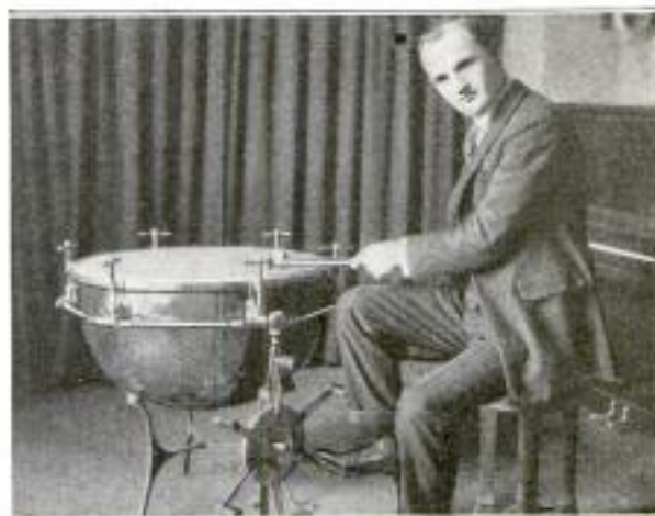
By Turning the Pedal Wheel of This Device, the Drummer Turns All the Tuning Handles, and Changes Rapidly the Pitch of the Drum
