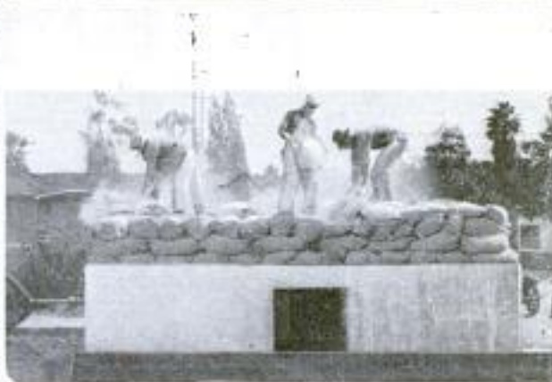
Illustrating a Type of Floor Construction in Which the Boxlike Concrete Blocks Rest on the Joists, Leaving Spaces between That are Filled with Wet Concrete, Forming a Solid Floor: A Floor 14 Feet Square Sustained a Weight of 100,000 Pounds without being Damaged, as Shown in the Lower View
