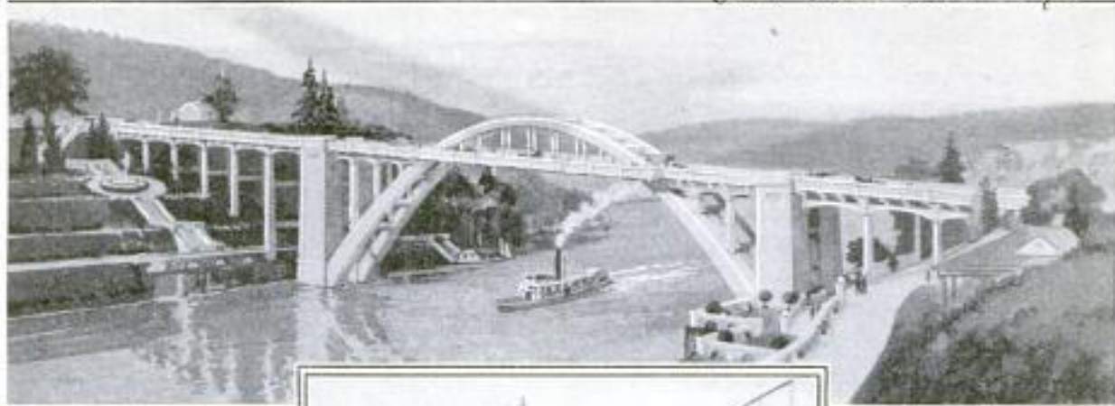
Above: As This Artistic Bridge will Appear When Completed. The Steel Work is Covered with Concrete as a Means of Protection and to Make It Harmonize with the Balance of the Structure
