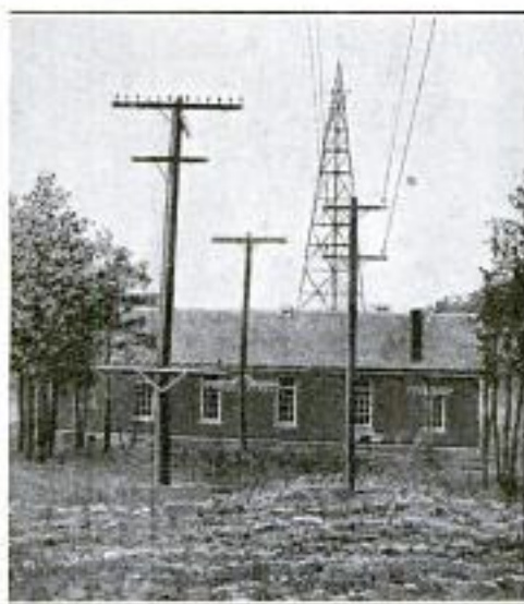
At the Right is Seen One of the Telegraph Poles That Carry the Eight-Mile Receiving Antenna. The Upper and Lower Wires on Each Side are Joined near the Station
