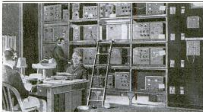
Four Tiers of Receiving Sets in the Station can Receive Messages from the Telegraph-Pole Antenna at the Same Time without Interfering with Each Other
