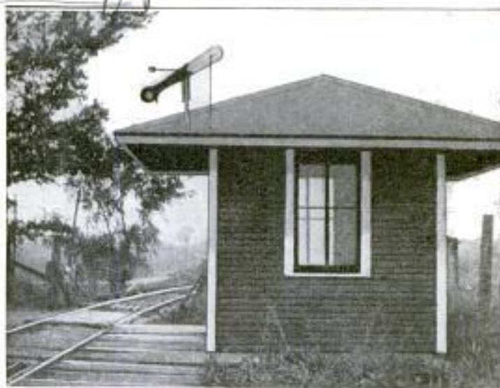
Semaphore on Interurban Station Which is Operated by Would-Be Passenger Pulling a Wire
