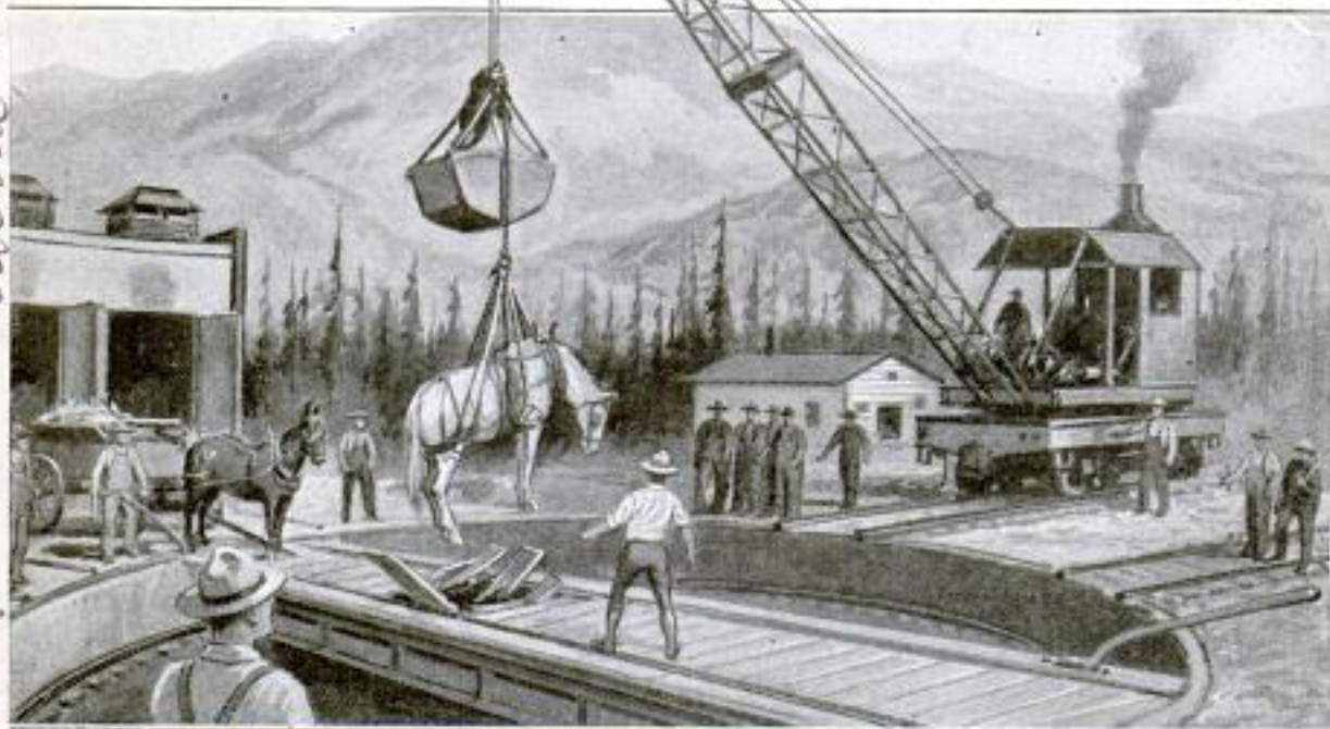
Clamshell Crane Shown in the Act of Hoisting the Horse from the Large Hole Seen in the Planking, Preparatory to Swinging the Unusual Load Clear of the Turntable to the Ground, Thus Avoiding the Necessity of Shooting the Imprisoned and Struggling Animal.
