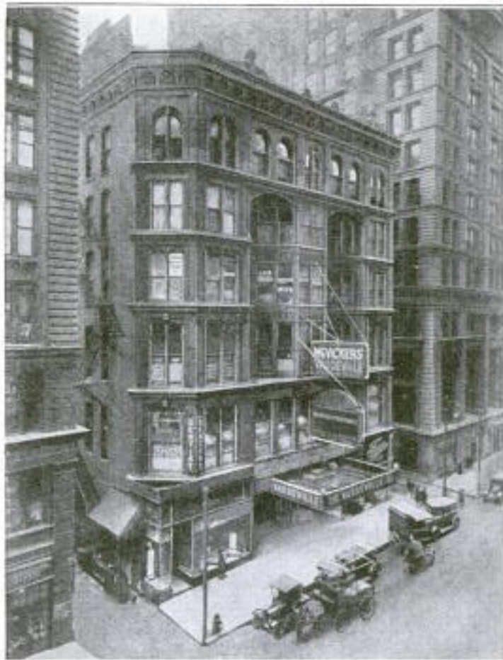
The Old McVickers Theater Building, Where for More than Four Months, Daily Performances were Given While Workmen Toiled Far Below Placing the Foundations for the New Building
