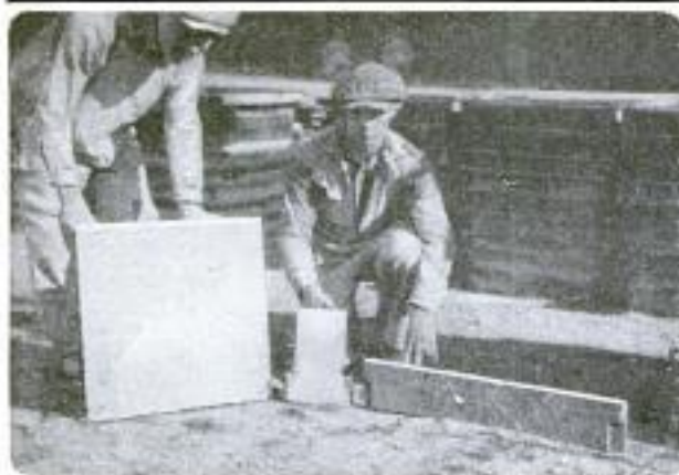
Three Views Showing a Form of "Concrete Lumber" in Which the Boards are Cast with Special Grooves in the Ends That Lock around Key Plates Set in the Wall: Built Up in This Way, the Wall Is Similar to Hollow Tile and is Then Washed Over with Wet Concrete That Joins the Boards into a Solid Wall
