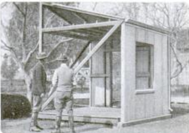
These Concrete "Boards" are Reinforced with Special Wire Forms and Develop Great Strength, as Shown in the Upper Views. Because of the Shape of the Boards, Regulation Wooden Studding and Laths can be Used on the Interiors, the Nails being Driven into the Joints, as Shown in the Lower Views
