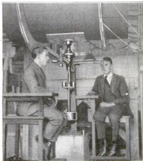
PHOTO COPYRIGHT, FRANK S. LINCOLN Two Observers Taking Readings from the Wind-Tunnel Balance: The Model being Tested Is above the Opening in the Tunnel Floor, over the Balance Stand
