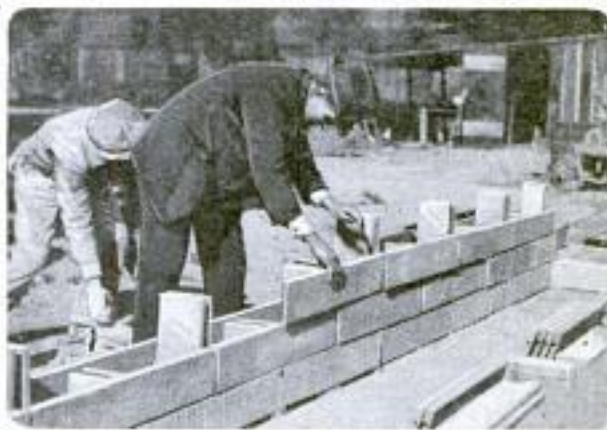
Three Views Showing a Form of "Concrete Lumber" in Which the Boards are Cast with Special Grooves in the Ends That Lock around Key Plates Set in the Wall: Built Up in This Way, the Wall Is Similar to Hollow Tile and is Then Washed Over with Wet Concrete That Joins the Boards into a Solid Wall
