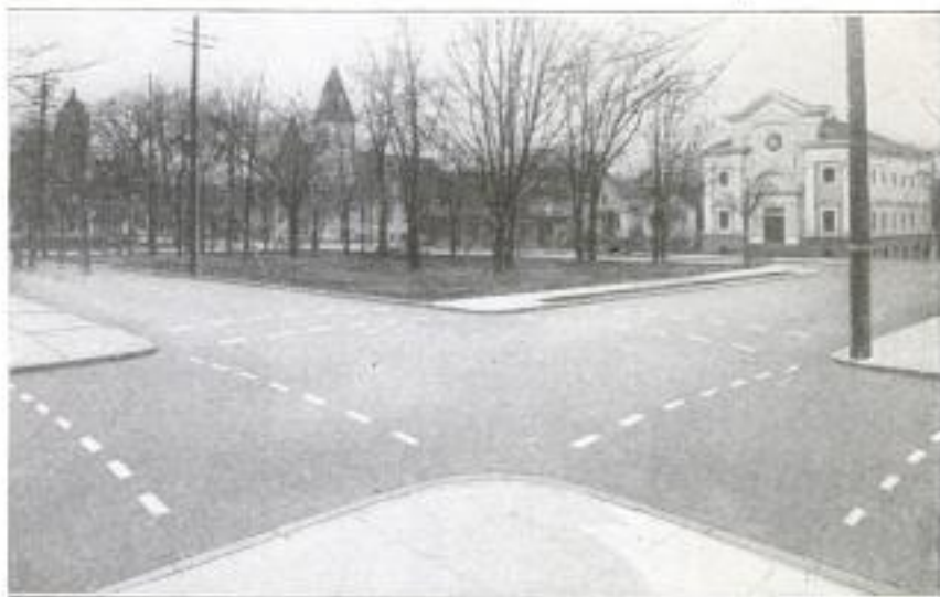
Hydraulic-Cement Blocks are Used to Mark Street Crossings in Portland, Oregon. Being Exceptionally Smooth, Hard, and Tough, They are Expected to Last Several Years, Thus Eliminating the Yearly Painting Job.
