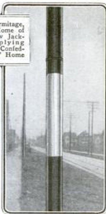
Trolley Poles at Stop Corners in Detroit were Formerly Striped with White Paint. Aluminum Paint is Now Used and is Found More Readily Visible at Night
