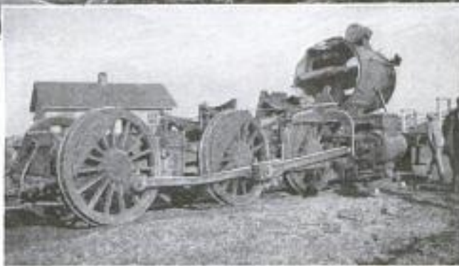
Locomotive Frame and Part of the Smoke Box That Remained Standing on the Track After the Boiler Exploded: The Engineer was Killed and the Fireman Injured
