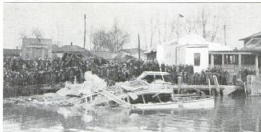
Wreck of the Ferryboat After Its Boiler Exploded: In the Background Is the House upon Which the Shell of the Boiler Landed
