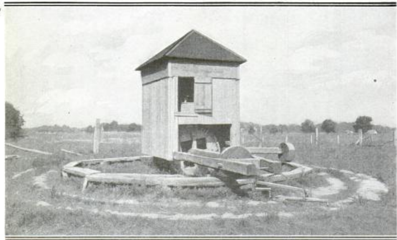
This Old-Fashioned Burr Mill is Still being Used Today, Although It Is More than 100 Years Old. Horses Walking around the Circular Path Furnish the Power
