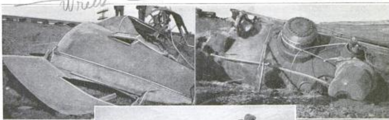
Top of the Cab Blown 25 Feet across the Track, When the Locomotive Boiler Exploded with Great Violence While on the Track
