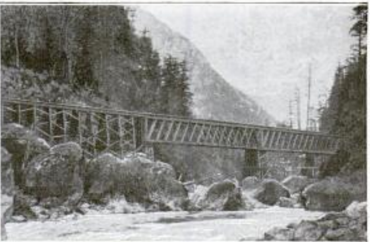
Two-Span Railroad Bridge, at Devil's Elbow, on the Skagit River in Washington. Showing, at Left, the Huge Natural Boulder That Supports the Pier between the Two Spans: The Approaches, One of Which is Shown to the Right, Are Ordinary Trestle Bents, and the Spans are Formed of Howe Trusses
