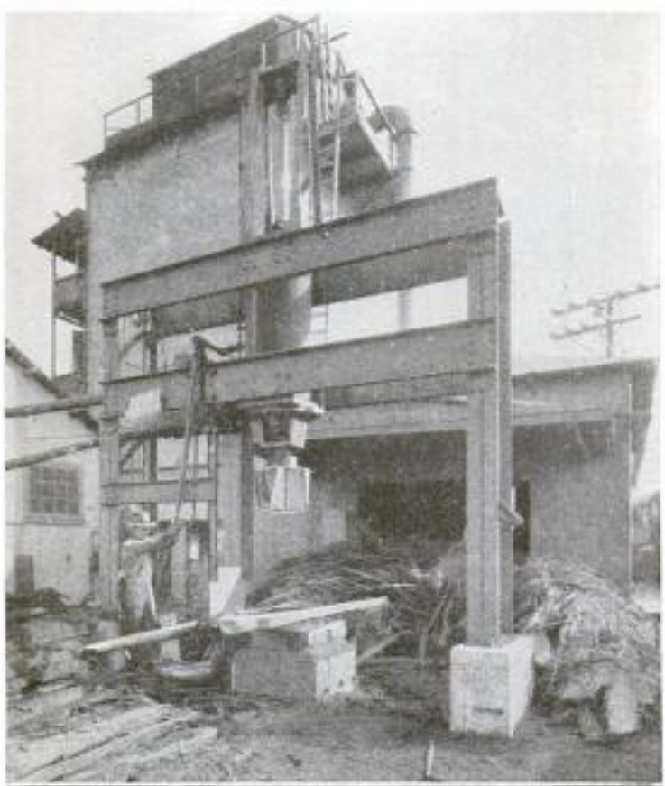
This Steam Ax Operates like a Steam Hammer, and is Equipped with a Four-Bladed Bit for Chopping Redwood Bark to be Used in the Manufacture of Roofing Material.
