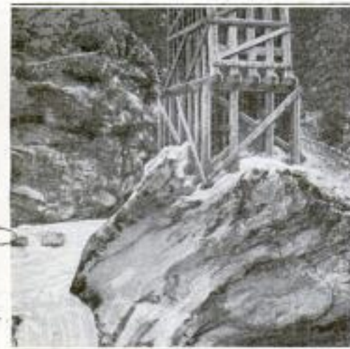
Two-Span Railroad Bridge, at Devil's Elbow, on the Skagit River in Washington. Showing, at Left, the Huge Natural Boulder That Supports the Pier between the Two Spans: The Approaches, One of Which is Shown to the Right, Are Ordinary Trestle Bents, and the Spans are Formed of Howe Trusses
