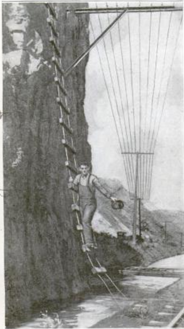
Placing the Wires on Steel Brackets Set in the Wall was Found to Be the Most Practical Method of Carrying the Wires through This Narrow Cañon
