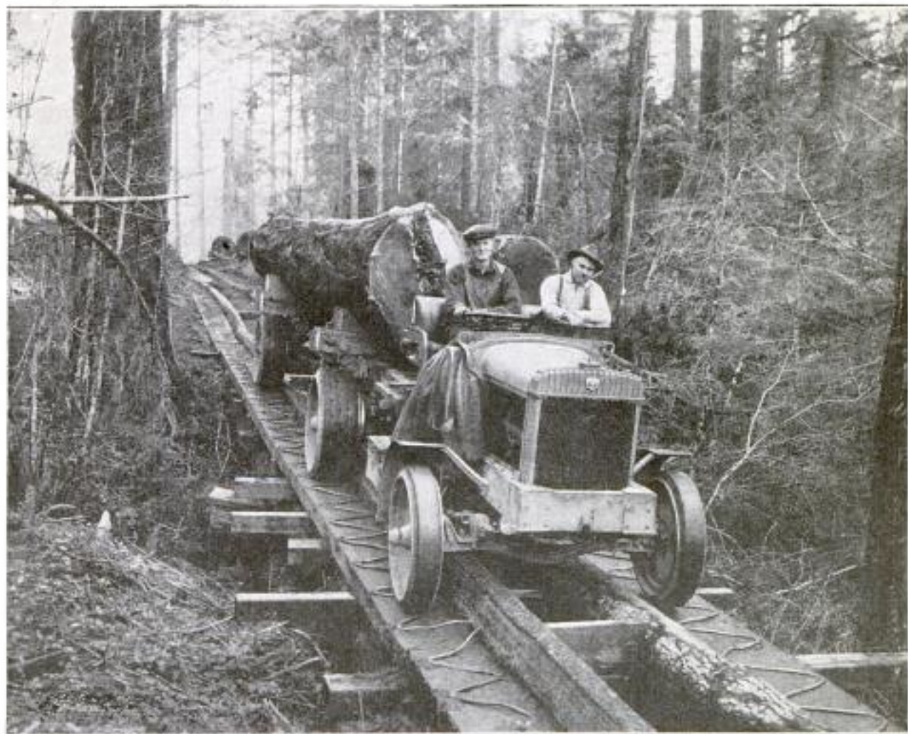
Specially Constructed Track for Hauling Heavy Loads on a Truck down a Very Steep Grade: Two Operators Are Necessary, the One on the Right Having Exclusive Control of the Brakes on the Rear Wheels. The Driving and Steering are Done Entirely by the Other Man
