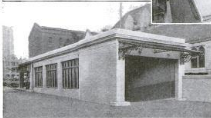
Entrance to the Underground Garage: Broad, Easy-Sloping Ramps Lead to the Two Floors below Ground Providing Space for Nearly 200 Cars. The Garage Is Directly under the Open Parking Space
