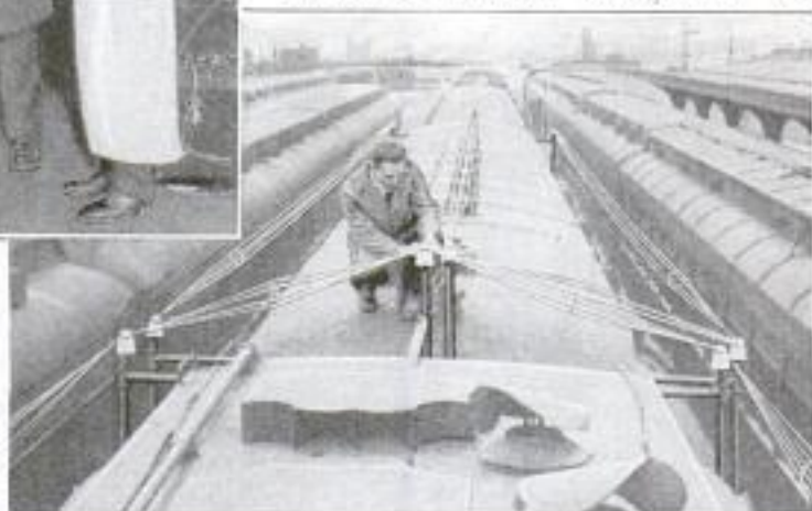
Specially Constructed Aerial for the Radiophone Equipment on the Lackawanna Railroad Buffet Car being Connected on Top of the Train before Making an Experimental Trip with the Apparatus
