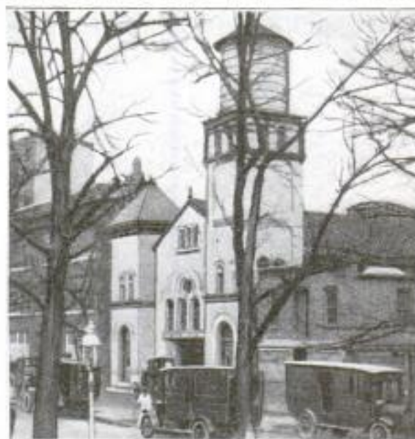
Between the Limbs of the Trees can be Seen the Front of a New Garage in an Old Abandoned Church Building. Part of the Old Steeple is Replaced by a New Water Tank
