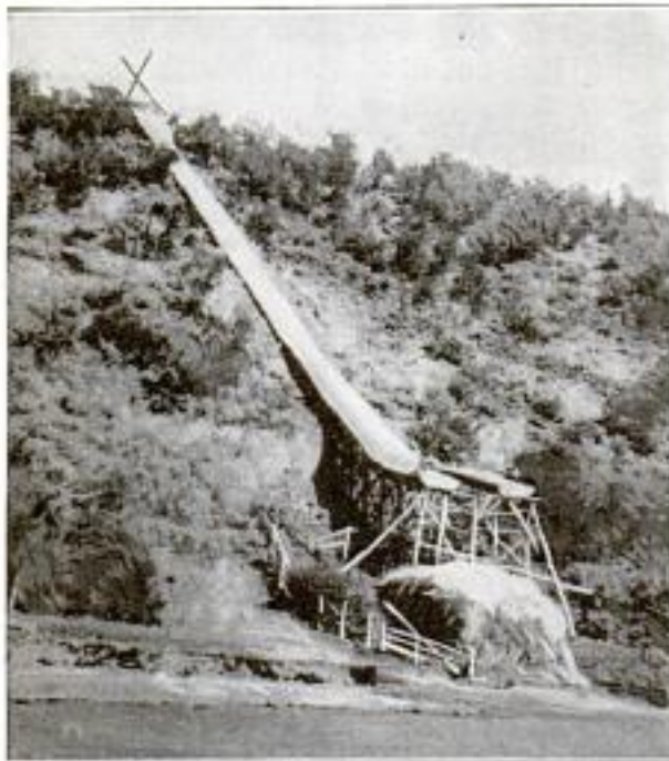
A Western Rancher's Method of Stacking Hay by Gravity: His Crop is Raised on the High Land, Whence It is Shot down a 400-Foot Chute to His Feed Lot in the River Bottom
