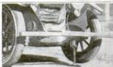
Automatic Jacks Permanently Installed, One at Each Wheel, Operated by Power from the Engine, and Controlled from the Driver's Seat: The Lift Is 5 1/2 Inches
