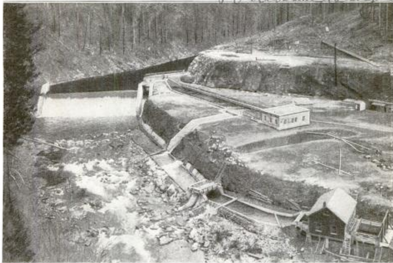
Waterworks Project. Showing the Dam Which Controls the River: Beginning at the River Just above the Dam can be seen the Canal That Leads to the Screen House. From the Screen House the Water is Carried through a Narrow Channel Leading to the Pipe Lines
