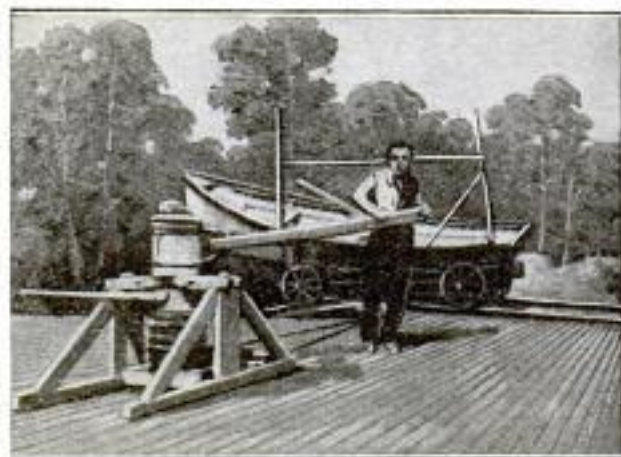
Hauling a Boat from One Lake to Another by a Miniature Marine Railway Is the Way a Body of Sportsmen Took to Avoid Digging a Canal to Connect Twin Lakes
