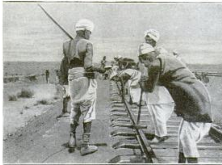
Section Boss and His Gang on the Hedjaz Railway: The Ties Used Are of Steel, as No Wood could Stand the Climate. This Railroad Is Turkish-Built, and Mainly Serves the Pilgrim Traffic
