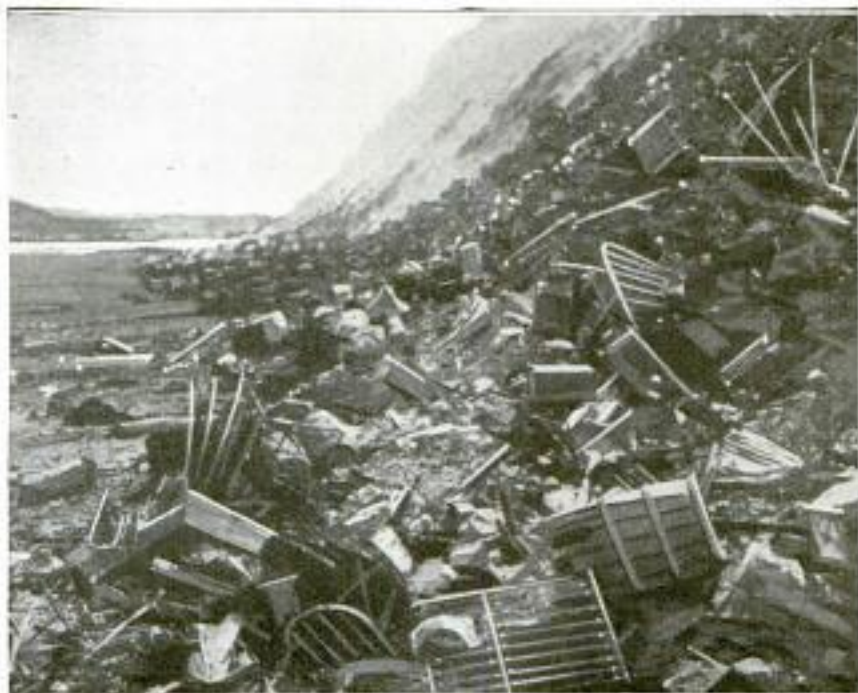
Embankment of Refuse Used in Building Up Riker's Island: Space to the Left will be Filled to the Level of the Hills Shown on Opposite Page
