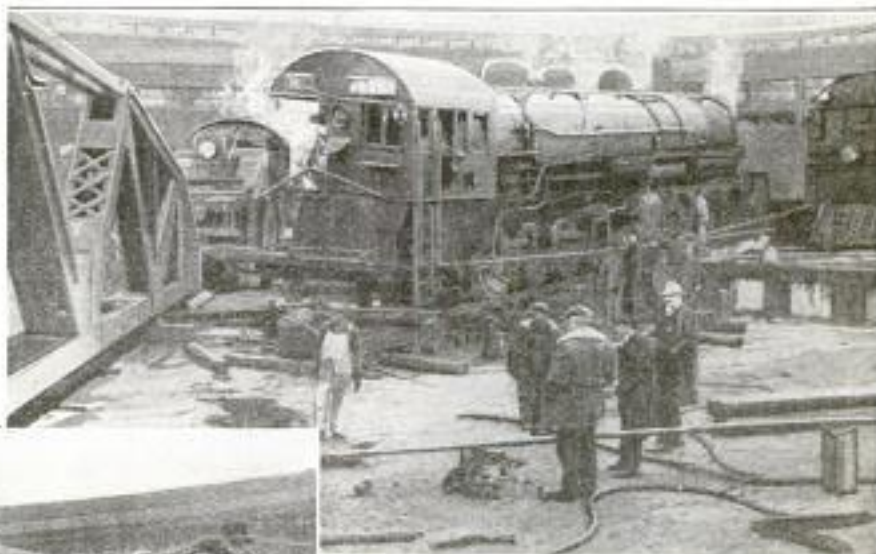
Workmen Raising the Runaway Engine upon Blocks Preparatory to Taking It Out of the Turntable Pit: The Damage to the Cab of the Engine can be Plainly Seen
