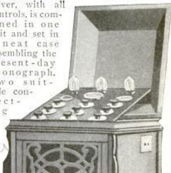
After Connecting to the Aerial and Ground Wire, the Radio Phonograph is Tuned In by Adjusting the Control Disk
