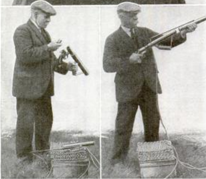
Above: Two Steel Boxes Hold the Complete Outfit. Below: Left, Inserting the Firing Cartridge in the Pistol; Right, Inserting the Self-Propelling Rocket with Line Attached
