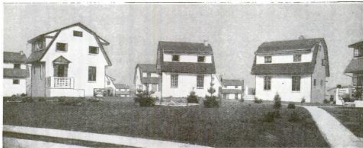
A Corner in the Village of Concrest, with Three Houses in the Foreground That Are Typical of the Rest: Built of Concrete, the Exteriors Are of Tinted Stucco, and the Roofs of Different Colors
