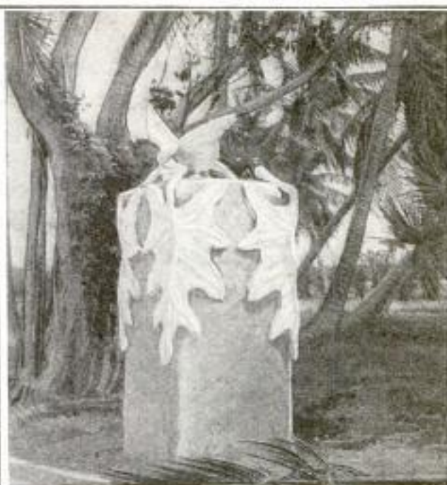
Left: A Fountain of Molded Concrete, in Which the Large Shell was Shaped Out of a Single Block as the Material was Setting, the Figure being Built Up on a Frame of Iron Pipe and Wire Mesh. Right: Decorative Pier, Seven Feet High, Cut from a Solid Block. The Bird on Top of the Pier is Molded over a Wire-Mesh Frame
