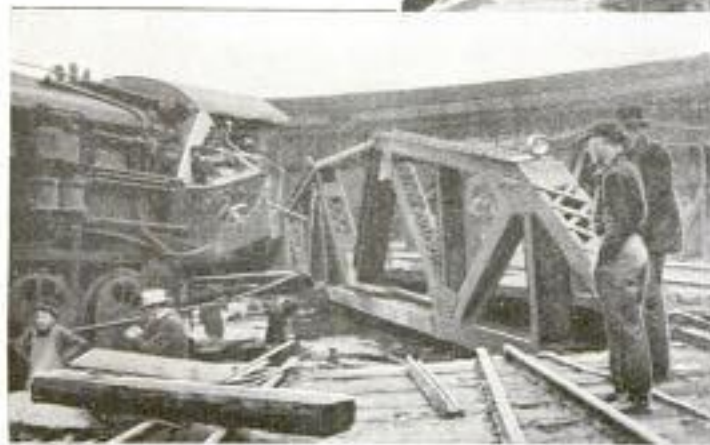
Runaway Engine Shown in Turntable Pit Immediately After It had Made the Disastrous Plunge
