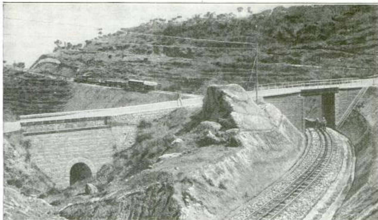
The Narrow-Gauge French-Built Line, Climbing the Mountains Back of Damascus: The Grades Are in Some Places Very Steep; Here, for Instance, the Gradient Is Six per Cent, and a Rack System Was Necessary to Secure Traction
