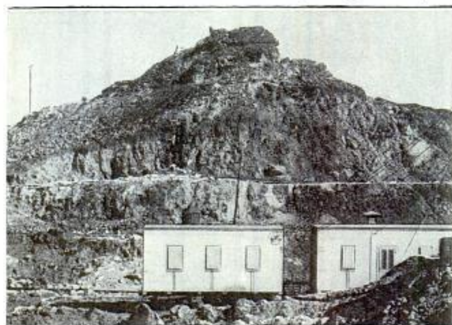
Crusher Station and Assay Office Which Travels by Railroad to the Different Mining Locations Where Samples of Ore are Analyzed and the Results Reported to the Operators
