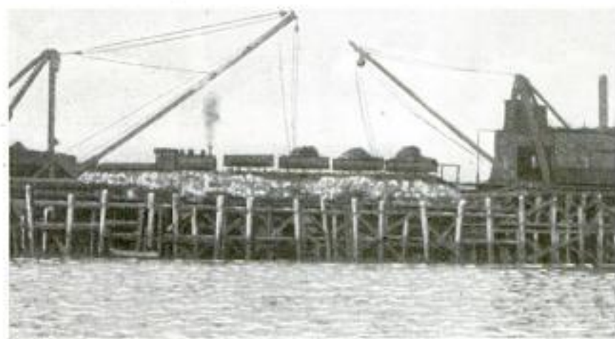
Loaded Cars Leaving Dock: About 50 Such Cars Are in Constant Use for Hauling the Refuse from the Landing Dock to Various Parts of the Island
