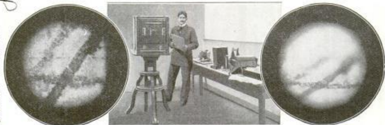
French Microphotographic Apparatus for Detecting Forgeries: At Left is Shown a Photograph, Taken in the Old Way, of a Figure "1" That was Later Changed to a "4," Which Shows the Horizontal Stroke Apparently below, Whereas It was Actually above, the "1," as Shown Clearly in the Photograph to the Right, Which was Taken by the New Method
