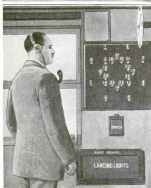
Above: The Controller of Traffic Using a Pistol Flashlamp from the Balcony of the Control Tower. Left: From the Inside of the Tower He can Communicate with the Approaching Flier by Wireless Telephone and Give Him Special Information as to Ground Conditions. All Landing and Signal Lights are Controlled from the Tower. Right: Using an Electric Flasher to Communicate with the Airman
