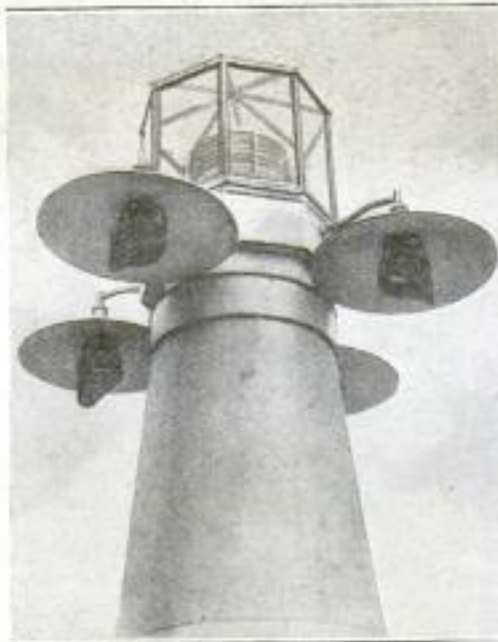
One of the Smaller Lighthouses on the London-Paris Route is Equipped with Lenses for Throwing a Horizontal Beam, and Four Reflecting Lights Which Project a Vertical Beam
