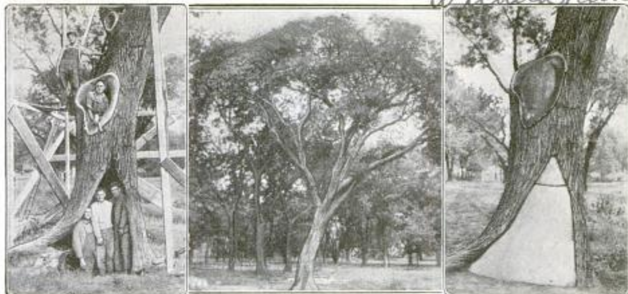
Left: Historic Old Elm After the City Forester had Scraped Out the Decayed Matter Which Extended to a Height of 20 Feet. Center: Elm in the Municipal Park, Showing the Opposite Side of the Tree. Right: Elm after being Filled with an Eight-Ton Mixture of Concrete and Scrap Iron
