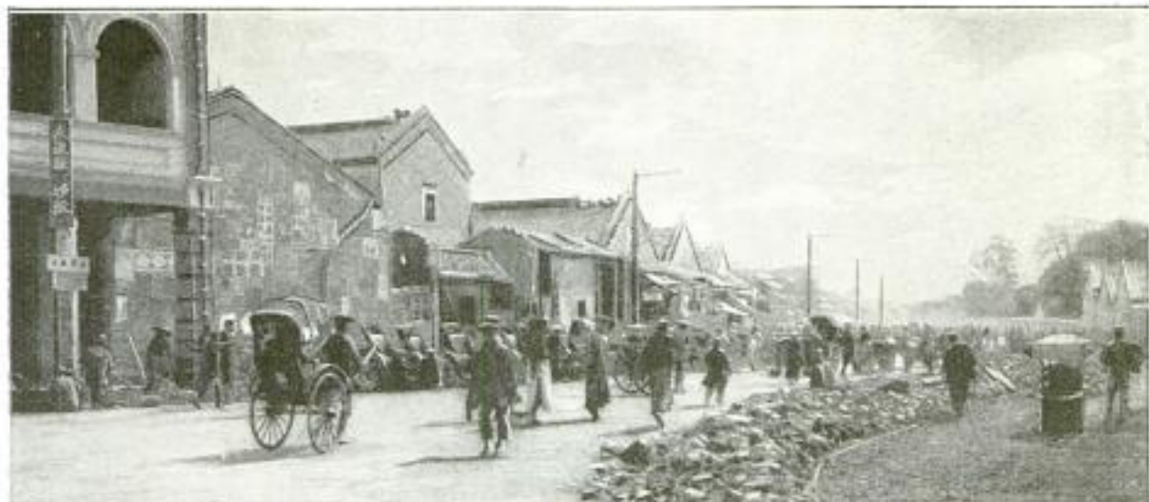
Mun Tak Maloo, Looking South, as It Appeared in 1920, Before the Boulevard Work had Progressed Very Far: One-Half of the Roadway had been Opened for Traffic While Work Went Forward on the Other Half
