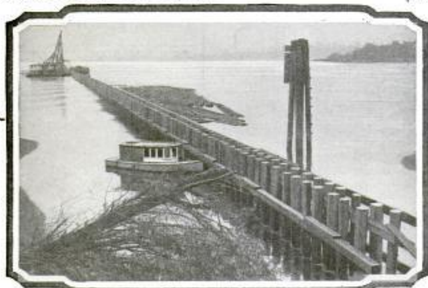
The Dike Built at the Confluence of the Willamette and Columbia Rivers to Prevent Shoaling of the Ship Channel
