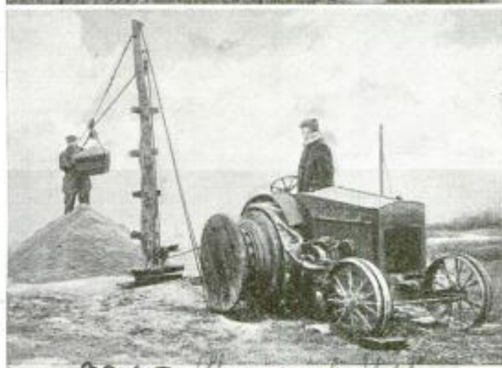
Above: Improved Hoisting Arrangement in Action, Showing One of the Loaded Buckets Midway of the Long Stretch of Trolley Line Used to Transport Sand from the Beach to the Bluff. Left: The Tractor was Used as a Hoisting Engine; Its Front Wheels were Blocked, the Rear Wheels Jacked Up off the Ground, and a Winding Drum Fitted to One of the Latter
