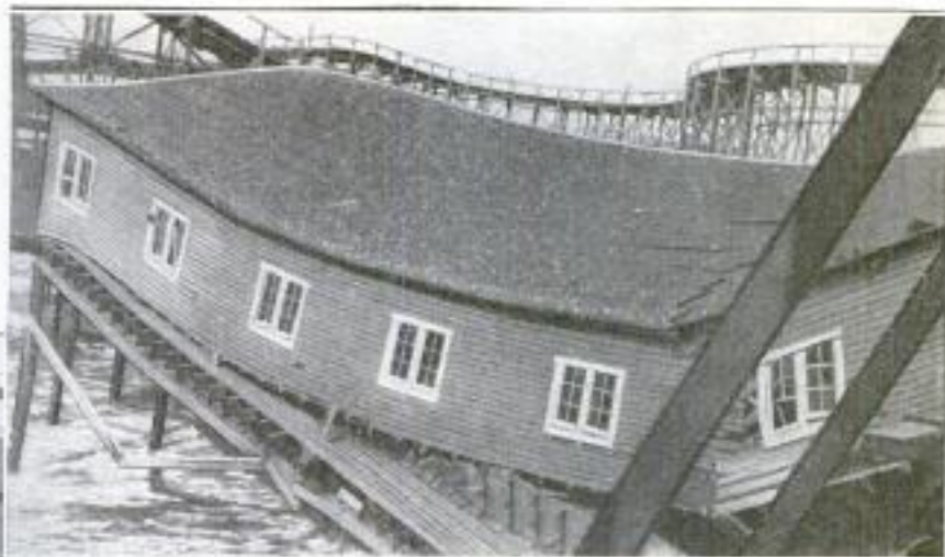
Above is Shown One of the Concession Buildings Which was Thrown from Its Foundations When the Barge, Seen at the Left, Wrecked the Amusement Pier
