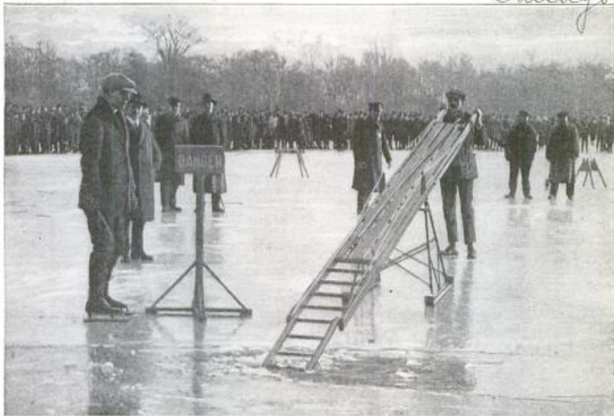
The Short Section of the Ladder is Depressed Until It can be Grasped by the Person Who has Broken through the Ice. The Rescuer Then Bears Down on His End of the Long Ladder and Drags the Victim Back to Safety
