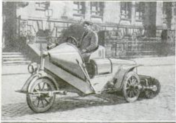
Above: Three-Wheeled Motor Car of European Design Which is being Used with Success as a Street Sweeper. Left: Same Type of Machine with a Water Tank Mounted on the Rear. The Lever Attachment for Applying the Rotary Brush to, and Lifting It from, the Pavement can be Seen on the Side of the Car at the Left of the Driver
