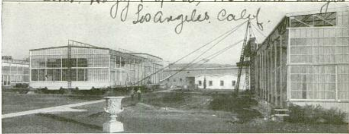
The Motion-Picture Studio at the Left being Moved across the Open Space to be Joined to the Studio at the Right: The Journey Took Four Days and was Accomplished without Accident
