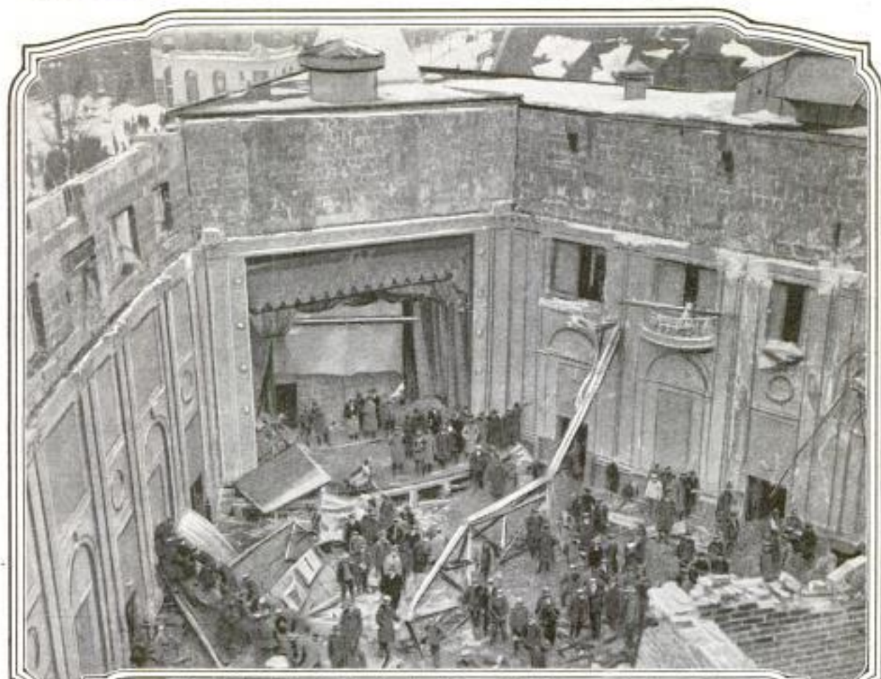
View of the Inside of the Knickerbocker Theater, Washington, District of Columbia, Taken Shortly after the Collapse of the Roof That in a Few Moments Changed the Building from a Theater into a Catacomb: Nearly 100 Dead Bodies Lay beneath the Fallen Roof, and Many More Injured. When This Picture was Taken, the Rescue Work, Carried Out by Firemen, Police, and Marines, was Well Advanced
