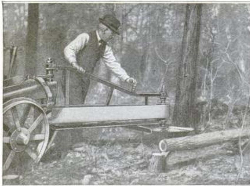
This Circular Saw, Mounted on a Swinging Frame at the Front of a Small Tractor and Driven by the Tractor Engine, can be Used in Clearing Land, or can be Swung into Position for Cutting Wood
