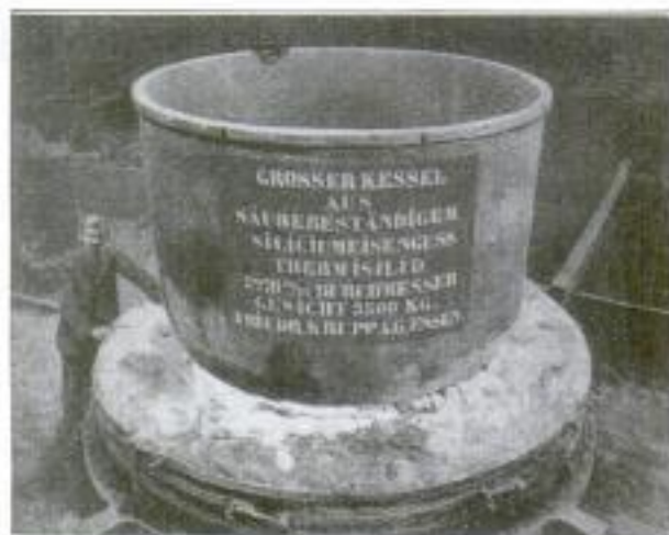
Iron-Silicon-Alloy Casting, Produced by New Combination-Process, Weighs Almost 7,700 Pounds
