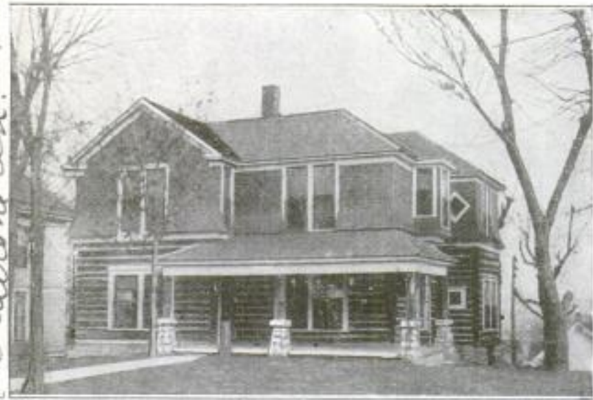
Economical House in Which Discarded Telephone and Lighting Poles Form the First Story and the Porch Supports: Seventy-Five Poles were Used in the Construction of This Dwelling
