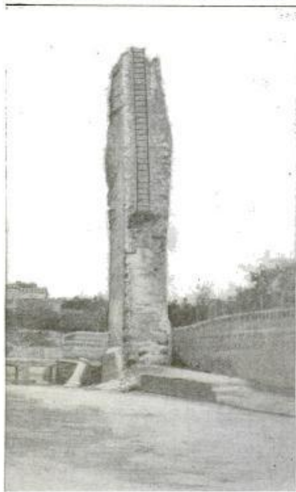
Tower in Palermo, Sicily. More Than 1,000 Years Old: The Upper Half Is Hollow and was Originally Used for Water Storage
