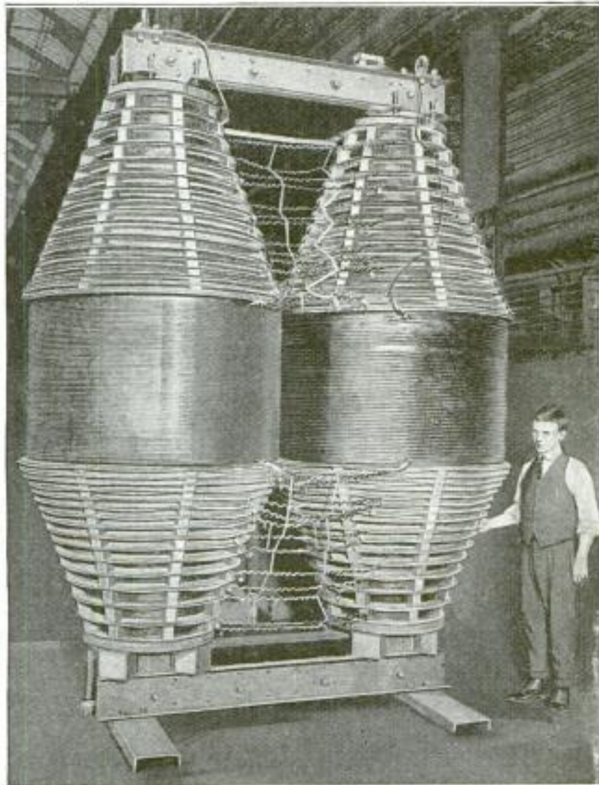
Million-Volt Transformer in Course of Construction, Showing the Completed Windings on the Two Legs of the Core and Illustrating How the Coils Increase in Diameter as They Decrease in Length
