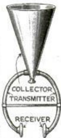
Experimenting with the Instrument Which Enables the Listener to Hear Otherwise Inaudible Sounds Made by Insects: At the Right is a Diagram of Its Construction
