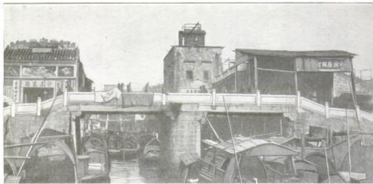
A Bridge over One of the Numerous Canals, Some of Which were Dug as Much as 3,000 Years Ago: In Many Cases the Material Excavated in Making the Canals was Used in Constructing the Great Wall
