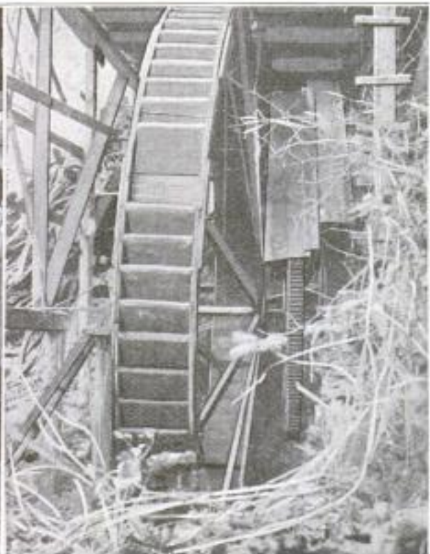
Left: Small Homemade Turbine in Homemade Mill on Spring Creek, Baxter County, Arkansas. Under a Full Head of Water It Develops 12 Horsepower. Right: Large Overshot Wheel That Develops 20 Horsepower and Operates a Sawmill, a Gristmill, and a Small Flourmill. Plants of This Kind Were the Only Ones in Existence before the Building of the Taney Dam in Missouri
