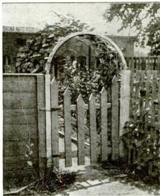
An Artistic Arbor for a Gate or Garden Seat That can be Easily Built from the Felloes of Old Wagon or Buggy Wheels
