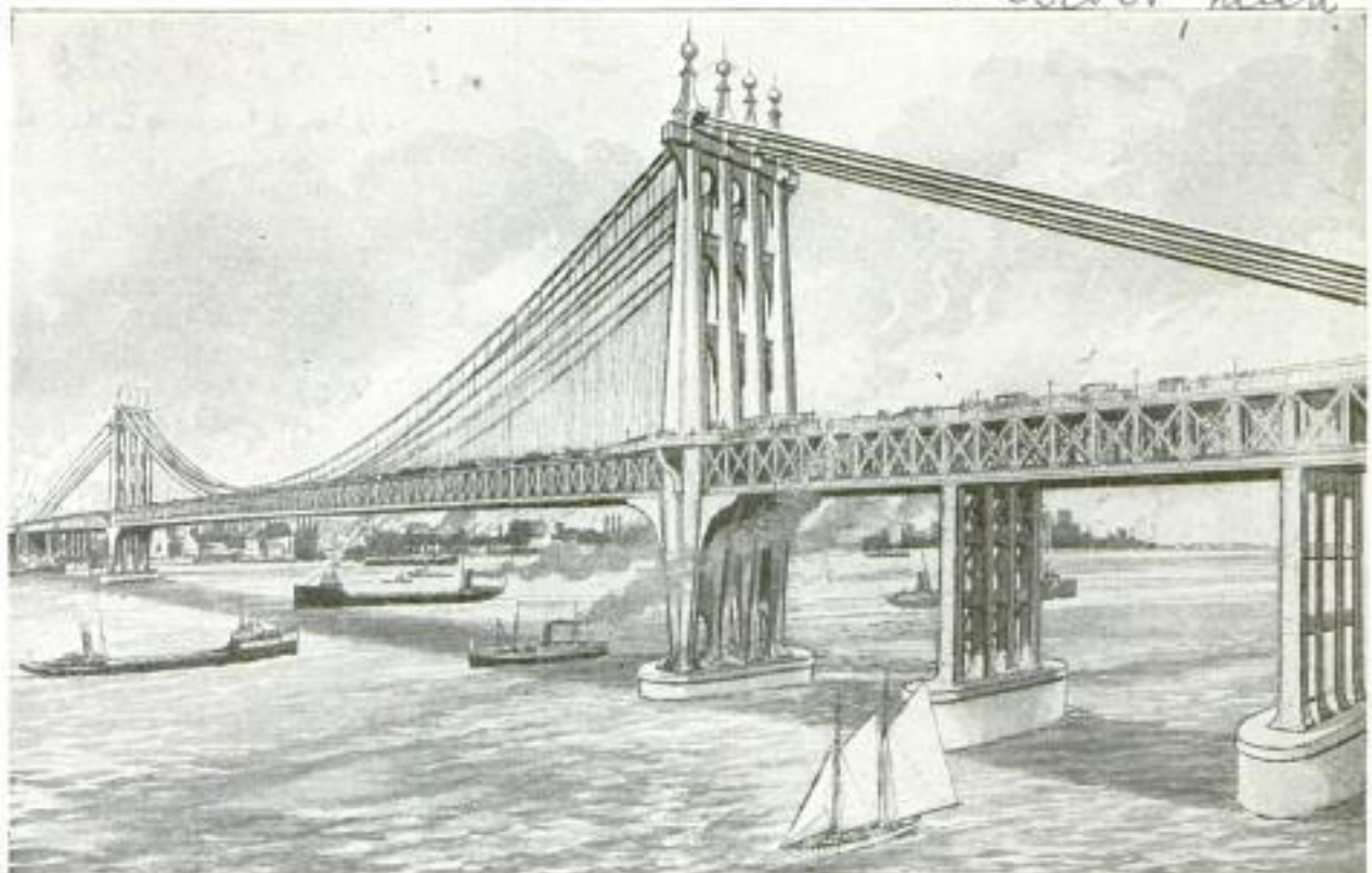
Huge International Suspension Bridge That is to Connect Detroit, Michigan, with Windsor, Ontario: The Main Span Is 1,803 Feet, and the Towers Rise 380 Feet above the Water. Of the Eight Cables Six will Be 21 Inches in Diameter, and the Other Two 18 Inches
