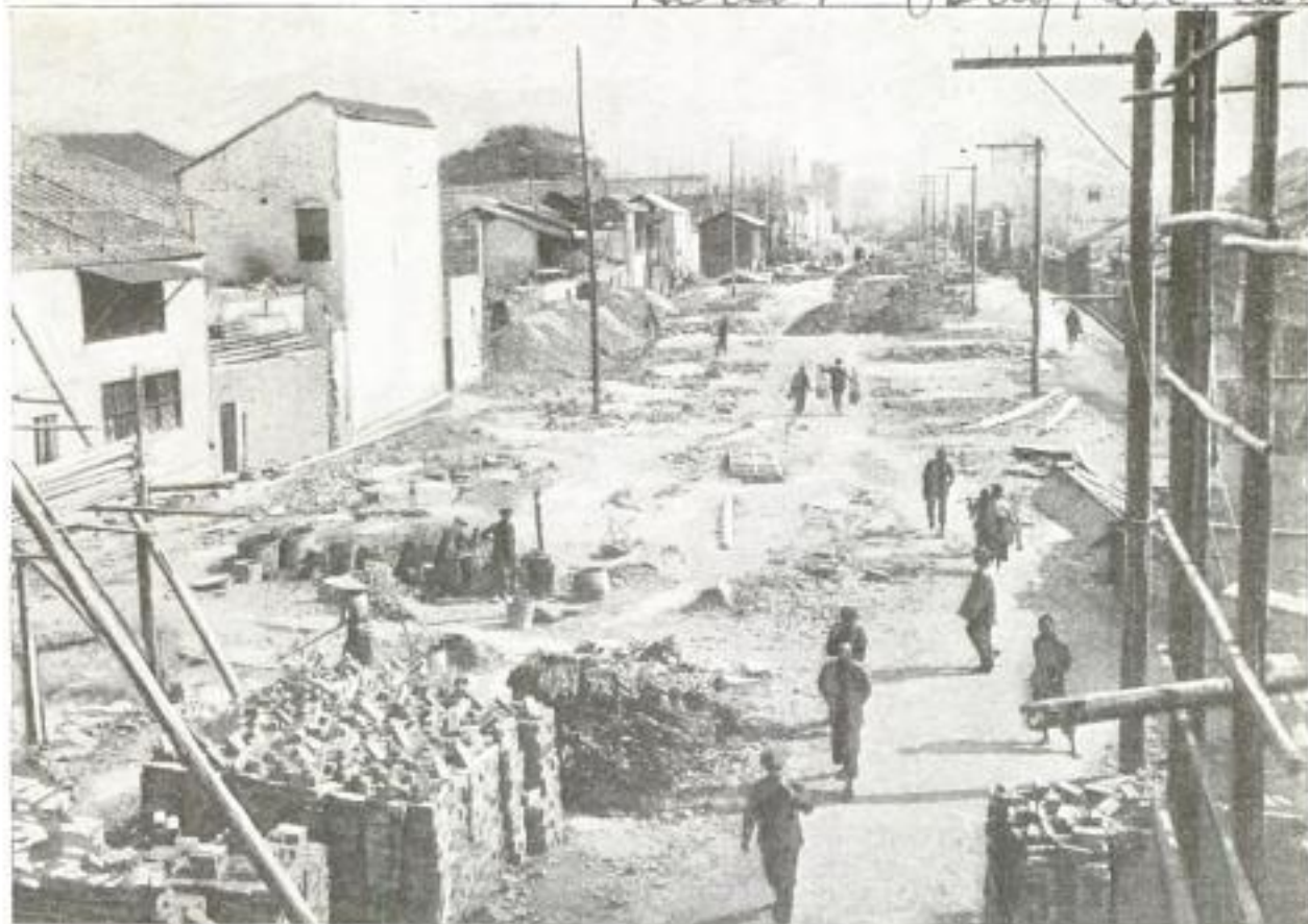
After the Great Wall was Torn Down, the Modern Boulevard was Constructed in Its Stead. The Boulevards Are from 80 to 125 Feet Wide, and Where Necessary, Shacks along the Sides were Torn Down to Provide Space
