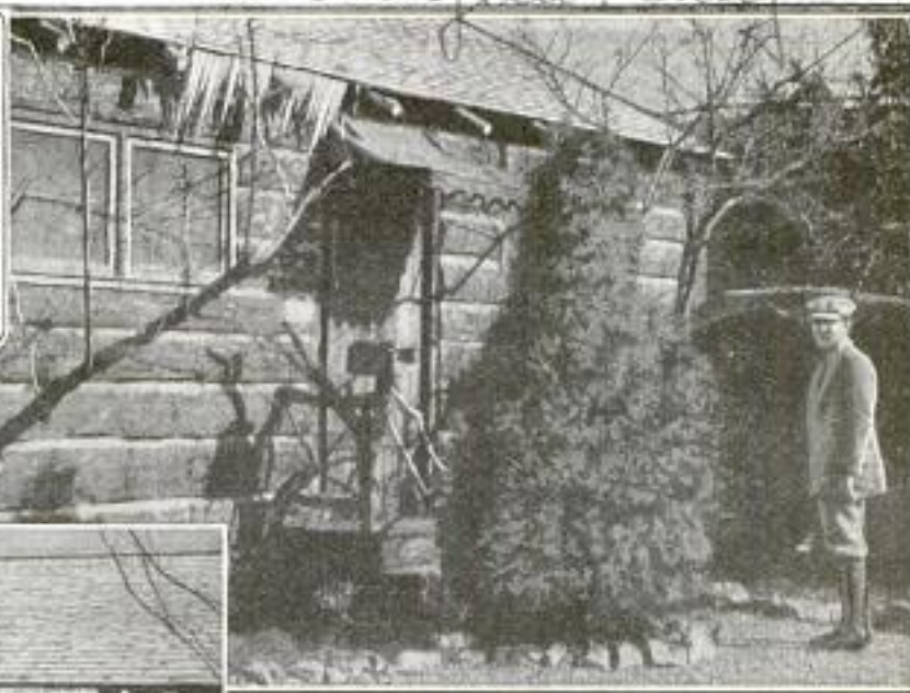
Front View of the Log Cabin, Which is Built in the Midst of Totally Different California Bungalows, and Which Possesses Counterfeit Wintry Decorations: At the Left are Seen Some of the Imitation Icicles Which are Made of Wood and Painted White. The Roof of White Sand is Also Shown, the Whole Giving the Appearance of Winter
