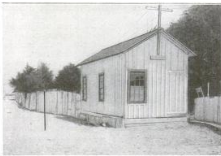
Prior to the Earthquake of 1906 This Building Stood at the Point Marked by the Black Stake. During the Quake the Building and Part of the Back Fence were Moved a Distance of 12 Feet to Their Present Location
