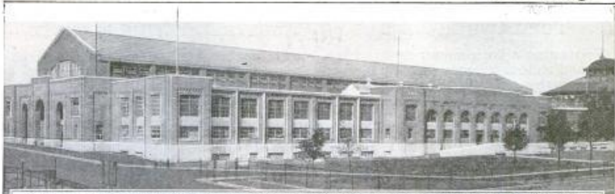
Exterior of the Mammoth Building Erected on the Minnesota State Fair Grounds for the Housing of Blooded Cattle While on Exhibition: It Contains the Most Modern Equipment in the Way of Ventilation, Sanitation, and Protection against Fire Hazard
