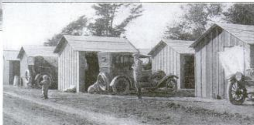
Another View of the Village Street, Showing Some of the Houses Which Contain Electric Lights, Running Water, and Two-Burner Gas Plates
