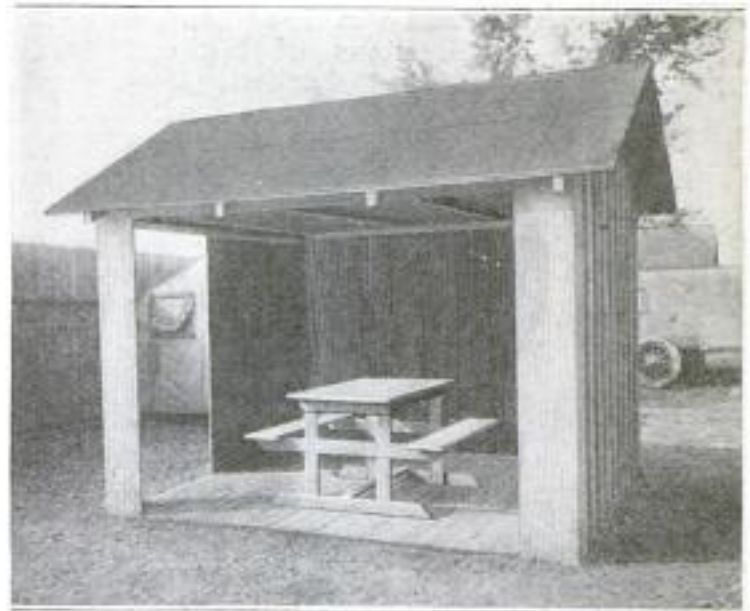
One of the "Shelter Houses" of the Village, Which Is Open on Two Sides: It Has a Combination Table and Benches Accommodating Four Persons, and Also a Two-Burner Gas Plate
