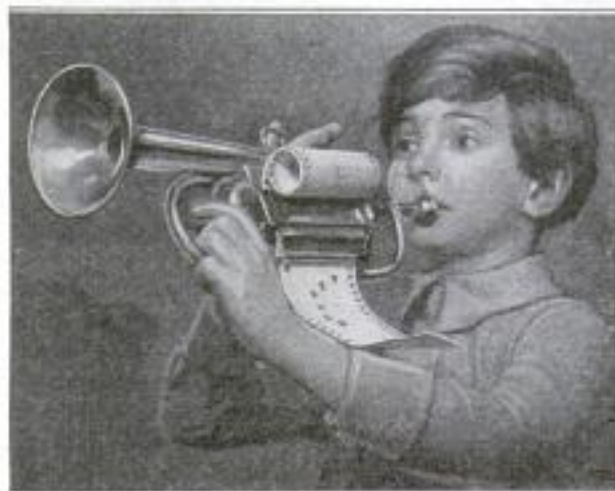
The Strip of Perforated Paper is Fed Through Mechanically, Causing the Proper Keys to be Depressed
