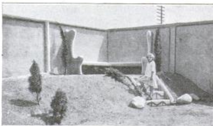
Another View of the Bungalow Garden, Showing a Corner of the Surrounding Wall into Which is Built an Artistic Seat. The Wall and Seat are Constructed in One Solid Mass
