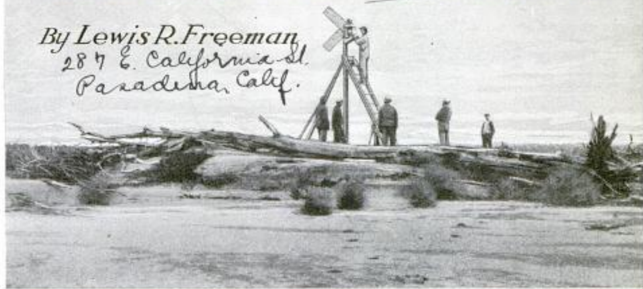
Setting Up a Beacon on a Sand Bar on the Mississippi River: It Is One of 700 Similar "Aids" That have been Established along the 1,200-Mile Course of the River between St. Louis and New Orleans, to Direct Navigation of the Constantly Shifting Channel
