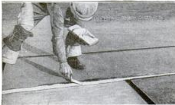
The Cement is Colored with Lampblack to Relieve the Glare, and the Lines are Made by Laying White Cement in Grooves in the Surface
