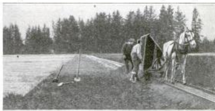
After the Bog has been Drained and Cleared Down to the Peat Bottom, Four Inches of Clean White Sand is Spread on Top of the Peat
