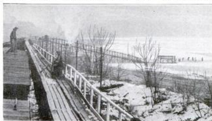
Loading a Whole Train at a Time with Ice on the Burlington Railroad: The Train is Sidetracked alongside the Runway from Which the Ice is Quickly Pushed through the Open Car Doors
