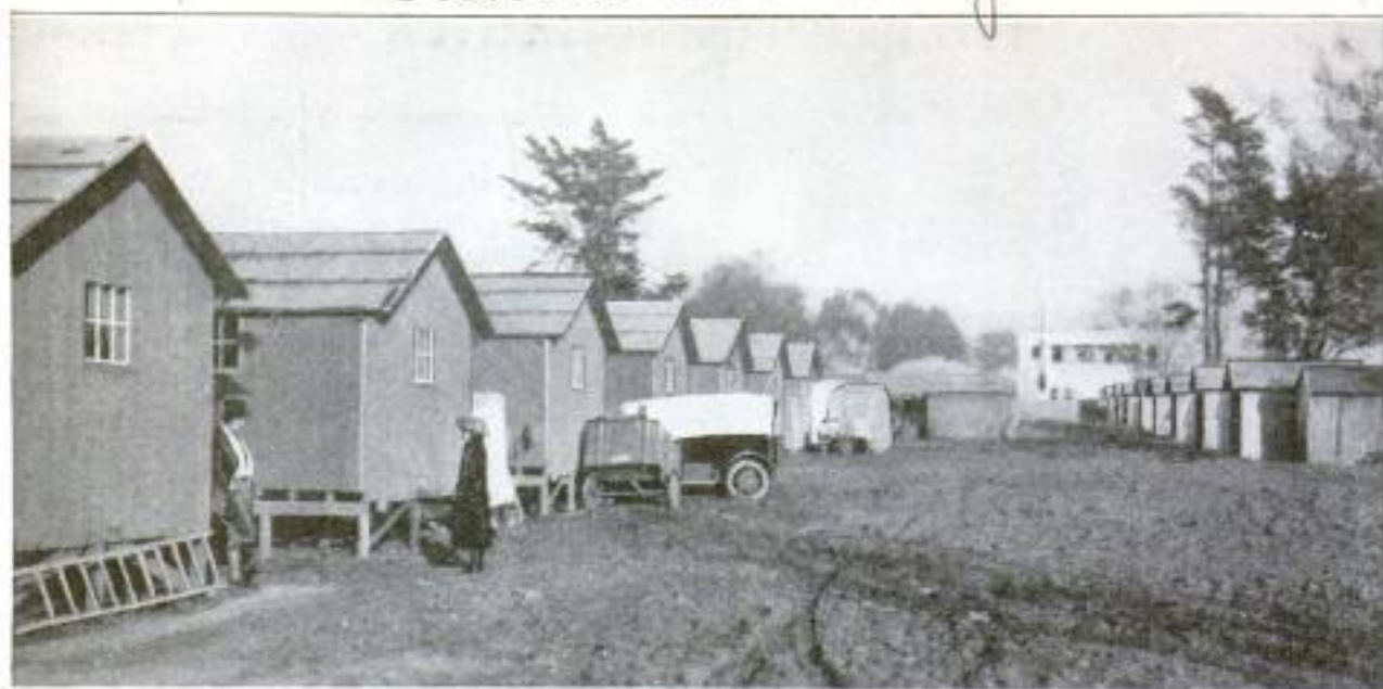
A Street in the "Bungalow" Village Which will Accommodate 500 Motorists When Completed: At the Extreme End of the Street, on the Right, can be Seen a Store Which was Erected Expressly for the Convenience of the Villagers. When Finished, This Street will be Paved with Crushed Stone
