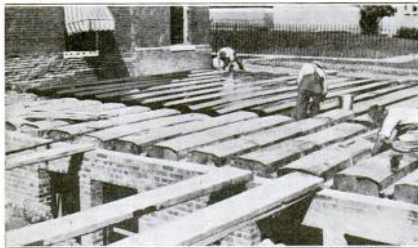
Sheet-Steel Forms for Pouring the Reinforced Concrete Floor on the Ground Level of an Addition to a New York City Bank Branch
