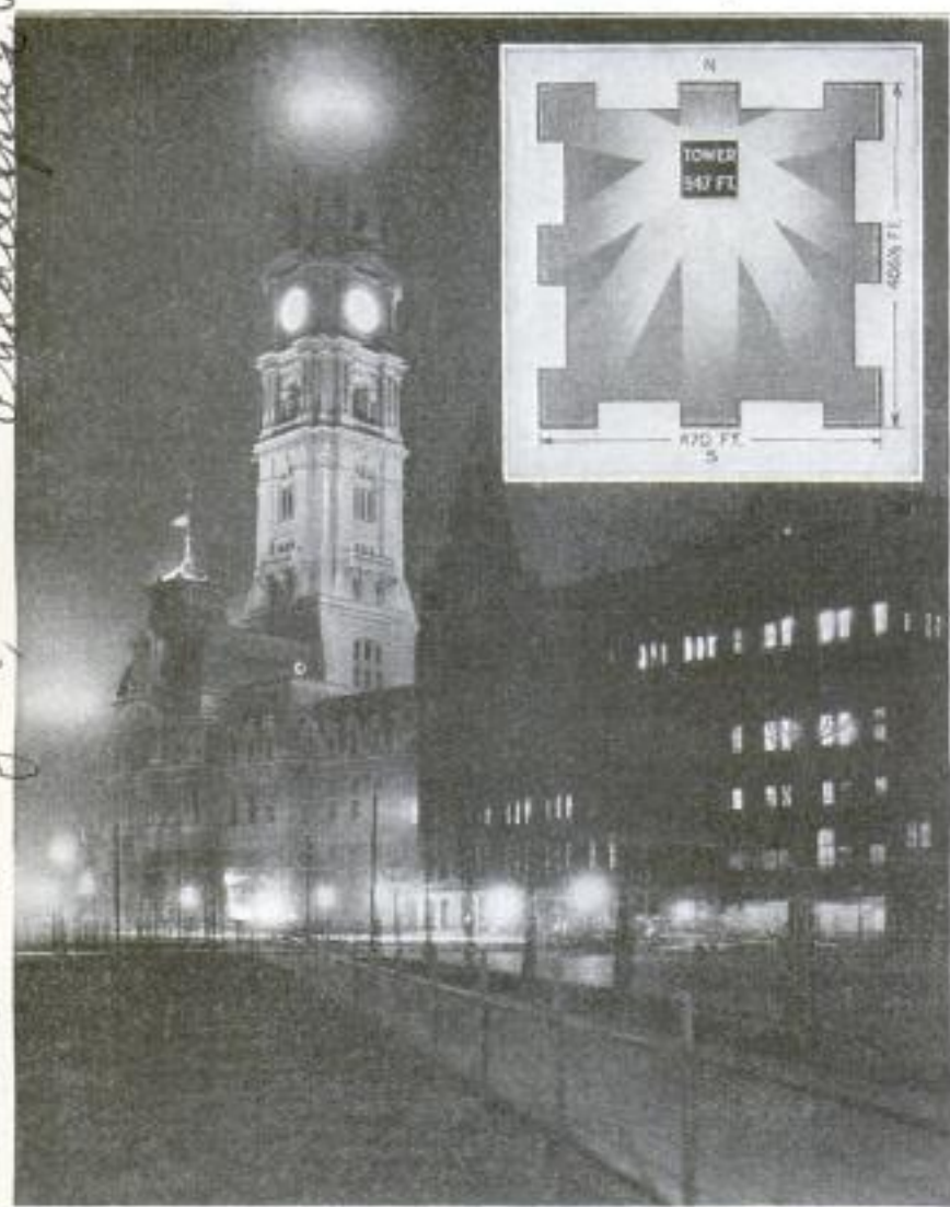
City Hall of Philadelphia Illuminated for New Year's Celebration: Two Faces of the Huge Clock are Seen on the Tower. Insert: Plan View of Building, Illustrating the Lighting Arrangement. Each Extreme Corner Has 38, and the Intermediate Points 37 Lamps
