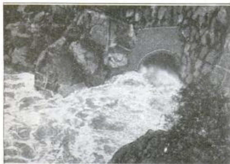
The Outlet of the Flood-Control Tunnel is Located at Some Distance down the Cañon in Order That the Released Waters Rushing Out may Not Undermine the Foundations of the Dam
