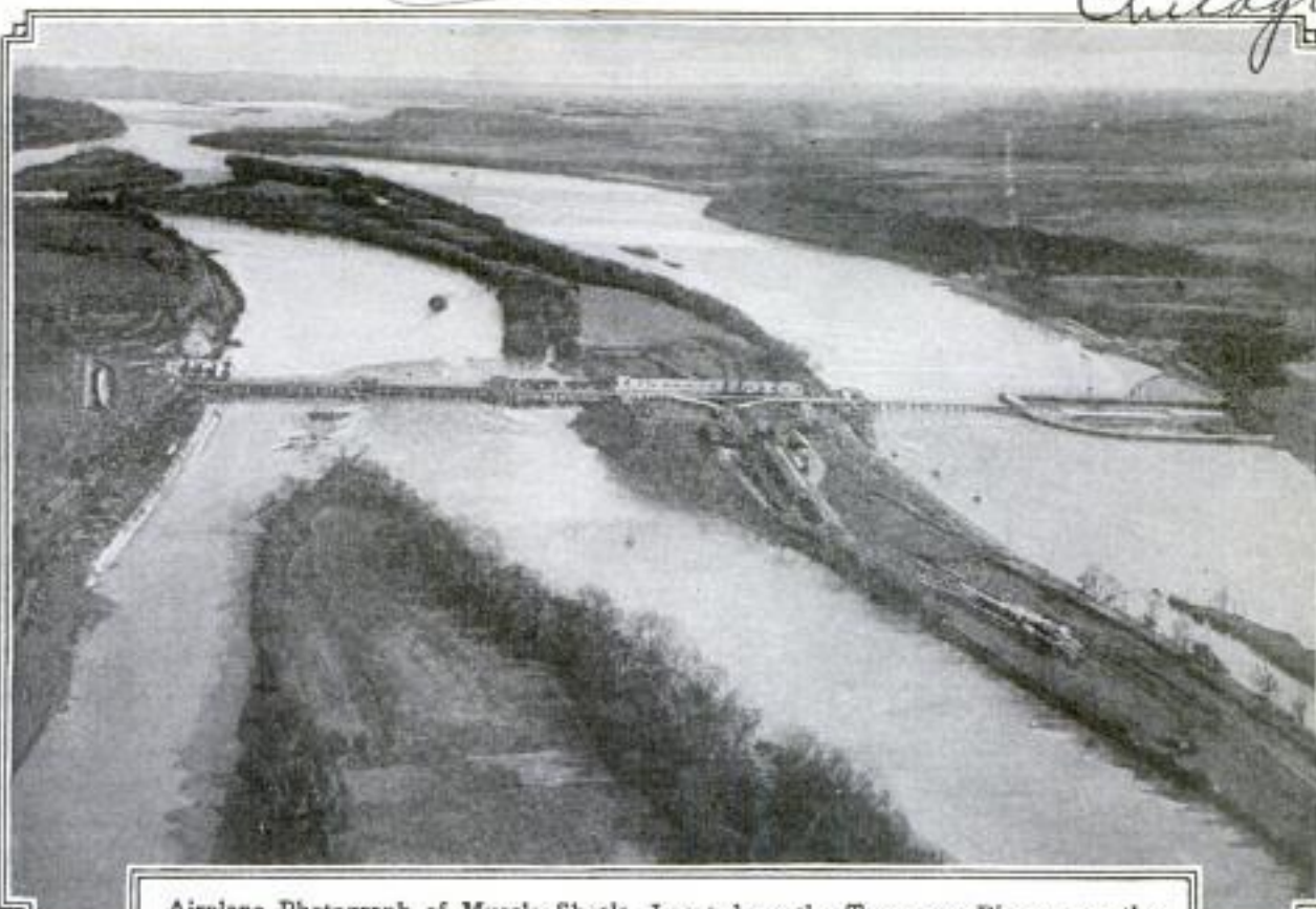
Airplane Photograph of Muscle Shoals, Located on the Tennessee River, near the Northwest Corner of Alabama: Across the Shoals is Seen the Wilson Dam, Now About One-Third Finished, Which will Be 4,426 Feet Long, and 160 Feet Wide at the Base—the Largest Example of Monolithic Concrete Construction in the World
