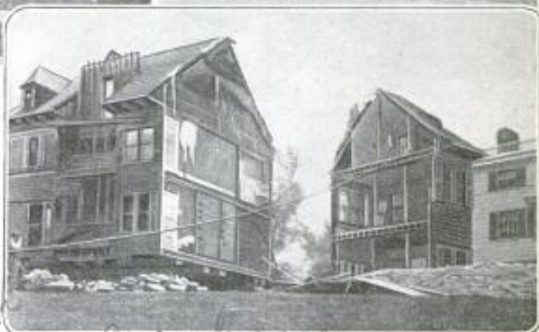
Above: Left, One of the Halves of the House Which was Cut in Two Parts, as It Appeared When Finished and Ready for Occupancy; Right, the Other Half of the Dwelling after having been Given a Covering of Tar Paper While Waiting for the Carpenters to Begin Remodeling. Below: The House Immediately After It had been Severed in Twain, with One of the Halves being Moved to a New Location. The Unusual Undertaking was Made Possible by the Substantial Manner in Which the Old Mansion was Originally Constructed
