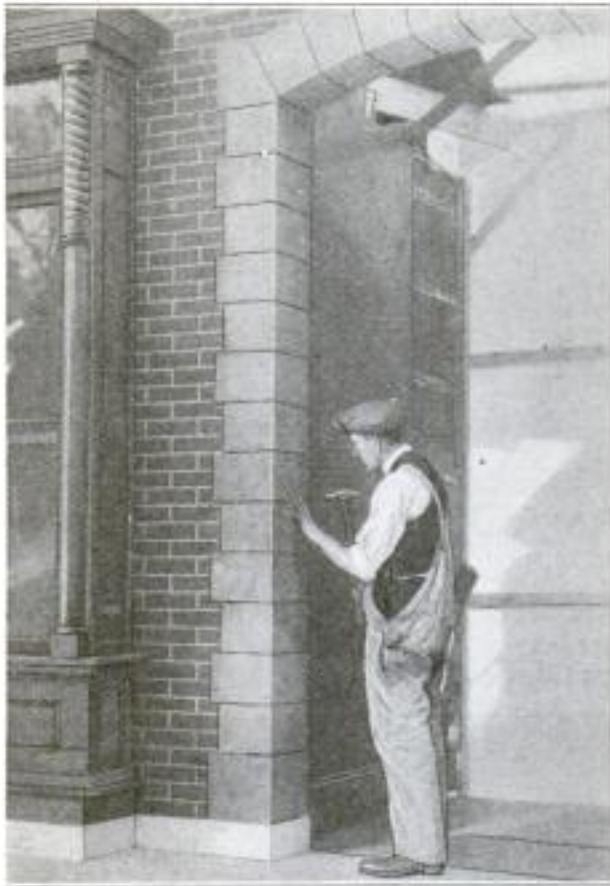
This Imitation Stone Doorway of a Motion-Picture Set is Made by Tacking Sheets of Sandpaper on Wood to Represent Concrete Blocks
