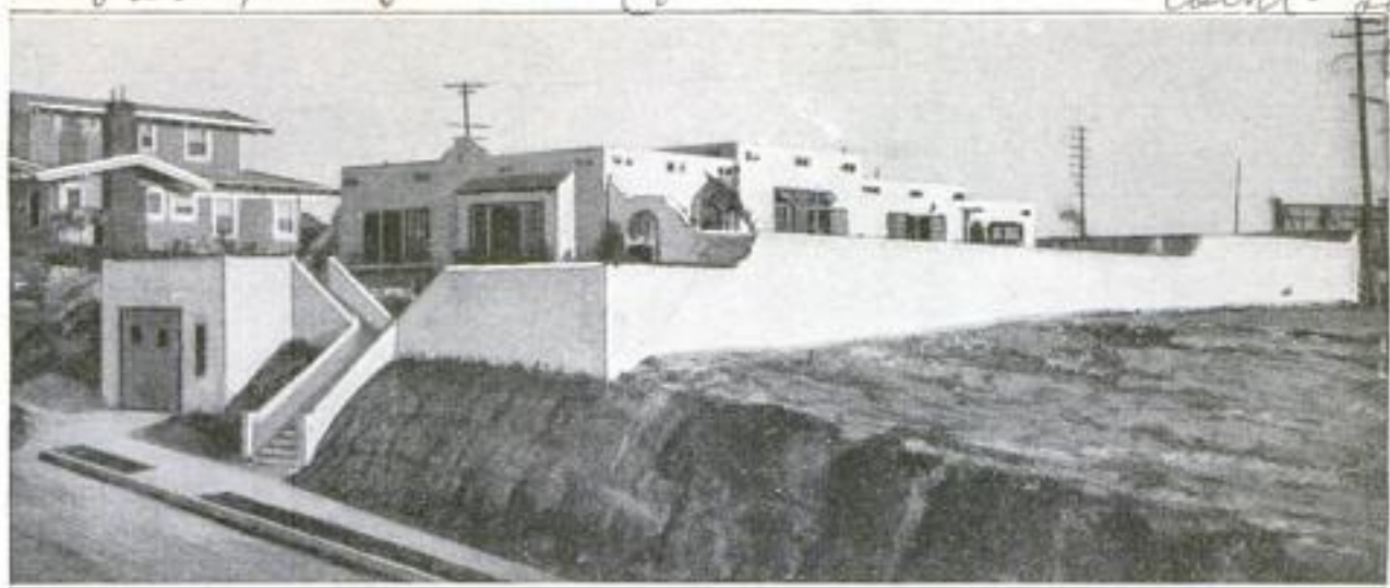
This Seven-Room Bungalow, with all Modern Conveniences, was Built by the New Cement-"Shooting" Process and Has Walls Five and Six Inches in Thickness. The Surrounding Garden Wall Is Only Two Inches Thick and Has Seats Constructed into It in Such a Manner That the Whole Is One Solid Mass
