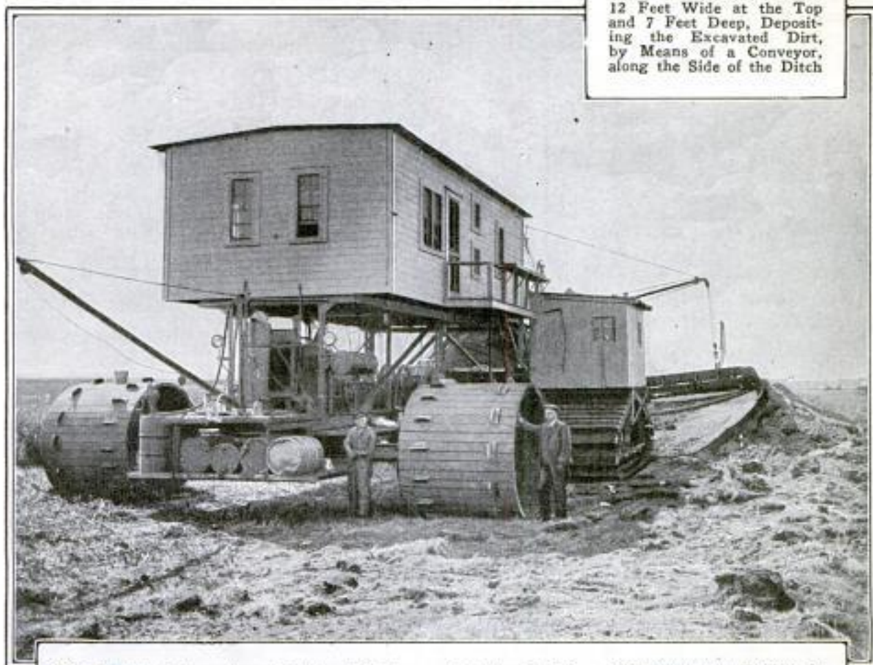
The Immense Excavator, Weighing 76 Tons and Equipped with a 110-Horsepower Engine, is Here Seen from the Front. It is 65 Feet Long over All, and 33 Feet Wide; the Front Wheels Are 8 Feet High by 7 Feet Wide, and the Track-Layer Wheels in the Rear, 20 Feet Long by 8 Feet Wide. The Crew Eats and Sleeps in the House on Top of the Machine
