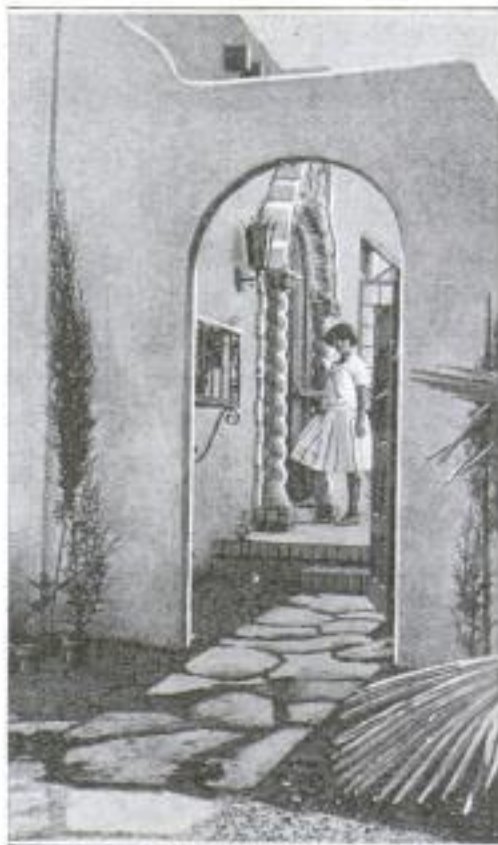
Garden of the Bungalow, Illustrating Some of the Ornamental Effects Obtained by Using the Cement-Shooting Process
