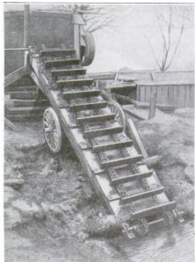
The End of This Peculiar Pump is Lowered into Canals Which are to be Emptied of Water for Cleaning. The Outside Box is Here Removed
