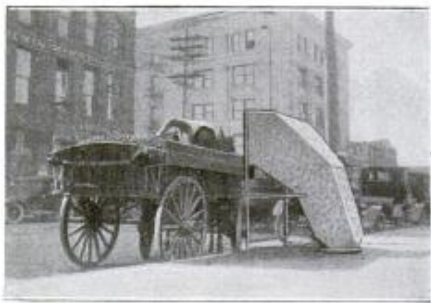
Inclosed Chute Placed in Position over a Manhole for the Purpose of Unloading Slack Coal without Producing the Usual Dust
