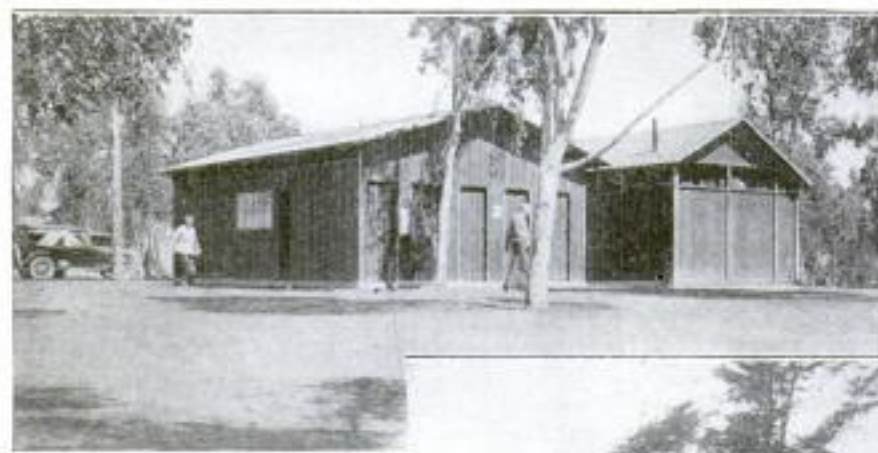
The Building on the Left Is One of the Sanitary Toilet Houses of the Village, While the One on the Right Is a Laundry. Both Structures Possess Modern Plumbing
