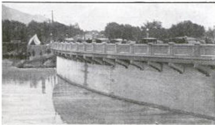
The Dam Presents a Curved Surface on the Upstream Side and Has the Appearance of a Concrete Wall along a Lake
