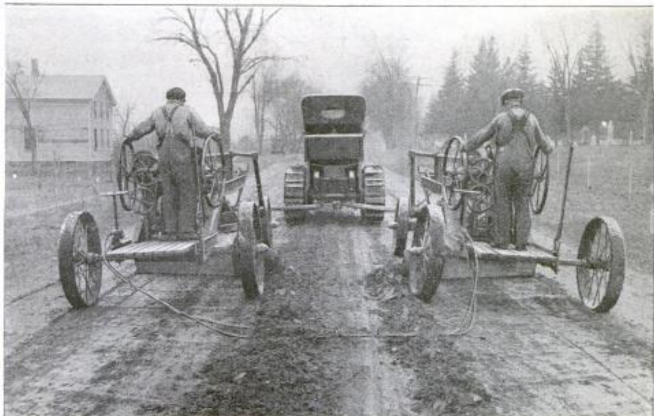
Showing How the Tractor Keeps to the Center of the Road: The Space between the Graders may be Varied to Suit the Width of the Road. The Cable is Used as a Towline in Crossing Narrow Bridges
