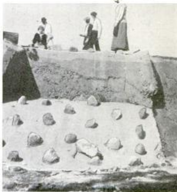
The Face of the Dam, Showing How the Rocks are Imbedded in the Concrete to Procure the Effect of a Foaming Waterfall
