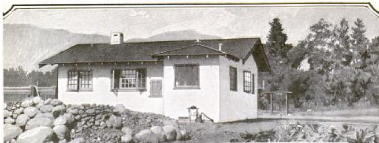
Rear View of the Bungalow: The Foundations were Kept Entirely below Ground to Avoid Giving the Appearance of a Box Sticking Up in the Air. The Effect of This Toylike House Is Artistic Throughout
