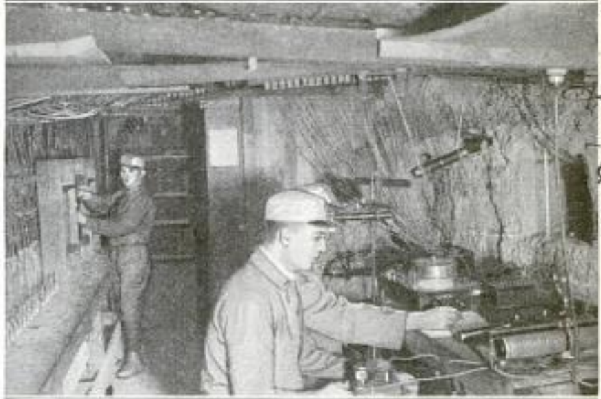
Air-Sampling and Temperature-Measuring Station at Entrance to Experimental Tunnel: Forty-Eight Samples from Different Parts of the Tunnel are Taken to This Station for Testing. Temperatures in All Parts of the Tunnel are Measured
