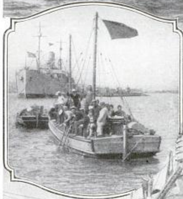
Left: In the Foreground Is the Small Tug Engaged in Pumping the Water Out of the U. S. Submarine "R-6" Which Sank Suddenly While Moored alongside the Submarine Tender "Camden." Seen in the Background, Behind the "Camden" Are Other R-Type Submarines. It Took Fifteen Days to Raise the "R-6." Only Two of the Crew Were on Board When It Sank
