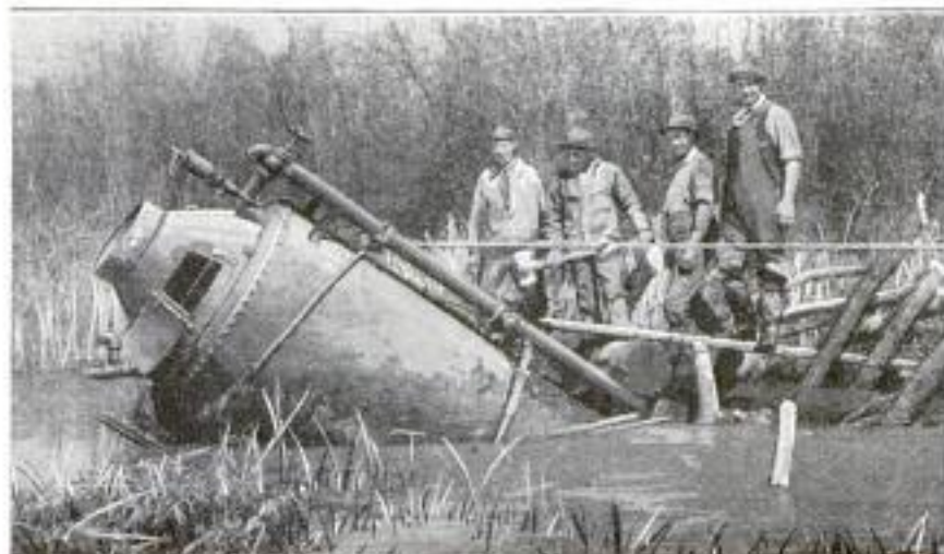
The Raising of the Donkey Engine by Means of the Stump Puller and a Rope Fastened around the Top of the Sunken Machinery: In This Manner the Engine was Dragged to Dry Land
