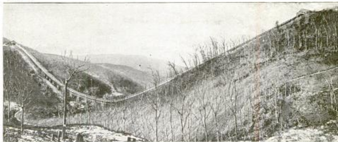
Long Conveyors Carry the Coal, from Mines on Opposite Hill-tops, to a Common Tipple, on a Railroad in the Valley Lying between the Hills
