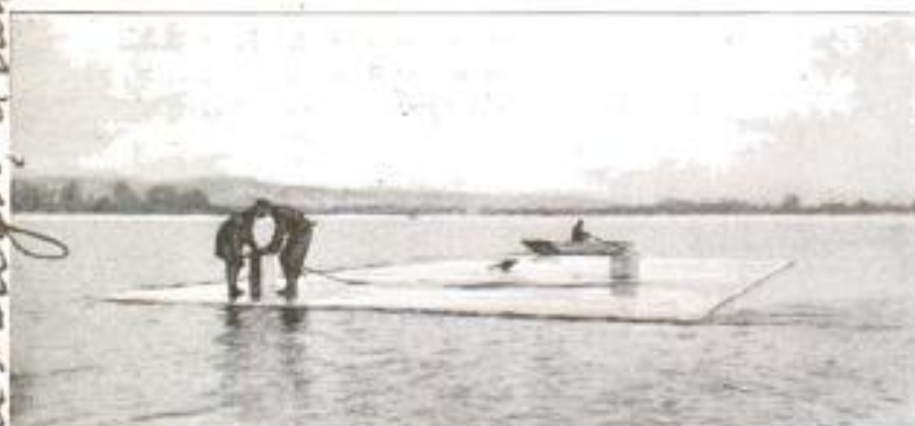
An Ice Cake being Carried along the Ferry Cable, Using the Current to Transport the Ice across the Open Channel
