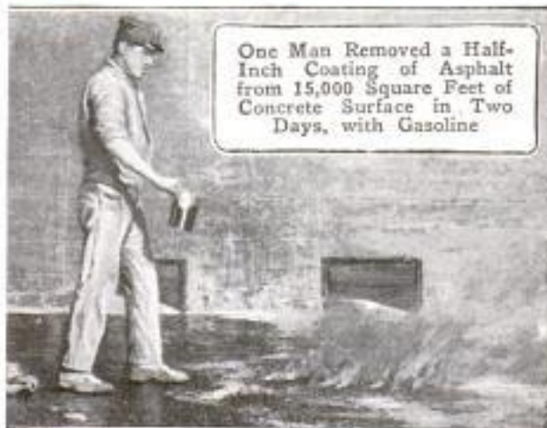
Photo from Waterproof Paint Co., Lancaster, Calif.
