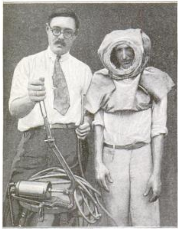
The Complete Diving Helmet and Air-Supply Pump Which Gives Satisfactory Results in Water of Any Depth Up to 20 Feet
