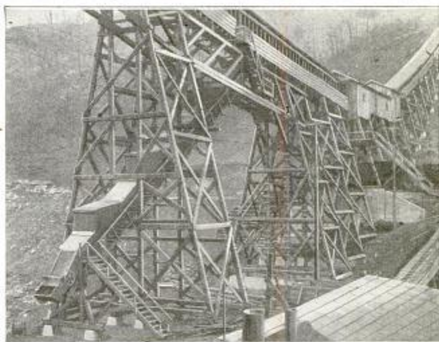
The Conveyor Trestles Consist of Towers and Trusses Built of Timbers Which were Shipped Ready-Cut and Numbered
