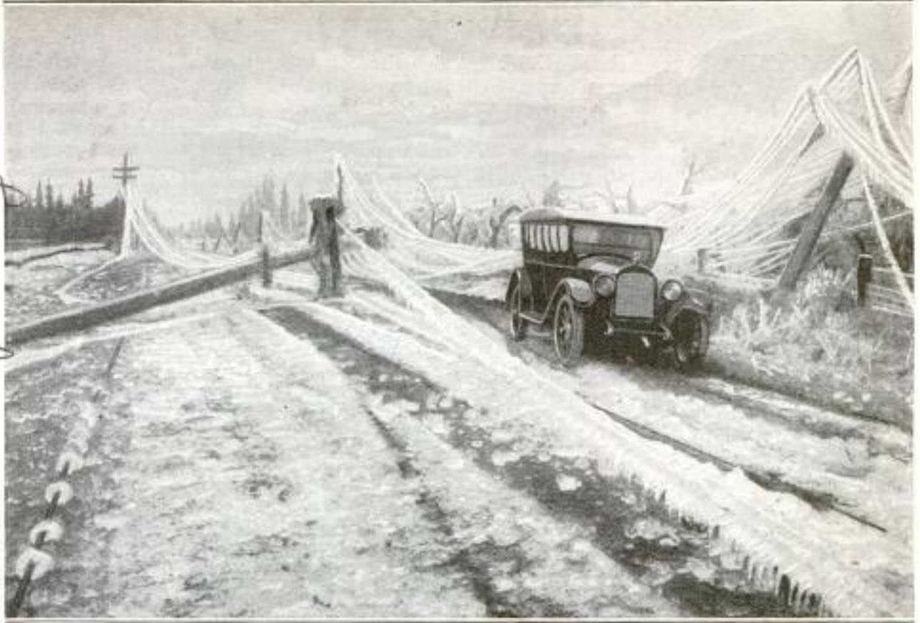
Near Portland There Was No Snow, but an "Ice Storm" Left the Country as Shown Above, with Telephone Poles Down, Trees Broken, and Orchards Ruined. Where the Snow Fell, Drifts Almost Covered Telephone Poles, as Seen Below. This View Also Shows a Path from a Train, to Take the Passengers to a River Boat
