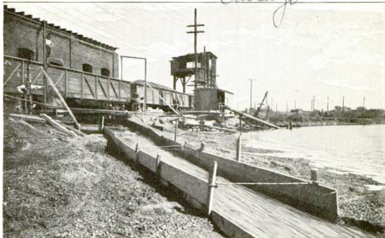
Illustrating the Manner of Unloading a Carload of Coal Screenings with the Aid of Water Which is Pumped from the Pond and Directed into the Cars at Either End: The Screenings are Washed down the Chute into the Pond, Where They Are Safe from the Danger of Spontaneous Combustion
