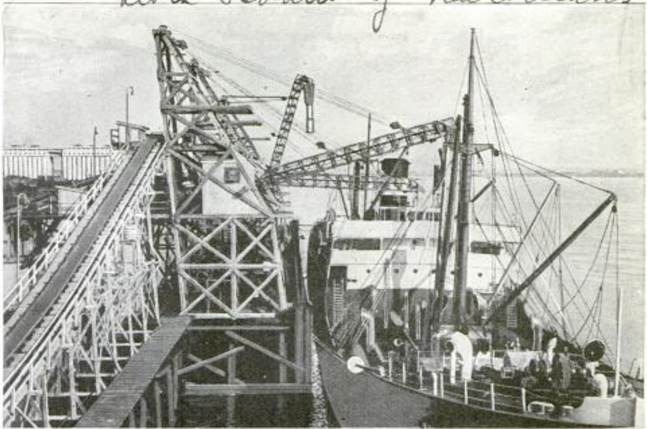
Steamship "Emergency Aid" being Loaded with 550 Tons of Coke at the New Coal-Handling Plant at New Orleans, Louisiana, Operated by the Board of Commissioners of That Port
