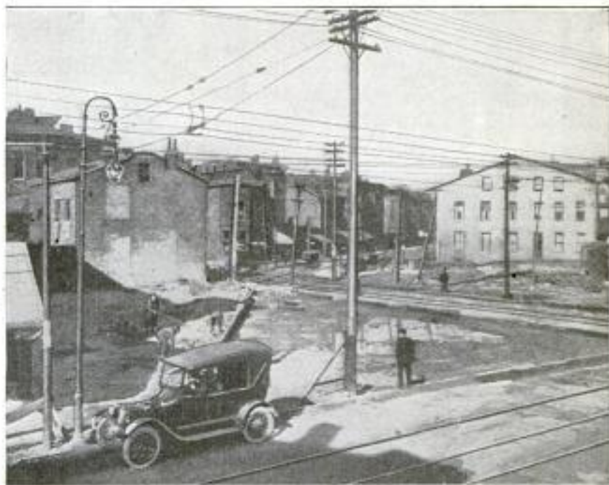
This Intersection Was So Narrow That One Street Car Turning the Corner Blocked All Other Traffic. Buildings have been Torn Down, and the Corner is being Widened. It will Be One of the Widest in the City
