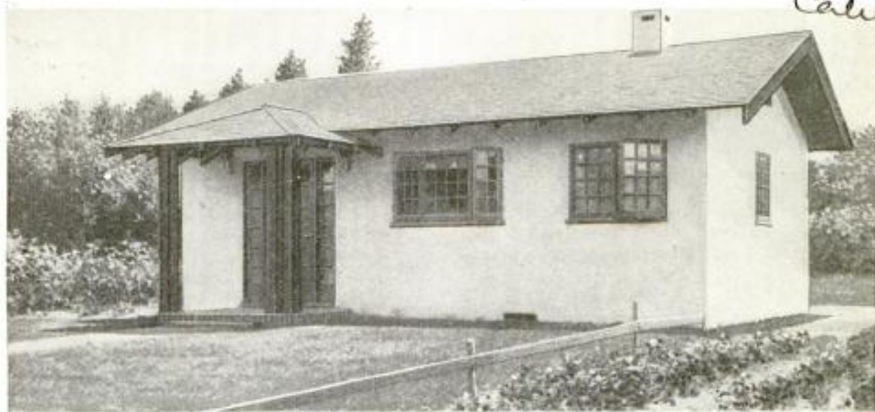
One-Room Bungalow, in Which the Owner Employed His Practical Experience as a Boat Builder to Utilize Every Inch of Space to the Best Advantage, without Sacrificing Attractiveness of Appearance
