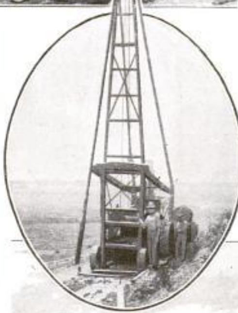
A Small Gasoline Engine Furnishes Power to the Pumps of an Entire Row of Wells through a Single Cable, Which is Fastened to the Pump at Each Well
