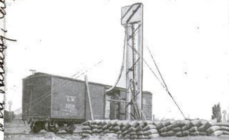
Loading a Box Car with Bulk Grain by Means of a Simple New Conveyor Device: It is Made in Two Sizes, One Handling 1,000 and the Other 2,000 Bushels an Hour, and Is Inexpensive to Operate
