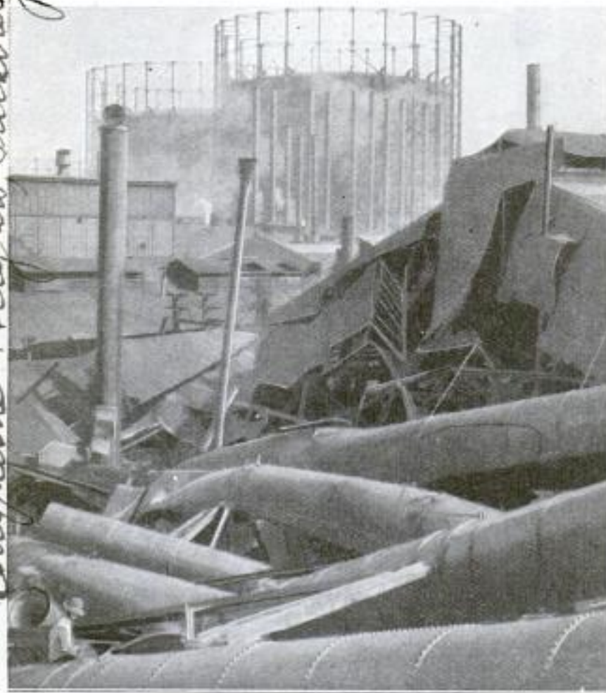
Showing the Havoc Wrought to 11 Steel Smokestacks at Pittsburgh by a High Wind: In the Foreground are Seen the Prostrate Stacks, Some of Which Smashed against and Wrecked Near-By Buildings
