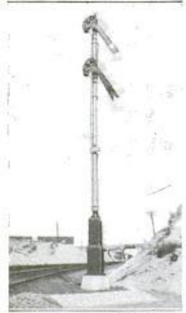
Ordinary Type of Railway Signal in Which Semaphores Hang Vertically to Indicate Safety or as Shown to Indicate Caution
