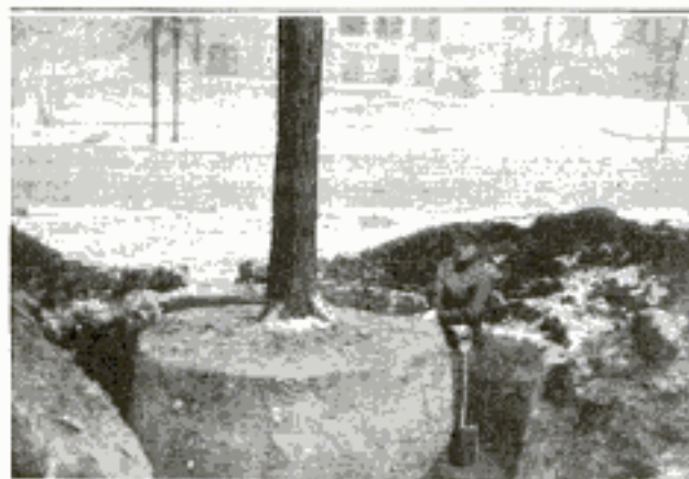
Showing the Method of Trenching around the Tree and the Appearance of the Root Ball: Many of the Feeder Roots are Cut in This Operation, and This Requires a Subsequent Thinning Out of the Branches
