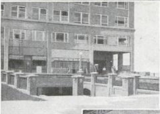
Third-Floor Street Entrance: The Steps Lead Down to the Lower Floors
