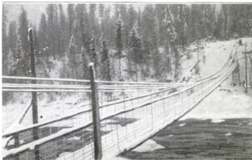
Footbridge Suspended by Means of Cables Which were Originally Intended to be Used as Part of a Telegraph Line from New York City to Paris, France, by Way of Alaska and Siberia
