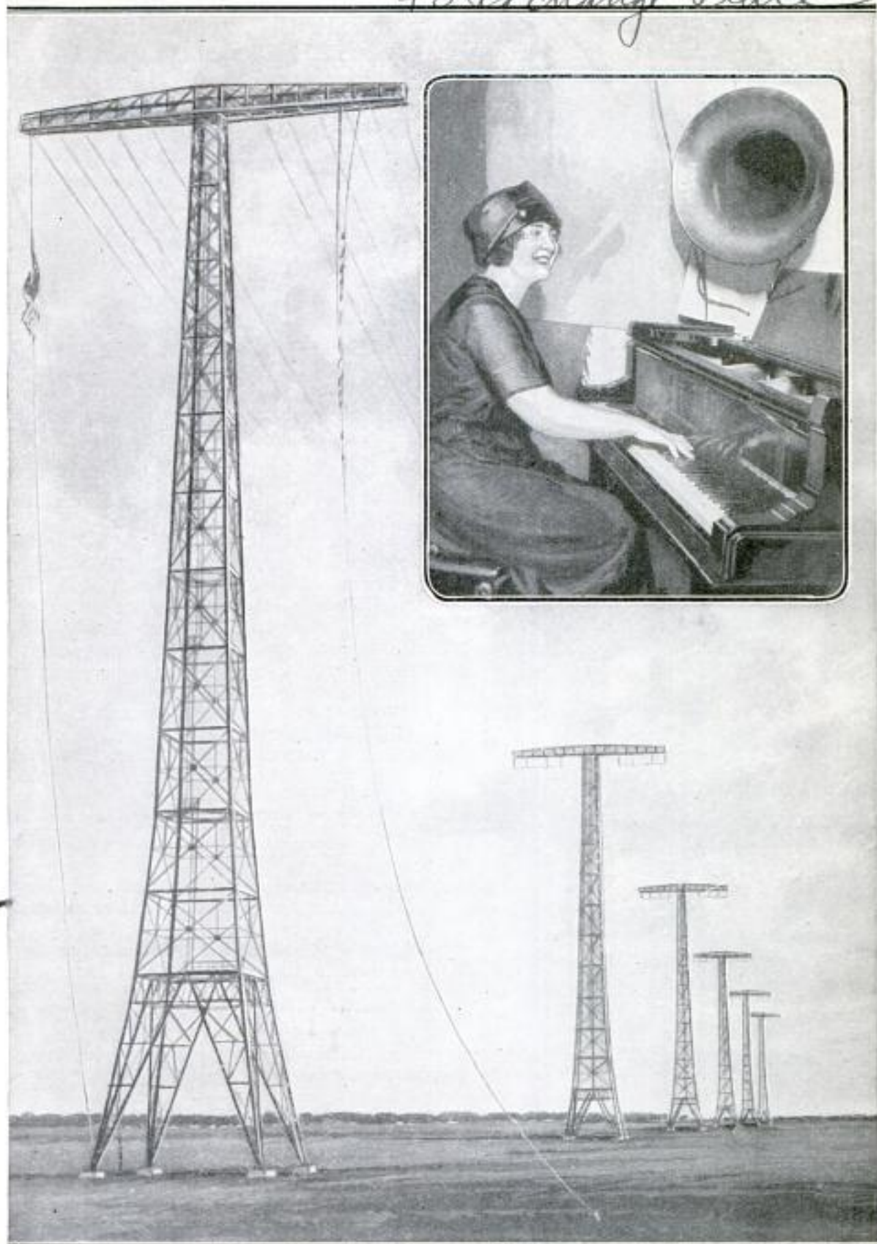
SIX of the 72 gigantic towers of the world's largest wireless station at Port Jefferson, L. I., which was formally opened by President Harding on Nov. 5, 1921, are shown here. The station, which was described by this magazine in the September 1920 issue, is operated entirely by remote-control apparatus from New York City—70 miles distant. Insert shows an artist giving a piano recital by wireless, said to be the first of this kind ever given, and estimated to have been heard by 35,000 persons between Maine and Texas.
