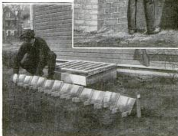
Outside Shutters Converted into Neat and Substantial Storm Windows by Merely Removing the Slats and Substituting Glass Panes: Even the Old Slats can be Used to Further Advantage for the Protection of Tender Plants, as Shown at the Left
