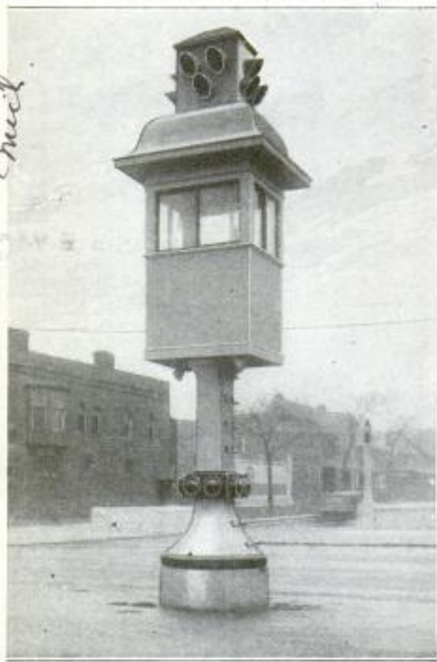
With Traffic Towers like This, It Is Only Necessary to Have a Traffic Officer Every Four Blocks to Get Perfect Traffic Control
