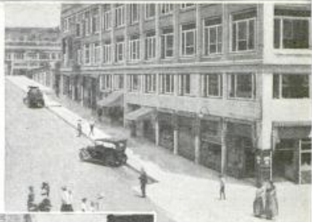
The Sloping Street, Showing How There Are Street Entrances to Three Floors
