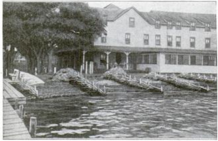
The Barriers are Built to Trap Seaweed at the Ebb of the Tide. The Weed is Then Raked into Stacks at the Farther End of Each Barrier
