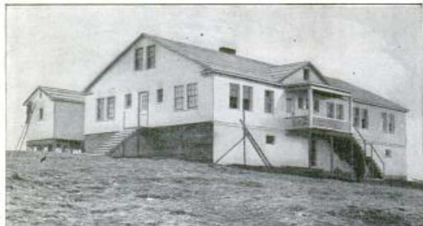
The Point Barrow Hospital as It Appeared When Completed Last Summer: The Building, Constructed of Wood and Tar Paper, was Finished with Two Coats of White Marine Paint
