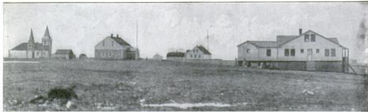
The Principal Buildings of Point Barrow, the Farthest-North Settlement in North America: At the Left Is the Church, in the Center the Mission School, and at the Right the New Hospital. The Two Nearest Modern Settlements Are 300 Miles to the South and 400 Miles to the East
