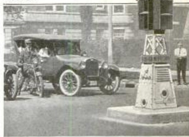
The Controller being Tried in Milwaukee: The Shutterlike Arrangement Is to Prevent the Light from being Seen from the Side
