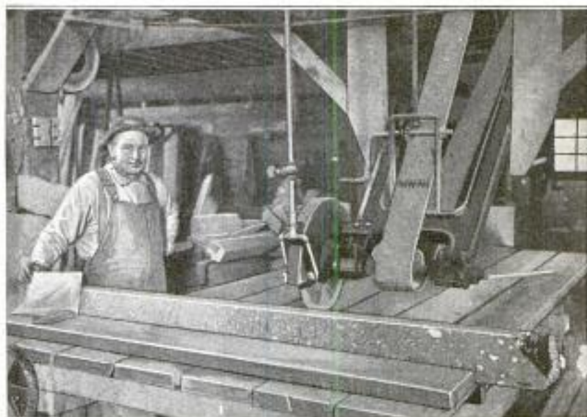
Another Scene in the Tufa "Lumber" Mill: Here the Stone is being Cut into Timbers, for Building Construction, by Means of a Carborundum Wheel, Used in the Same Way as a Circular Saw. This Machine Shows the Greatest Variation from the Lumber-Mill Type Equipment
