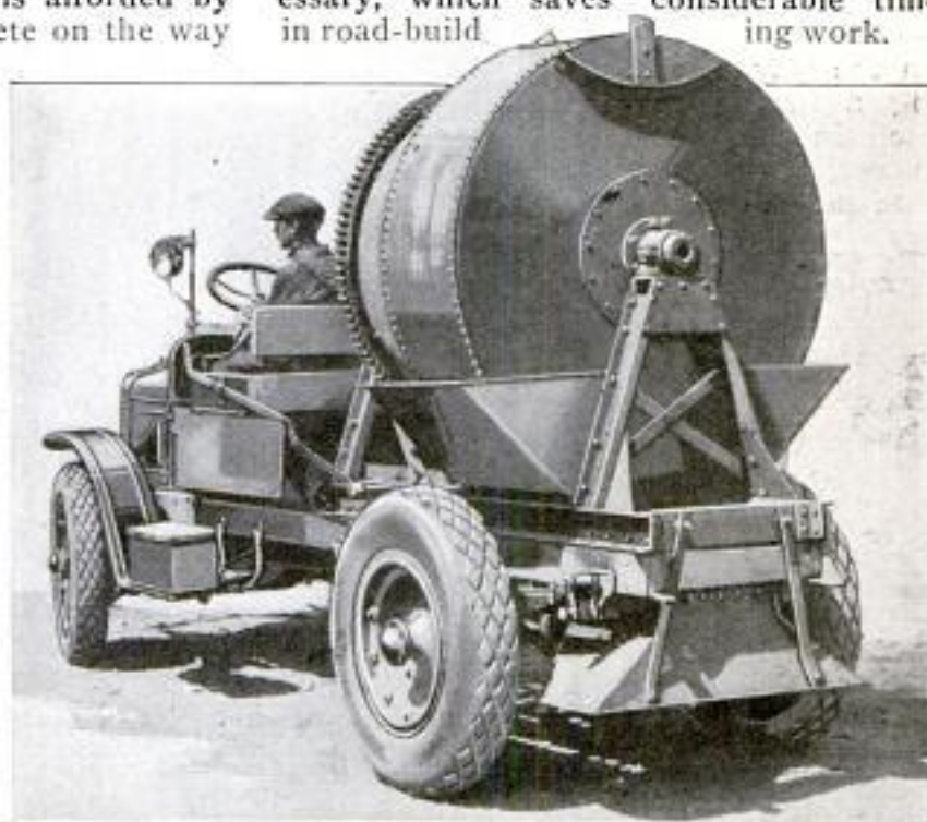
This Concrete-Mixing Drum is Operated by the Motor of the Truck on Which It is Mounted. It can be Rotated While the Truck is Moving at Any Speed, or While It is Standing Still
