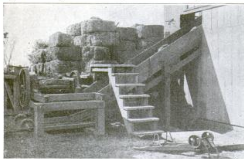
Baled Bagasse, the Waste Product of Sugar Mills, being Received at the "Lumber Factory" Where, by a New Process, It is Made into a Building Board Which Serves as a Substitute for Wood
