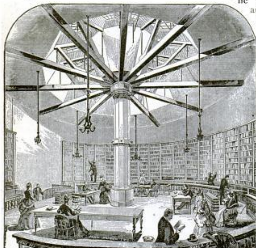
BY COURTESY OF THE CHICAGO BOOK BULLETIN An Iron Water Tank, 60 Feet in Diameter, 30 Feet High, and Standing on a 35-Foot Masonry Base, Which had Survived the Fire, was Provided with a Skylight, Bookshelves, and Tables, and This Became the First Chicago Public Library
