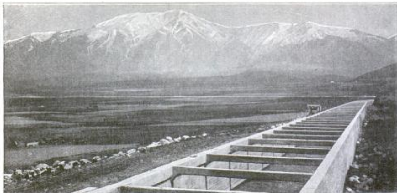
A Colorado Irrigation Canal Built Entirely of Precast Concrete Sections: For the Smaller Canals, This Method is Often Preferred to That Shown in the Preceding Illustrations
