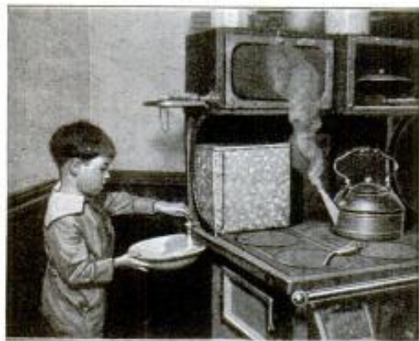
A Three-Gallon Tank, Made from Galvanized Iron, Provides an Ever-Ready Supply of Hot Water for the Kitchen
