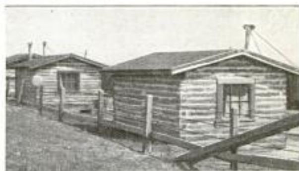
Huts Built of Ties Bound with Cement are Now Used Instead of Dilapidated Box Cars for Housing Laborers along the Southern Pacific Railway
