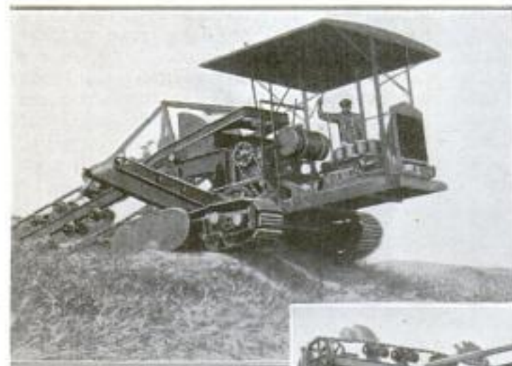
Trenching Machine with Endless-Tread Traction Resembling That Used on Military Tanks
