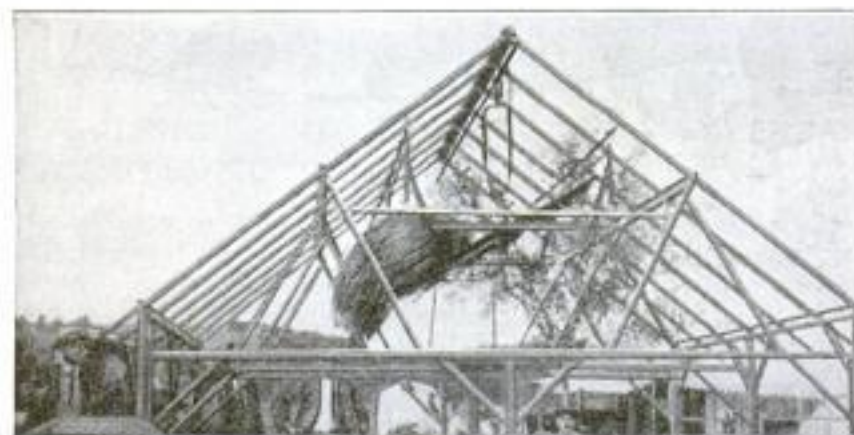
When the Rope is Pulled, the Platform of the "Mower" Tips to the Side, as Shown Here, and Dumps the Hay Well Over to the Side of the Loft, So That It Requires No Hand Distribution
