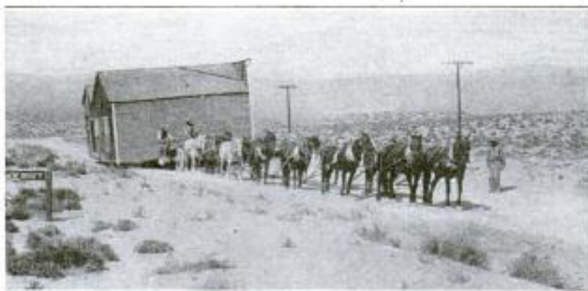
Hauling a House from Goldfield to Tonopah, Nevada, across 35 Miles of Desert: This Was a Common Sight during the Recent "Boom," When the Population of Tonopah Jumped from 3,000 to 15,000 in Four Weeks
