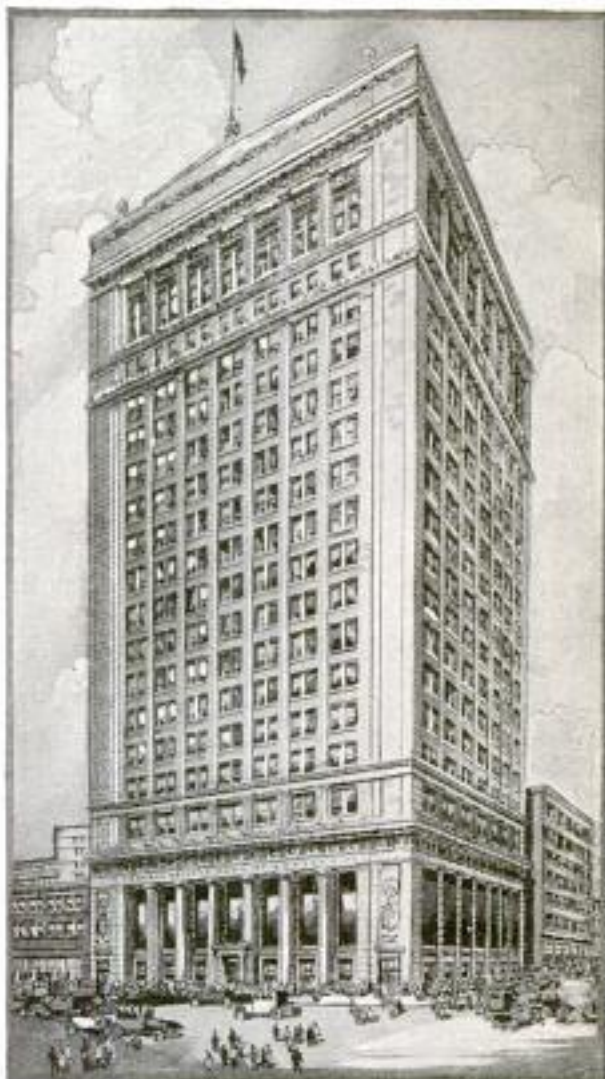
The New Federal Reserve Bank Building, Nearing Completion in Kansas City, Missouri
