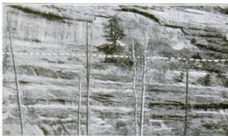
At the Cliff the Roadway will Be 20 Feet Wide. Traffic will be Protected from the 40-Foot Drop Below by a Concrete Wall along the Outer Edge of the Roadway
