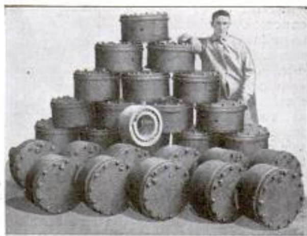
The Roller-Bearing Equipment of a Single Door of the Great Lakehurst, New Jersey, Dirigible Hangar is Shown Here
