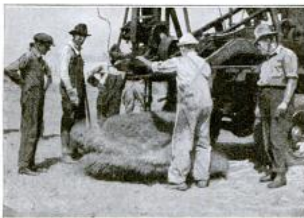
The Bit is Then Whirled and the Dirt Falls Off, Not Back into the Hole but, Because of the Whirling Motion, beside the Hole
