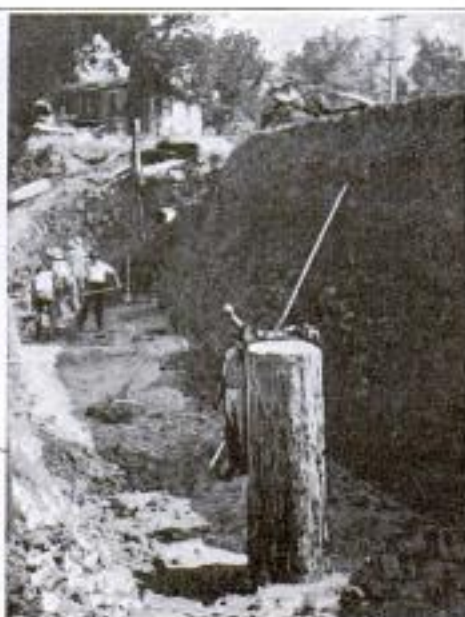
At the Left: The Interurban Tracks as They Appear Since being Moved onto the Roadway, Out of the Way of Construction. Beside Them Are the Old Tracks along the Edge of the Bluff. At the Right: The Excavation for the Retaining Wall Which is to Keep the Road from Sliding Downhill
