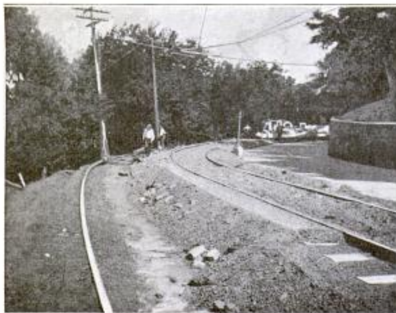
At the Left: The Interurban Tracks as They Appear Since being Moved onto the Roadway, Out of the Way of Construction. Beside Them Are the Old Tracks along the Edge of the Bluff. At the Right: The Excavation for the Retaining Wall Which is to Keep the Road from Sliding Downhill
