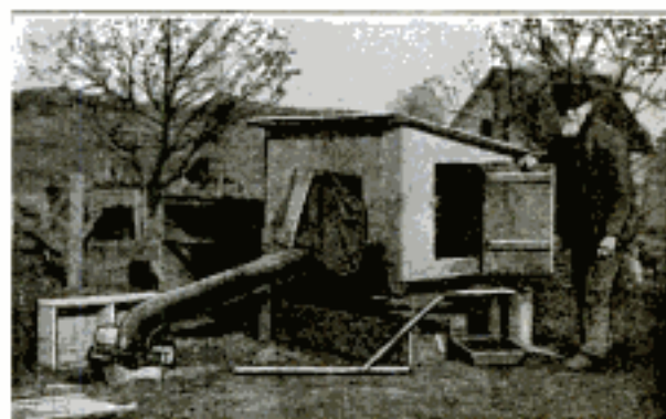
An Improved Smokehouse for the Curing of Pork can be Built and Operated at Practically No Expense. Hickory Wood or Corncocks are Used for Producing the Smoke
