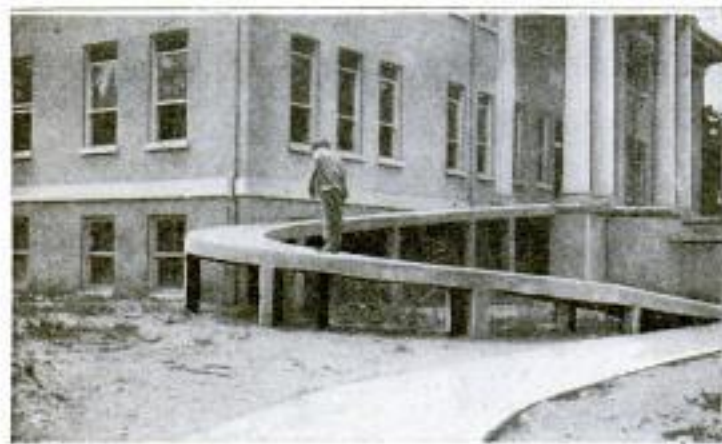
For the Wheel-Chair Patients in an Adjoining Sanitarium, the College Hall has been Made Accessible by Means of This Concrete Incline, Which Affords an Easy Mode of Entrance
