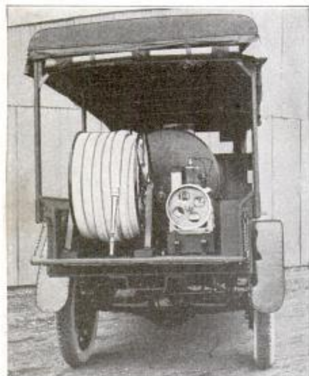
The Equipment of These Trucks Consists of a Water Tank, Hose, and Pumping Engine, besides the Tools Commonly Used in Fighting Forest Fires
