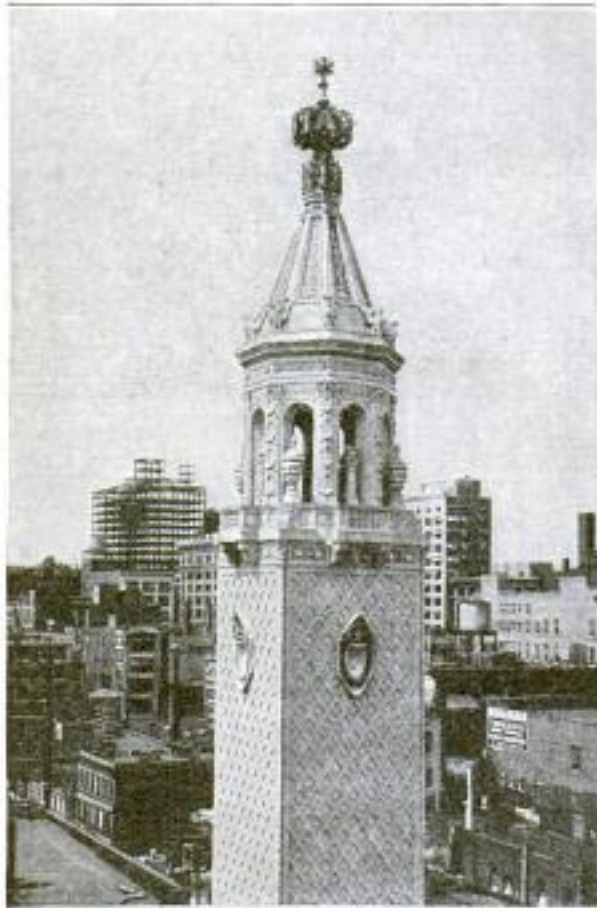
The Tower of a New Theater in Kansas City, Missouri, Surmounted by a Revolving Illuminated Sign Bearing the Name
