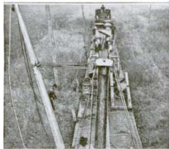
A Method of Stringing Wires along a Railroad Right of Way That Resulted in the Job being Finished Ahead of Contract Time: The Equipment Is Simple and Enables a Much Smaller Crew to Do the Work with Less Labor, Especially Where Very Heavy Wire is Handled
