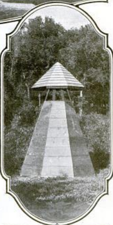
One of Several Wooden Dressing Shelters along the Banks of the Red River, in North Dakota, Which Resembles a Glorified Indian Teepee: It Is Octagonal and is Inclosed to a Height of Eight Feet, with an Umbrellalike Roof Above
