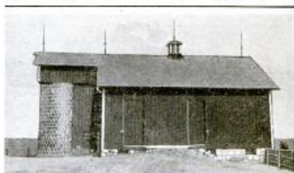
By Building the Silo Close to the Barn and Extending the Roof of the Latter over It, the Silo is Well Braced against the Wind
