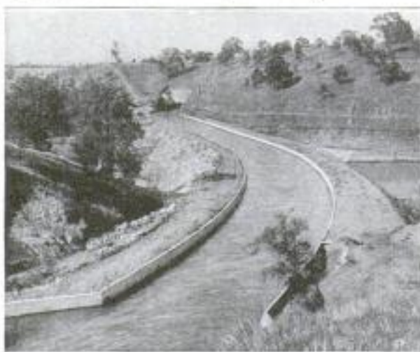
The Canal, Shown under Construction on the Opposite Page, Completed and in Use
