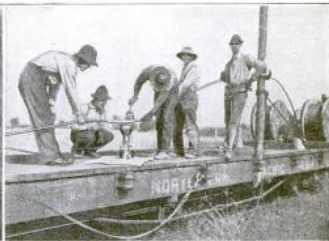
A Method of Stringing Wires along a Railroad Right of Way That Resulted in the Job being Finished Ahead of Contract Time: The Equipment Is Simple and Enables a Much Smaller Crew to Do the Work with Less Labor, Especially Where Very Heavy Wire is Handled
