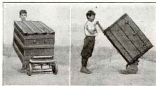
When the Mower is Reversed the Blades do Not Revolve as the Load is Pushed Forward
