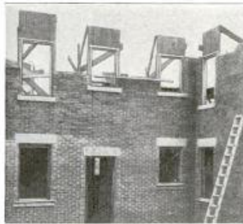
Window Frames with Screens, Sash, and Box Heads Built as a Unit: Above, They are Seen being Built into a New Wall; Immediately to the Right is an Outside View of One, Showing Relation of All Parts, Which, Farther to the Right, are Described by Notations
