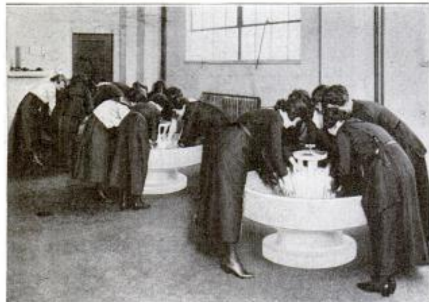
The Fountain Washbowl in Use: The Fine Streams of Water, Controlled by the Hand Valve on Top, Are Very Effective. The Fountain is Equipped with Sanitary Liquid-Soap Containers, or Receivers for Cake Soap, as Desired
