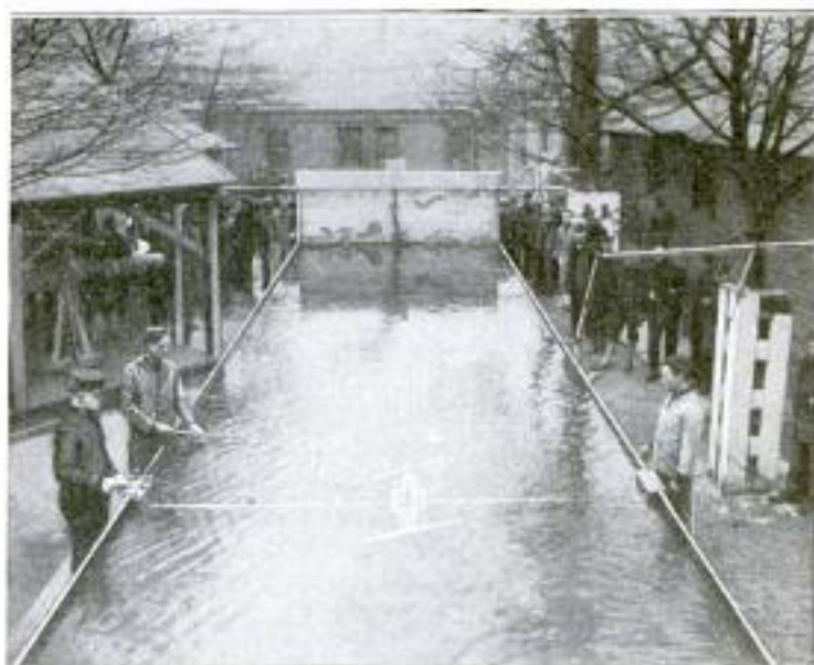
The Men at the Sides are Using the Submerged Movable Air Tubes to Show with a Bubble the Range and Deflection Called by the "Spotter." Left: The Movable Air Tube Shown in the Empty Tank
