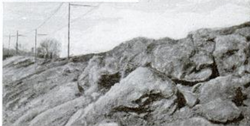
This Is How the Railway Embankment Looked after the Extinction of the Fire. It will be Seen That There Was Not Much Destruction of Material
