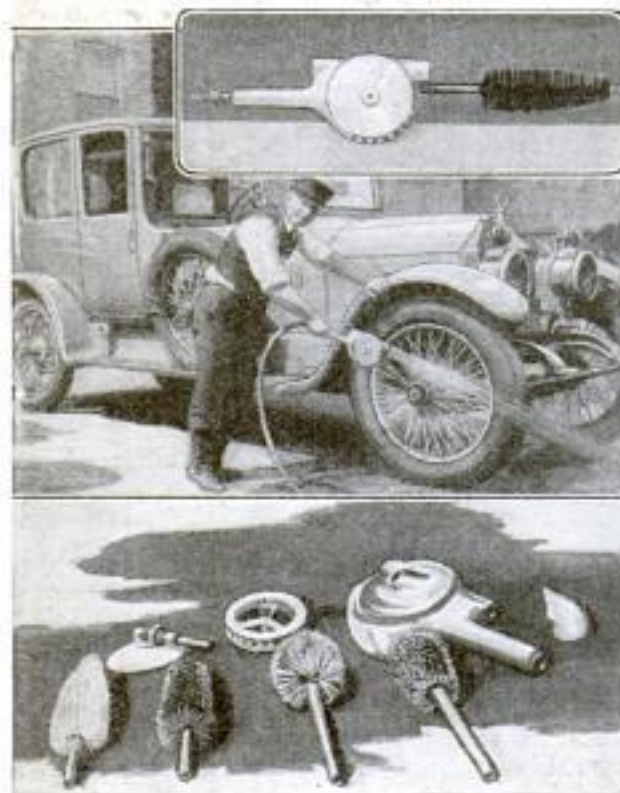
Upper Right Corner: Turbine Auto Brush. Center View: Force of Water from Garden Hose Revolves and Sprays Brush for Cleaning. Bottom Picture: Brush Disassembled
