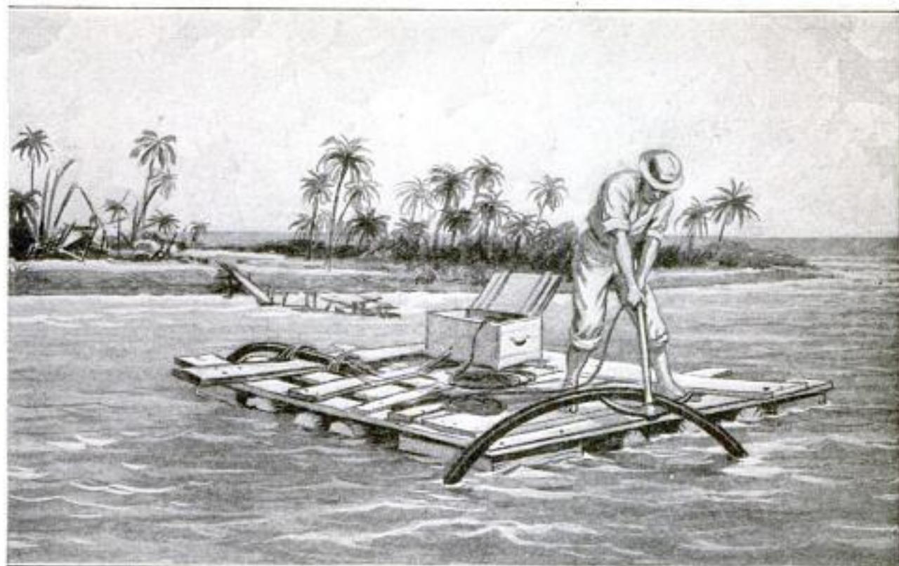
The Officer at Fanning Island, after the German Raid and Destruction of the Cable Station, is Seen Raising One End of the Cable with a Pickax, the Only Form of Grappling Hook Available, Which He Later Spliced to the Other End, Previously Tied to His Improvised Raft
