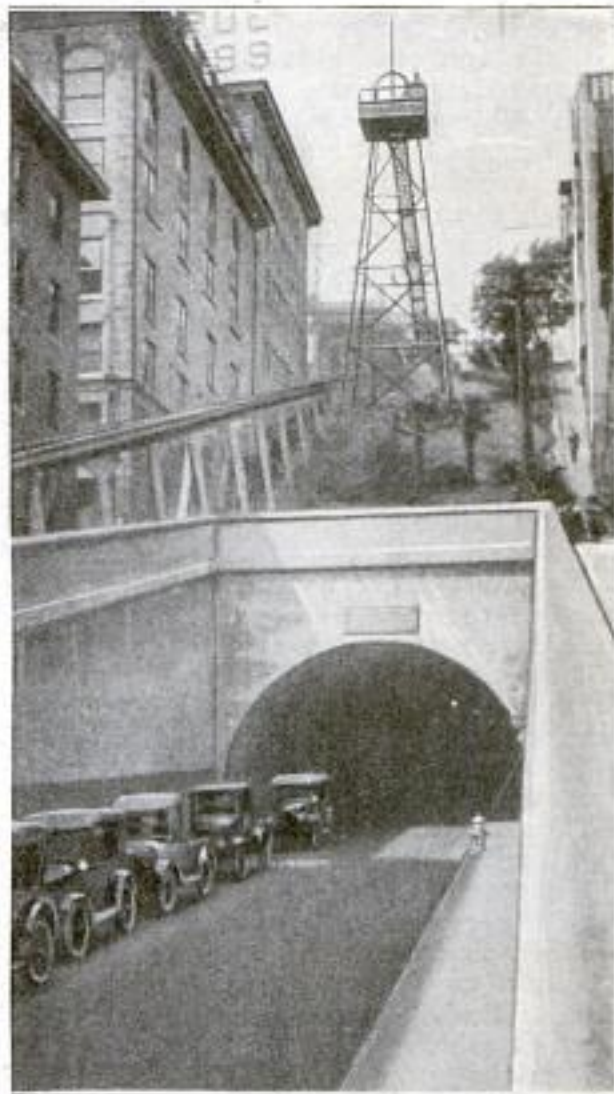
East Entrance to Third Street Tunnel, Showing the Manner in Which Motor Vehicles Line Up in This Poorly Ventilated Passageway When Traffic Is Heavy
