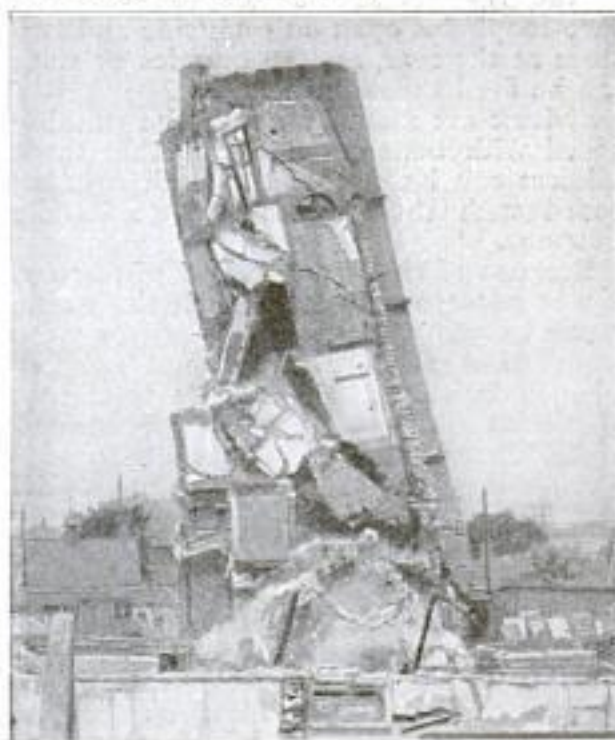
Church Tower at Toronto Photographed Just as It Began to Fall: The Walls had been Undermined in Connection with Street Improvements Requiring the Razing of the Church
