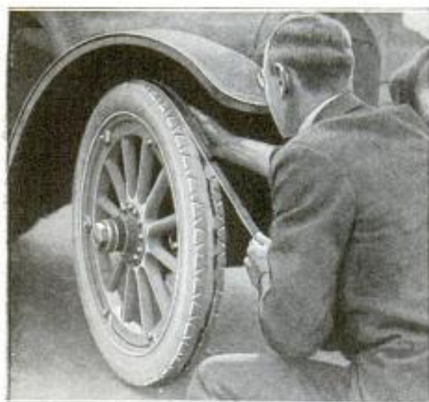
Winding a Patented Rubber Strip Circumferentially about the Casing Is a New Method of Repairing Worn Tire Treads
