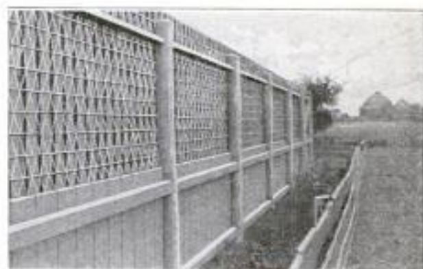
Outside View of Fence with Tight Board-Bottom Section and Reinforced Woven-Wire Upper Section, Resists Efforts of Wild Horses
