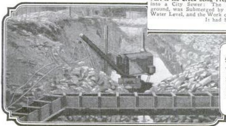
An Example of the Rocky Excavations That had to be Made in Places by Means of Heavy Blasting. The Side Walls and the Floors of These Excavations have to be Trimmed
