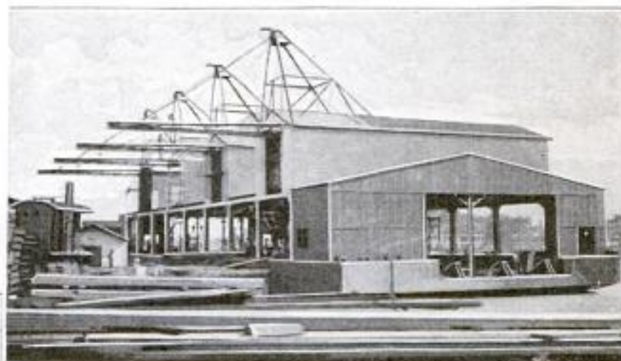
Above: Floating Wharf for Loading and Unloading Freight from Barges to the Shore in the Greatly Varying Water Levels of the Mississippi River. At the End can be Seen the Bumpers for Three Tracks, on Which Cars are Loaded and Unloaded by the Four Cranes on the Runways Above. Left: View of the Other Side of the Wharf
