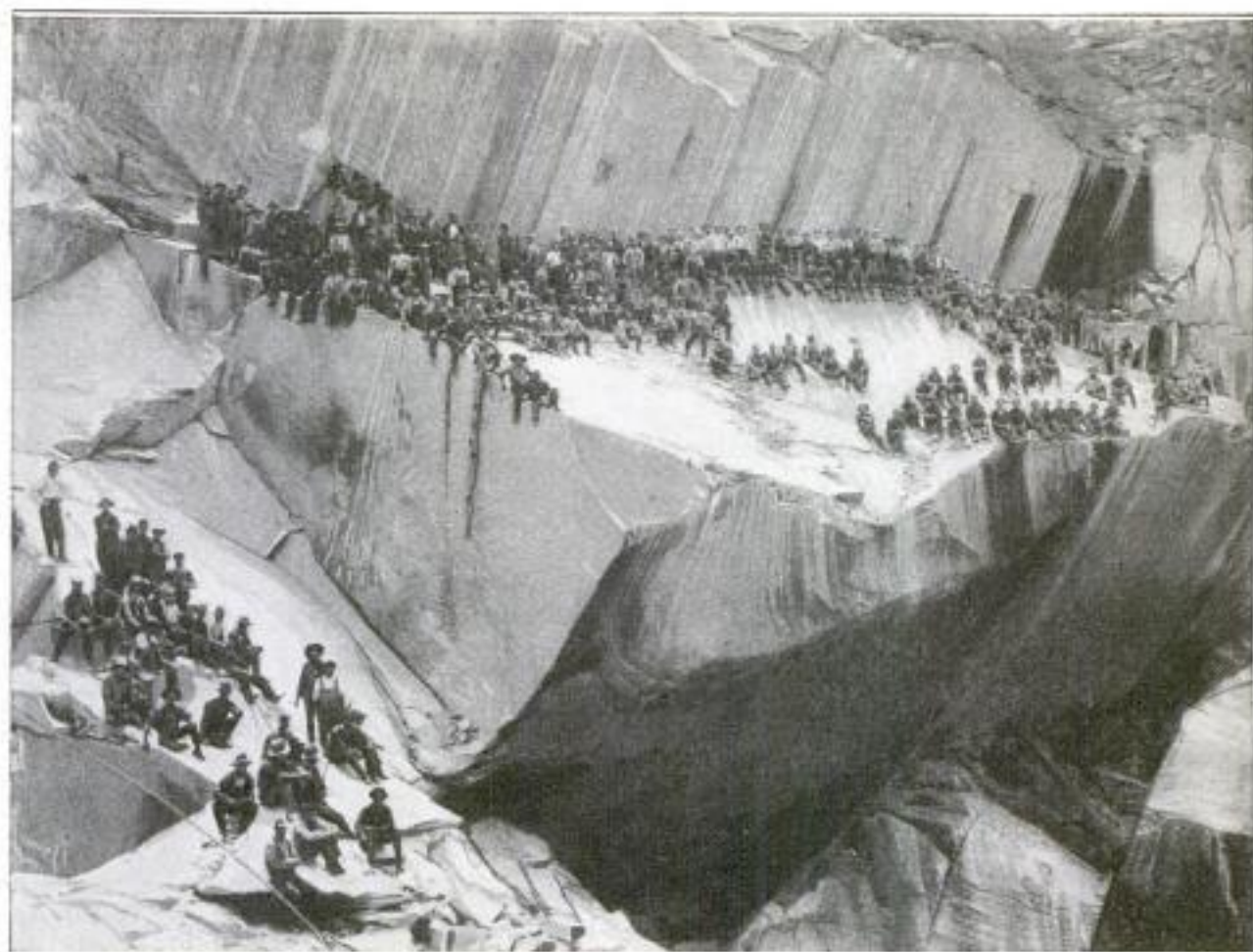
The Largest Block of Granite Ever Quarried in One Piece—Large Enough to Accommodate on Its Upper Surface the Crowd of More Than 300 Workmen Shown in the Picture. Subsequently, the Huge Block was Worked into Smaller Blocks Suitable for Monuments
