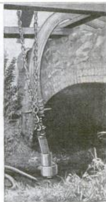
Above: The Old Fire Engine, Quite a Relic of the Past as Compared with Modern Fire-Fighting Machines, Is at Work Proving That It Still Has Vitality Enough to Pump All the Water Needed for Road-Building Purposes. Right: Hanging Over the Bridge with Its Nozzle in the Water Is the Hose through Which the Veteran Fire Engine is Pumping the Water
