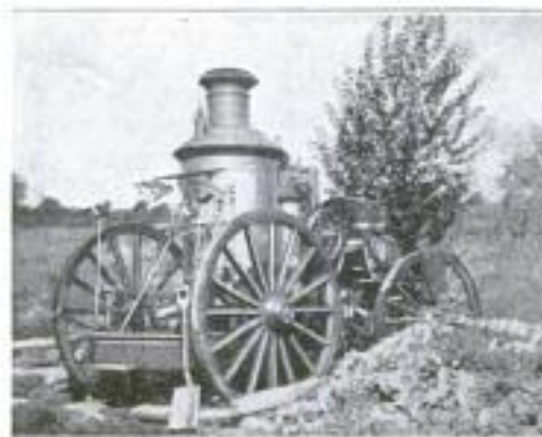
Above: The Old Fire Engine, Quite a Relic of the Past as Compared with Modern Fire-Fighting Machines, Is at Work Proving That It Still Has Vitality Enough to Pump All the Water Needed for Road-Building Purposes. Right: Hanging Over the Bridge with Its Nozzle in the Water Is the Hose through Which the Veteran Fire Engine is Pumping the Water
