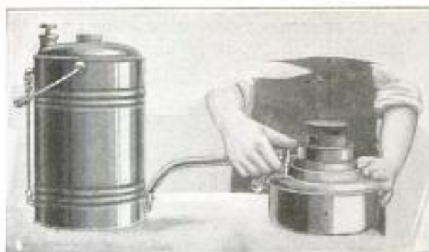
This Fountain Oil Can was Designed with a View to Safety in the Transfer of Oil from the Receptacle to the Reservoir of Some Other Device. Pressing the Trigger Releases the Oil in a Quick Stream
