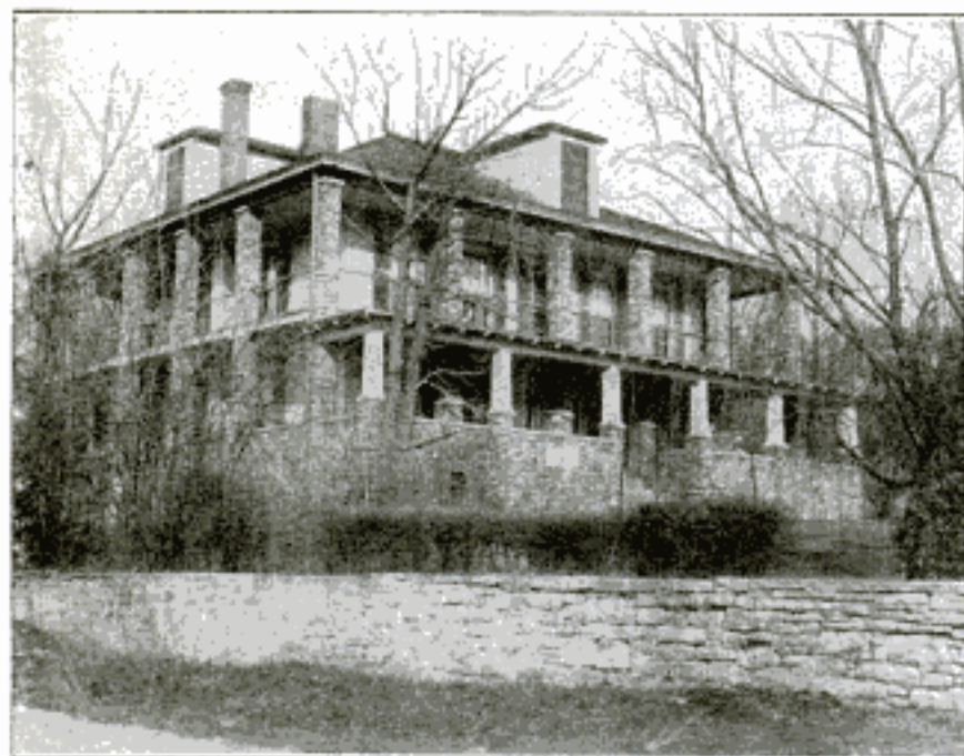
The Rocks and Gravel Used in the Construction of the Veranda and Columns of This Home in Milford, Ohio, were Secured by the Owner from a Near-By Stream, Thus Effecting a Partial Solution to the Problem of Building-Material Costs
