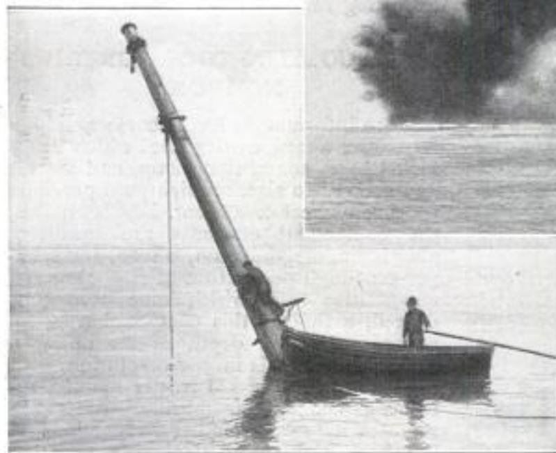
In Preparing the Wreck for Destruction, the Final Act Was to Connect the Firing Cable to the Top of the Mainmast Which Was Above Water, as Shown in the Illustration, Where the Men are Preparing to Leave the Finished Job
