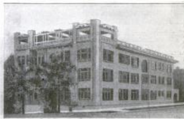
Unusual Roof-Garden Effect Formed by Extending the Concrete Columns One Story Above the Front of the House: Cross Trellises Heighten the Garden Effect
