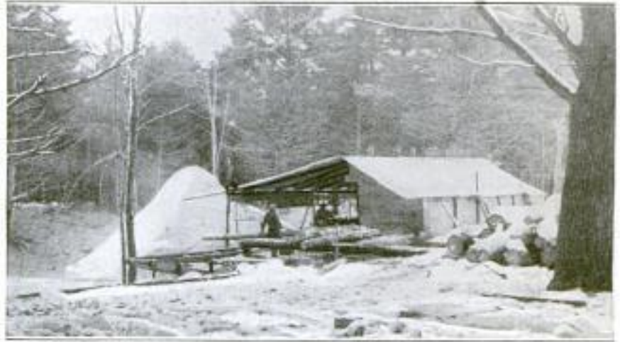
In the Depths of a Forest, Where Wood Fuel Abounds, This Sawmill is Electrically Driven. It is Said to Be the First of Its Kind to Change from Steam to Electricity
