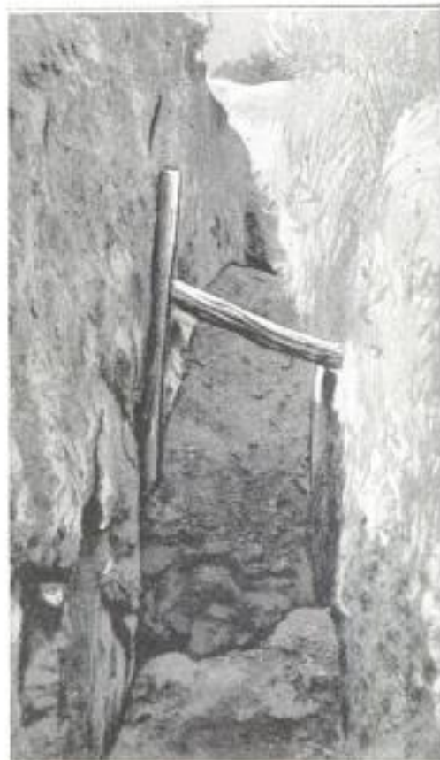
One of the Trenches Dug by the Discoverers of the First Mine: It Runs Laterally to the Fissure That Contains the Ore, and is Braced with the Limbs of Trees
