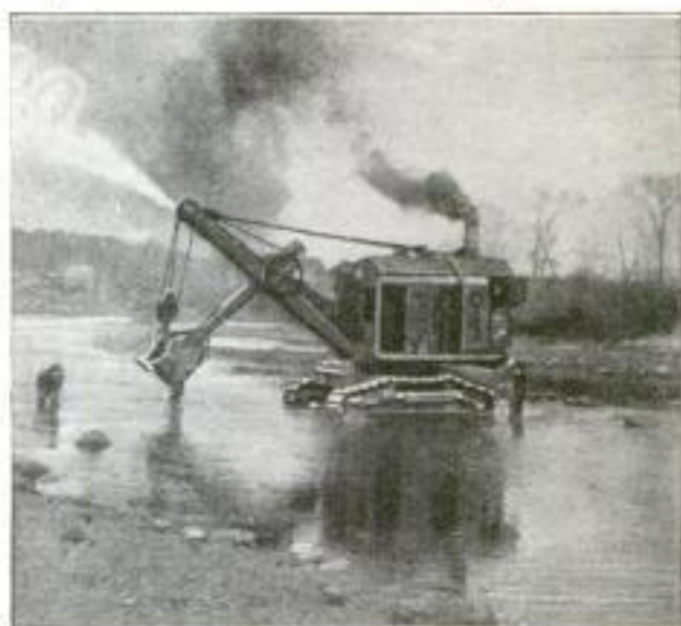
The Steam Excavator is Forging the Mississippi River on Its Tractor-Tread Wheels Just as it Travels on a Dry Road. With its Excavating Bucket It Clears the Way Ahead of It
