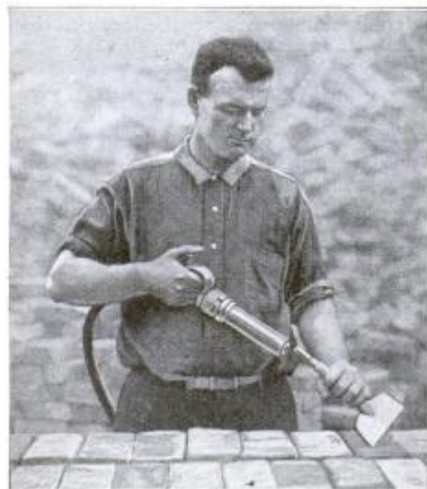
An Ordinary Pneumatic Hammer with a Broad-Faced Chisel Connection for Cleaning Mortar from Bricks
