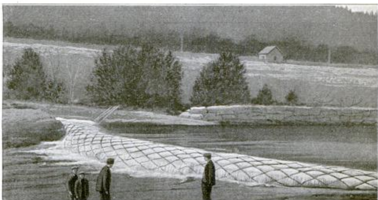
Showing the Completed Dam and the Water Backed Up behind It After the Water-Filled Canvas Hose has Been in Position for Some Days: The Tube is Protected by Rope Netting
