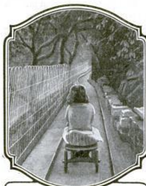
The Grade of This "Kiddie Ride" in a San Francisco Park Is Steep Enough to Insure a Good Start, with a Gradual Reduction to Guard against Accidents
