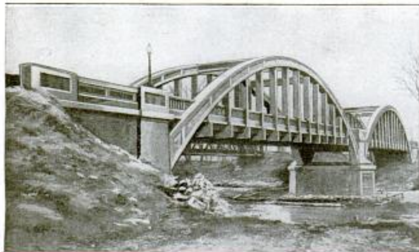
A Departure in Concrete-Bridge Construction: The Weight is Suspended from the Arches Instead of Resting upon Their Tops as in the Conventional Design
