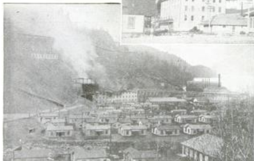
A View Taken Immediately after the Fire. While the Lower Part was Still Burning, That Shows the Great Gap in the Plant Made by the Fire
