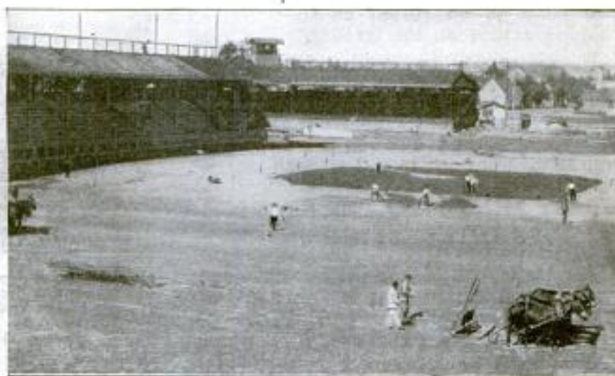
Moving the Grassy Infield: The Sod was Cut into Strips of Equal Width and Thickness and Transferred to the New Site; the Park Was Then Complete in the New Place
