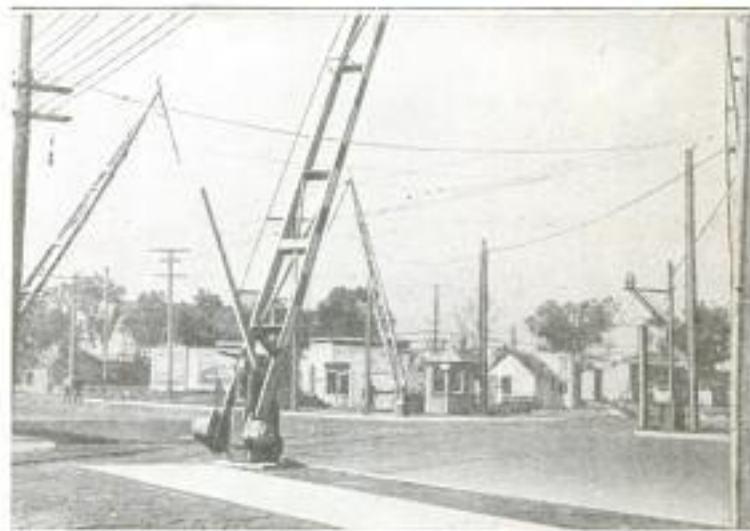
Crossing Gates, Wigwag Signals, Electric Gongs, Signs, and a Crossing Tender Combine to Protect This Crossing
