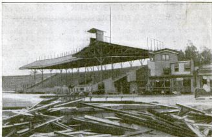
In Moving the Los Angeles Ball Park, the Grandstand and Bleachers were Shifted in Sections to Foundations Previously Prepared. The View Above Shows the Main Grandstand Section on Its Way to the New Location, 200 Feet Away. The Picture on the Left Shows One Section as It Appeared When Placed on Jacks for Moving. In the Background are the Remaining Sections. The Method of Reinforcing the Sections with Heavy Timbers is Shown in the Picture Below
