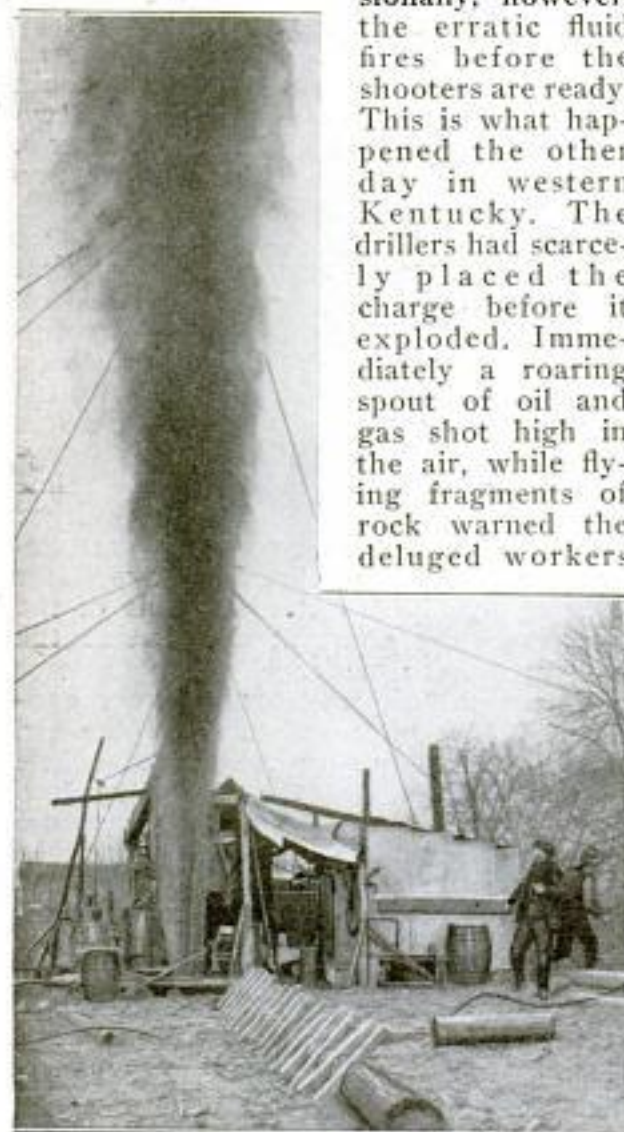
Oil Spout Started by a Premature Explosion of Nitroglycerin Used to "Shoot" the Well: The Workers are Running for Cover from the Flying Rocks
