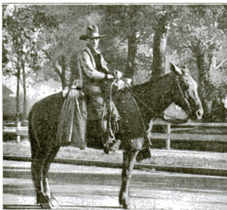
Chief White Eagle and His Faithful Mount, "Red Bird": It Is Quite Likely That They Know Nearly as Much about the Custer Battlefield Hiway as the Engineers in Charge of Its Construction, Having Traveled 900 Miles of Its Length
