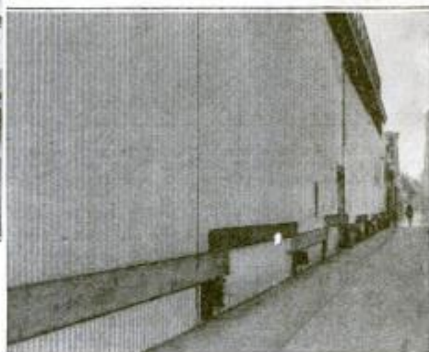
In Moving the Los Angeles Ball Park, the Grandstand and Bleachers were Shifted in Sections to Foundations Previously Prepared. The View Above Shows the Main Grandstand Section on Its Way to the New Location, 200 Feet Away. The Picture on the Left Shows One Section as It Appeared When Placed on Jacks for Moving. In the Background are the Remaining Sections. The Method of Reinforcing the Sections with Heavy Timbers is Shown in the Picture Below
