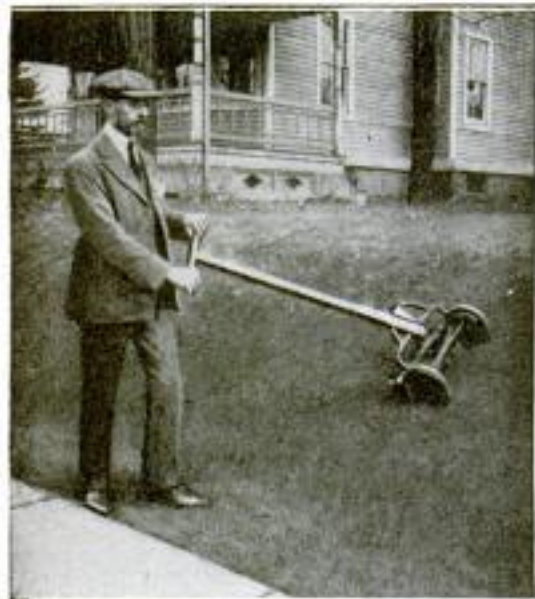
A Swivel Arrangement in the Handle Fitting of the Terrace Lawn Mower Allows the Operator to Walk on the Ground and Mow the Incline
