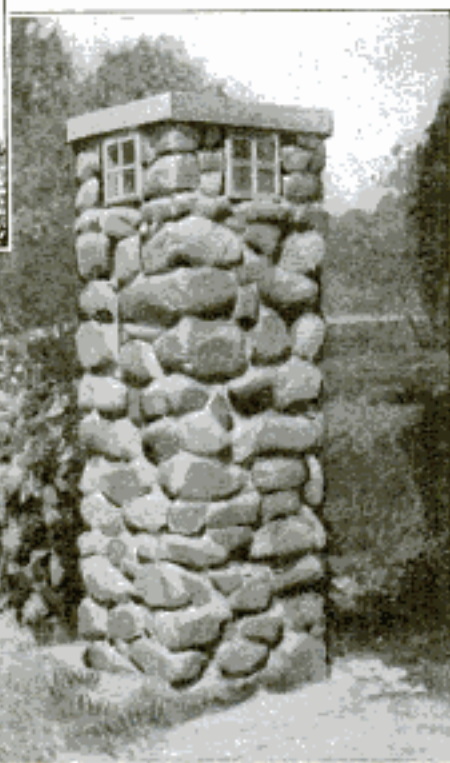
An Electrically Illuminated Gatepost of Concrete and Field Stone Provides an Attractive and Substantial Entrance to Public or Residential Premises
