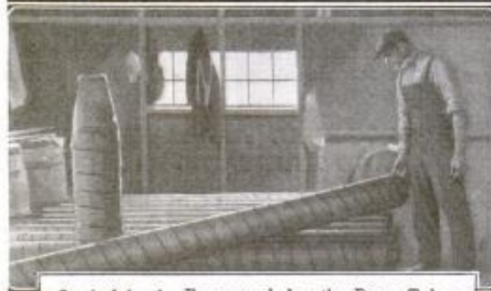
Stacked in the Foreground Are the Paper Tubes, Ready for Spraying with Concrete. Standing at the Left Is a Framework for One of the Solid Points Used on Each Pile
