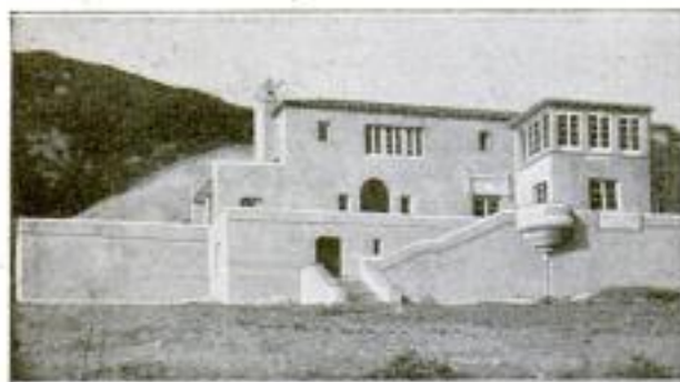
The Home and the High Concrete Wall Are Suggestive of an Old Fort
