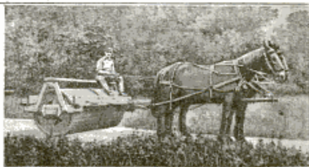
Good Roads Are Not a Luxury, but an Economic Necessity. The Roller Shown will Help to Make and Maintain Good Roads in the Rural Community
