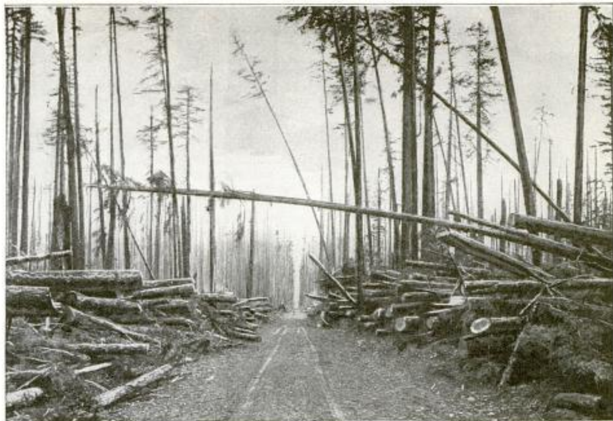
A Region of Smaller Timber, Where the Road has been Opened by Sawing through Actual Thousands of Sticks of the Average Size of Telephone Poles, a Herculean Task That was Performed with Remarkable Speed
