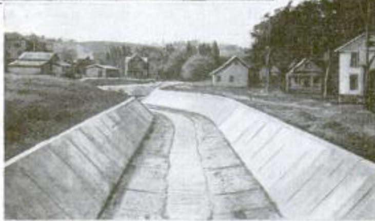
The Channel of the Creek Completely Lined with Concrete, with a Top Width of 48 Feet inside the Walls: Expansion Joints are Placed Every 30 Feet
