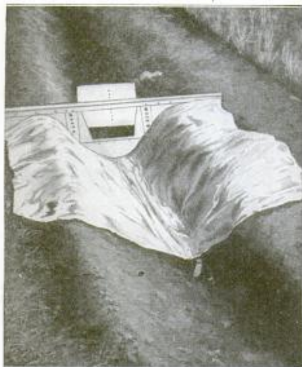
The Portable Irrigation Dam is Fastened Lengthwise in the Ditch. It Has the Additional Advantage of Being a Measuring Weir
