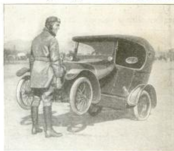
The Tiny Car Has Standard Lines but Is So Small and Light That One Man can Lift Either End. The Fenders and Headlights Swing with the Front Wheels
