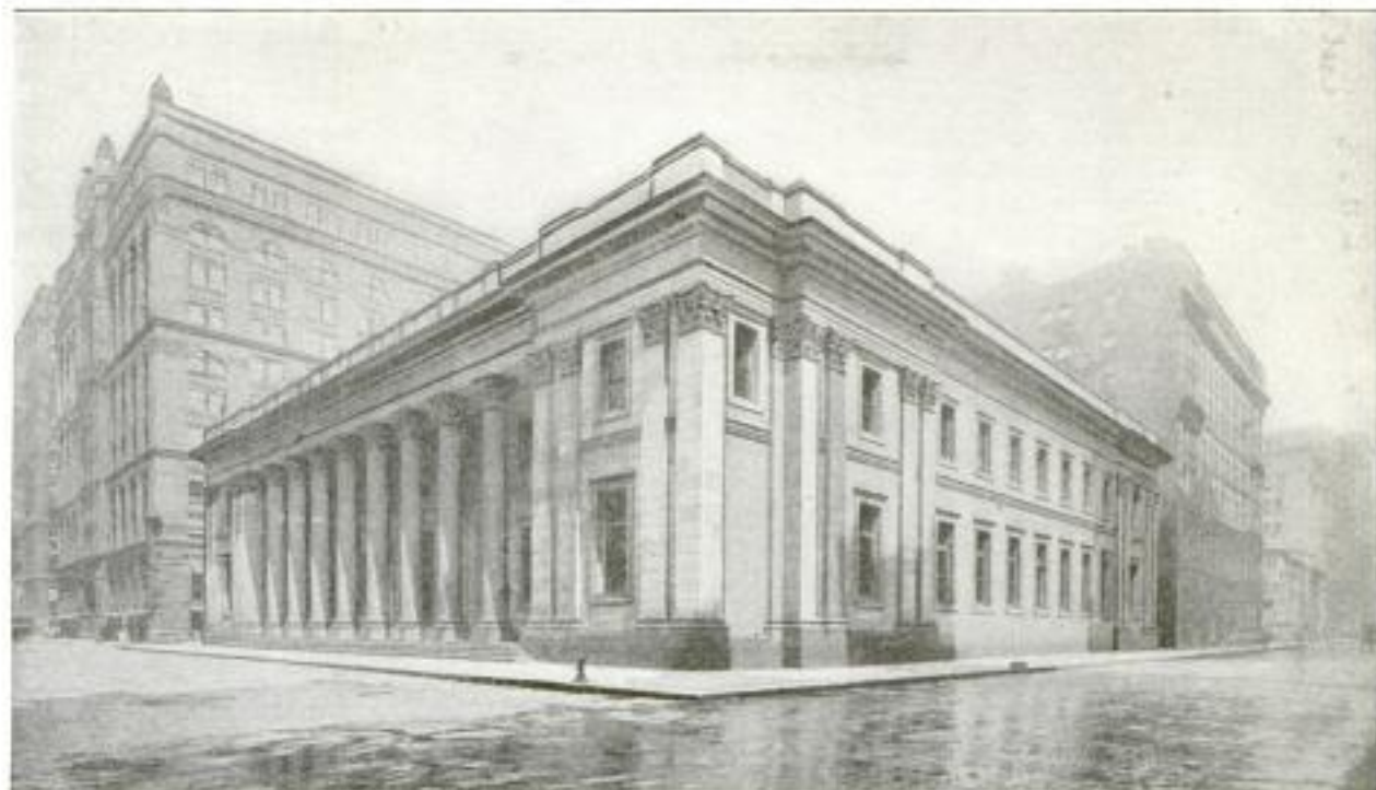
The Big Chicago Bank Building, Built of Steel and Granite, Which It is Proposed to Sell for Dismantling and Removal to Some Other City, There to be Rebuilt at a Fraction of a New Building's Cost
