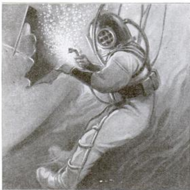
The Acetylene Torch, with Its Improvised Guard Cup, being Used under Water for Emergency Repairs to a Sinking Ship
