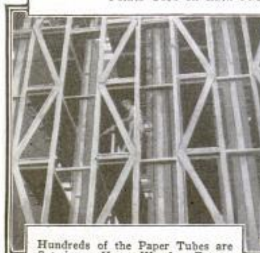
Stacked in the Foreground Are the Paper Tubes, Ready for Spraying with Concrete. Standing at the Left Is a Framework for One of the Solid Points Used on Each Pile
