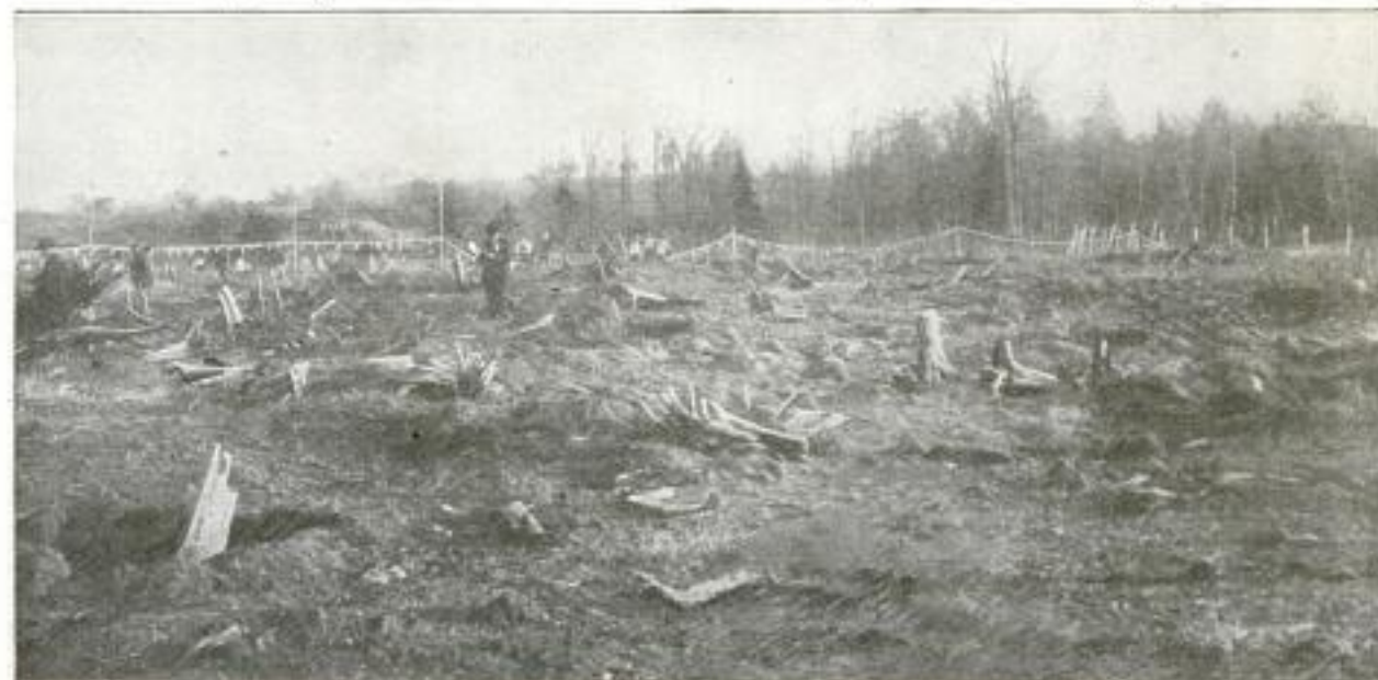
After the Blast: The Photo Shows the Remains of Stumps Blown Out at a Single Blast from an Acre of Ground near Wausaukee. The Big Blast Was the Closing Celebration of the Clearing Job
