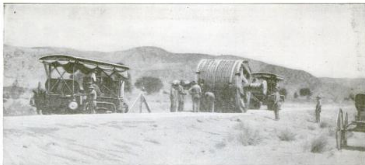
Hauling 70-Ton Electric-Generator Rotors Over Ten Miles of Mountain Road by Tractor: The Rotors were Lagged with Wood to Nearly 10 Feet in Diameter, and Rolled Along by Cables Wrapped around Them
