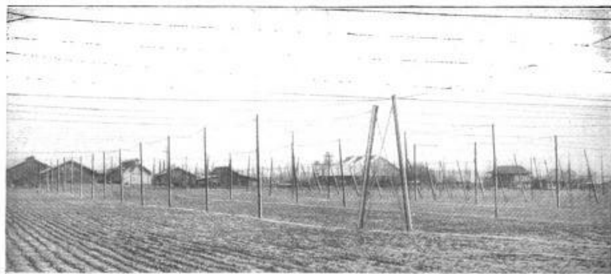
The Trellis System Used for Growing Hops in the Fields of California: The Vines, Trained on These Structures, Grow 15 to 18 Feet Long, with Heavy Clusters of Leaves; and a Stout Support Is Necessary
