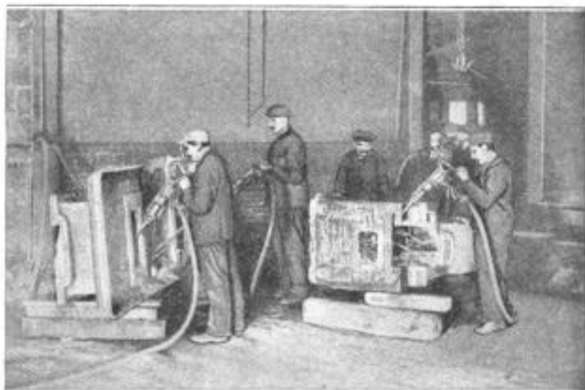
Foundrymen Using the New Compressed-Air Tool for Breaking Up Cores in Castings, One Operator Doing Work Formerly Requiring Two Men with Hand Bars and Hammers
