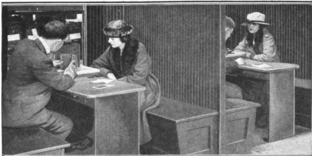
Inspection Booths Where Customers are Shown the Insides of Their Batteries and Defects are Pointed Out by the Rubber-Gloved Salesman: The Battery Covers are Steamed Off in the Room Just Beyond, and the Cells Brought In, after Which the Communicating Window, Seen Open, is Closed to Exclude Fumes
