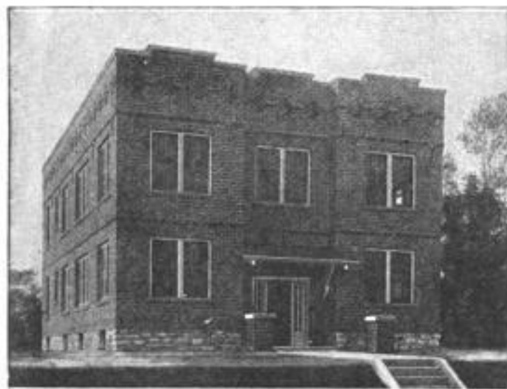
Front View of the Modern Four-Flat Building That Promises Good Future Returns Even on Present Costs
