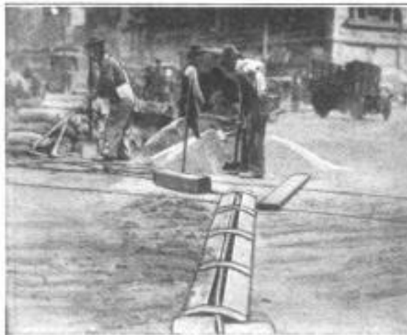
The Hose, Crossing the Street under a Metal Shield, is Protected from Injury without Hampering Traffic
