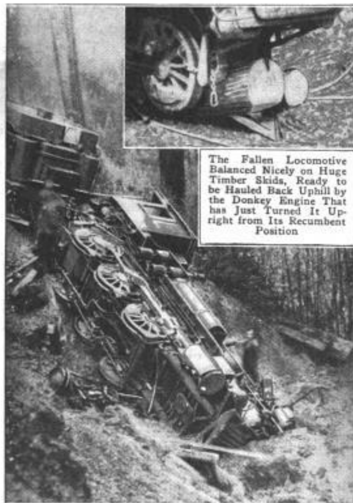
A Discouraging Problem: The Locomotive on Its Side on the River Bank, after a 20-Foot Downhill Plunge, and No Wrecking Crane Available
