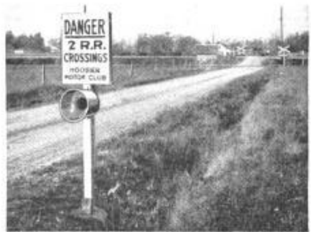
A Novel Railway-Crossing Warning: At Night the Reflector Returns the Light from Auto Headlamps in a Bright, Red Beam
