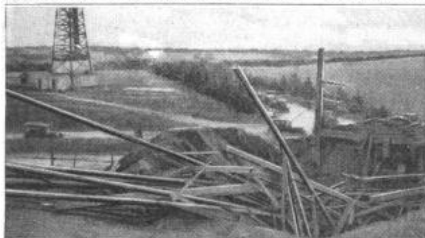
The Shattered Remnants of the Derrick, Partly Buried in the Chasm Created by the Sudden Blow-Out of Gas
