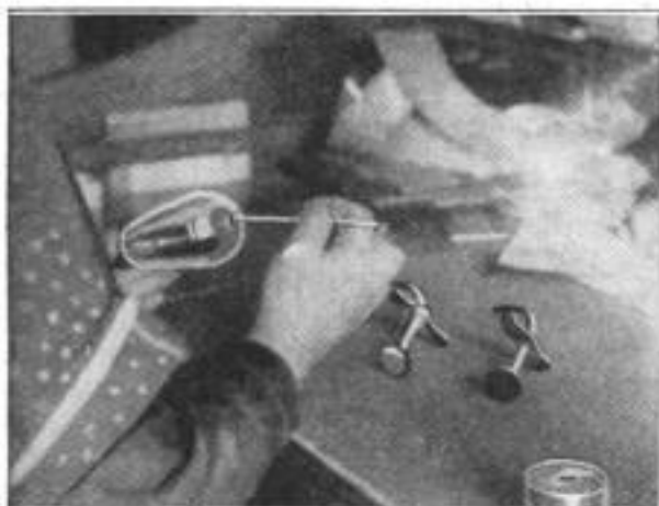
Left: Cleaning Out the Old, Burned-Out Tungsten Wire through the Reamed Hole in the Tip, Preparatory to Relacing with New Wire. Right: The Reaming Table, Where, after Warming the Glass, the Tip is Removed, and the Opening Enlarged to a Half Inch
