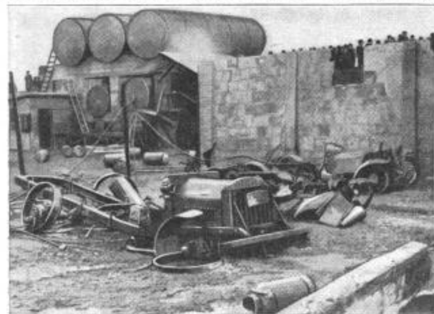
Interior of the Plant after the Explosion: Autos and Trucks Parked Inside were almost Dismembered, Becoming Mere Masses of Scrap, While the Plant Itself Was Wrecked
