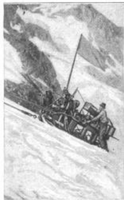
Left: The Mine-Drill Power Plant Pulling Itself up the Face of the Glacier by Means of a Cable. Right: The Shaft, 30 Feet in Depth. Later a 50-Foot Shaft was Sunk through the Solid Ice and Snow
