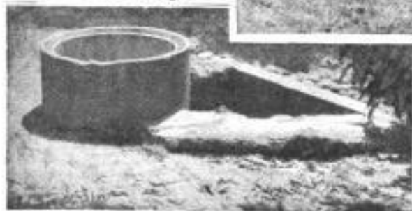
The Water Enters the Round Pipe and Overflows into the Triangular Trough
