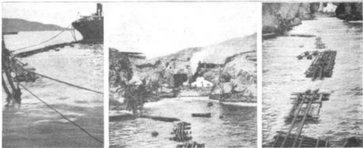
Left: A Tank Ship Discharging Oil into the Floating Pipe Line. Center: The Shore End, Where the Oil is Pumped into Tanks. Right: The Six-Inch Steel Pipes, Mounted in Pairs on Rafts, and Connected Together, and with the Ship and Shore Lines, by Rubber Hose
