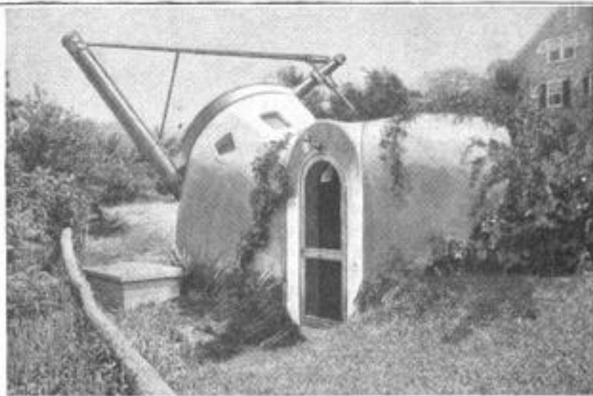
View of the Inventor's Observatory from the Entrance Door, opposite the Turret: The Structure Also is Entered through a Tunnel from the House, and Contains a Comfortable Office besides the Observation Room
