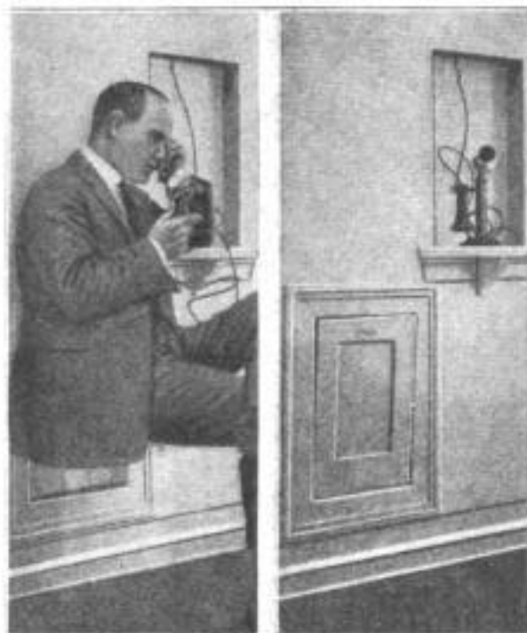
Left: The Folding Telephone Seat in Use. Right: Seat Folded into Its Recess. The Instrument may be Concealed by Drapery
