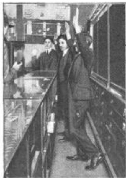
Left: The Store Clerk, in a Demonstration Holdup, is Pressing the Contact Board with His Heel. Right: The Sign That Appeals for Help
