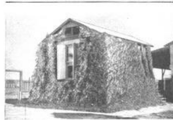
Office Covered with Morning-Glory Vines, Whose Moist Leaves Keep the Interior Cool on the Hottest Days
