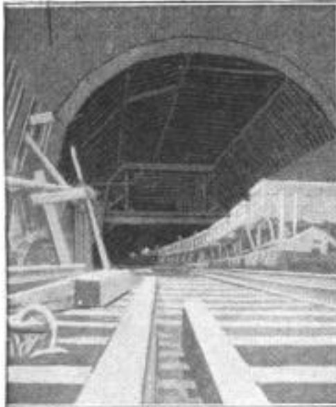
Two Views of Pittsburgh's New $3,000,000 Tunnel. Left: The Finished Bore of the Vehicle and Pedestrian Tube. Above: Almost Ready for Concreting. The Smaller Tube Is for Street Cars Only. The Larger will Accommodate All Other Traffic
