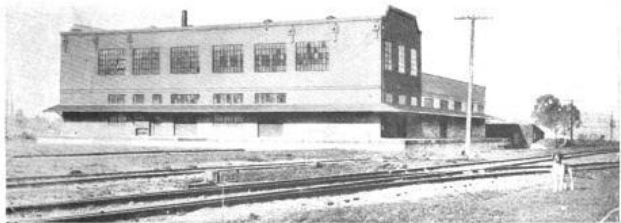
The Growing Importance of Fruit and Vegetable Dehydration as an Industry is Indicated by California's New Concrete Plant, the First of a Series. Automatic Machinery for Peeling, Slicing, and Handling Makes It Unnecessary for the Workers to Touch the Product at Any Stage
