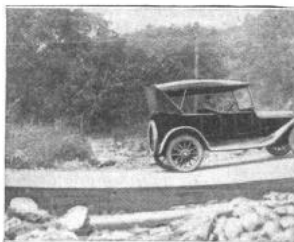
The Bed of the "Dry Run" is Paved with Cement. This Stops the Damage and Also Makes a Smooth Road
