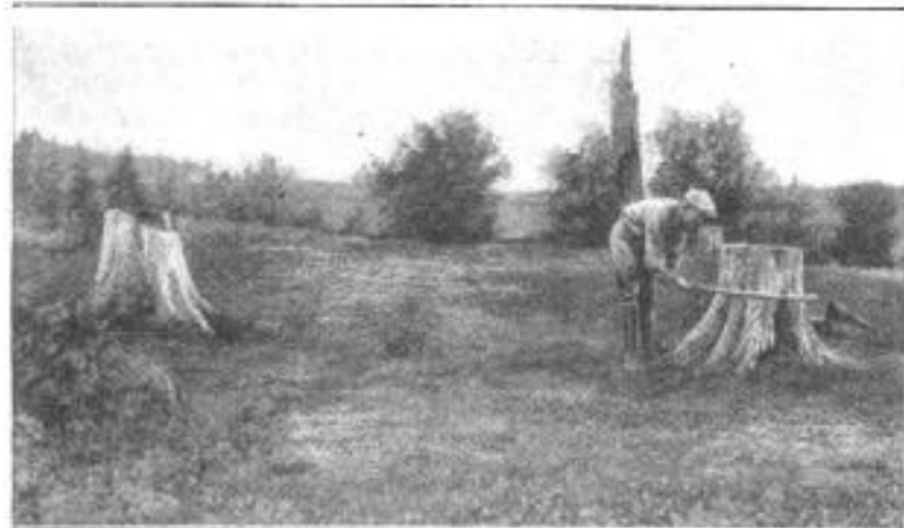
The Blaster Measures Each Stump with a Tree Caliper, and Then Computes the Proper Charge of T. N. T. Required for Its Destruction
