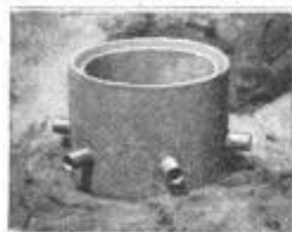
Form of Irrigation Outlet, with Six Small Pipes to Distribute the Water over a Field. Right: The Water Passes from the Square to the Round Trough
