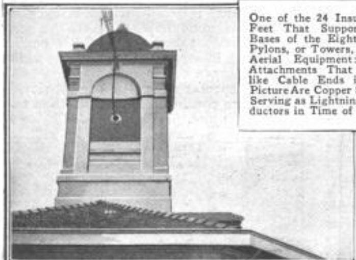
The Tower on Top of the Station's Main Building, Where the Leading-In Wires from the Antennae Enter: There Are 16 Parallel Aerials, Supported by Four Cross Wires on the Pylons, and from Them 10 Connecting Wires Go Down to an Insulating Support on the Tower, are Formed into a Cable, and Pass through a Conduit into the Station
