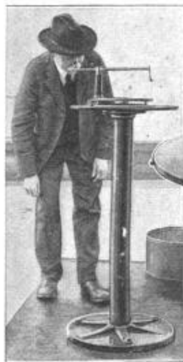
Left: A Weather Observer Using the New Form of Nephoscope to Gauge the Movements of Clouds, to Determine Upper-Air Currents for the Benefit of Flyers. Above: A Close-Up of the Instrument, Showing the Mirror, Straightedge, and Sighting Pedestal, with Tiny Peepholes in the Brackets at the Ends of the Horizontal Arm
