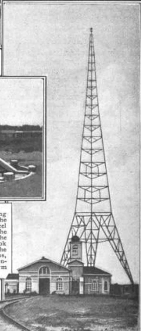
One of the Steel Aerial Masts, or Pylons, 820 Feet High, with a Three-Legged Base Supported by Insulating Feet, and Resembling the Eiffel Tower in General Outline: There Are Eight of These Huge Masts, in Two Rows, All Spaced About 1,300 Feet Apart, and Supporting the Four Cross Wires That Carry the Antennae
