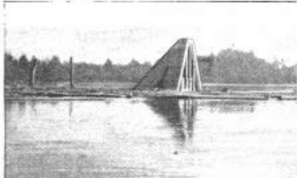
A New-Type Logging Pier, Used in the Rivers of the Logging Country, is Built of Concrete Instead of Logs and Rock, as were the Older Type
