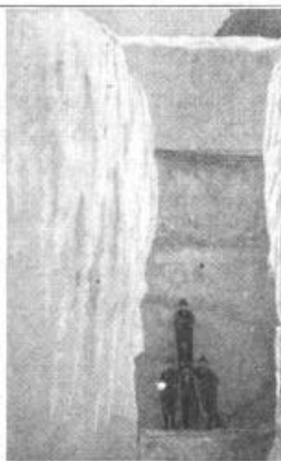
Left: The Mine-Drill Power Plant Pulling Itself up the Face of the Glacier by Means of a Cable. Right: The Shaft, 30 Feet in Depth. Later a 50-Foot Shaft was Sunk through the Solid Ice and Snow
