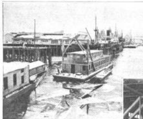
The Barge Repair Shop, in Mid-Harbor, on Its Way to a Mooring alongside a Vessel, Which It will Repair While Unloading Progresses Uninterruptedly
