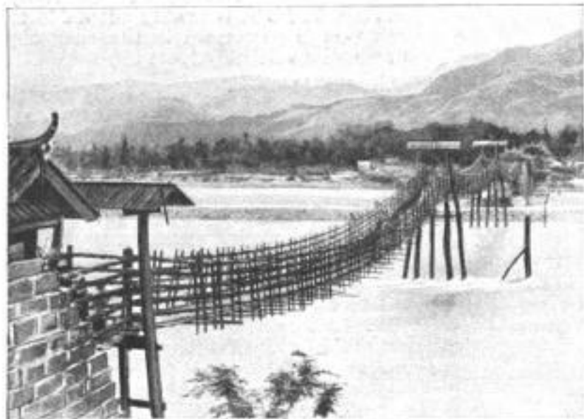
Bamboo and Wire Are the Structural Materials of This Ancient Suspension Bridge across the Min River in the Chinese Hinterland
