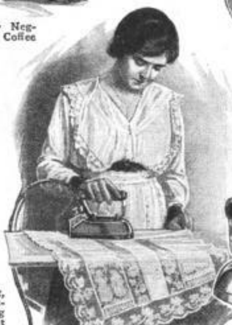
An Improved Electric Iron, Seen in Use on Delicate Work Above and in Detail at the Right, Contains a Thermostatic Control That Regulates the Temperature and Prevents Overheating
