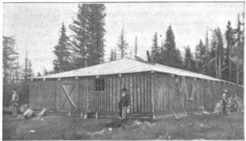
New-Style Lumber-Camp Cabin: The Logs are Set on End, the Chinks Plastered with Clay, and the Interior Walls Covered with Tar Paper
