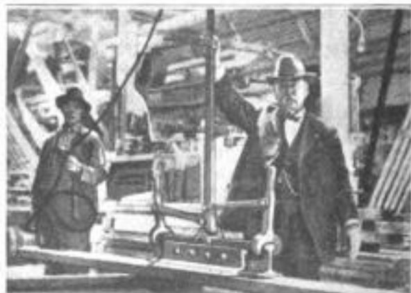
The Rail Ends are Brought Together at the Joint by Moving the Long Lever to the Left
