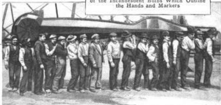
By Comparison, the Crew of 17 Conveys an Idea of the Length of the Minute Hand. It is Built Up of a Brass Framework, Covered by Sheet Copper, and, with Its Counterpoise, Tips the Scales at 640 Pounds
