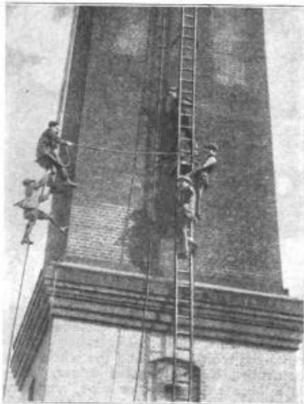
Steeplejacks in the Making: The Instructor, an Ex-Airman, is Demonstrating How to Ascend or Descend a Rope
