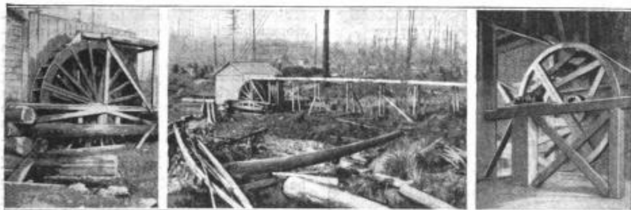
Left: The Homemade Overshot Water Wheel by Which a Tiny Creek is Made to Supply Power for Farm Lighting. Center: The Long Wooden Flume. Right: The Big Wooden Pulley Driving the Dynamo. The Plant Operates Continuously, Employing No Storage Battery
