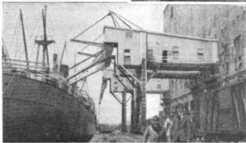
Loaded Grain Cars are Moved over the Grain Pits by the New Car Handler and the Load is Shoveled Out. From the Pits, the Grain is Elevated to Spouts Which Conduct It to the Ship's Hold
