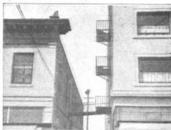
This Odd Bridge Fire Escape Is the Result of an Unusual Agreement between the Owners of the Two Buildings
