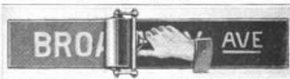
Street Signs are Quickly Brightened by Applying New Background Paint with a Composition Roller
