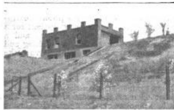
This Garage Gives the Chauffeur a Ground-Floor Residence. The Cars Occupy the Top Floor
