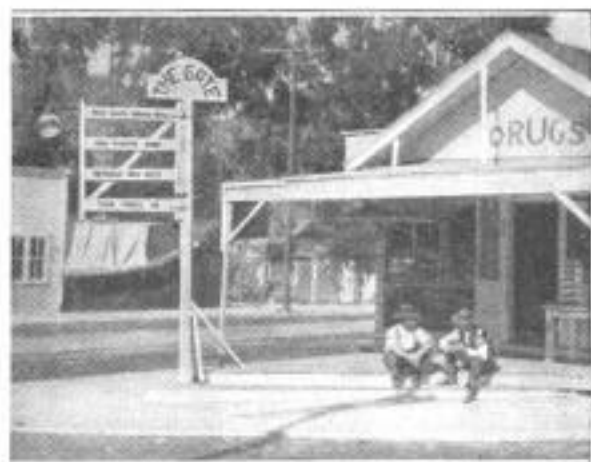
The Trade of This Store, Which is Located in a Pacific-Coast Village, is Increased by a Novel Swinging-Gate Advertising Sign
