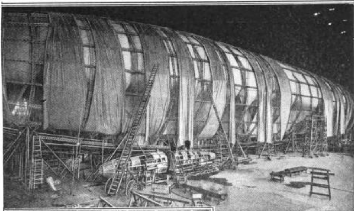
The Gas Containers Are 15 Ballonets Made of a New Exceptionally Light and Gas-Tight Material. This Illustration Shows the Inflation of the Containers While Undergoing Test. The Small Framework Is That of the Combination Navigator's Cabin and Main Engine Room
