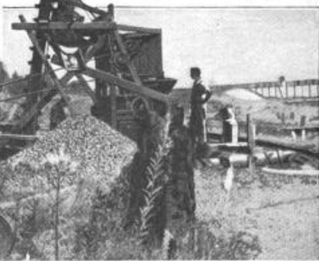
A Full-Fledged Mining Machine Set Up on the Site of a Former Rifle Range: It is Reclaiming Lead, Copper, and Nickel at the Rate of About 1,200 Pounds per Day from a Hillside That Formed the Back Stop to the Range. The Metal Is the Remains of Government Ammunition Expended in Training Our Fighting Men
