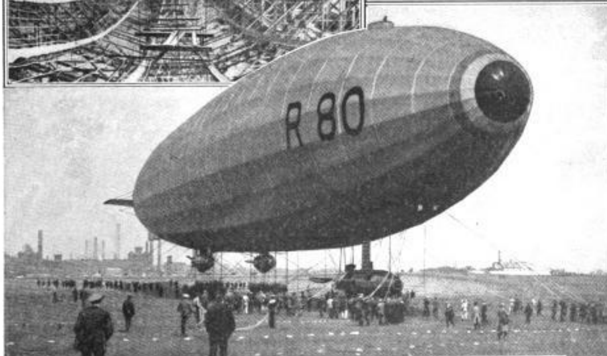
The "R-80" Undergoing Trial: A Gun Platform, on Top, Mounts One Two-Pounder and Six Lewis Machine Guns. All Cars are Provided with Buffers Which are Buoyant Enough to Support the Machine on Water. The Steering Cables and Rods are Inclosed by a Shaft Which Connects the Ship's Hull and the Forward Car
