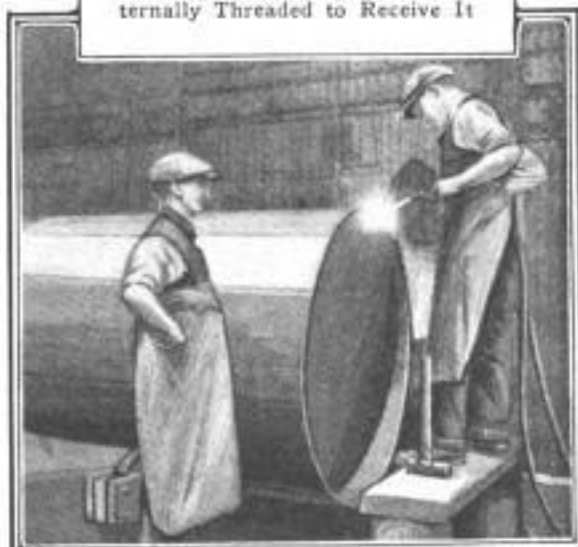
Arc-Welding a Head into a 1,000-Gallon Gasoline Tank: As in the Heading of Barrels, After the Heads are Pressed In, Thin Rings of Steel are Placed on Both Sides of Them. These, the Head Rims, and the Barrel Edges, are Fused into a Solid Mass by the Welding Arc
