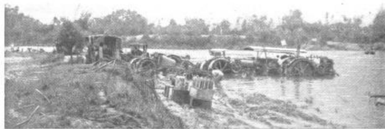
The Demonstration Tractors Gradually Emerging from the Flood That Caught Them Overnight in a Partly Plowed Field: After the Magnetos had been Dried, the Machines Returned to Town Unharmed
