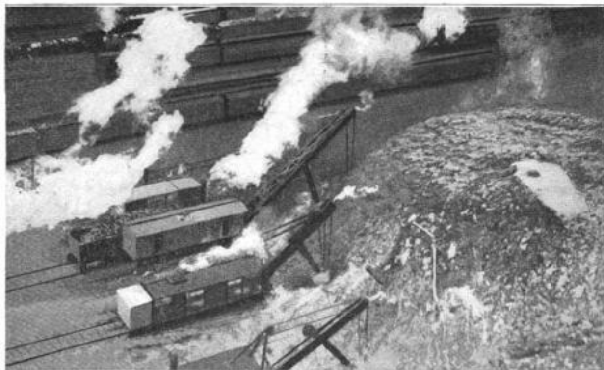
Big Steam Shovels of the Pennsylvania Railroad, Working to Uncover the Eight Tracks Buried under 40 Feet of Earth by the Huge Pittsburgh Slide, Which Issued from a Precipitous Hill
