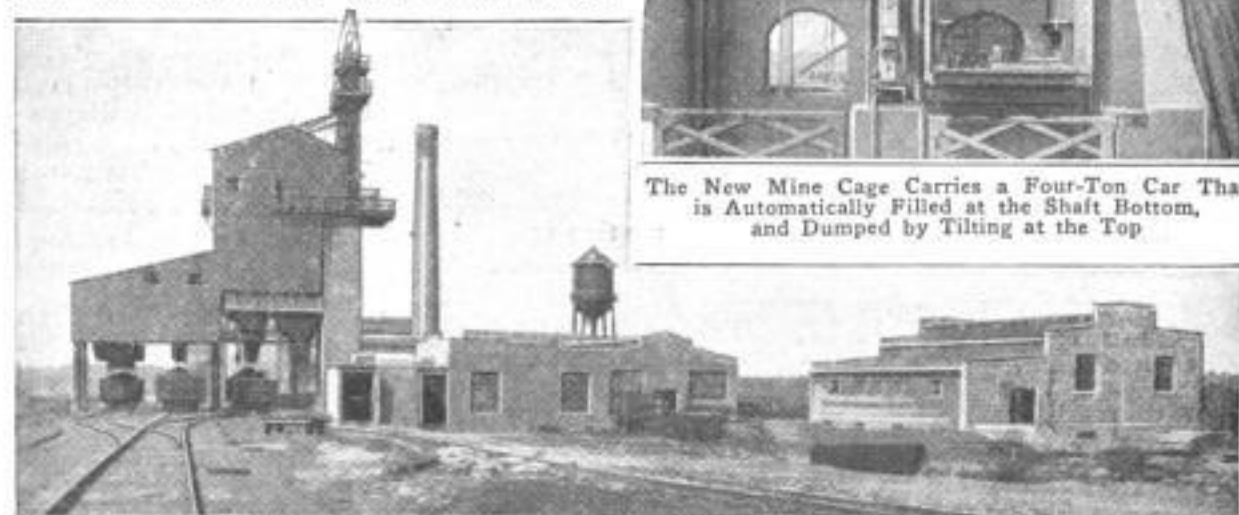
The $1,000,000 Equipment of an Ultramodern Coal Mine Now being Completed in Southern Illinois: Loading, Unloading, and Many Other Operations Are Automatic. A Bathhouse for 50 Miners Is at the Right
