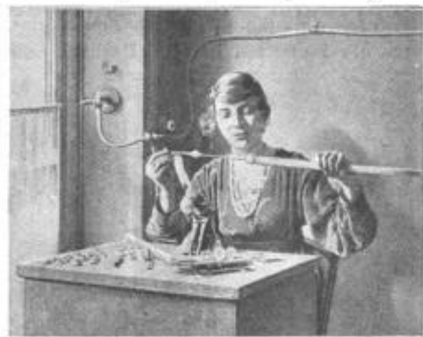
Transforming a Glass Tube into Artificial Eyes with a Gas Blowtorch, While the Customers Wait
