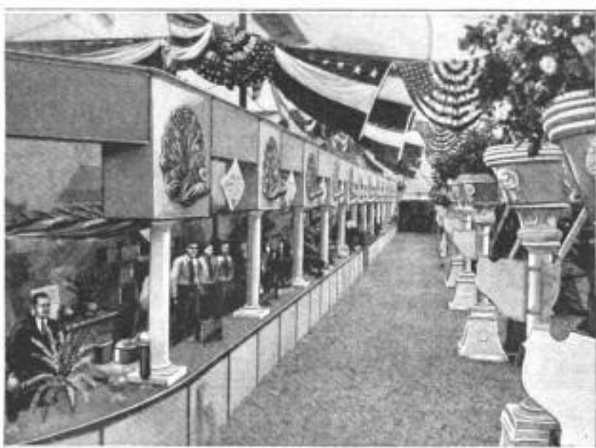
Above: Papier-Mâché Takes the Place of Composition Board in the Making of Light Panels, and of Plaster for Ornamental Pieces, Such as Urns, Vases, Artificial Flowers, Fancy Columns, Pedestals, and Capitals. Left: St. Gaudens' Famous Lincoln Reproduced in Papier-Mâché; Also Imitation Pipe-Organ Tubes Which Mask the Real Tubes Placed Behind
