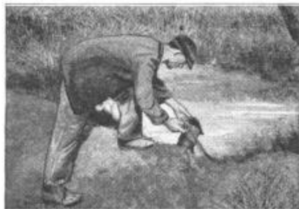
Closing One of the Outlet Pipes of an Irrigating System with a Lock Cover to Prevent Youngsters from Filling It with Rocks
