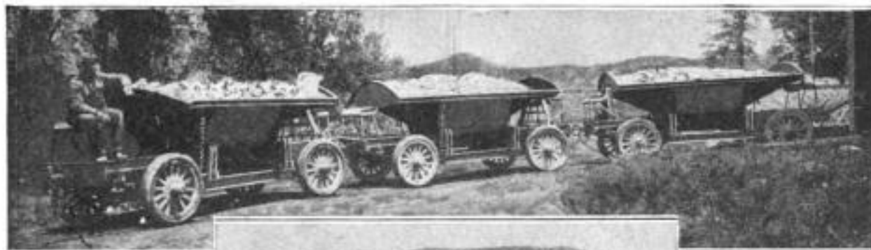
Left: The Low Side of the Trailer Facilitates Loading. This Construction is Made Possible by the Use of a Double-Drop-Frame Chassis. The High Ends of the Body Prevent the Spilling of Loose Materials
