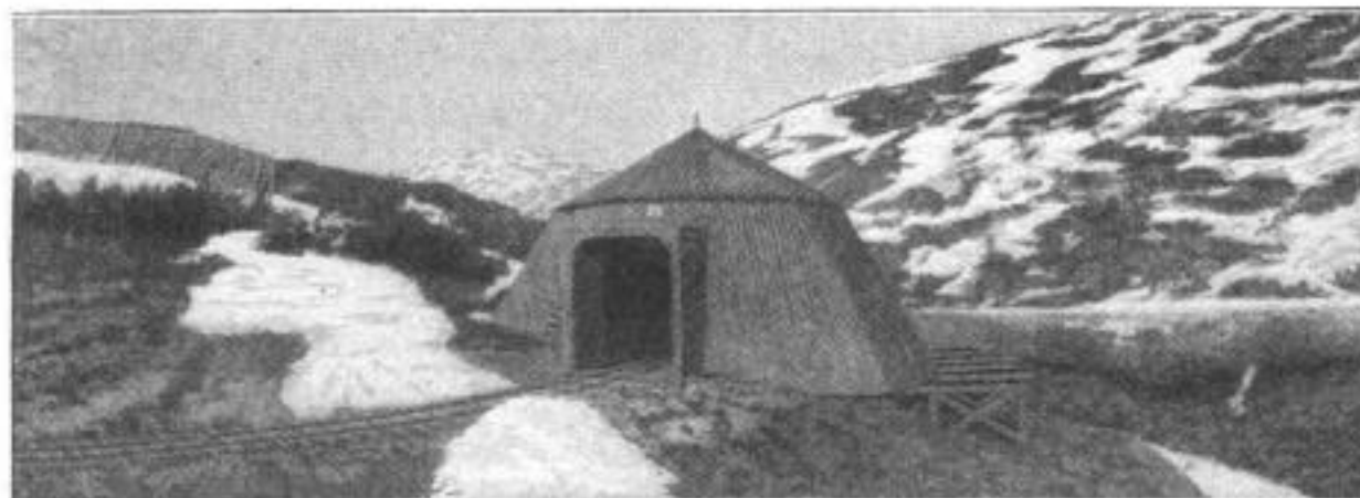
This Peculiarly Shaped Building Is a Snowshed Inclosing a Locomotive Turntable. In the Left Background is Seen One of the Snow Fences Which Line the Right of Way and Serve to Break the Full Force of the Drifts
