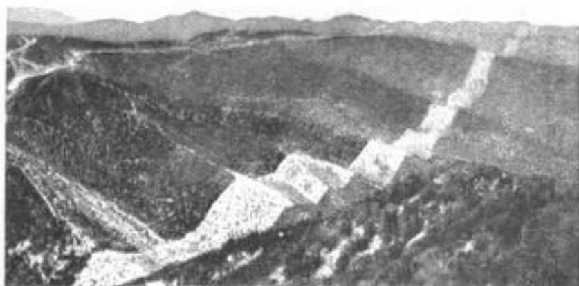
The Broad, Barren Streak of the Firebreak, 125 Feet Wide and 65 Miles Long, Makes a Conspicuous Mark against the Forested Mountain Sides
