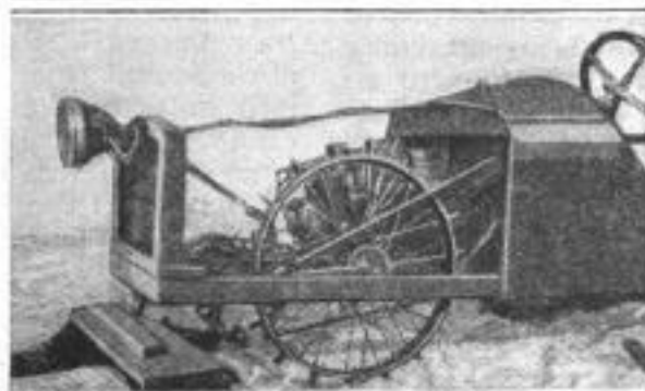
Built along the Lines of a Light Automobile or Cyclecar. This Machine is Driven by a Twin-Cylinder Motor. A Toothed Wheel, Which Adjusts Itself to the Surface Irregularities, Is the Propeller in This Type
