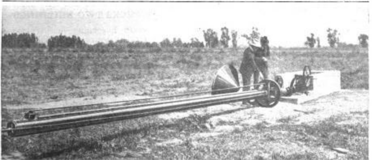
The Steel Mast is Folded in a Horizontal Position by Turning the Hand Winch Mounted on the Concrete Base, and a Counterweight within the Base Makes It Just as Easy to Raise It to the Vertical
