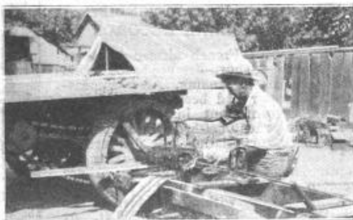
A Silo Contractor Threads the Scores of Iron Rods Needed for a Concrete-Stave Silo by Jacking Up His Truck and Attaching a Thread-Cutting Die to the Wheel
