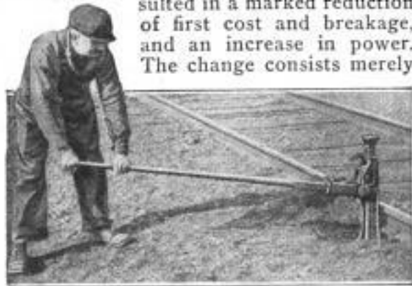
Using a Standard Steel Lining Bar as a Handle for a Square-Socket Railroad Track Jack
