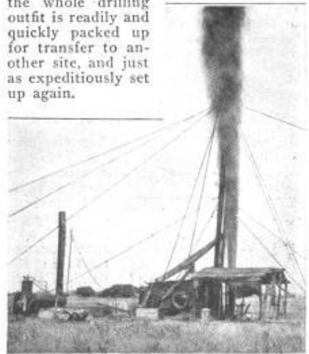
A Boom of Timber and a Winding Drum That can be Reversed with a Clutch, Make Up This Simple Drilling Outfit for Shallow Oil Fields. It is Easily Dismantled for Moving
