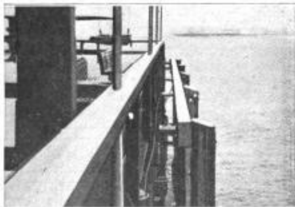
An Effective Pier Shock Absorber: The Auxiliary Piling Breaks the Force of the Waves. The Partially Absorbed Impact is Further Dissipated by Large Spiral Springs Which Also Have the Effect of Distributing It over a Wide Area
