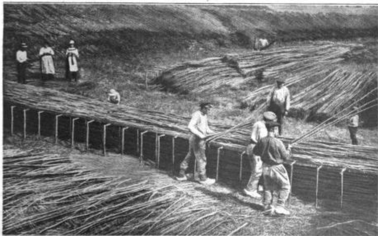
Enormous Mats are Prepared by Tying Branches of Trees into Bundles and These into Larger and Still Larger Bundles. The Mats are Used as the First Stage of the Foundation of the Dike Damming the Zuyder Zee
