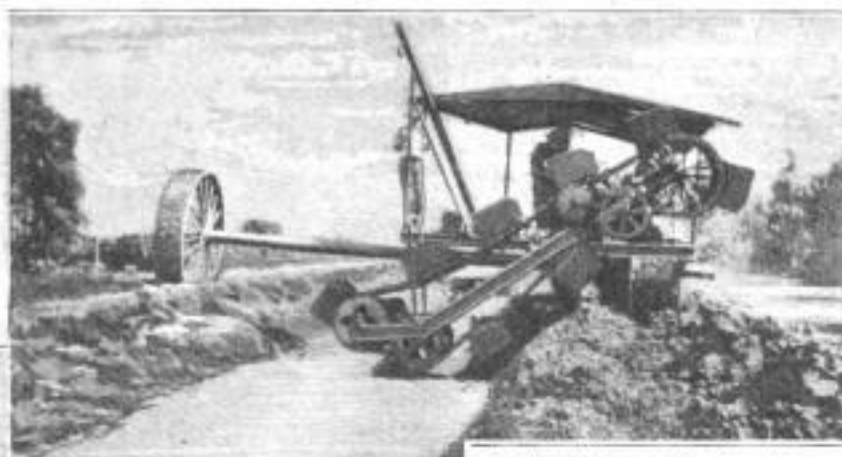
In This View of the Machine are Seen the Buckets and, at the Right, the Silt Brought from the Ditch Bottom. The Wheel has been Extended About 14 Feet
