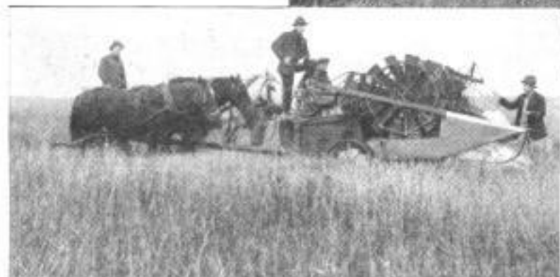
Above: Front View of the Machine That Threshes Sweet-Clover Seed in the Field, Indicating the Method of Bending the Plants into the Beater Wheel without Cutting Them. Right: Rear View, Showing That the Four Horses Push, Instead of Pull. This Curious Implement. Below: The Thresher Seen from the Side, as It Appears in Action, Threshing Sweet-Clover Seed over About 15 Acres a Day
