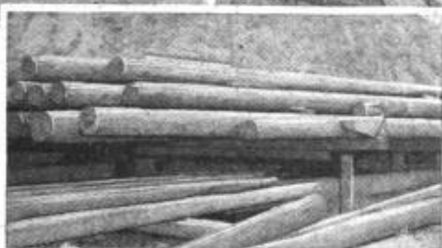
A Stack of the Old Piling Just Removed from the Water: In Spite of Their 28 Years of Submarine Service, They Are as Good as New, and Ready for Use in Building the New Pier
