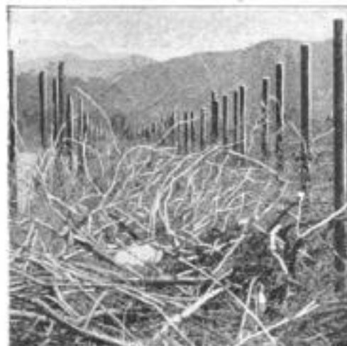
By Constructing Many Miles of Double Wire Fence on Each Side of a Stream, an Effective System of Flood Control has been Devised to Meet the Requirements of Conditions in Southern California
