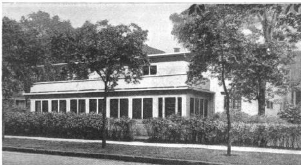
View Approaching the House from the Center of Its Block: The Long Glassed Porch Is Very Much in Evidence, and the Height of the Wall around Its Roof Makes the Latter a Safe Balcony-Playground. Behind the Porch Roof, the Gallerylike Second Story Is Visible
