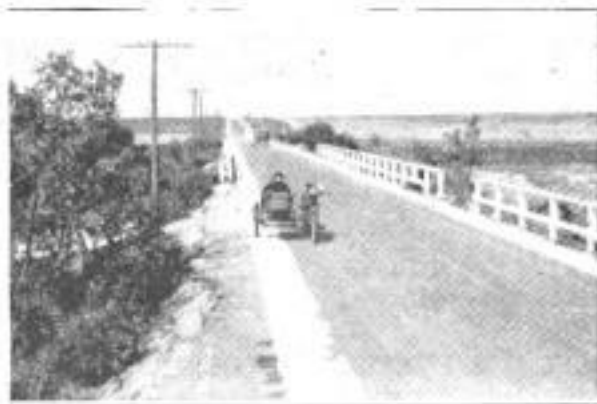
The Concrete Strips Keep the Surface from Spreading, and Help the Motorist to Keep to the Road at Night
