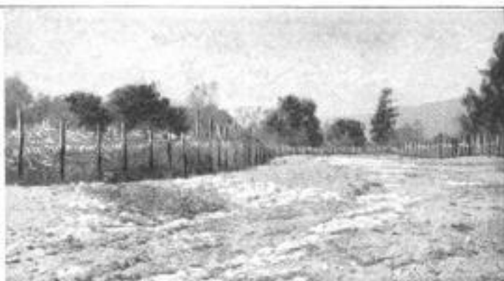
By Constructing Many Miles of Double Wire Fence on Each Side of a Stream, an Effective System of Flood Control has been Devised to Meet the Requirements of Conditions in Southern California
