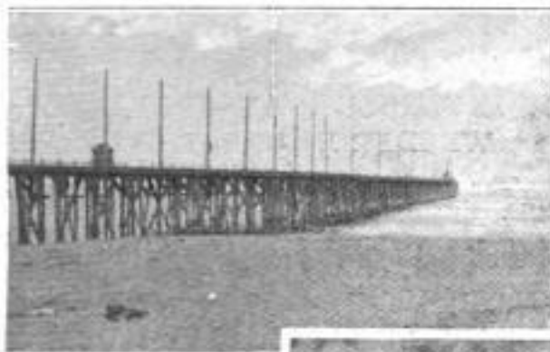
The Long Pier from Which the 28-Year-Old Piling was Removed and Found to Be Still in Good Condition
