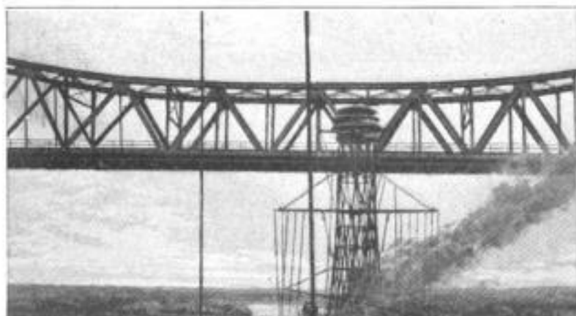
One of the Bridges across the Kiel Canal, That Smashed the Ship's Antenna Masts, Because It was Answering a Hurried Call for Help and Had No Time to Lower Them
