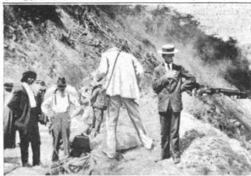
A Landslide of Considerable Magnitude Covered the Tracks of a Costa Rican Railway. Just Missing the Passenger Train Shown in the Background. The Tracks are Buried under the Débris Shown in the Foreground
