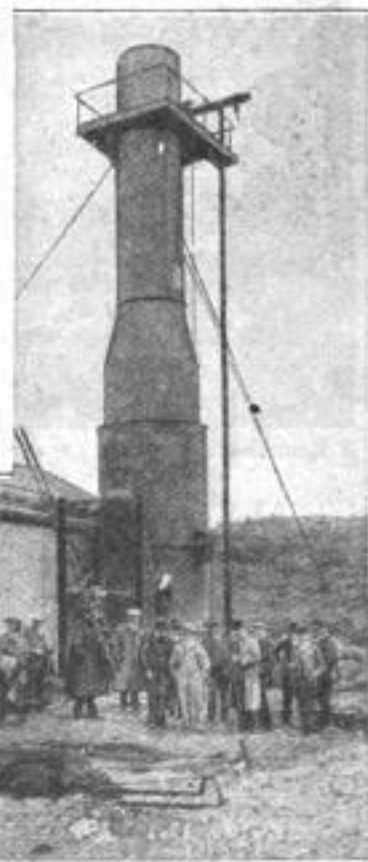
The Blast Furnace, and the Elevated Platform from Which the "Ferro-Coke," Made of Baked Iron Sand and Coal Dust, is Dumped into It
