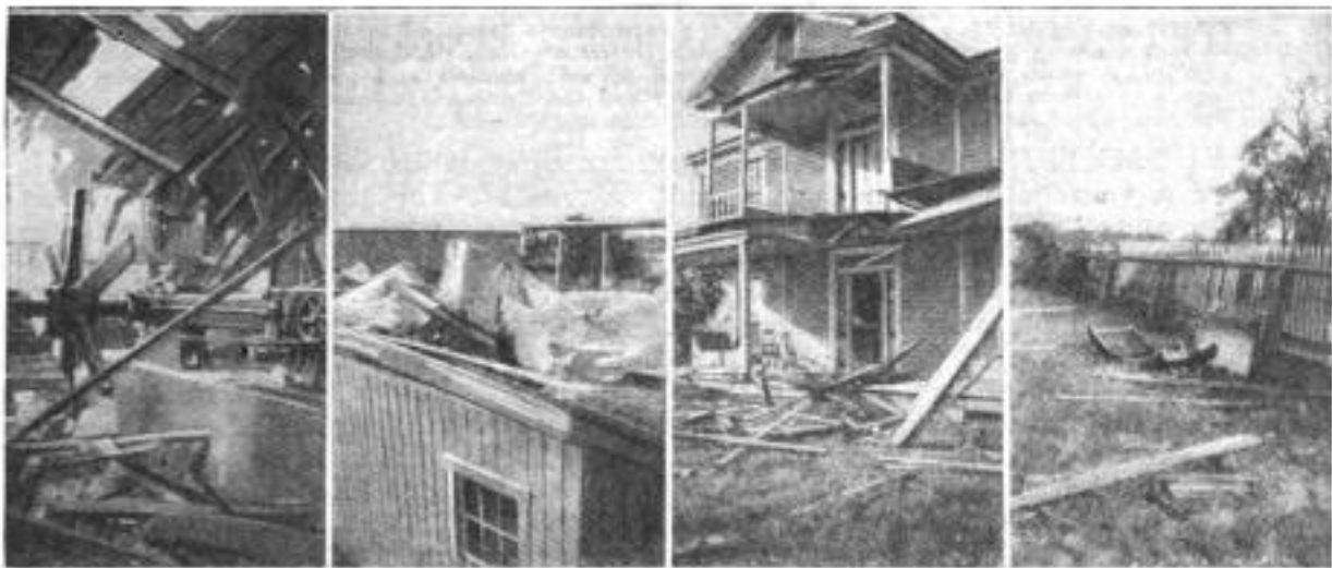
Wreckage Caused by the Bursting of a Large Flywheel. Left to Right: The Wrecked Engine; the Roof of the Engine Room; the Demolished Porch of a Dwelling, and a Section of the Wheel Found 500 Feet Away
