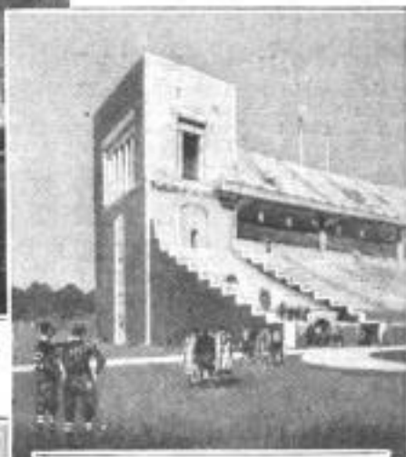
The Southwest Tower of the Stadium, 107 Feet High, with One of the Structure's 56 Stairways That Lead to 112 Aisles
