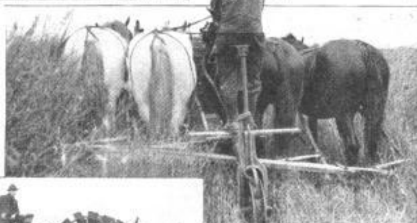
Above: Front View of the Machine That Threshes Sweet-Clover Seed in the Field, Indicating the Method of Bending the Plants into the Beater Wheel without Cutting Them. Right: Rear View, Showing That the Four Horses Push, Instead of Pull. This Curious Implement. Below: The Thresher Seen from the Side, as It Appears in Action, Threshing Sweet-Clover Seed over About 15 Acres a Day
