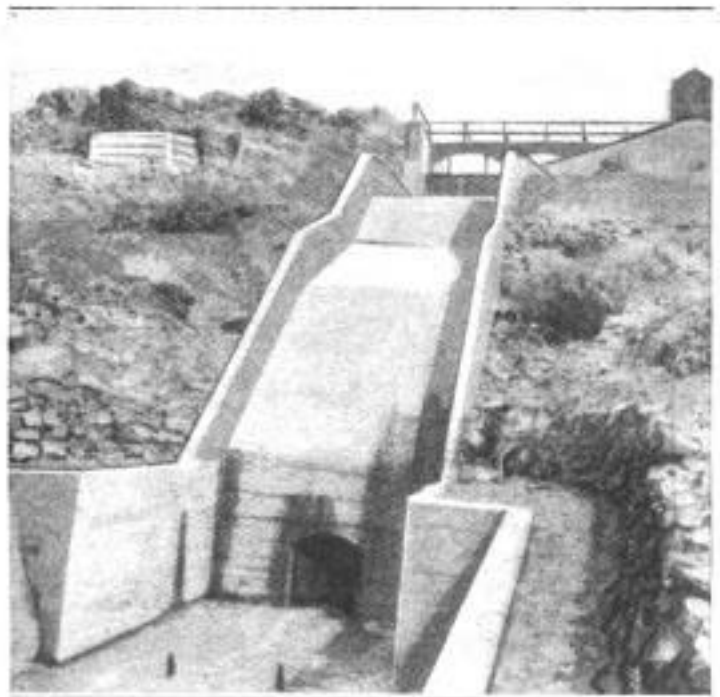
The Concrete Spillway of One of the Two Dams Already Built at Little Salt Lake. Designed to Convert That Useless Saline Basin into a Reservoir of Fresh Water, from Which 10,000 Acres of Land will be Irrigated
