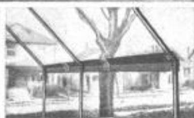
Top: The Frame Erected, Ready for Its Canvas Cover. Left: The Four Steel Tubes and Connecting Lugs of a Single Form. Right: A Detail of the Completed Structure, Showing the Sheet-Metal Connector
