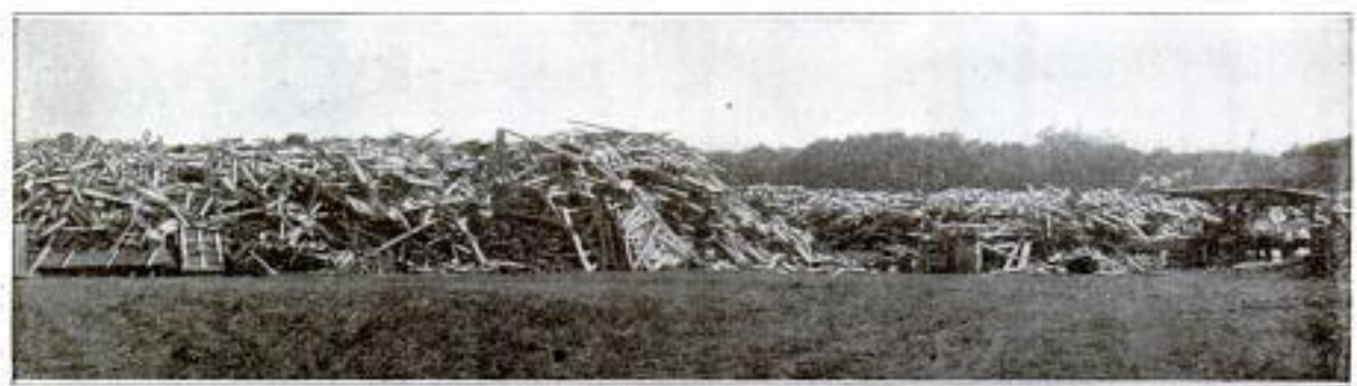
One of Two Immense Piles of Scrap Lumber Accumulated While Erecting Buildings at Camp Funston, Fort Riley, Kansas: At the Right can be Seen a Crew of Men with a Buzz Saw Engaged in Sorting and Trimming the Good Pieces
