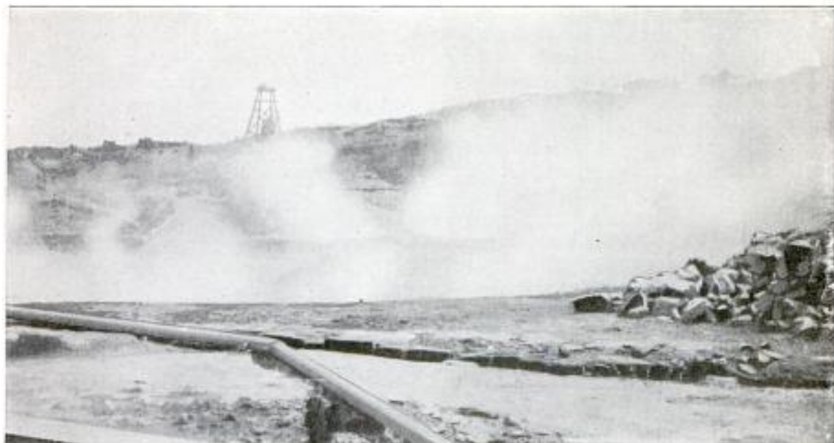
In the Background, Partly Clouded, Is One of the Squat Derricks, and in the Foreground a Pipe Line That Carries Subterranean Steam to the Power Plant
