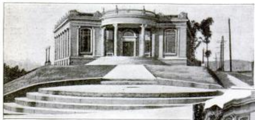
Front View of Library Showing How Circular Steps in Foreground Take Up the Difference in Street Levels: Note That the Building's Plan Conforms to the Shape of the Lot
