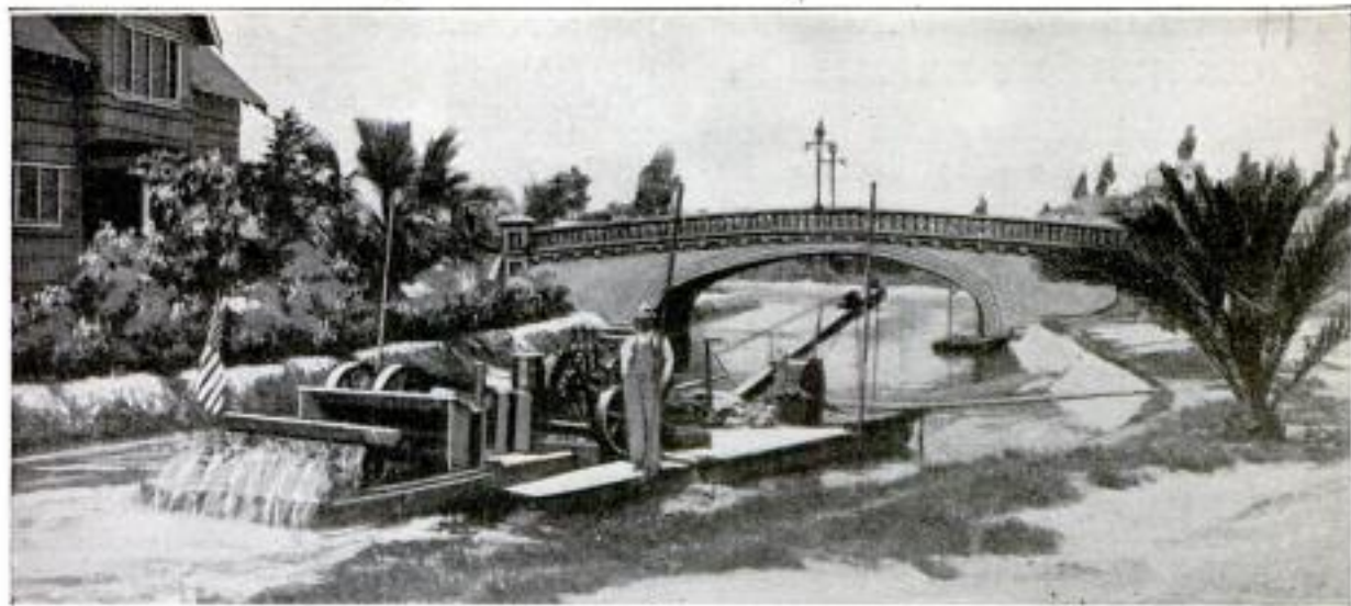
An Anchored Scow with Which Water is Kept Moving through a System of Canals by Driving the Rear Paddle Wheel at Full Speed: Scum and Débris are Collected in a Net Stretched across the Channel
