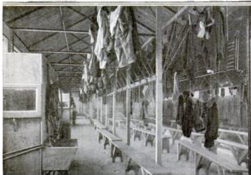
One Section of a "Change House" in Which Provision is Made for Drying the Work Clothes of Miners
