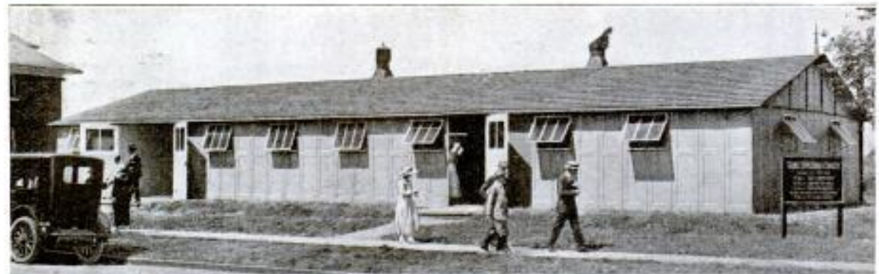
An All-Steel Church. Built for Temporary Use: Its Walls are Composed of Interlocking Panels Which can be Readily Taken Apart When the Time Comes to Move It to Make Room for a Permanent Structure
