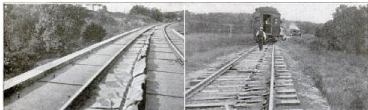
Left: Railroad Bridge Showing Rut in the Sheet-Iron Covering Made by a Derailed Tender Truck. Right: This Photograph Shows the Point at Which the Cars Came to a Stop After the Engine and Tender Broke Away from Them; had This Not Happened the Whole Train Might have been Plunged into a Ravine
