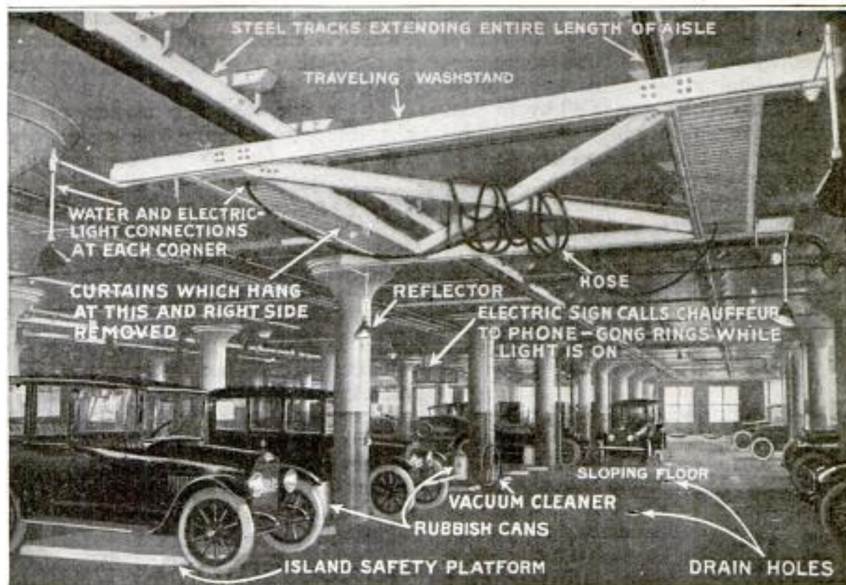
General View of One of the Floors Showing the Movable Wash Rack Suspended from Overhead Tracks: The Rack is Placed above a Car That is to be Washed and Curtains are Drawn Down from It to Inclose the Automobile so That Near-By Cars will Not be Splashed
