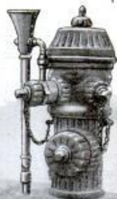
By Making Direct Connection with One of the Outlets of a Fire Hydrant This Convenient Drinking Fountain has been Installed in Galion, Ohio, at Slight Expense. The Overflow Leads to a Sewer Below
