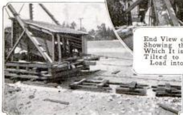
Above: The Mouth of Tunnel Extending under Piles of Material. Below Is a View of the Shovel That Pulls Itself on Skids
