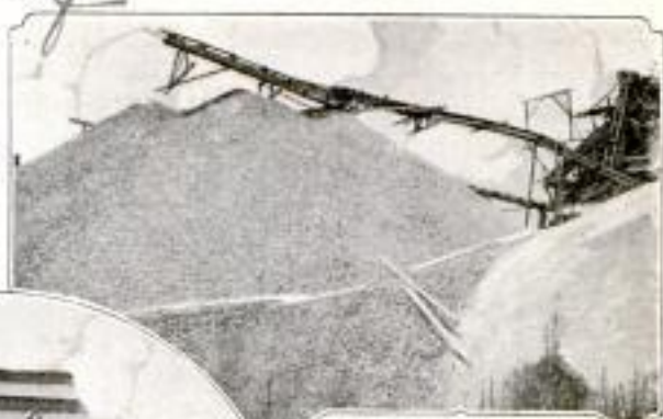
The Extensible Conveyor Platforms over the Piles are Shown Above. Below Is a Rear View of the Steam Shovel in the Arroyo
