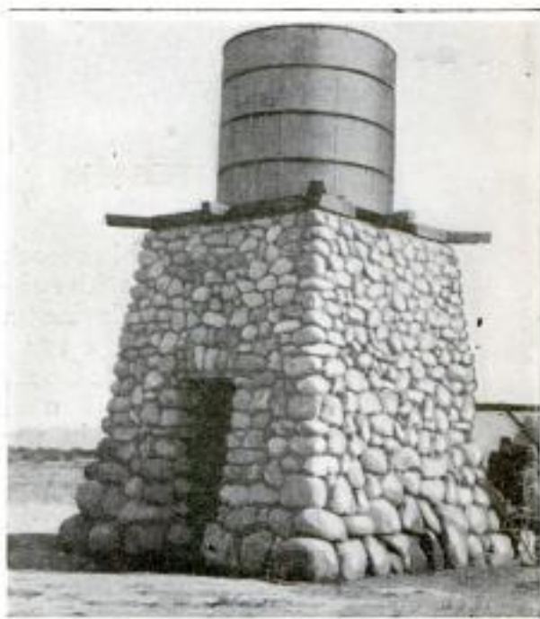
By Utilizing Boulders Picked Up on His Land a Rancher Was Able to Build a Tank House at Low Cost
