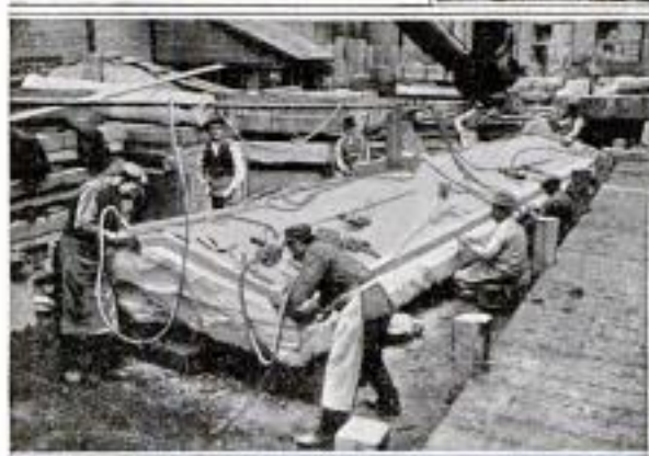
Workmen Spent Six Months in Quarrying and Finishing This Massive Roof Stone. The Building is Situated in a Small Park in the Heart of the Town Where the Late President was Born
