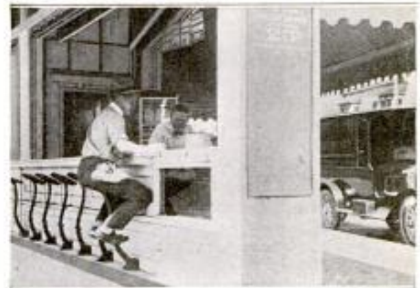
Lunch Room in V-Shaped Area with Counters So Arranged That the Patrons' Stools Project over the Sidewalk
