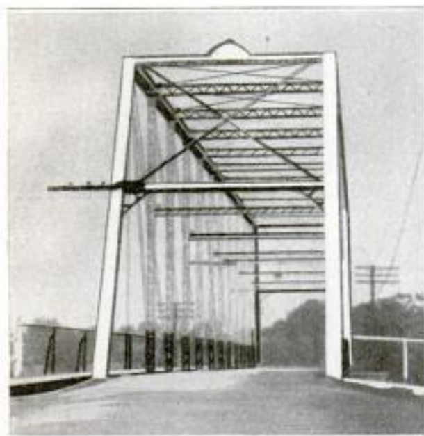
Under the Glare of Motor-Car Headlights the White Bridge Stands Out Conspicuously at Night
