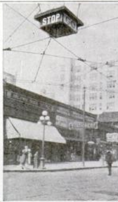
A Central Traffic Signal Which is Supplemented by Semaphores at the Street Corners
