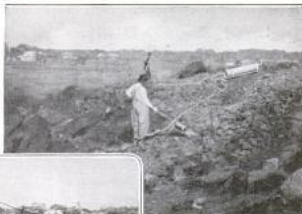
View Showing a Torch, Pressure Tank, and Some of the Rocky Ground being Scorched
