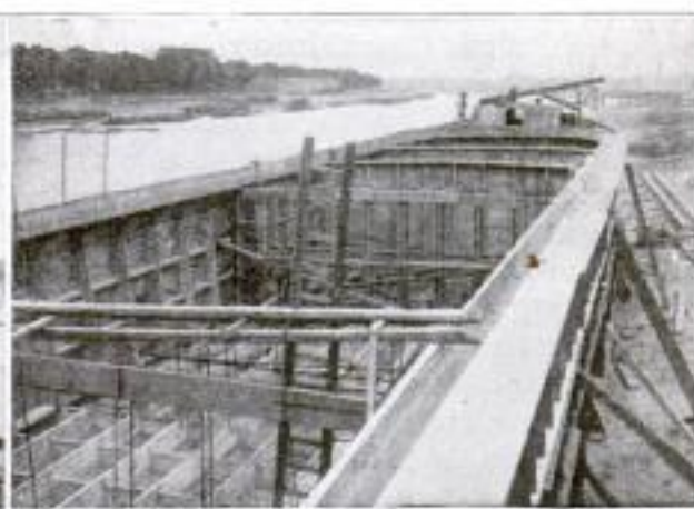
Stern View of One of the Big Concrete Barges after the Partial Removal of the Outside Forms; Right: The Interior of a Boat Nearing Completion with Forms in Place
