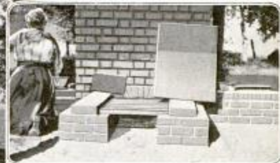
In Providing These Sheltered Fireplaces—of Which There Are Four, with Their Flues in the One Chimney—Pueblo, Colorado, Safeguards Beautiful Fairmont Park against Forest Fires and Makes the Preparation of Meals Easy for Motorists. Each Fireplace Has a Removable Sheet-Iron Cover and Also a Grate. Pine Fuel is Furnished Free
