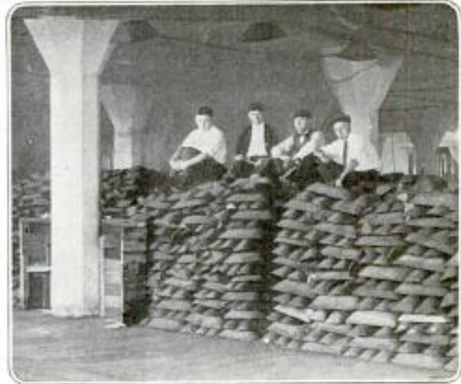
Left: Measuring the Stress on Steel Rods Imbedded in the Concrete. The Stress on Some of the Reinforcing Was 52,000 Pounds per Square Inch. Right: A View Showing Part of the 1,224,000 Pounds of Iron Piled on an Eight and One-Half Inch Concrete Floor in an Unsuccessful Effort to Break It
