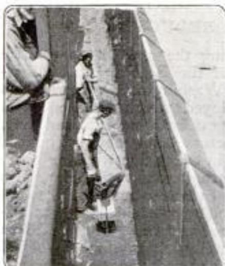
A Testing Hole between Two Rows of Cars: One Advantage of This Outfit Was That It could be Used in a Switchyard Where Cars were being Moved Frequently
