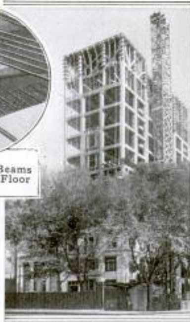
Left: Section of Partly Completed Floor. The Metal Lath are Imbedded in Under Face of T-Beams. Right: General View of 12-Story Concrete Office Building in Process of Construction. The T-Beams in the Floors can be Seen in Several Places
