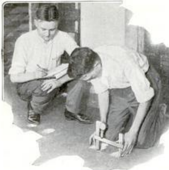
Left: Measuring the Stress on Steel Rods Imbedded in the Concrete. The Stress on Some of the Reinforcing Was 52,000 Pounds per Square Inch. Right: A View Showing Part of the 1,224,000 Pounds of Iron Piled on an Eight and One-Half Inch Concrete Floor in an Unsuccessful Effort to Break It
