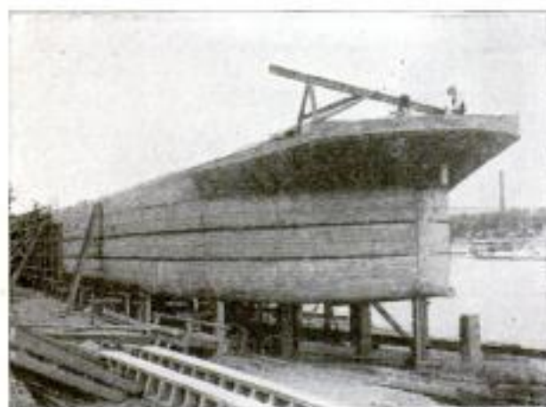
Stern View of One of the Big Concrete Barges after the Partial Removal of the Outside Forms; Right: The Interior of a Boat Nearing Completion with Forms in Place
