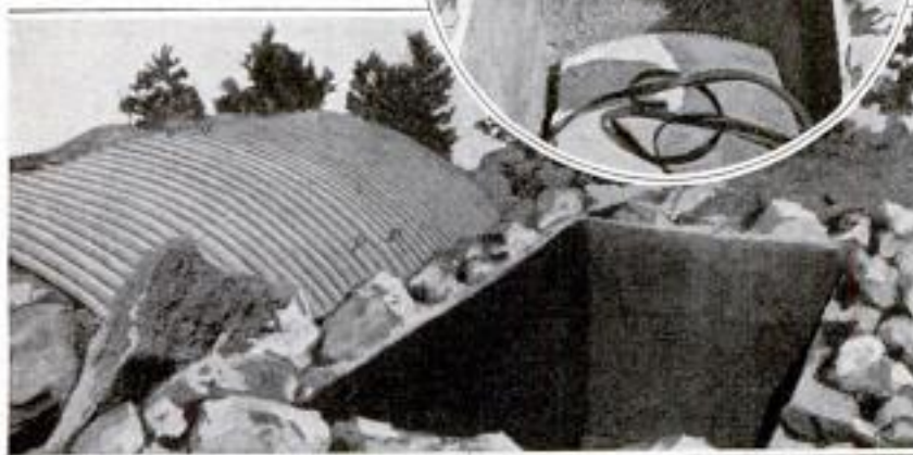
Buffalo Bill's Grave Blasted Out of Solid Rock: The Arched Sheets of Corrugated Iron Helped Form the Roof over the Burglar-Proof Case Which was Inclosed in Concrete
