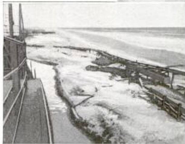
By Dredging the Sand from around It, an Artificial Lake of Sufficient Depth to Float the Vessel was Established on the Beach
