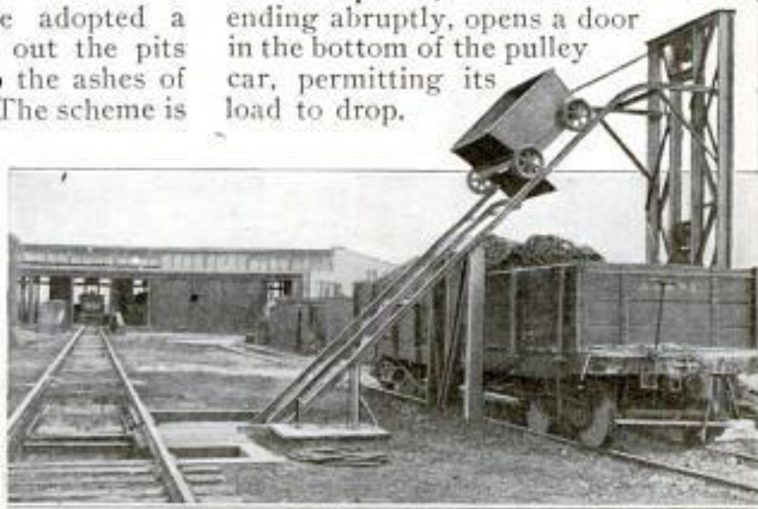
The Small Car on the Incline Runs Down into the Ash Pit beneath the Railroad Track at the Left, and There Receives the Ashes from a Locomotive, Hoists and Dumps Them into the Waiting Gondola
