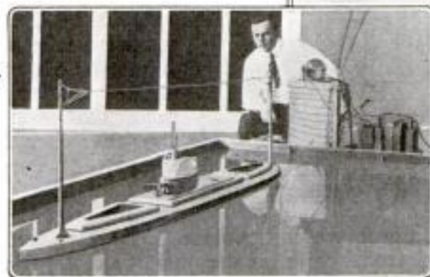
Eight-Hundred-Pound Model Submarine Navigating under Radio Control: The Vessel Responds Instantly to the Whims of Its Inventor
