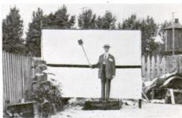
Oilcloth Screen and Green Glass with Which Police Test Automobile Headlights
