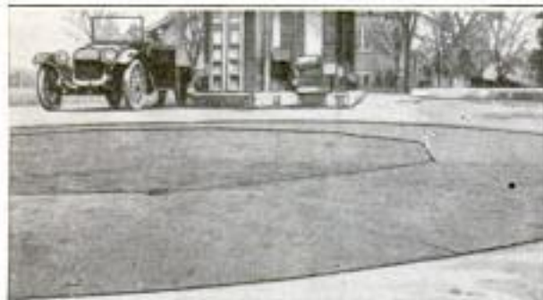
In the Foreground Is an Electrically Operated Turntable Located in a Confined Area Adjoining a Gasoline Station and Used to Turn Patrons' Cars Around
