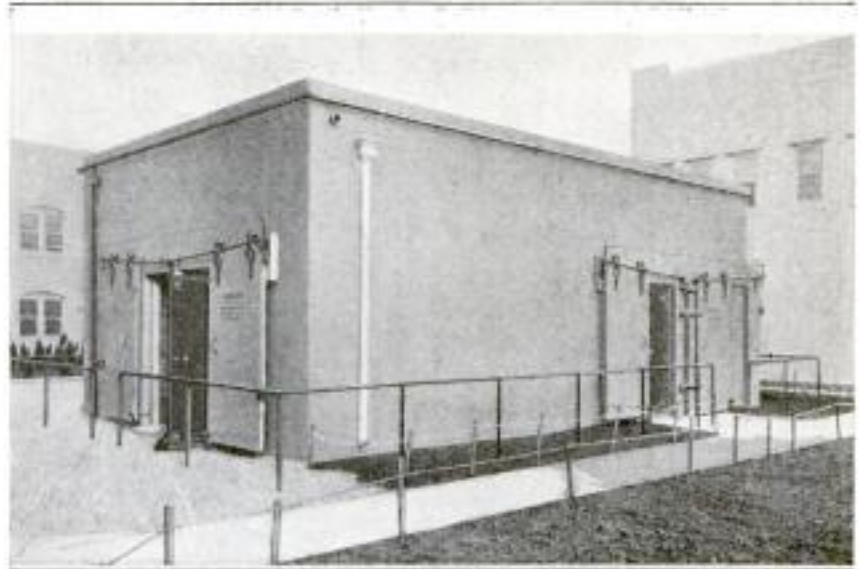
Safety Vault for Picture Film at a Movie Studio: The Building Is of Solid Concrete and Its Roof Is a Water Tank. At Times It Holds $500,000 Worth of Film
