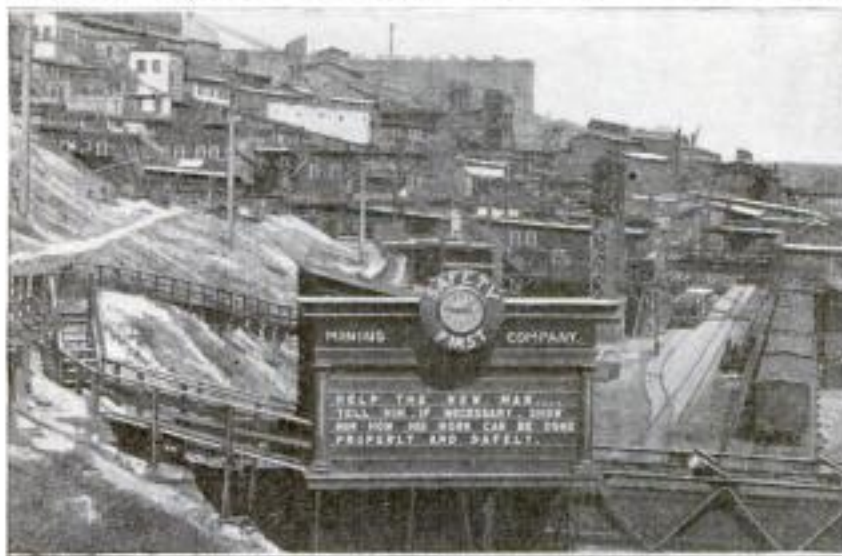
Changeable Safety-First Sign near Entrance to Mining Company's Works: New Legends are Placed on It Daily so That the Men Get in the Habit of Looking at the Board as They Pass
