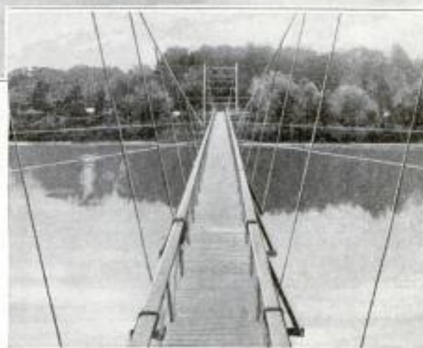
Suspension Bridge, 550 Feet Long and Four and One-Half Feet Wide, Leading to Tyngs Island in the Merrimac River: Access is Gained to It by Passing through a Coin-Operated Turnstile
