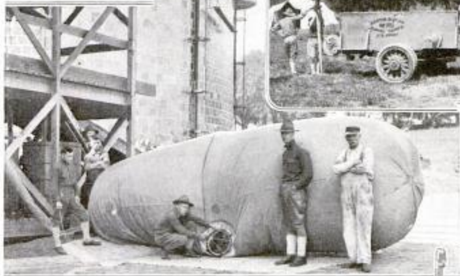
Inflating What is Called a "Nurse" Balloon. Used under Certain Conditions to Supply Limited Quantities of Hydrogen to Big Balloons
