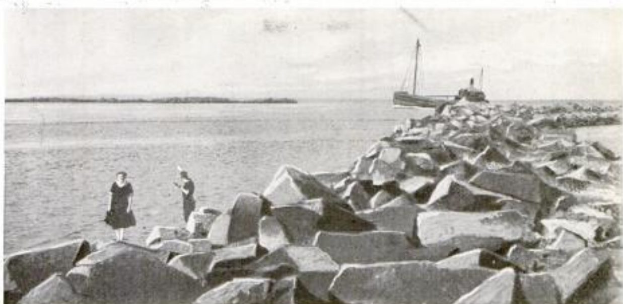
Getting Sand at Low Cost: Dredger Entering River to Load Up with Sand from the River Bottom, Which Formerly was Purchased on a Near-By Island and Carried Aboard in Wheelbarrows
