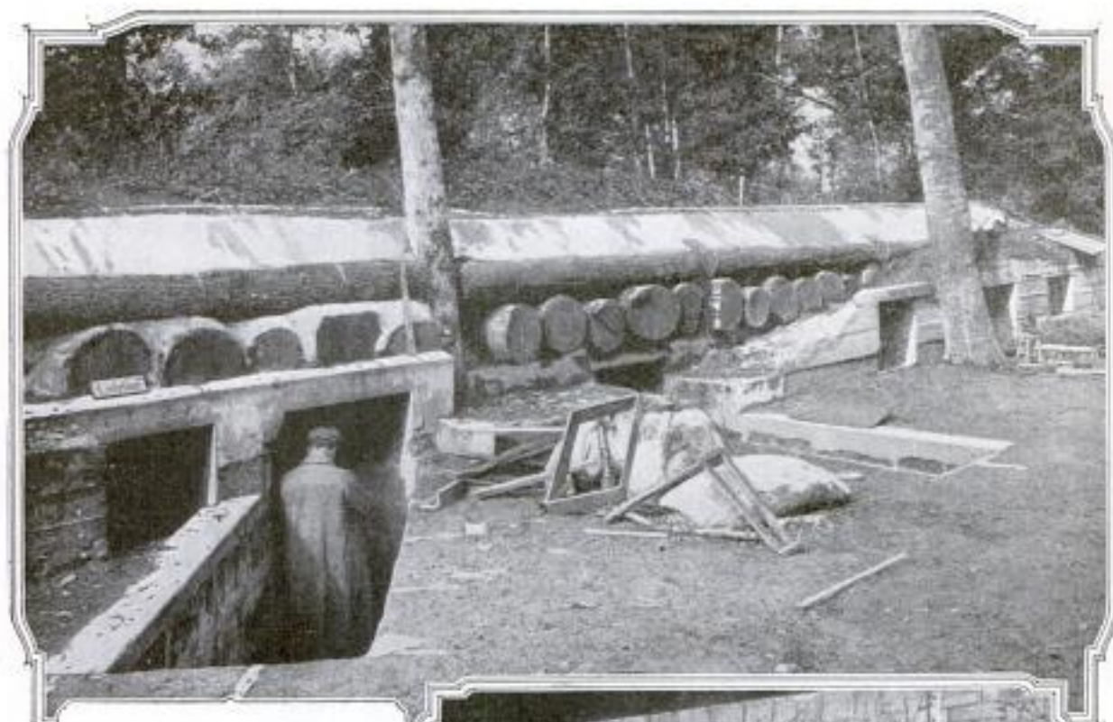
Heavy Timbers and Reinforced Concrete were Used Here in Fortifying the Roof of a Subterranean Post Occupied by the Germans in a Forest on the Western Front. It is an Excellent Example of This Type of Military Construction
