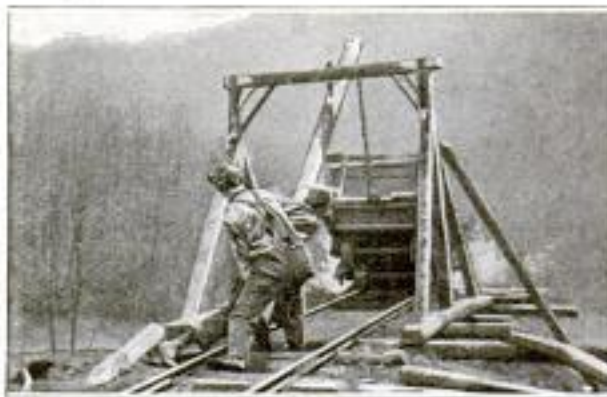
Tipping an Ore Car and Discharging Its Contents on the Dump, with the Aid of a Powerful Lever
