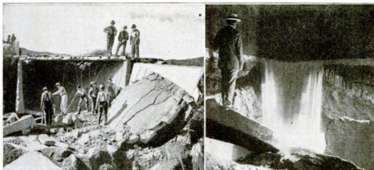
Los Angeles' Great Aqueduct was Broken, as Shown Above, When an Earthquake Caused a Hillside to Slip and a Large Section of the Concrete Flume to Settle Six Feet
