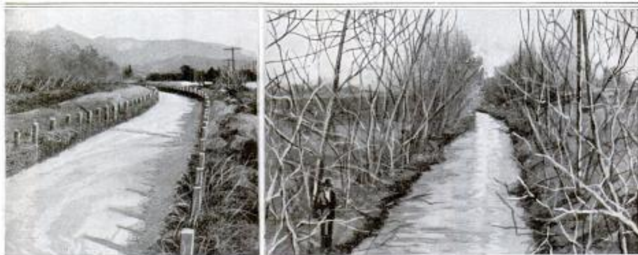
Left: Drainage Ditch in the Dry Season, Showing a Section in Which Railroad Ties were Used in Making a Protective Fence. Right: Portion of the Ditch Lined with Cottonwoods That Grew from Posts
