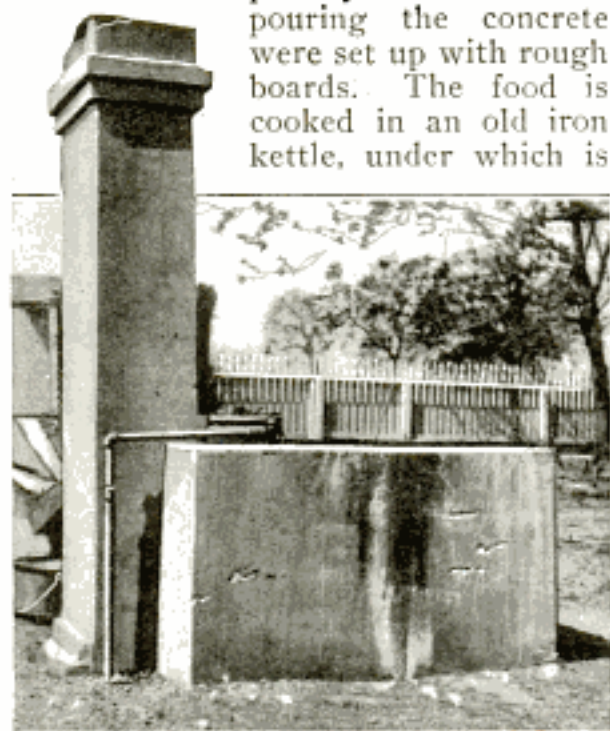
This Concrete Outdoor Farm Cooking Stove can be Made Handily with Simple Forms
