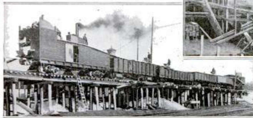
Above is a view of a portable concrete-mixing outfit, including a tower, mounted on a car. At the near end of the material-and-construction train in the left-hand picture, the mixer car is shown with tower removed.
