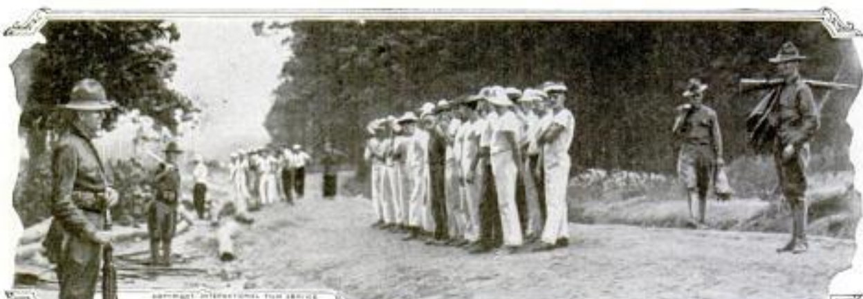
INTERNATIONAL TOUR SERVICE Interned Sailors of the "Kronprinz Wilhelm" Lined Up to be Counted before Beginning Work. The Men are Employed in Erecting Quarters near Fort McPherson, Georgia, Which will Shelter 2,500 Germans
