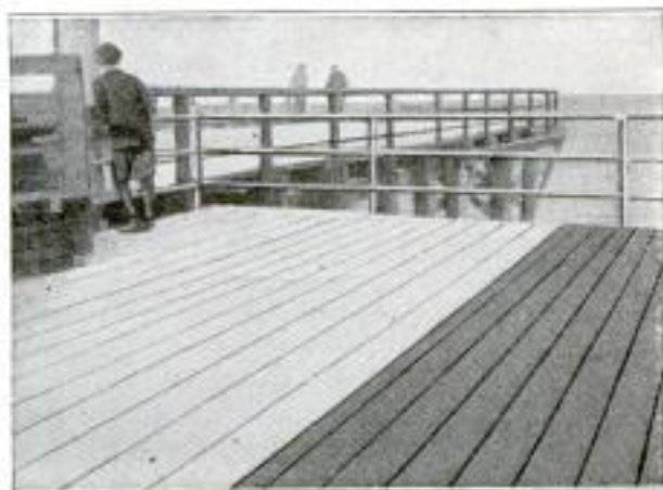
Board Walk at an Ocean Resort Which has been Repaired in Part with Planks of Concrete: These have been Found Very Durable but Less Pleasing to Walk On Than Wood
