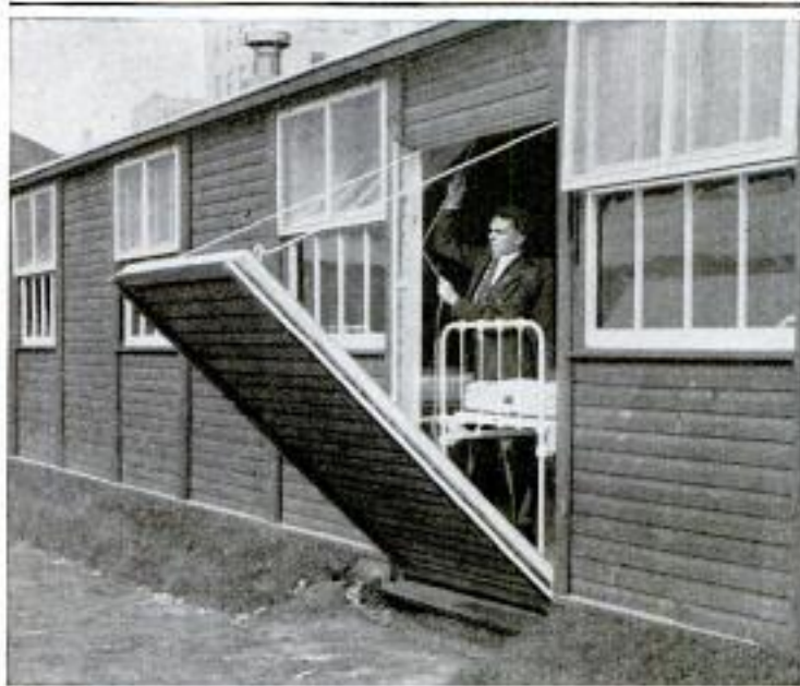
Hinged Panels are Provided to Permit Speedy Evacuation of the Ward Buildings in Case of Fire. This Shows One of Them being Lowered
