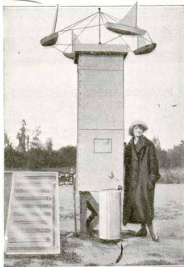
Sailboat Windmill Which Drives the Pump of the Solar Water Heater Seen below It
