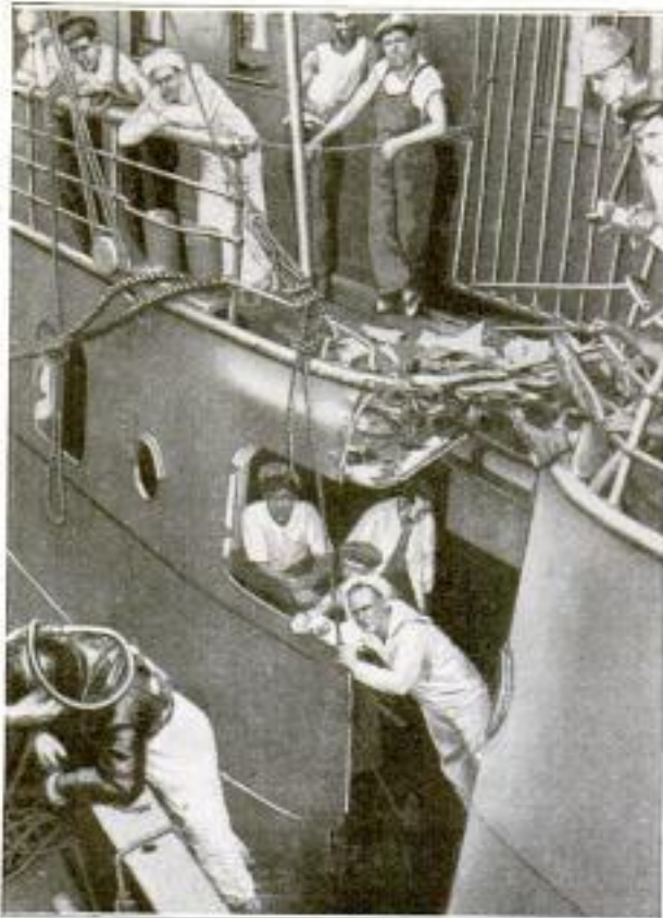
COPYRIGHT, INTERNATIONAL FILM SERVICE A Diver Descending to Determine the Extent of the "Saratoga's" Injuries: The Picture Shows the Hole Torn in the Port Side of the Transport by the Steamship "Panama"
