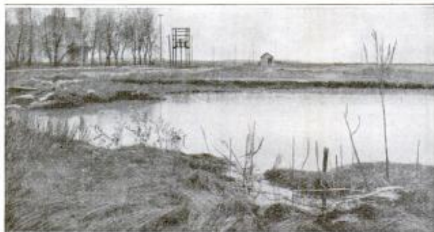
Crater and Deep Lake Formed by the Bursting of an Artesian Well That Threatened to Undermine the Business Part of a North Dakota Village
