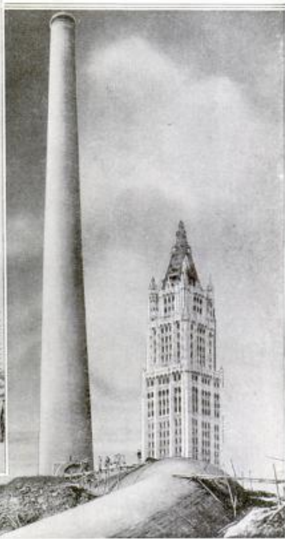
If the Woolworth Building Stood on the Ground beside the Smelter This Chimney Serves, the Stack would Tower above the Building About as Shown
