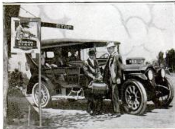
Station on an Auto-Stage Route in the West Showing Semaphore in Front, by Which Drivers are Apprised of the Presence of Waiting Passengers
