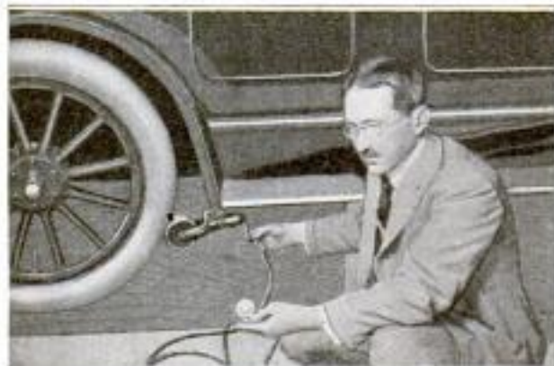
Demonstrating the Method of Attaching the Pump to a Car and Operating It
