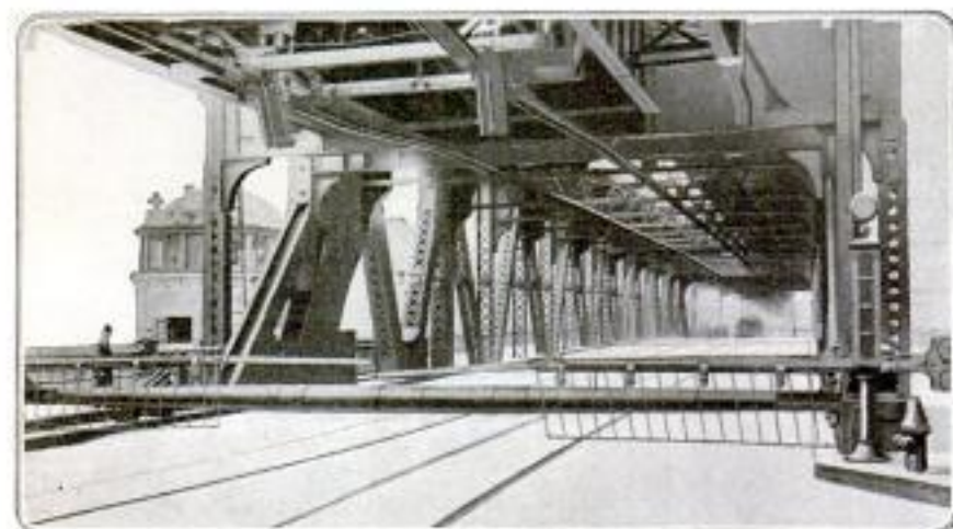
The Heavy Buffer is Shown Just Back of the Safety Gates: The Beam with Its Supports Weighs About Two Tons, and It is Stated That It will Stop a 4,000-Pound Car, Running 30 Miles an Hour, without Accident to the Occupants
