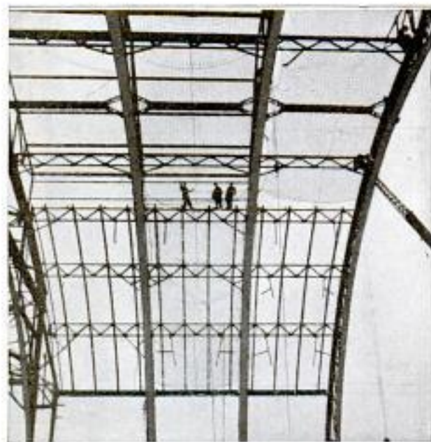
The Safety Nets Pictured Here Were Supposedly the First To be Used in Structural Work; They were Employed at Chicago and Saved the Lives of Two Painters
