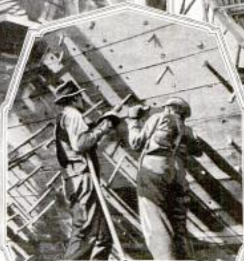
Driving the Pins into Place with a Compressed-Air Hammer, One of the Important Stages in the Construction of a Wooden Hull: The Vessel Has a Cargo Capacity of 2,000 Tons
