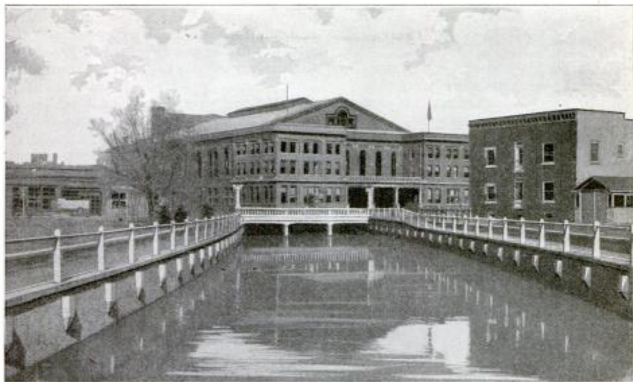
Municipal Convention Hall in Hutchinson, Kansas, Built Directly above a Stream: By Erecting This Attractive Structure, Together with Proper Retaining Walls, an Unsightly Location has been Changed into One of Value and Service
