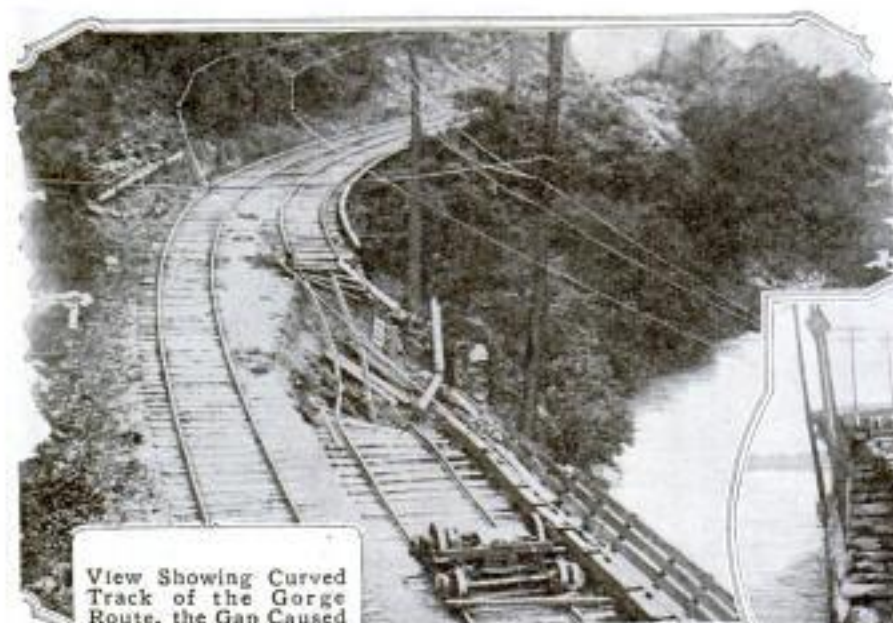
What Fragile Things the Steel Rails Proved to Be When the Embankment was Washed Away is Shown Here
