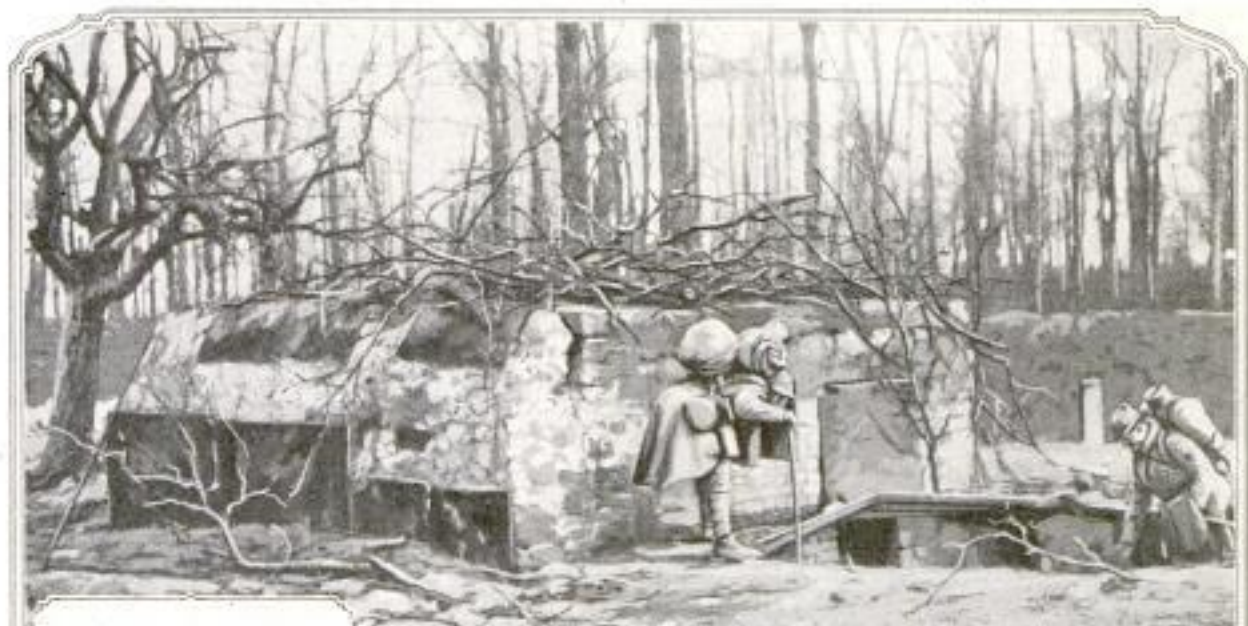
Captured German Machine-Gun Emplacement in Naked Timberland on the Western Front: The Walls are Built of Concrete, Brick, and Flagstones, and on the Fighting Side are Four Feet in Thickness. Entrance to It is Gained through an Underground Doorway. Branches of Trees Cover the Roof to Shield It from the View of Airmen
