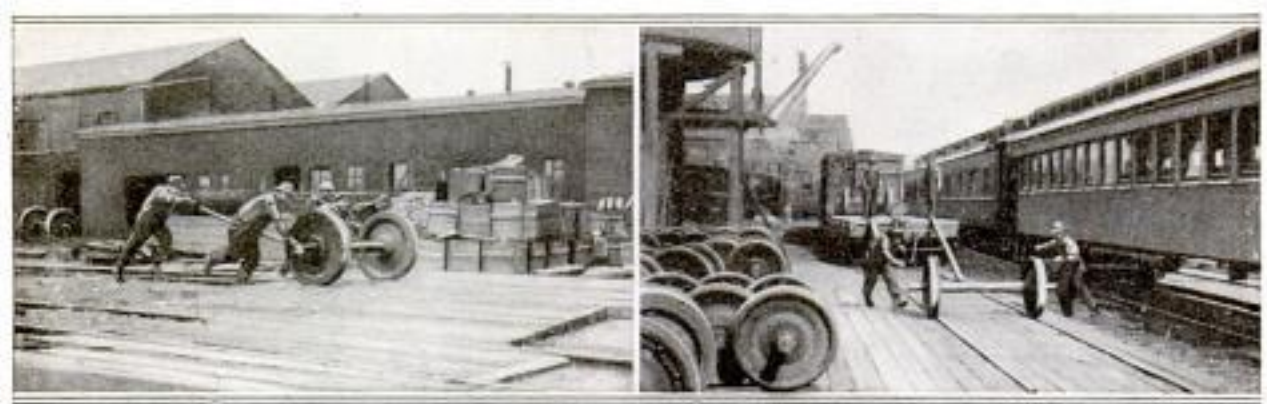
Right: While Dropping down the Incline the Wheels Attain a High Velocity; They are Stopped by the Same Method That a Cowboy Uses in Catching a Steer or Pony — by Lassoing. Left: Starting the Wheels for the Final Rush up the Incline to the Car Floor. The Same Skid is Used for Loading and Unloading
