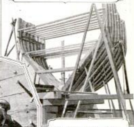
The Hull of the Boat is Constructed of Oregon and California Pine. This Picture Shows How the Ribs are Put in Place, One at a Time. The Ship is 271 Feet in Length
