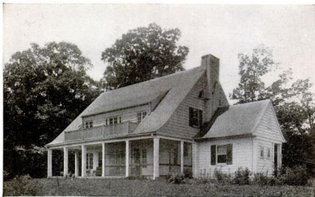
House near Alexandria, Virginia.
