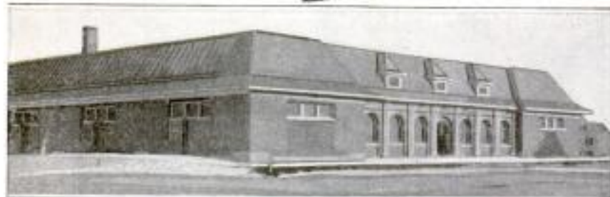
Unusually Large One-Story School at Westfield, Massachusetts, Which Accommodates Nearly 700 Pupils: Considerations of Economy Were Instrumental in Designing This Type of Building. The Rooms are Lighted Chiefly from Above, Like a Studio
