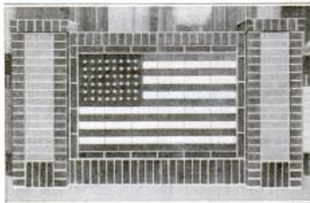
Stars and Stripes in Durable Form: A Brick Reproduction of the Flag, Measuring 48 by 32 Inches. The Stars were Cut from White Brick with a Chisel
