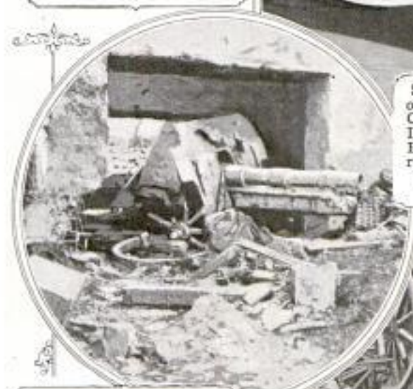
The Strength of the Reinforced-Concrete Emplacements is Indicated by the Picture Above, Which Shows a German Gun Silenced by the British. Apparently the Projectile Fell from a High Elevation, Thus Passing the Parapet in Front. The Explosion Wrecked the Cannon, but Did Little Damage to the Surrounding Walls
