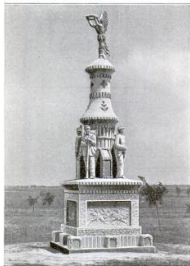
The Figures and Panels on the Memorial Are Free-Hand Modelings in Concrete
