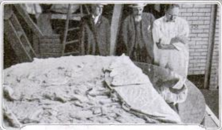
The Layers of Cotton Turned Back to Show a Small Section of the Silvered Surface of the Mirror: It Is the Largest Reflector of Its Kind in the World and will Enable Astronomical Investigations That Are Not Possible with Smaller Instruments.
