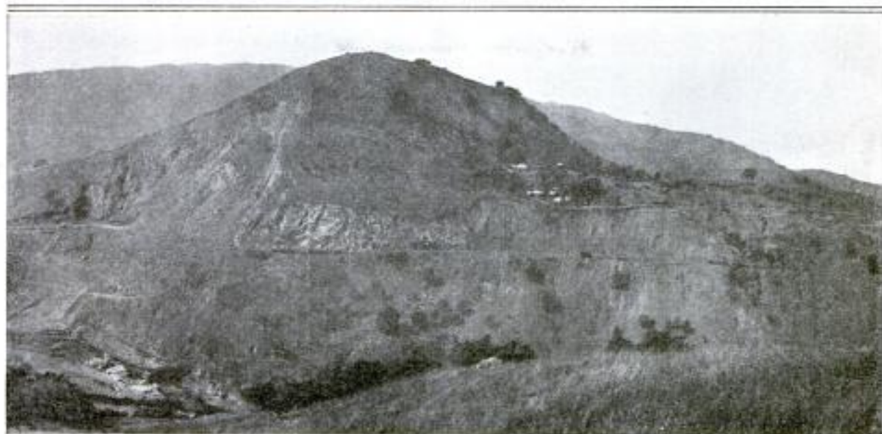
the City's Water Supply and will Be the Largest Earth Dam in the World: The Length at the Crest will Equal Outlet-Control Tower, 239 Feet High, and Working Camp in the Background
