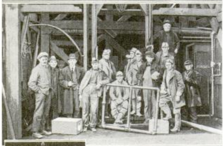
Group of Tunnel Workers in Cleveland with Portable Storage-Battery Lights in the Foreground. Some of the Men's Caps are Equipped with Electric Lamps Also
