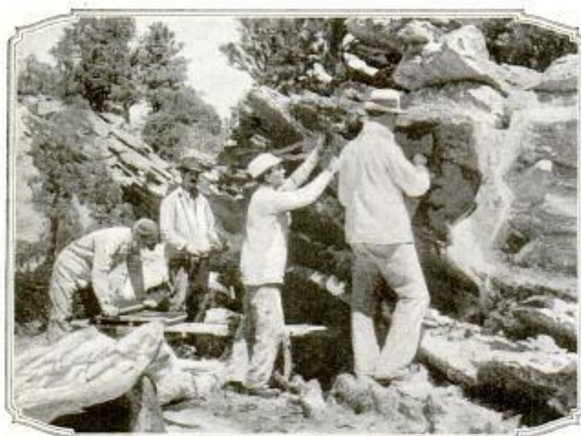
The First Step in Preparing a Replica of a Cliff: Covering It with a Layer of Clay One-Half Inch Thick
