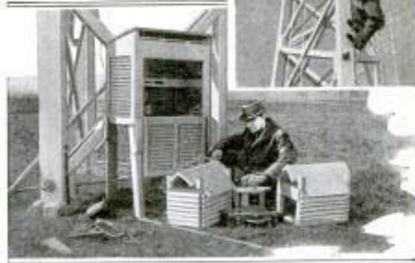
Placing Instruments in Shelters for Hoisting to the Top and Middle of Wireless Tower Used as a Meteorological Observatory by Oregon Fruit Growers; Below are Shown the Housings Used for the Instruments
