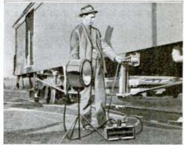
Portable Lighting Outfit for Repair and Inspection Crews Supplied with Current from the Car's Storage Batteries: The Resistance Coil Shown is Employed to Keep the Light Constant as the Supply of Electricity Diminishes
