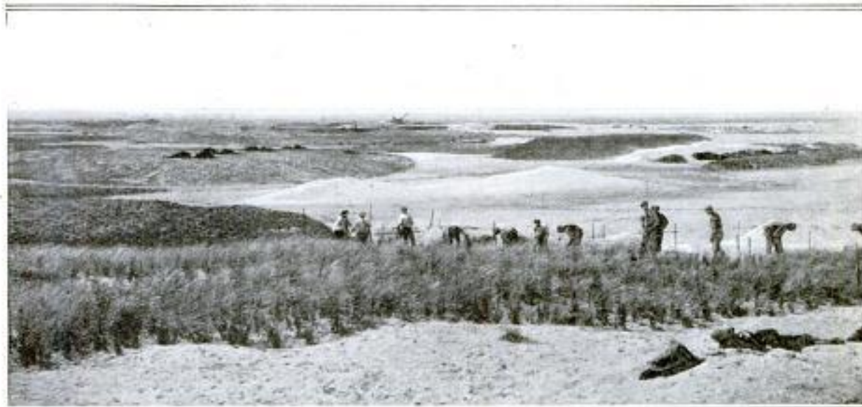
Preparing Subsoil and Putting In Eelgrass: The Latter was Employed at Various Points to Prevent the Sand from being Swept Away by the Strong Winds. Other Parts were Tufted and Covered with Grass to Serve as Tees and Bunkers
