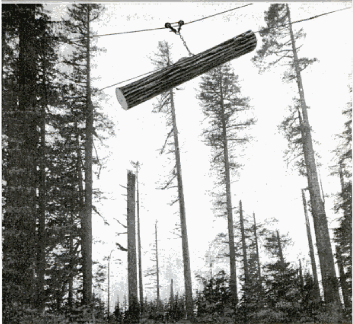
Hauling a Log Out of the Woods with a Sky-Line Trolley: The Top Cable is Held Fast by a Donkey Engine, Which Also Pulls the Log Out by the Line Attached to Its Forward End
