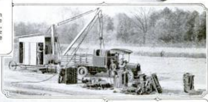
Unloading the Asphalt Blocks from the Cars: To Reduce the Handling of Material to a Minimum, the Blocks are Piled into Low-Wheeled Cages, Some of Which are Shown on the Top of the Car. The Derrick Transfers Them Bodily to the Waiting Truck, from Which They are Eventually Unloaded, by Similar Means, near the Pavers
