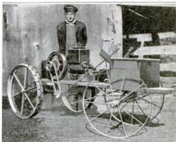
Fig. 2. The Belting of the Power from the Engine Shaft to the Lower Shaft, Which Connects with the Pitman Shaft on the Opposite Side, and the Clutch-Control Rod are Shown in This View
