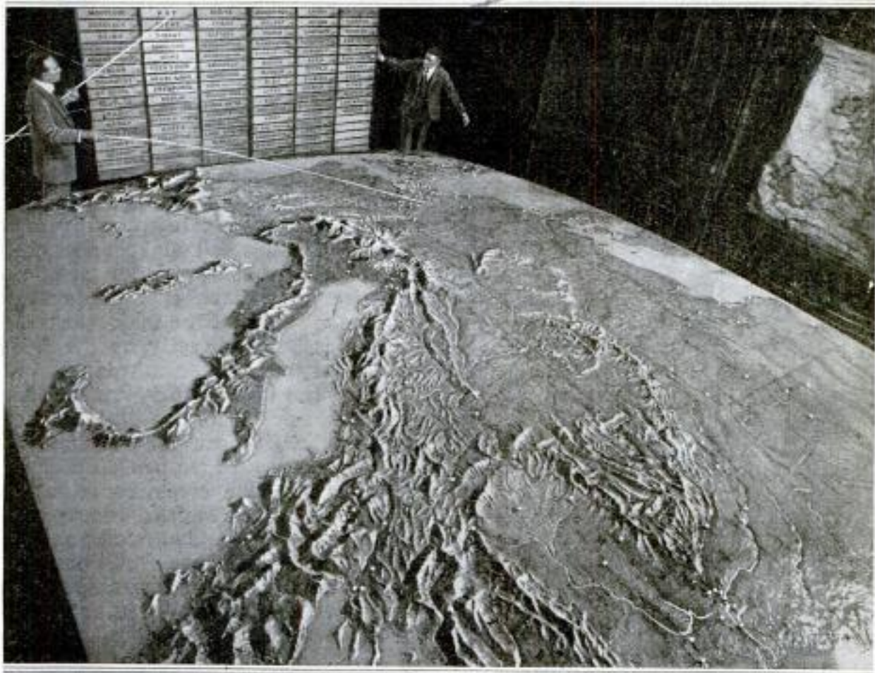
Curved Relief Map of Europe Measuring 15 by 20 Feet: The Location of 200 Places is Indicated by Electric Bulbs Which can be Lighted as the Demonstrator Desires. The Names and Numbers of the Index are Illuminated Simultaneously with the Corresponding Bulbs
