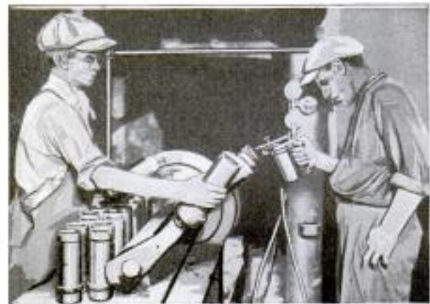
COURTESY OF MACHINERY With This Machine Two Boys can Spray a Varnish Coating on the Inside of 400 Shells per Hour
