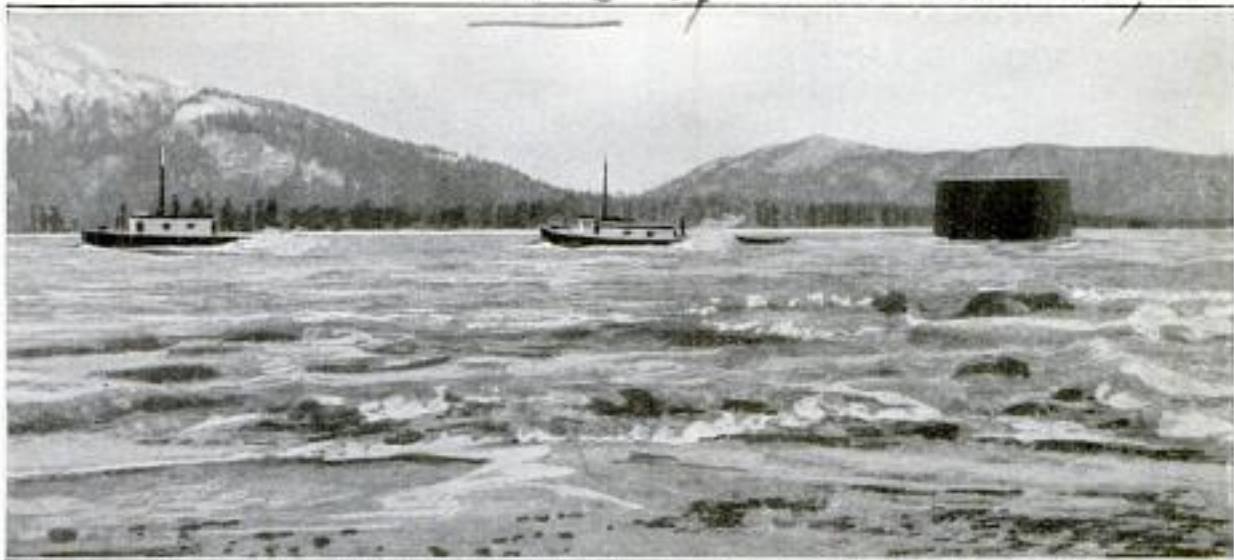
Towing an Oil Tank along the Alaska Coast to a New Location: The Tank Is 45 Feet in Diameter and Drew Only Six Inches of Water When Floated for the Voyage
