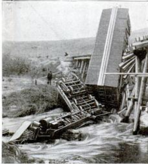
View of Railroad Wreck That Occurred When a Freight and Passenger Train Started to Cross the Wooden Bridge, Which had been Weakened by a Freshet
