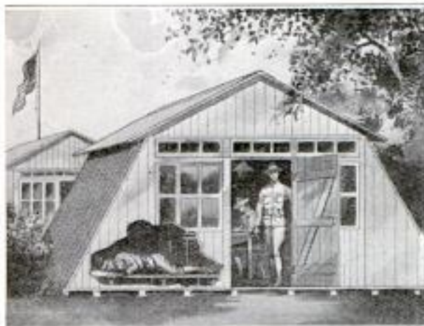
Wooden Hut Made of Sections That can be Quickly Assembled: Its Spreading Side Walls Allow Sleeping Space on the Floor for Two Rows of Soldiers. Rifle Racks are Provided Adjoining the Side Walls
