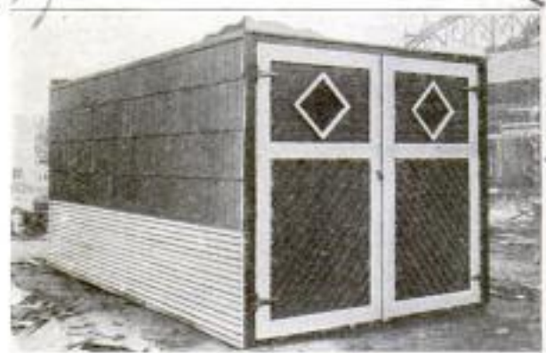
Type of Portable Garage Which Measures 17 by 9 by 8 Feet and Rents for $2.50 per Month: It can be Transported Either Knocked Down or with Parts Assembled
