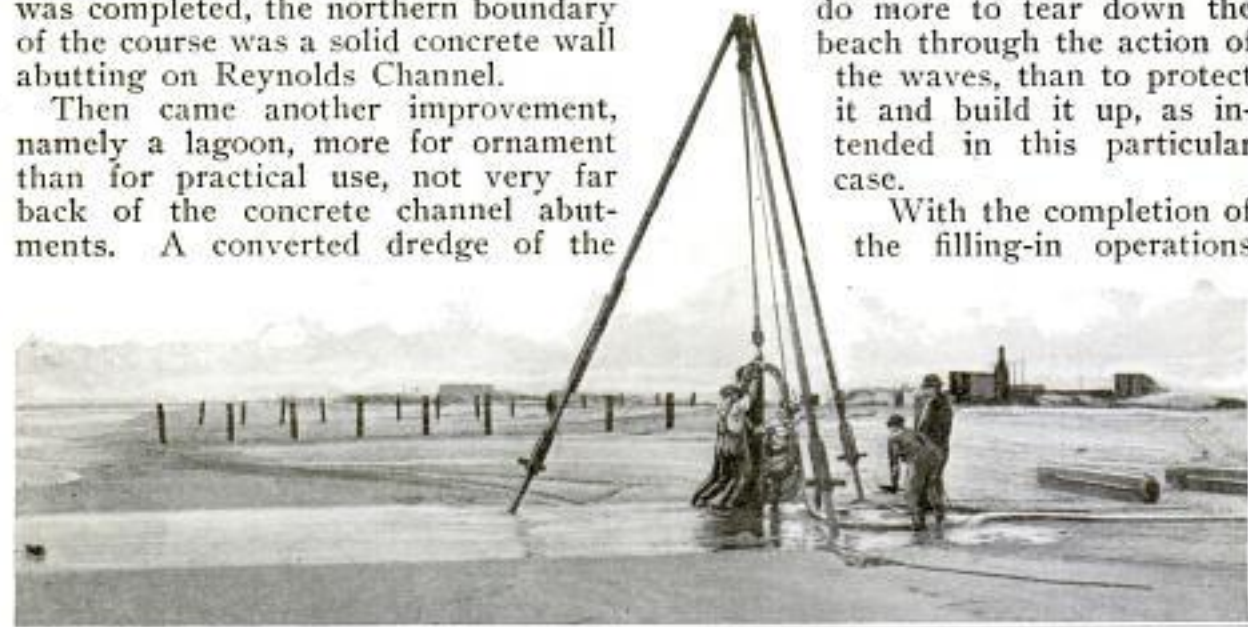
Protecting the Ocean Side of the Golf Course from the Action of the Waves: Wooden Piles were Sunk at Intervals and Boarded Up in Such a Way as to Avoid Producing Destructive Eddies
