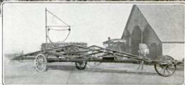
The Harrow Folded Together at the Central Wheel for Transportation
