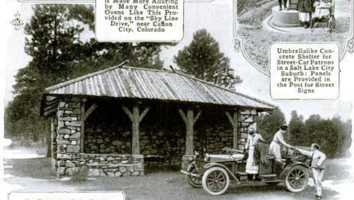
An Example of the Provision Made for Visitors in Its Beautiful Mountain Parks by the City of Denver: Stone and Undressed Pine have been Used Very Effectively in This Shelter
