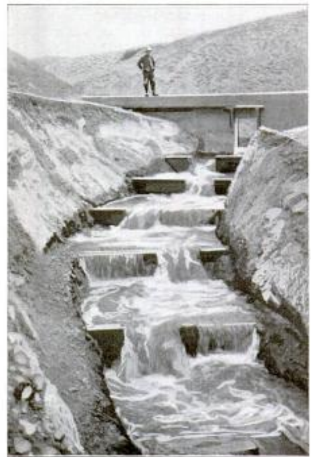
Runway in a Nevada Stream, Comprising a Series of Low Artificial Falls Constructed so That Small or Weak Fish can More Easily Make Their Way Upstream to Spawn
