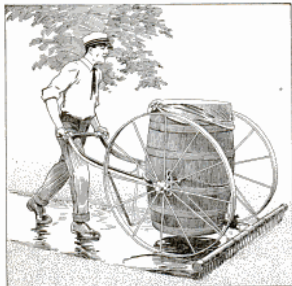
Occasional Oiling of Roadways with a Homemade Sprinkler will Keep Down Dust around the Home
