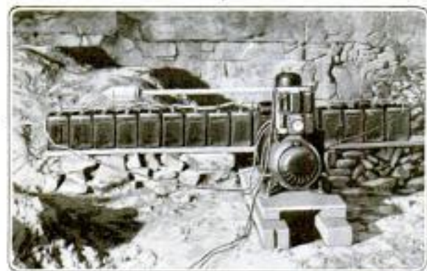
Electric Lighting Plant Newly Installed in the Mammoth Cave of Kentucky, Hitherto Lighted by Oil Lamps
