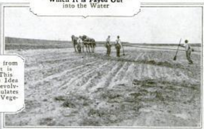
Team of Horses Pulling in the Cable about Which the Moss has Accumulated: The Long Steel Line is Divided into Sections by Swivels Which Permit the Various Parts to Revolve Freely as They are Drawn Across the Bottom of the Reservoir
