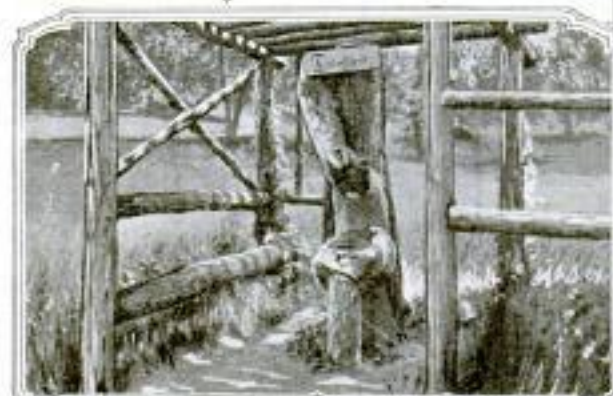
A Rustic Fountain in Sioux City, Iowa, Having as Much Charm as an "Old Oaken Bucket": The Hollow Knot That Serves as a Bowl, to Which Concealed Pipes Lead, is Cement-Lined
