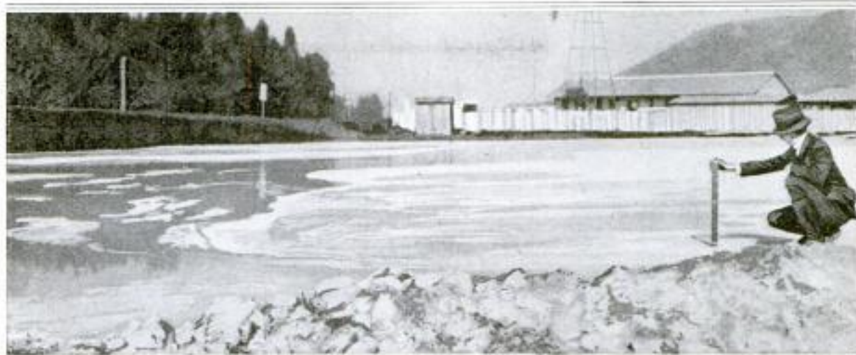
Sludge Pit of an Acetylene-Gas Charging Station, Containing the Slaked-Lime Residue of Calcium Carbide. Now Used for Plaster and Whitewash: Such Pits Are Sometimes Several Feet Deep
