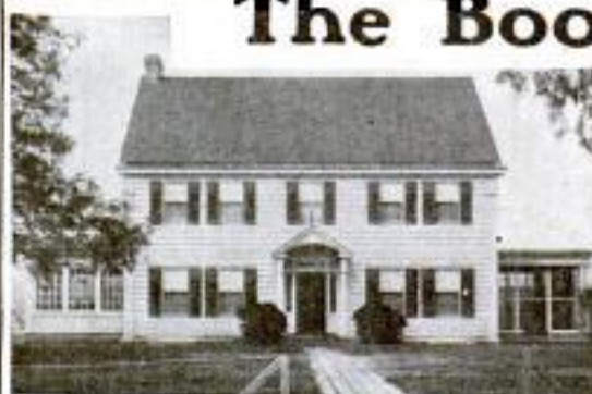
Walls finished with Cabot's Old Virginia White. Roof stained with Cabot's Creosote Stain Person & Goodrich, Architects, N. Y.
