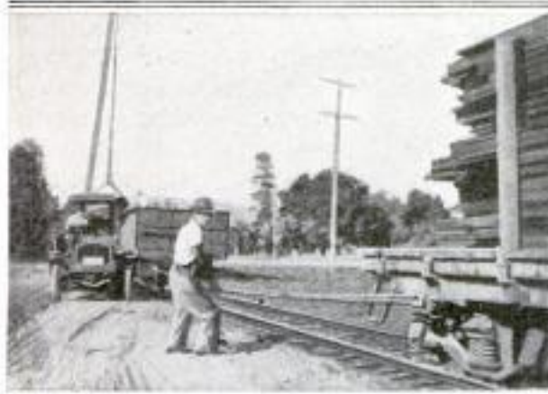
Two Views Showing the Way in Which an Automobile Truck was Employed to Hoist Heavy Water Mains from a Gondola Car and Then Lower Them onto Itself
