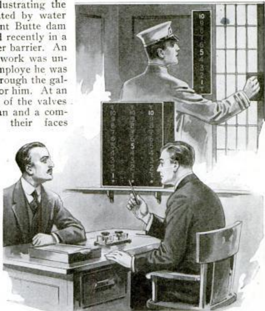
In Each Elevator There Is an Indicator That Shows the Operator the Positions of All the Cars. Only the Progress of the Pursuing Car Need be Watched to Keep All of the Lifts in the Proper Order
