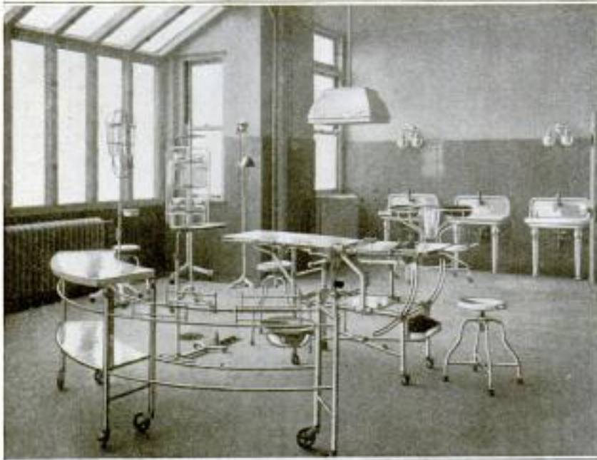
One of the Rooms in the Operating Pavilion of a Cincinnati Hospital: Note the Studio-Lighting Effect, and the Wheeled Furniture Which can be Moved without Handling
