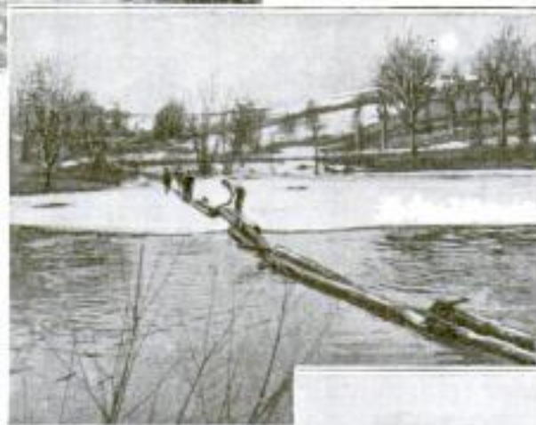
Citizen Volunteers Stringing a Boom across the River to Save the Dam from Further Damage by the Ice
