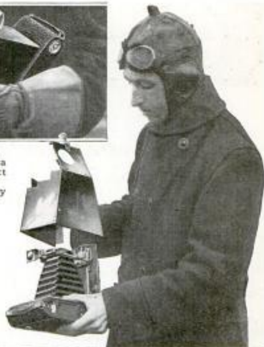
The Shield Is of Aluminum and is Made Like a Collapsible Carton so That It can be Folded Up and Carried in the Pocket
