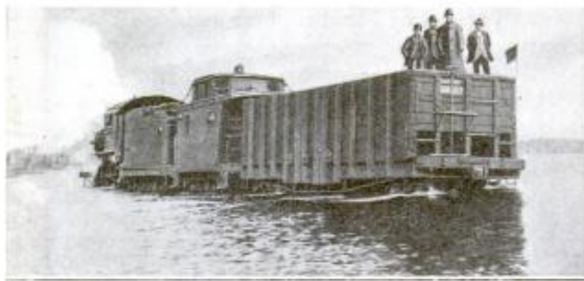
Railroad Men Investigating Condition of Submerged Track by Backing a Short Train onto It Very Cautiously
