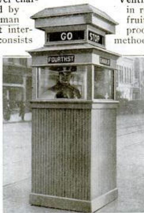
Comfortable Shelter for Traffic Policeman in Dayton, Ohio: The Booth is Lighted and Heated by Electricity
