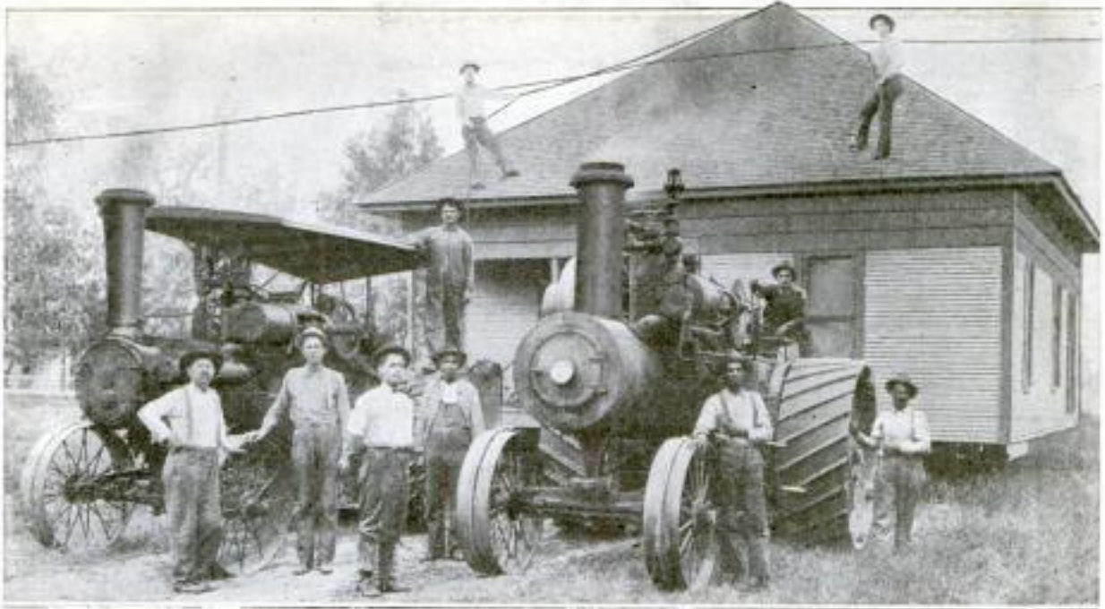
Moving an Oklahoma Town to a New Town Site on a Railroad: The Buildings are Hauled by Tractors, as Shown, Sometimes to Distances of 10 or 20 Miles from Former Sites
