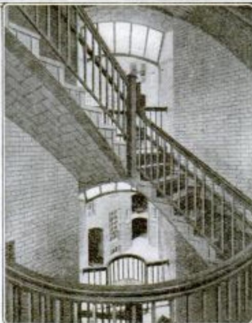
The Open Stair Eliminates the Hallway of the Tenement, and Increases the Privacy of Each Apartment
