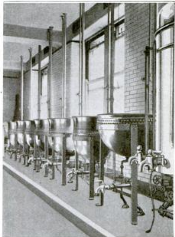
Battery of Aluminum Kettles in Kitchen of a Chicago Hospital; These Vessels are Partly Inclosed in Jackets into Which Steam is Injected to Heat the Contents of the Kettles
