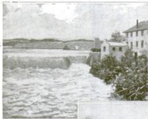
Scene When the Mazeppa, Minnesota, Dam was Expected to Give Way, After Part had been Torn Out, as Shown
