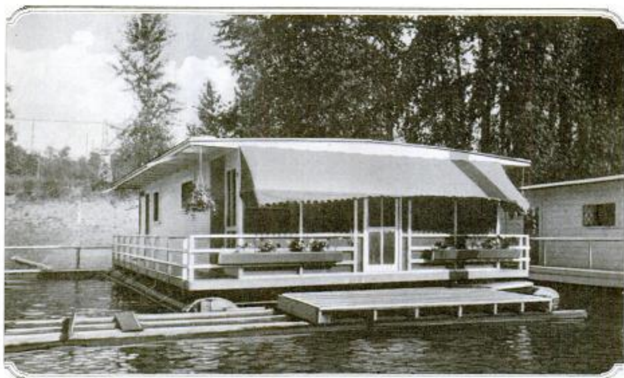
Typical House Boat of the Willamette River Colonies: This One Has Four Rooms and Bathroom. Entrance from the Board Walk Is at the Rear. Note the Ideal Diving Platform, the Flower-Bedecked Porch, and the Big Logs on Which the House Floats
