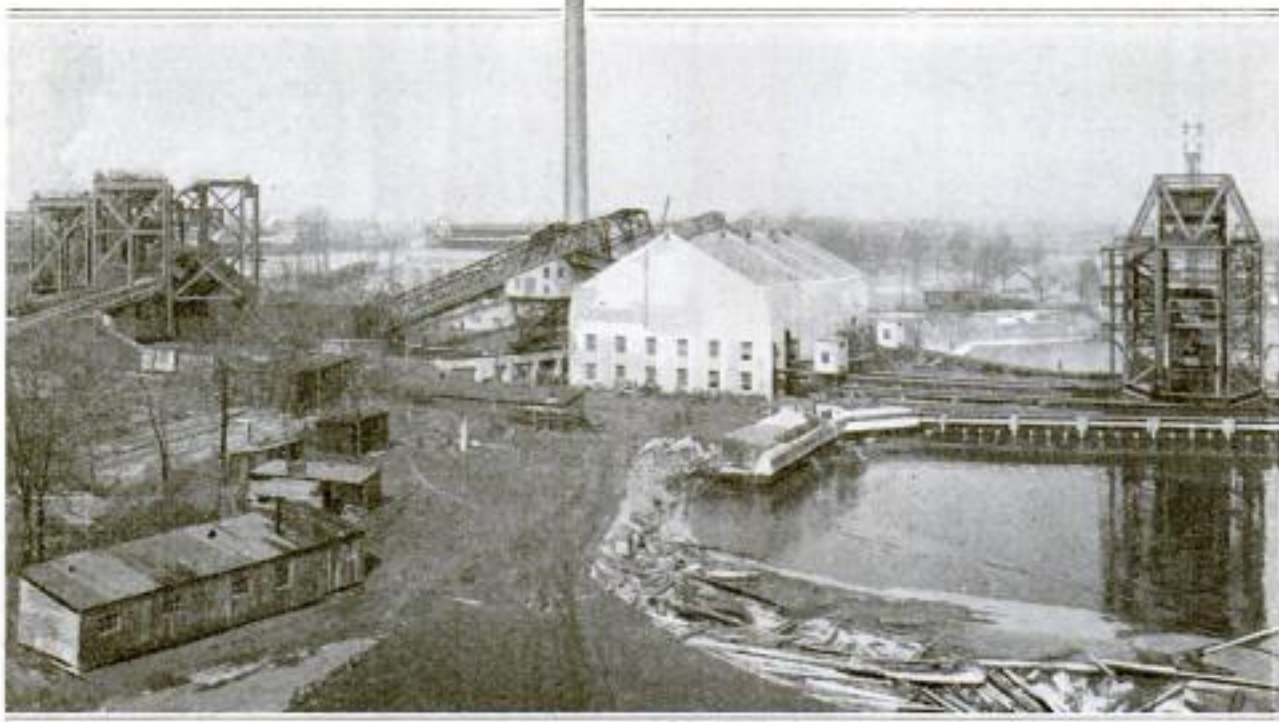
New Coal Pier near Baltimore Which Has a Capacity of 7,000 Tons per Hour: With the Four Loading Towers Vessels with Bunker and
