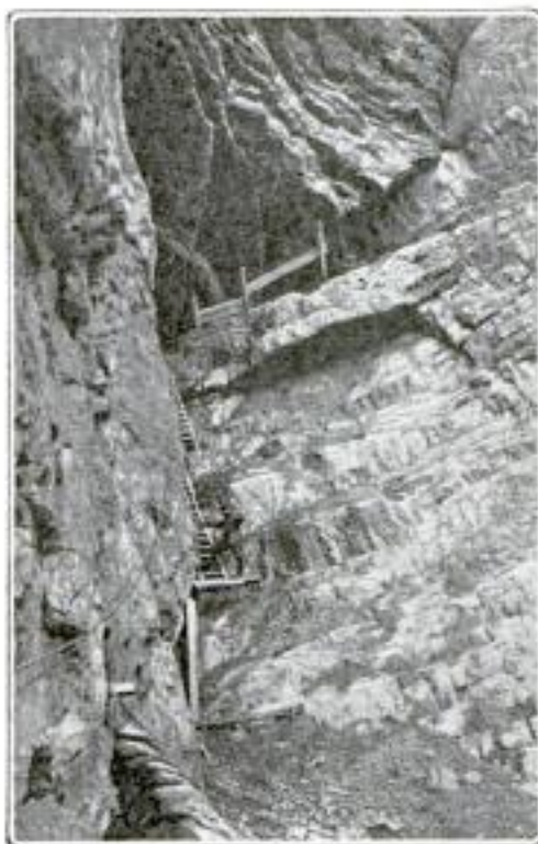
Ladders and Stairs Leading to the Mouth of the Tunnel
