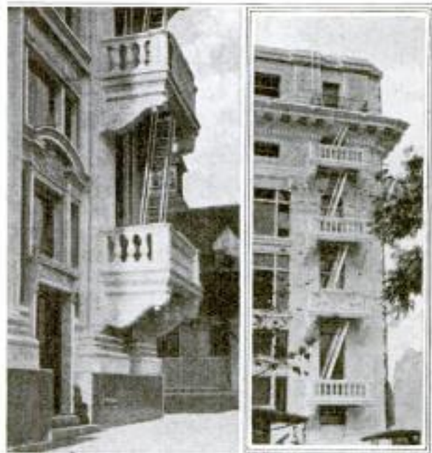
Two Views of the Fire Escape on a New Building in Los Angeles, so Designed as to Be Truly Ornamental
