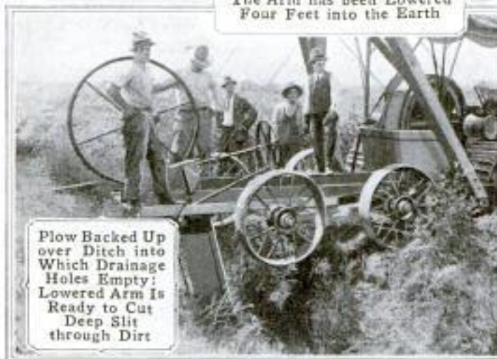
Plow Drawn by Three Tractors: The Arm has been Lowered Four Feet into the Earth
