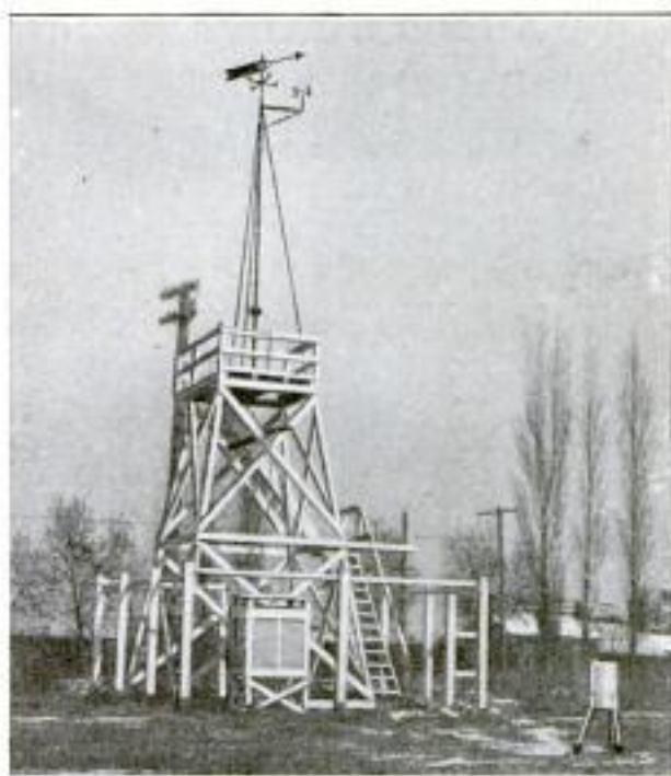
Weather Station Maintained by a Western Smelting Company: Here Records are Kept Which Often Aid in Determining the Justness of Claims Based on Alleged Damage to Near-By Property
