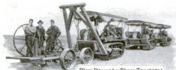
Plow Drawn by Three Tractors: The Arm has been Lowered Four Feet into the Earth
