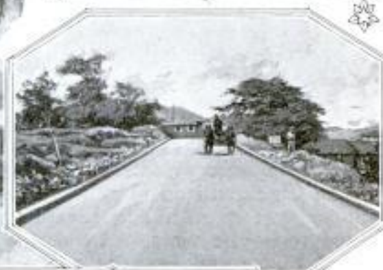
One of the Recently Finished Asphalt Streets at Balboa: With a Base of Broken Stone, Layer of Macadam, and Surface of Asphaltic Concrete, They Stand the Tropical Rains Well
