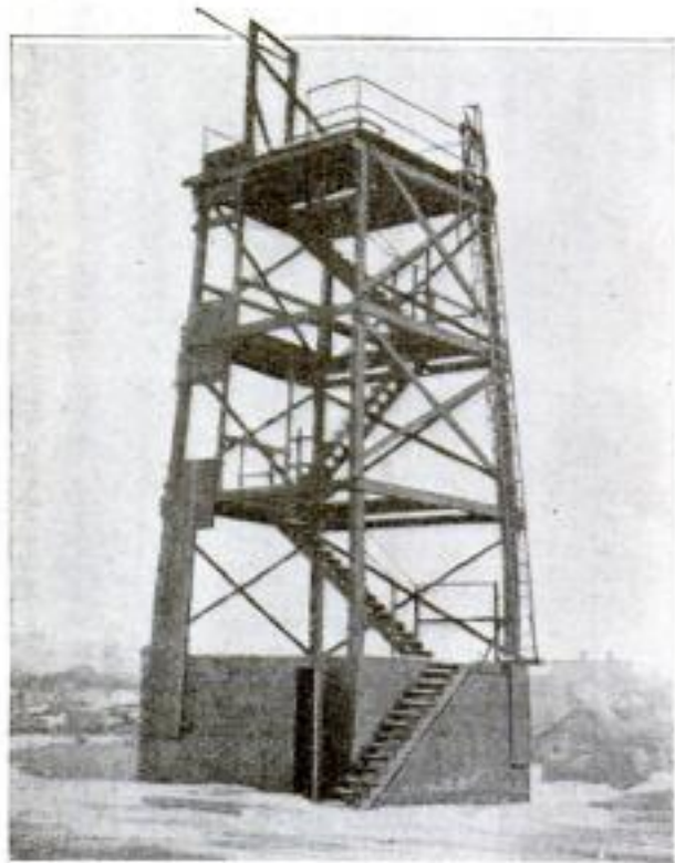
Firemen's Practice Tower in Pueblo, Colorado, with a Room That is Occasionally Filled with Smoke so That the Men can Practice Rescue Work
