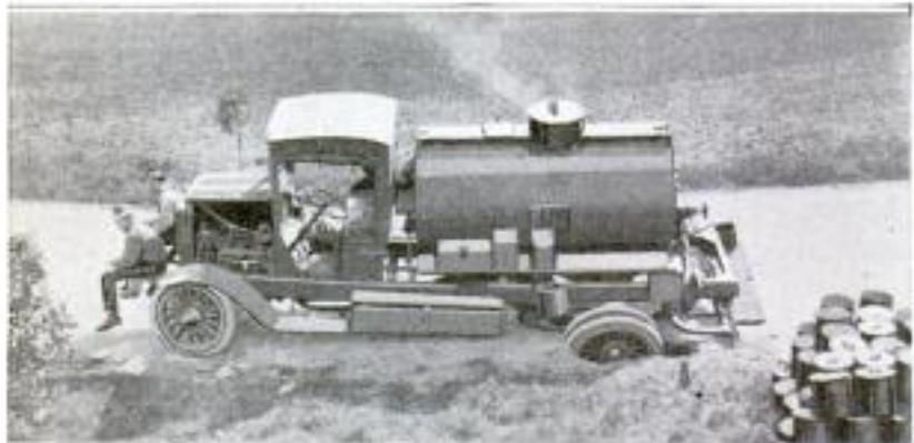
Twelve-Ton Oil-Laden Truck with Wheel Sunk through a Paved California Roadway
