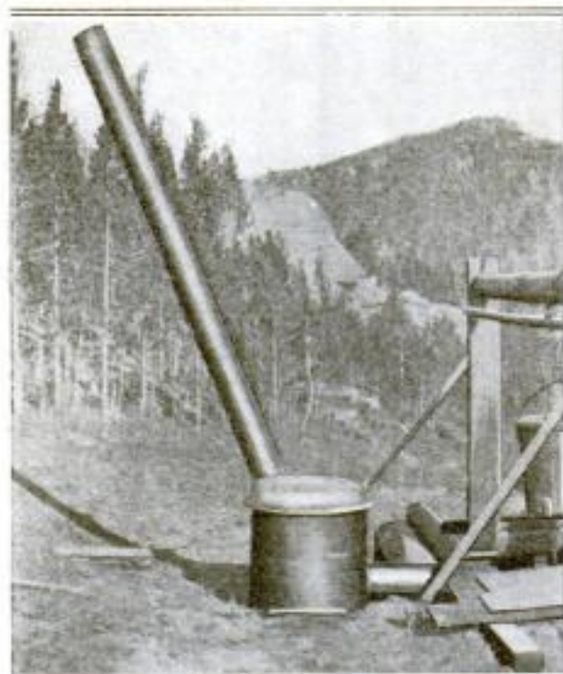
Ventilating a Prospect Hole by Means of a Stove: The Shaft beneath the Windlass in This Photo Is 60 Feet Deep
