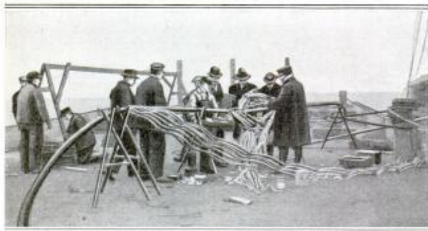
Splicing Ends of the Big Cable While the Scow Lay in the River
