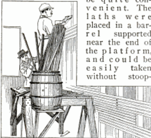
The Rapid Work of the Lather is Made Even More Speedy by the Use of This Stand
