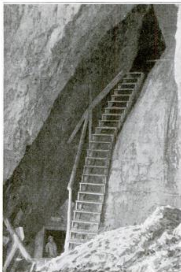
Left: Portion of Stairway inside the Tunnel. Much of the Tunnel was Driven on a Gradient of Over 45 Degrees. All of the Explosive and Much Material had to be Carried up This Stairway on the Backs of Men. Right: Natural Fissure in the "Castelletto" Encountered by the Tunnel of the Mine. Fumes Rising through a Similar Fissure Gave the Italians Warning of the Direction of an Austrian Countermine
