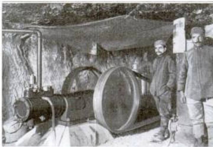
One of the Air Compressors in a Chamber of the Tunnel: The Two Italian Engineers Are of the Enduring Type That Made the Feat Possible
