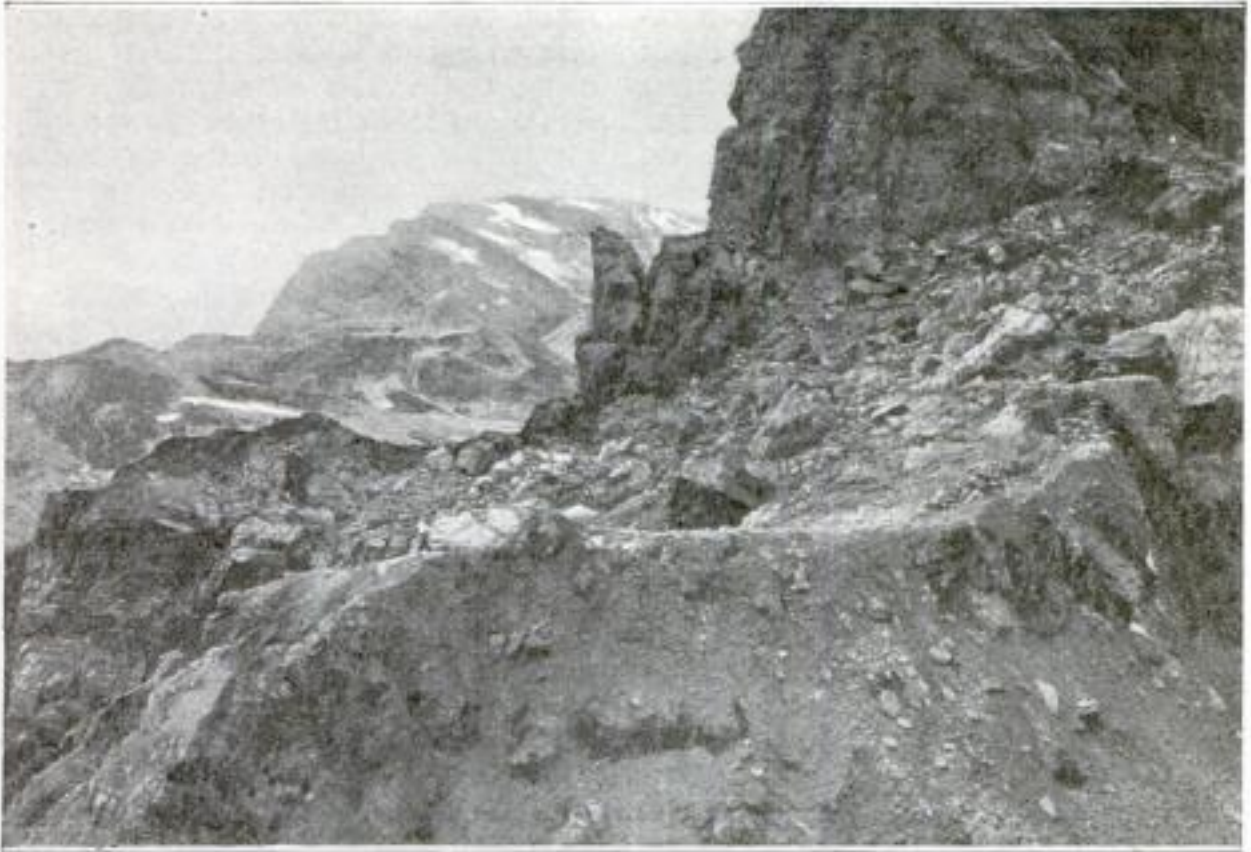
Portion of the "Castelletto" Crater Formed by the Mine Which the Italian Engineers Exploded from Their Tunnel Far Below
