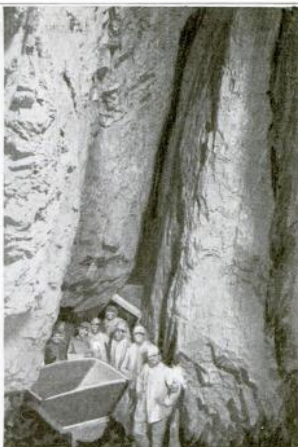
Left: Portion of Stairway inside the Tunnel. Much of the Tunnel was Driven on a Gradient of Over 45 Degrees. All of the Explosive and Much Material had to be Carried up This Stairway on the Backs of Men. Right: Natural Fissure in the "Castelletto" Encountered by the Tunnel of the Mine. Fumes Rising through a Similar Fissure Gave the Italians Warning of the Direction of an Austrian Countermine
