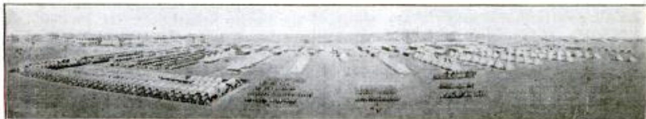
Aerial View of Motor Truck Group at Ft. Sam Houston, Texas. Major F. H. Pope, Cavalry, Commanding
