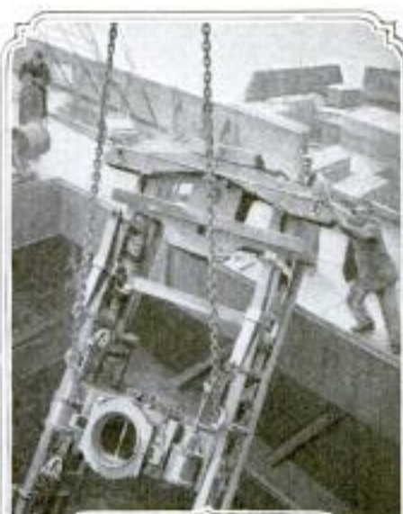
Lowering the Underframe of One of the Electric Giants into the Hold of a Freighter in New York for the 40-Day Voyage to the Chilean Port
