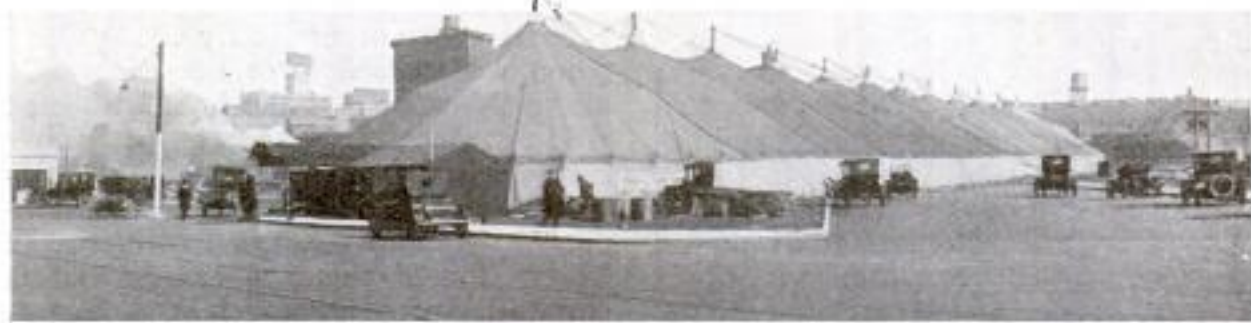
Big Tent of Paraffined Khaki Canvas, Covering More than 42,000 Square Feet, Used to House a Tractor Show in Kansas City, Missouri
