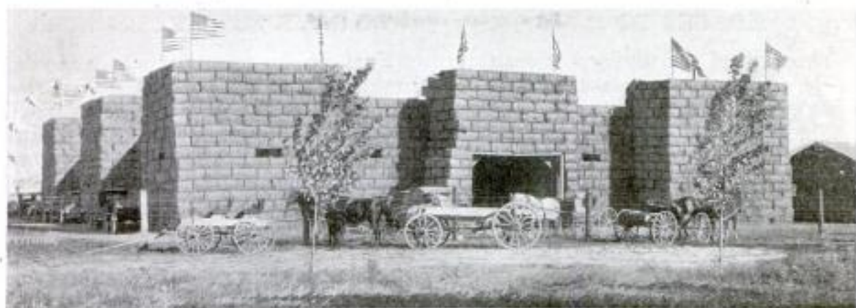
Unusual Structure Made from 600 Tons of Baled Alfalfa, in Which Washington Farmers Held Their Country Fair. The Walls Were 25 Feet High and the Building was Electrically Lighted
