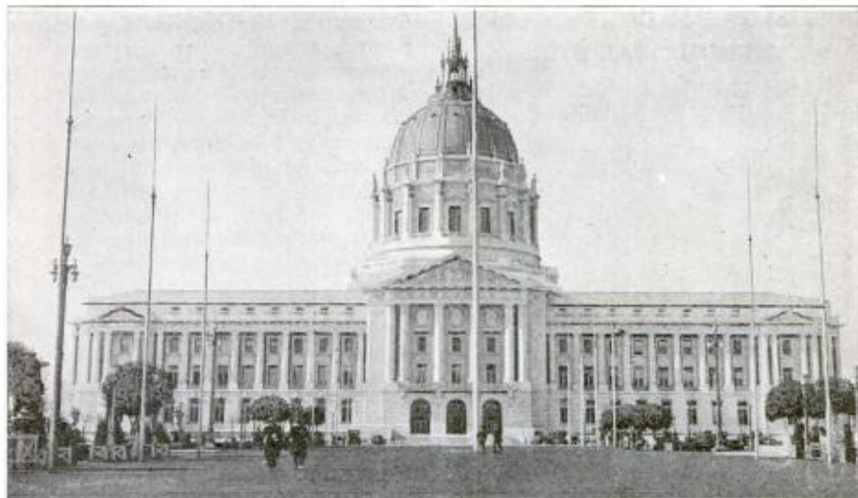
San Francisco's New Edifice Housing the City and County Offices, Which with Its Site Cost Nearly $5,000,000; The Building Measures 420 by 285 Feet and the Dome Is 306 Feet High. The Exterior is Finished in White Granite, While Bedford Stone and Marble have been Used Extensively on the Interior
