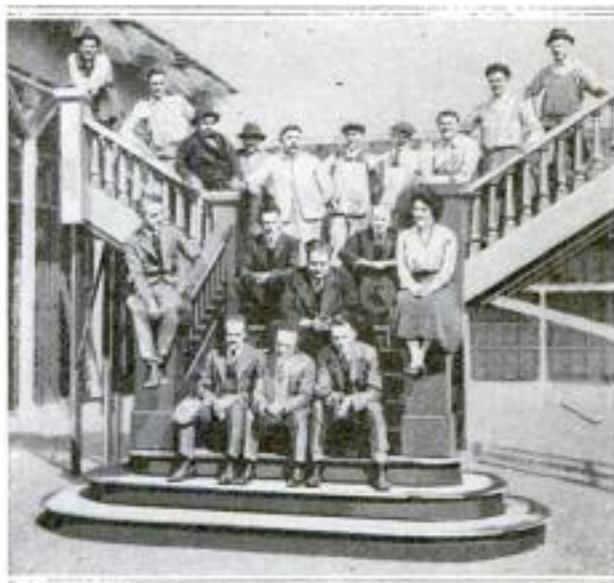
This Demountable Staircase, Used for Various Purposes in a Motion-Picture Studio, was Set Up in Seven Minutes
