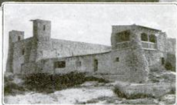
Old Indian Mission Church at Acoma, New Mexico, Which was Copied in Many Particulars in Designing the New Museum Shown Above
