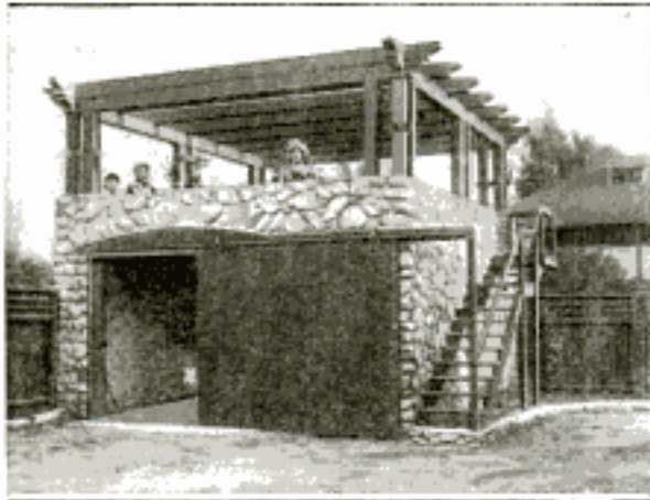
The Roof of the Garage was Fitted Out as a Useful Play Area and Recreation Spot
