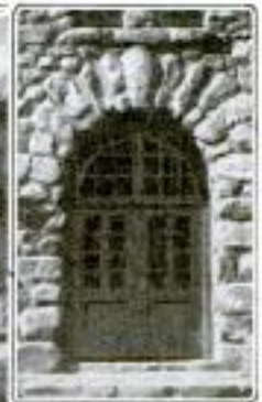
The Main Entrance, Showing How Even the Arches and Steps were Built of Bowlders
