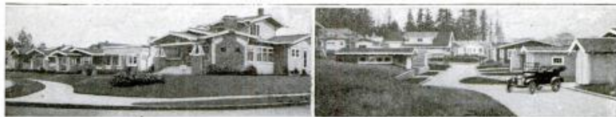
All Houses in This Block Have Garages Facing on a Common Artistic Driveway, Thus Avoiding the Necessity of Private Entrances. Right: Paved Driveway on Which All Garages in the Block Face
