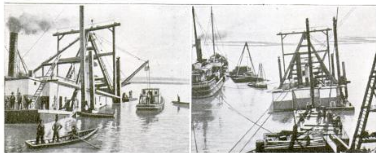
Left: View of Sunken Dredger, Which was Pumped Out by Another Dredging Craft, Showing the Elevated Stern under Which Divers Sawed Off Piling. Right: This Shows the Rescuing Vessel at the Scene; Also the Large Suction Pipe Running to the Wreck, and Diving Operations at the Stern
