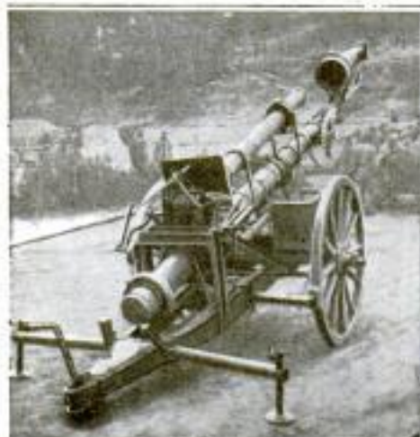
A Powerful Land Periscope, Captured by the French from the Germans, Which can be Reared to a Height of 80 Feet. It is Shown Extended at the Right, and at the Left Collapsed, in Which Position It Closely Resembles an Ordinary Field Gun
