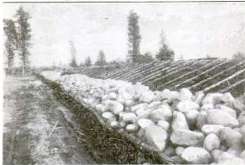
An Alaskan Inland Breakwater, for the Protection of Farming Lands from a Deluge of Glacier Waters: Such Breakwaters are Constructed by the Government for the Benefit of Settlers
