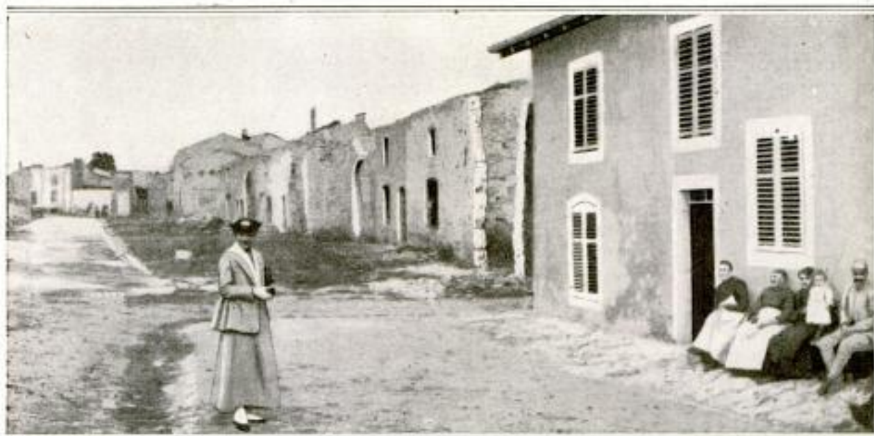
San Francisco, is Supervising the Rebuilding of Vitrimont, a Village near Nancy. The Work is Financed by a Great Earthquake and Fire in 1806, and the Period Following
