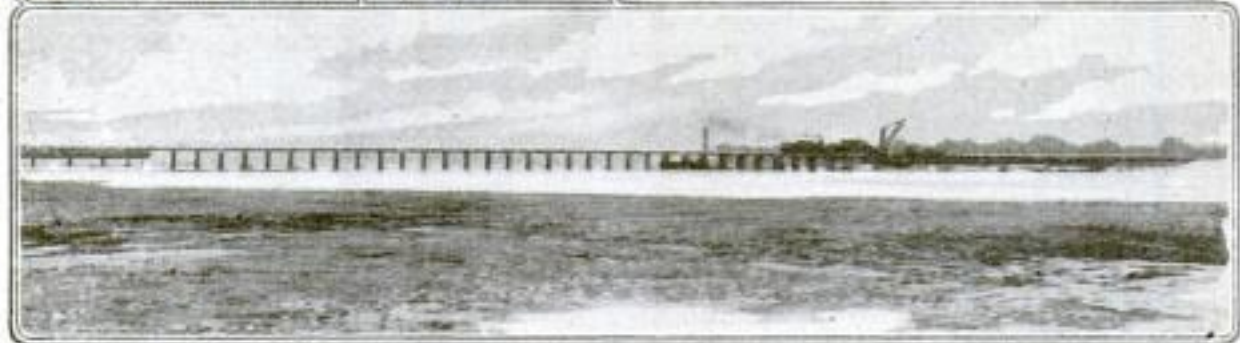
General View of Bridge across Platte River at Yutan, Nebraska, Showing Girder Spans at Either End and 700 Feet of Trestle in the Center. Above, Left, Temporary Bridge from Which Material was Supplied for the Construction of Concrete Piers; Right, Pneumatic Caisson in Operation, Showing the Pipe through Which Sand and Dirt is Forced Up from Below
