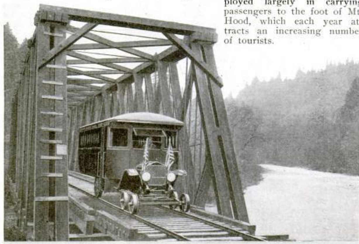
Thirty-Passenger Auto Bus, with Four-Wheel Truck in Front, Built to Run on a Standard Railway Track in the Hood River Region in Oregon
