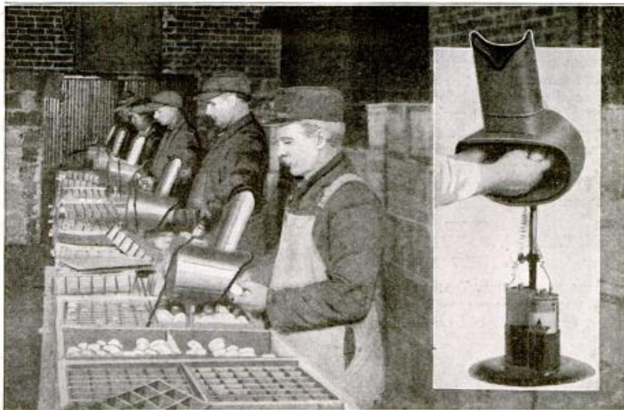
Grading Eggs with a New Candling Device That can be Used in a Lighted Room or Out of Doors, Doing Away with the Insanitary and Sight-Destroying Dark Room in Produce Houses: An Inclosed Electric Light Illuminates the Eggs
