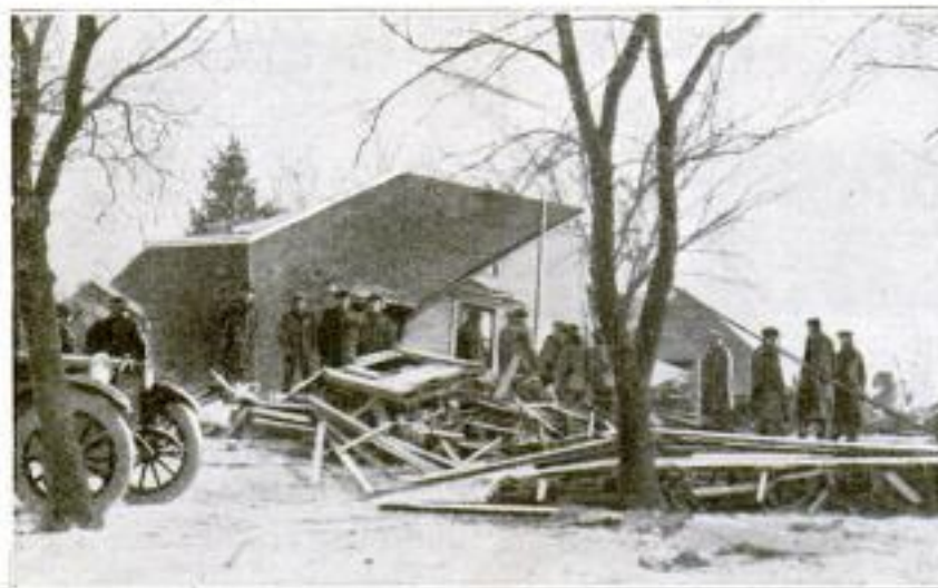
This Farmhouse Wreck was Caused by an Explosion of Leaking Gas from an Acetylene Plant in the Basement, Three Persons being Killed
