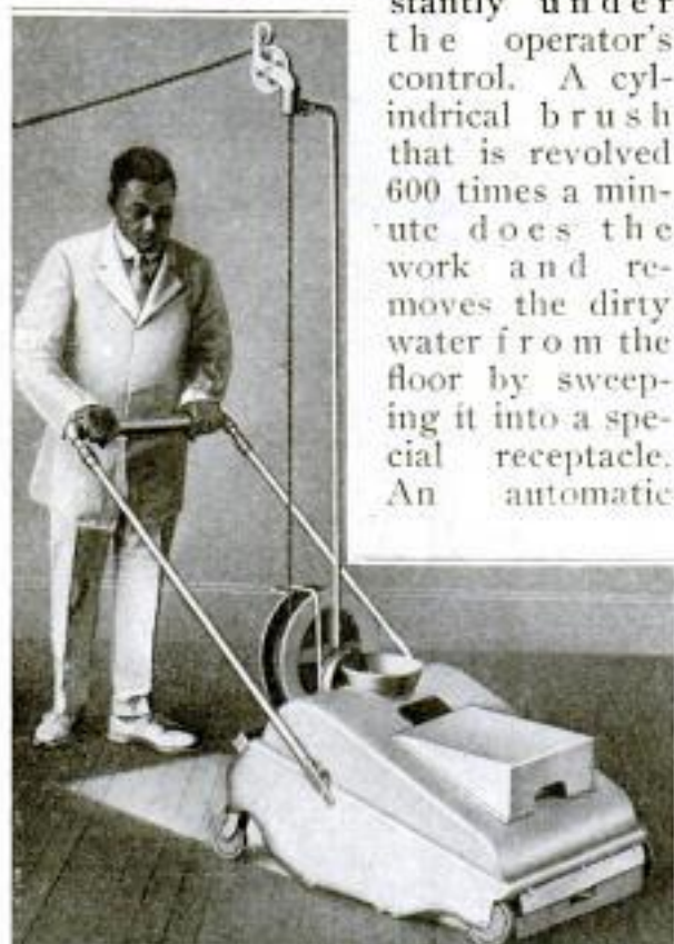
This Machine Sweeps and Scrubs a Floor in a Single Operation and Does Its Work Rapidly
