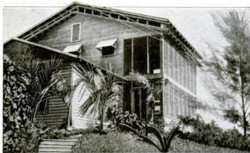
A Javanese Style of Architecture Introduced in Florida: Note the Double Roof and Large Screened Porches on Three Sides
