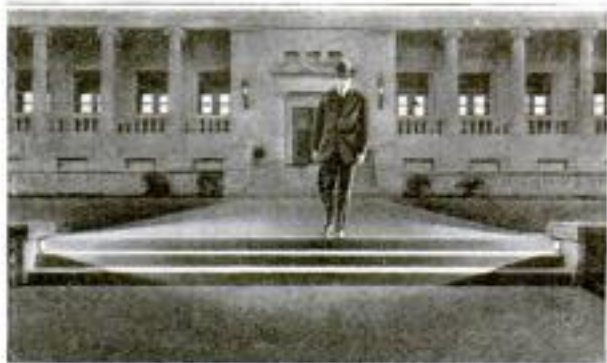
Three Steps in Front of the Alhambra, California, Public Library Which are Well Illuminated at Night by Lights Recessed in Stone Abutments Either Side of the Walk
