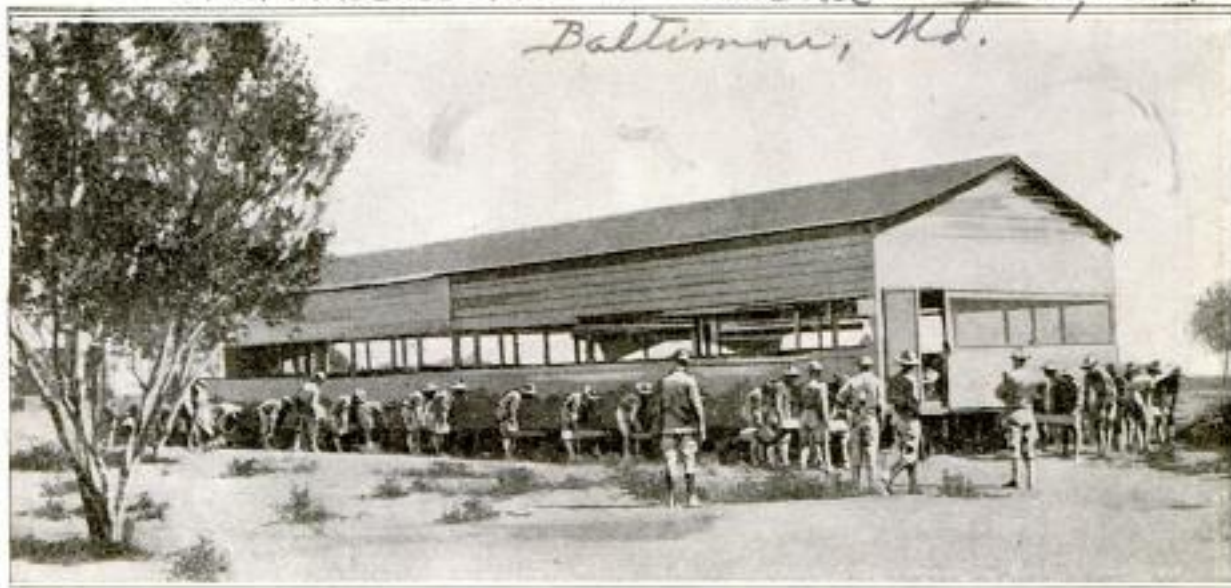
Two Hundred and Fifty North Dakota Troopers at Mercedes, Texas, Carrying the Christian Association Building, Weighing Six Tons, to a New Site
