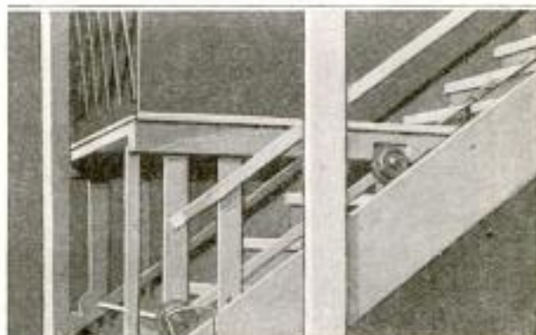
Stair-Climbing Elevator. Just After It has Left the Lower Floor Level, Where It Normally Rests Out of the Way
