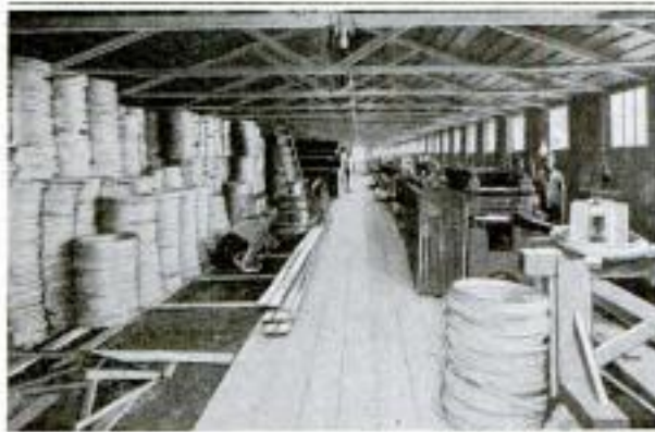
Interior of Factory Building of Steel Sections Rapidly Put Together: Note the Plan of Roof Construction and Method of Lighting by Window Panels.
