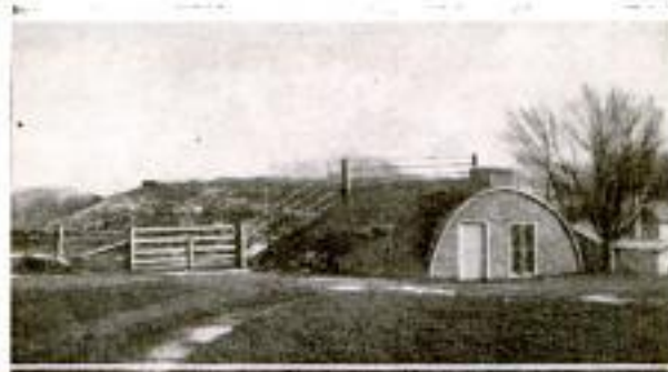
Farm Building, 72 Feet Long, with Barrel-Arch Roof of Reinforced Concrete. The Wooden Form for the Curved Portion has been Retained to Give It Added Strength
