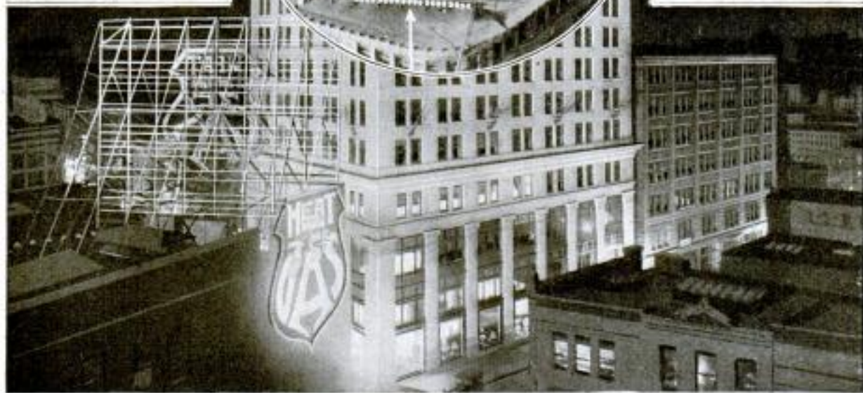
Twenty-Story Building in Baltimore Flood-Lighted by Batteries of Lamps Located on the Roofs of Buildings across the Street. Insert Shows Batteries of Electric Lamps and Reflectors Installed on the Roof of a Low Building on the Opposite Side of the Street from the Skyscraper
