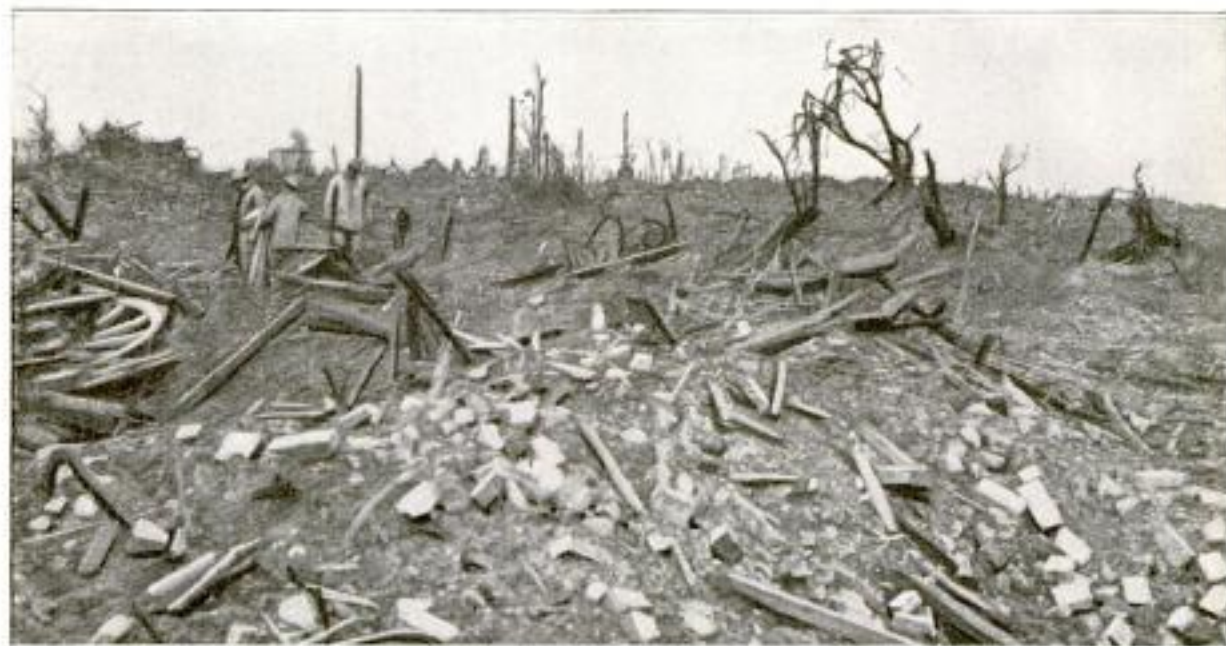
The Remains of a Village on the Somme: This Is One of the Extreme Instances Mentioned by Mr. Freeman. The Very Bricks and Stones are Pulverized, and It Is Not Probable That Any of the Old Material can be used in Rebuilding
