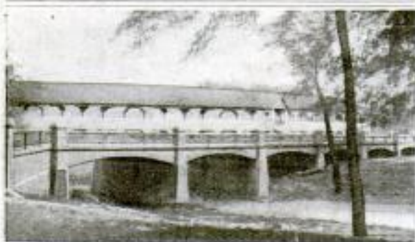
New Concrete Bridge Built to Divert Farmers from the Grounds of an Indiana Resort: Baseball Grand Stand in Background
