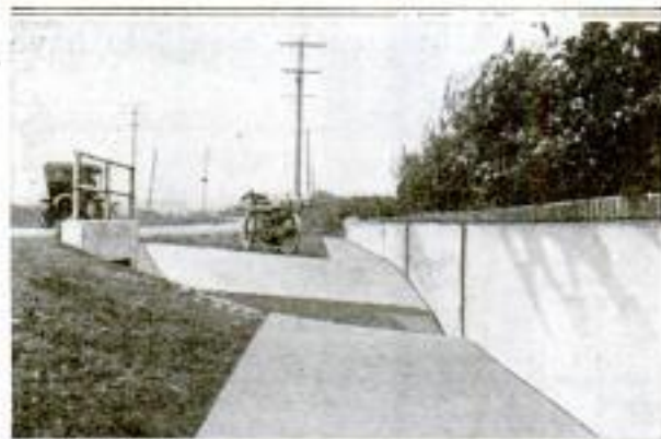
Barrier Erected at the Side of a California Lemon Orchard Which Serves as a Fence and Gutter, and as a Dam That Holds Back Occasional Flood Waters
