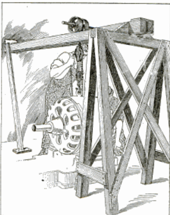
This Support for Differential Tackle was Devised in an Emergency for Taking Down a Generator
