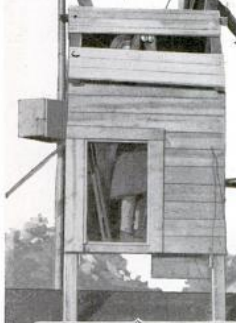
Lookout Tower on Top of a Hangar. An Observer with Binoculars is Stationed Here Whenever Flights are Made. He Summons the Ambulance in Case There is an Accident, and Dispatches a Mechanician When Motor Trouble Occurs
