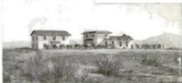
Top: Distant View of New Naval Radio Plant at San Diego, California, Showing the Huge Towers. Left: Concrete Base of One of the Towers; Insulation Plates of Porcelain Are Visible below the Steel. Right: The Building on the Right Houses the Engine and Generator, While the One on the Left Contains the Transmitting and Receiving Instruments
