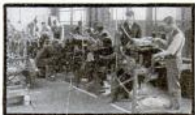
Block Testing and Motor Department
