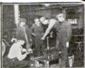
We teach the newest and best way to re-bore cylinders as a part of the complete Auto Course. No need to have big, heavy, expensive machines. This is very important instruction.
