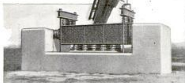
Top: Distant View of New Naval Radio Plant at San Diego, California, Showing the Huge Towers. Left: Concrete Base of One of the Towers; Insulation Plates of Porcelain Are Visible below the Steel. Right: The Building on the Right Houses the Engine and Generator, While the One on the Left Contains the Transmitting and Receiving Instruments
