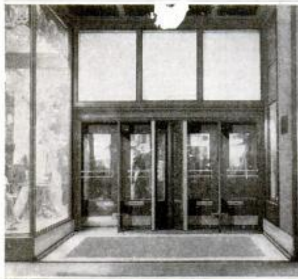
At the Right, a Chicago Window Display as It Appears at Night When the Store is Closed. At the Left, the Vestibuled Entrance in the Space Occupied during the Night by the Disappearing Show Window. Note the Floor, Which Rises with the Ascending Window Display in the Evening
