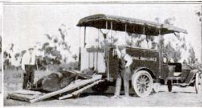
Left: Rolling a Hobbled Horse onto a Wheeled Platform with the Aid of the Rope and Windlass, the Latter Shown in the Inset. Right: Drawing the Wheeled Platform and Its Burden into the Car
