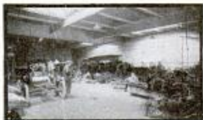
"Y" Auto School Repair Shop
