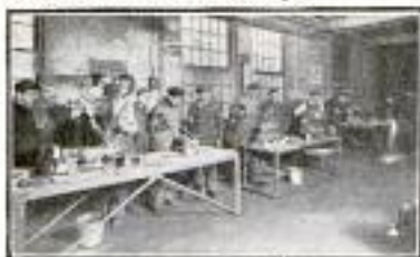
This is a section of the Brazing, Welding and Cutting Department. Each man handles the torches and works with an individual outfit.
