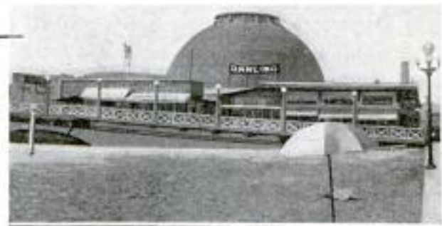
Hollow Hemisphere of Concrete Used as a Dance Hall at a California Ocean Resort
