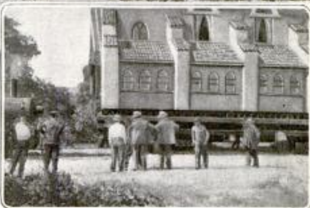
Two Views of an Old Church in South Bend, Indiana, being Drawn Five Blocks to a New Site by a Freight Engine
