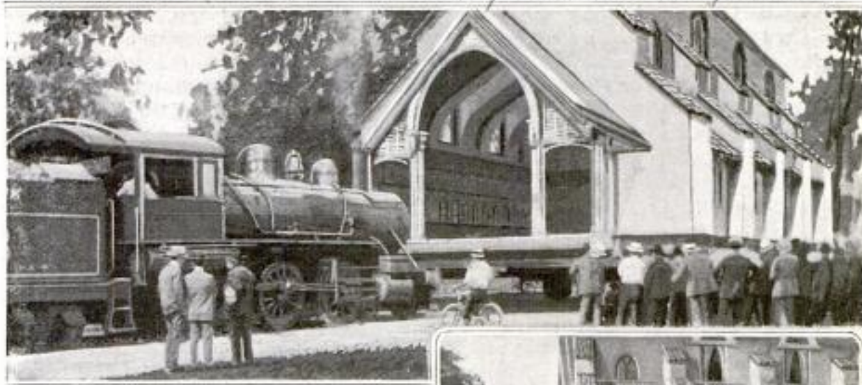
Two Views of an Old Church in South Bend, Indiana, being Drawn Five Blocks to a New Site by a Freight Engine
