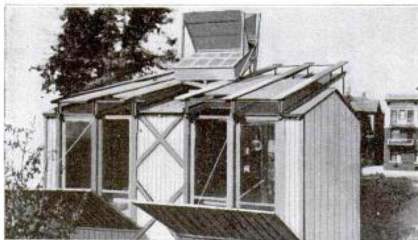
Solarium Mounted on a Circular Track so That It can be Made to Face the Sun All Day Long. In It Patients are Given Sun Baths Followed by Shower Baths in Sun-Heated Water
