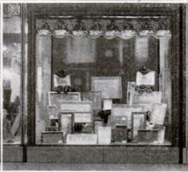
At the Right, a Chicago Window Display as It Appears at Night When the Store is Closed. At the Left, the Vestibuled Entrance in the Space Occupied during the Night by the Disappearing Show Window. Note the Floor, Which Rises with the Ascending Window Display in the Evening
