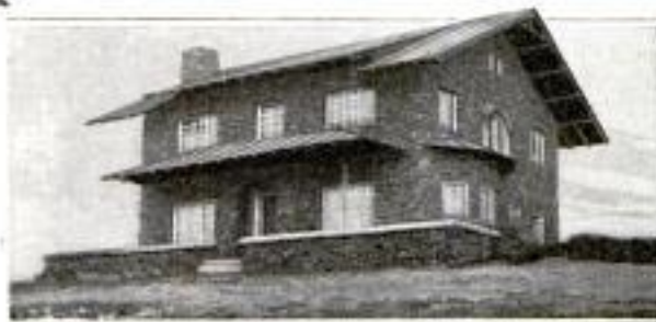
This House, Modeled after a Swiss Chalet, Contains a Large Quantity of the Precious Metals in the Quartz Rock of Its Walls and Foundation
