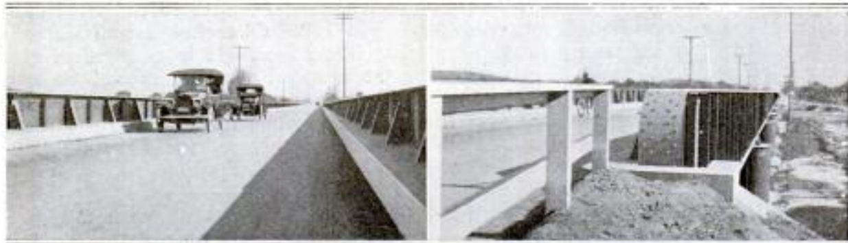
Left: Note the Wide Curb That Prevents Cars from Running Too Close to the Heavy Railings. At the Right are Shown the Steel Girders of the Bridge Extended above the Floor Level to Form the Side Railings
