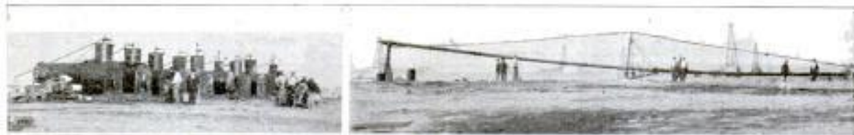
Left: Battery of Nine Boilers Installed on Field to Develop Steam with Which to Combat the Flames. Right: The Heavy Iron Cap was Moved Forward by Horses and Placed over the Well, Snuffing the Blaze and Controlling the Flow
