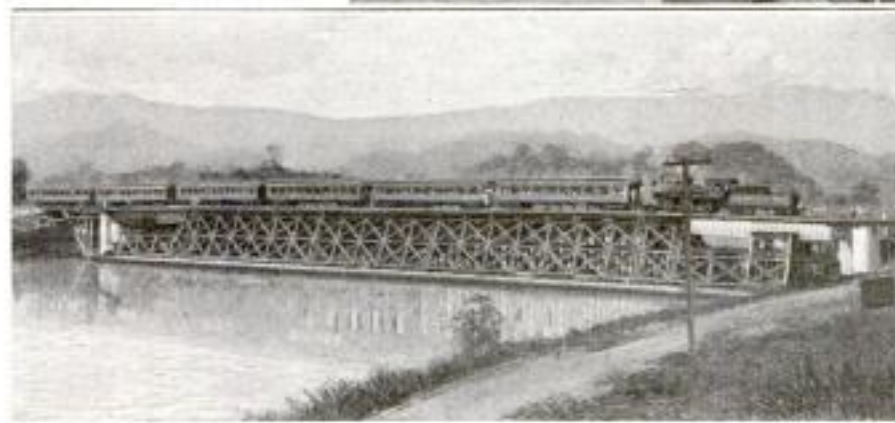
The Floating Bridge Accommodates Railway Traffic between Opposite Banks of the Canal at Paraiso. When Opened, It is Swung Out of the Channel into a Recess
