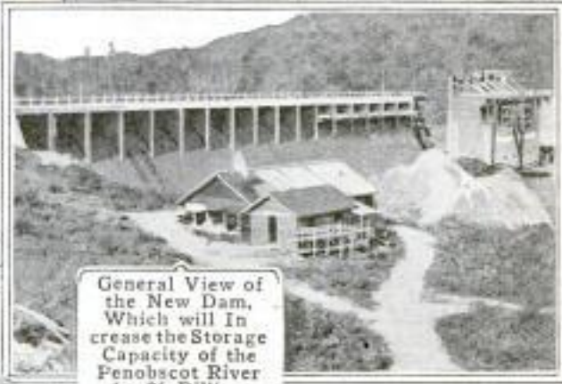
This Shows the Old Ripogenus Log Dam in the Foreground, and the New Cement Structure Rising in the Rear. The Old Dam will Be 60 Feet under Water When the New Lake or Reservoir Fills Up
