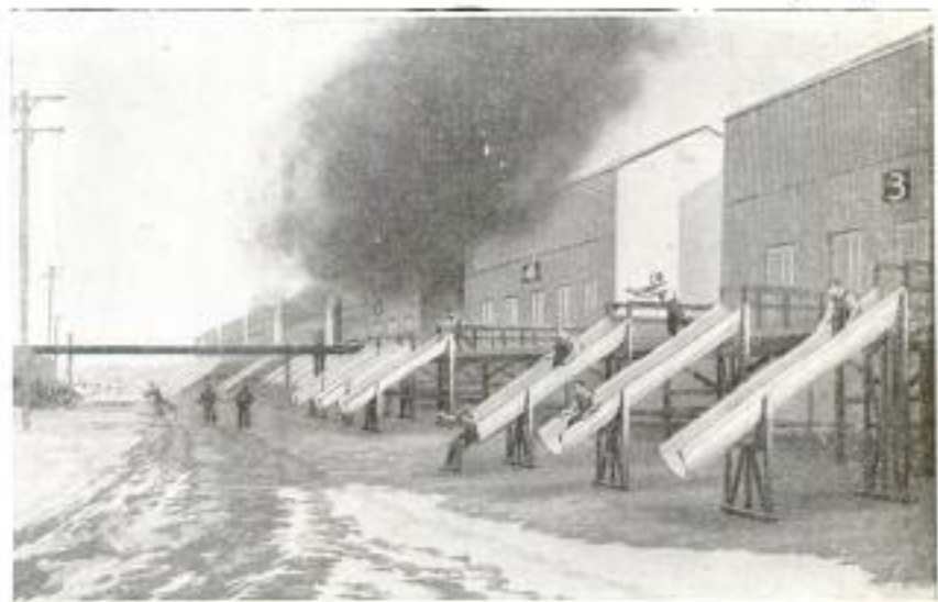
View of Smokeless-Powder Plant at Carney's Point, New Jersey. Showing the Large Metal Chutes Which Serve as Fire Escapes for the Workmen
