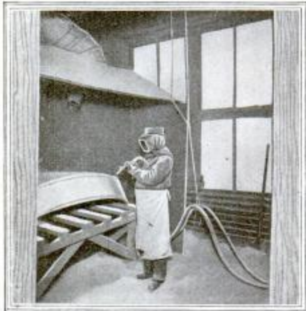
In This Old Method of Sand-Blasting the Workman can Lay Aside the Safety Helmet When He Chooses and Still Do the Work, Though at the Peril of His Health through Inhaling Particles of Sand
