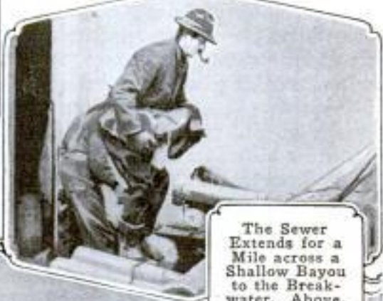
Whittling a Hole in the End of a Dynamite Stick Preparatory to Inserting a Percussion Cap: An Operation That Curdles the Blood of the Inexperienced, but Which is Really Not Dangerous at All
