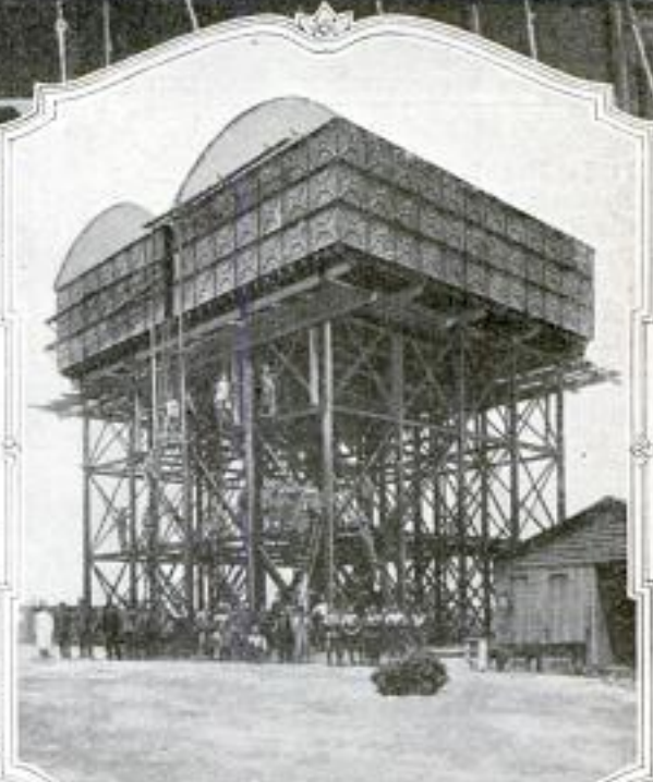
The Photograph Above Shows One of Several 100,000-Gallon Tanks Installed by the British at Military Camps at Home, in France, and in Belgium. It Indicates How England is Meeting the Perplexing Problem of Supplying Her Troops with Water
