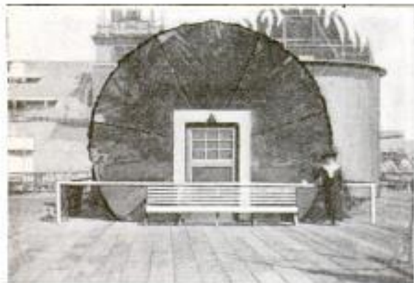
This Queer-Looking Structure Consists of Two Massive Redwood Logs, Hollowed and Joined Together
