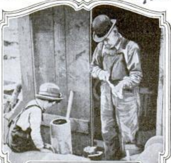
Whittling a Hole in the End of a Dynamite Stick Preparatory to Inserting a Percussion Cap: An Operation That Curdles the Blood of the Inexperienced, but Which is Really Not Dangerous at All
