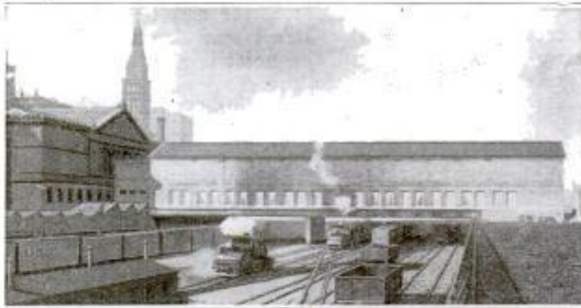
New Addition to the Chicago Art Institute, Which Extends across Several Railroad Tracks and Has a Framework Very Much Like a Steel Bridge
