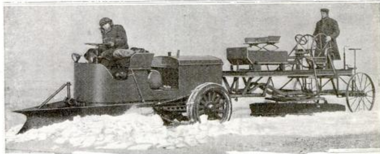
Electric Tractor Carrying a Snowplow and Hauling a Street Grader on Michigan Avenue, Chicago, after a Snowstorm This Winter: The Man Behind Raises and Lowers the Grade Plow as Required; in Front of Him Is the Seat of the Team Driver, the Grader being Usually Drawn by Horses
