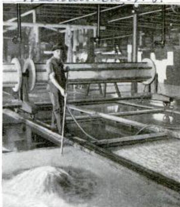
Stirring the Contents of a Tannery Vat with Compressed Air: Air is Forced through the Pipe Held by the Workman at a Pressure of 90 Pounds and Agitates the Fluid More Thoroughly Than could be Done by Hand
