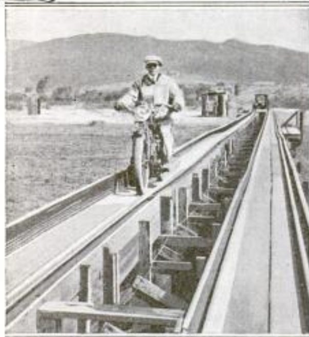
This Temporary Double Trestle Serves as a Railway Bridge across the Mexican Border. Note the Rails on Either Side of the Open Center
