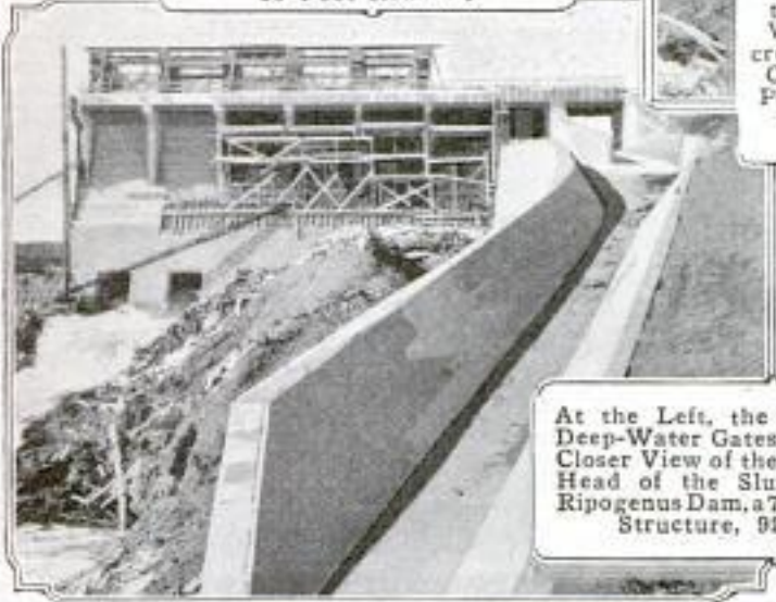
Section of Front of the New Ripogenus Dam: The Cement Walls Seen Rising from the Face of the Dam Support a 16-Foot Roadway
