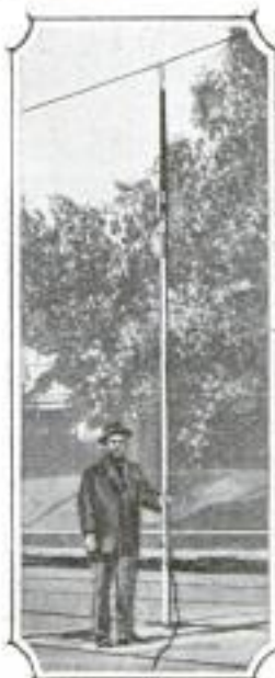
Roller Used on the Streets of St. Louis Which Derives Its Power from a Near-By Trolley Wire, View at Left Showing How the Cable is Attached to the Trolley Wire
