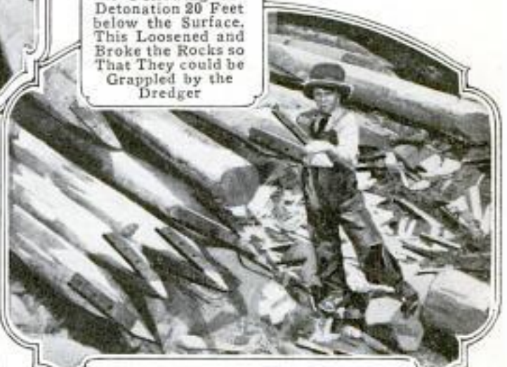
After Enough of the Rocks had been Removed to Permit It, Steel-Pointed Piles were Driven to Form a Foundation. The Conduit Is 10 Feet in Diameter and Drains the Hilly Sections of San Francisco's North Side
