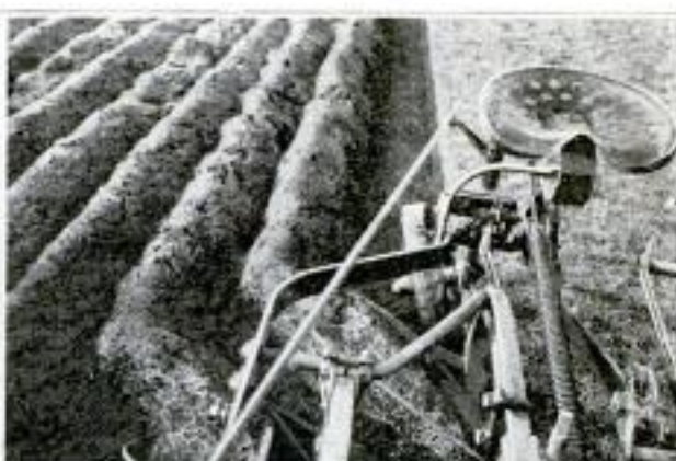
These Photographs Show the Evenness and Level Character of the Furrows Made by a New Plow That Works Equally Well When Drawn by Horses or by a Tractor
