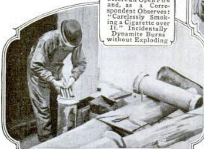
A Section of Sewer Pipe and Plenty of Dynamite Makes a Good Bomb. The Blasting was Done for the Purpose of Making an Opening in a Stone Breakwater at San Francisco through Which a Large Storm Sewer was to Reach the Bay.
