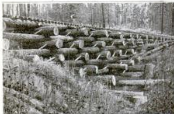
A Good Example of the Crisscross Type of Railway Bridges Erected in Many Regions of the West Where Lumber Was Plentiful and Skilled Labor Scarce
