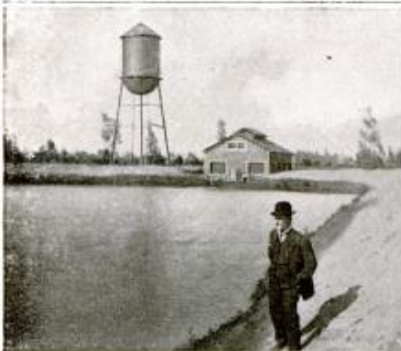
One of the Settling Basins at Brawley, California, into Which Silt-Laden Water is Run before being Pumped into the City's Water Tank
