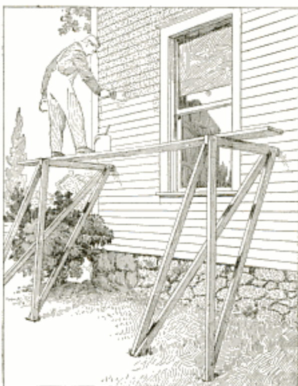
These Supports for a Scaffold Are More Convenient than the Use of a Ladder, Especially for Work at a Comparatively Low Height
