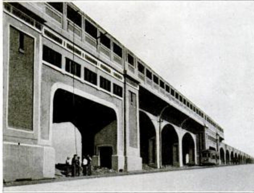
This Concrete Viaduct of Ornamental Design Carries Elevated Trains for a Mile along Queen's Boulevard, Long Island City, and Is in Striking Contrast with the Ordinary Elevated Steel Structure
