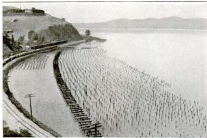
These Piles Are Practically All That is Left of the Great Wheat Elevators That Housed Much of California's Wheat Crop in Other Days
