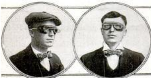
Goggles Which Are Open Directly in Front of the Eyes but Which Have a Projecting Wall of Celluloid That Protects Them Entirely from the Wind
