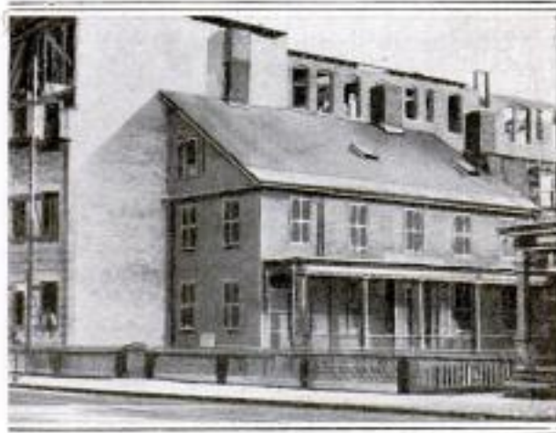
Old Frame Dwelling in Cambridge, Massachusetts, Which has been Cut in Two Lengthwise to Make Room for a Modern Brick Structure
