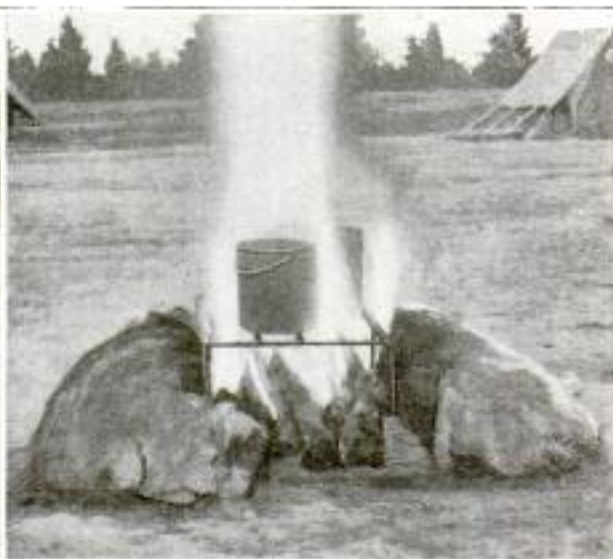
Camp Incinerator for the Disposal of Refuse, Constructed at the Training Camp of District of Columbia Troops, Fort Myer, Virginia
