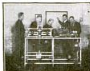
Complete working Delco System as used in Buick, Hudson, and Packard Twin "6."
