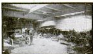
"Y" Auto School Repair Shop
