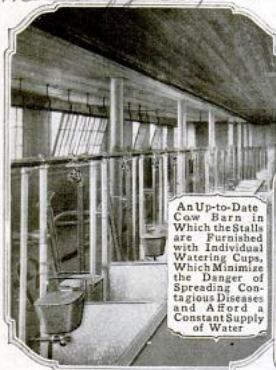
At the Right, an Individual Watering Cup with Its Feed Piping: The Level of the Water in the Cups is Kept Constant by a Regulating Tank and Valve. The Cow can Easily Open the Cup to Drink, but cannot Slop Out the Water
