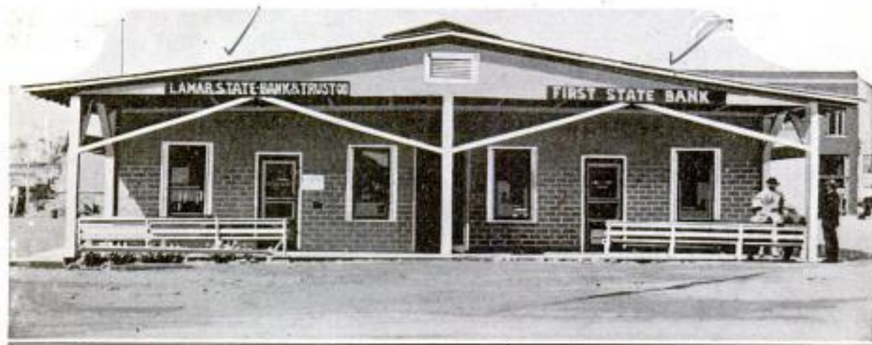
View of Temporary Building Erected after a Big Fire in Paris, Texas, to House Four Banks. The Single Brick Vault in the Structure Contained $4,000,000 in Cash at One Time
