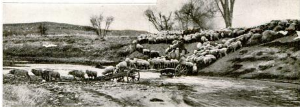
A Strikingly Beautiful Scene on a Ranch near Buffalo, Wyoming, Showing a Portable Bridge Made with Wagon Running Gear and Logs and Used in Getting Thousands of Sheep across Streams
