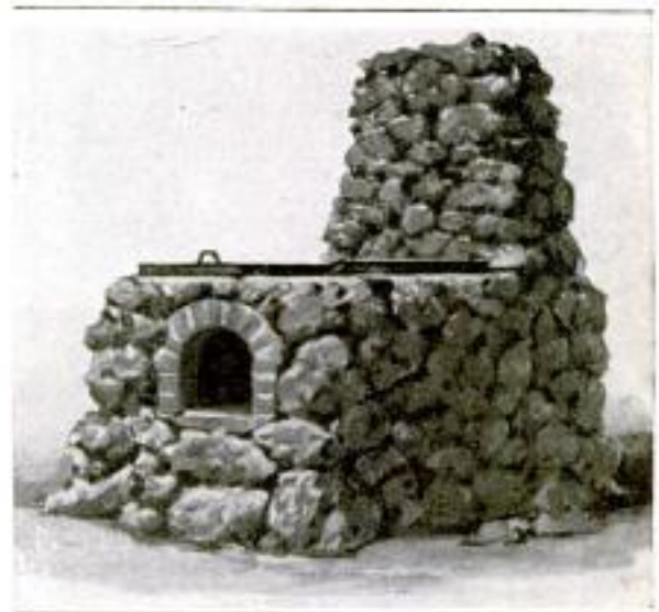
Substantial Stone and Brick Oven Erected on the Beach by the City of Santa Monica, California, for the Use of Picnickers in Warming Coffee or Cooking Meats
